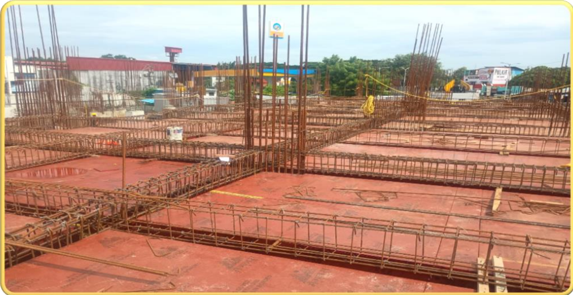
Main building – Pour 2 Stilt floor roof beam reinforcement work completed
