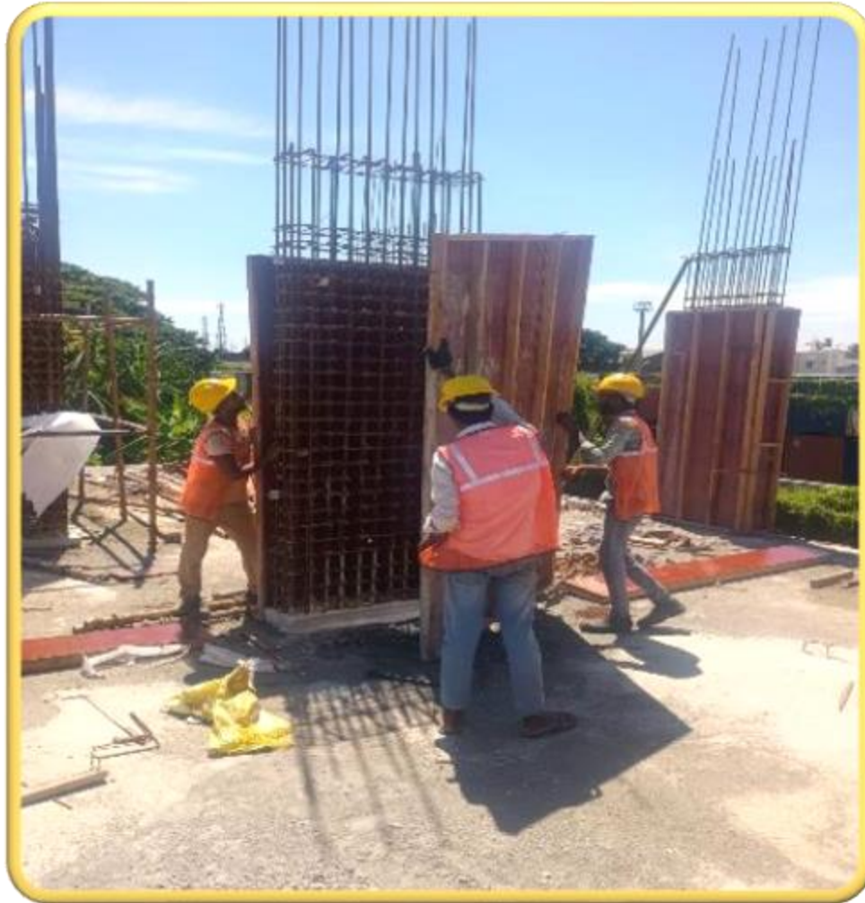
Main building – First Floor Pour 1 column Shuttering work
