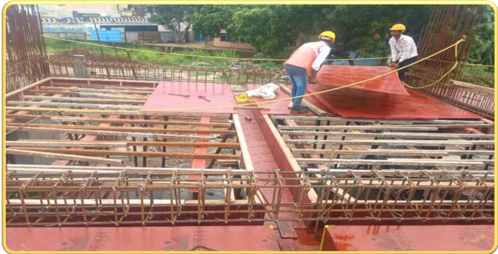
Main building – Stilt floor roof pour 2 slab shuttering work in progress
