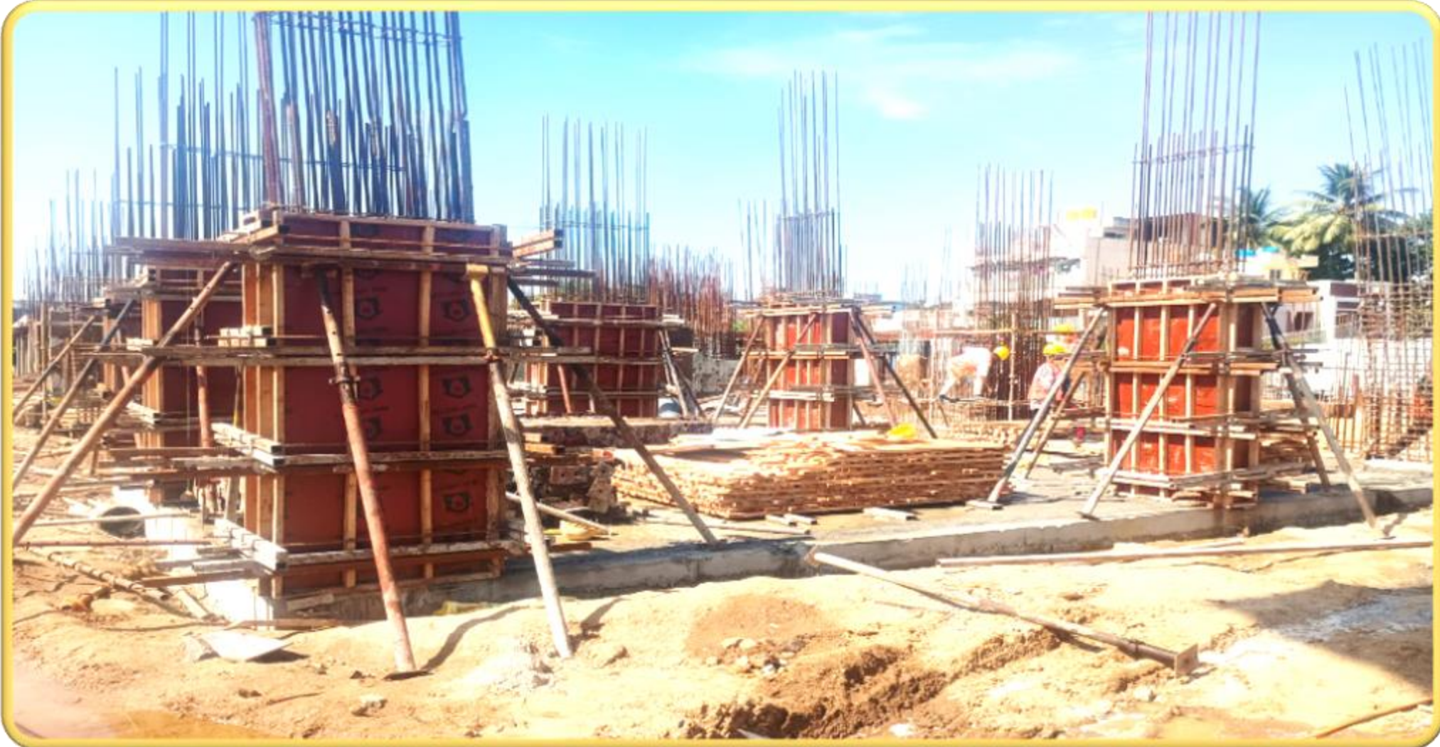
Main building – Pour 2 2 nd lift column shuttering work completed
