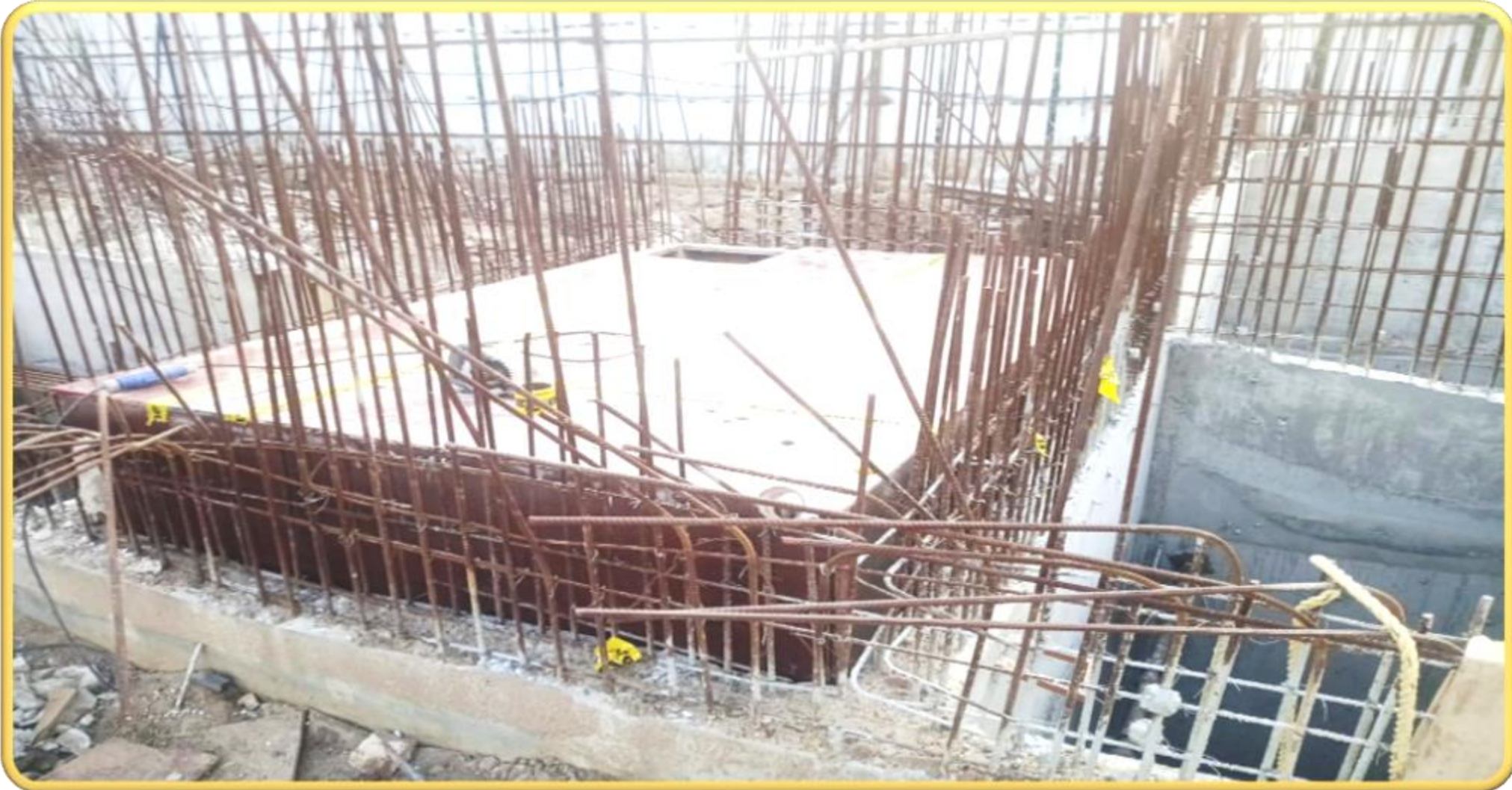
STP – Cover slab shuttering work in progress
