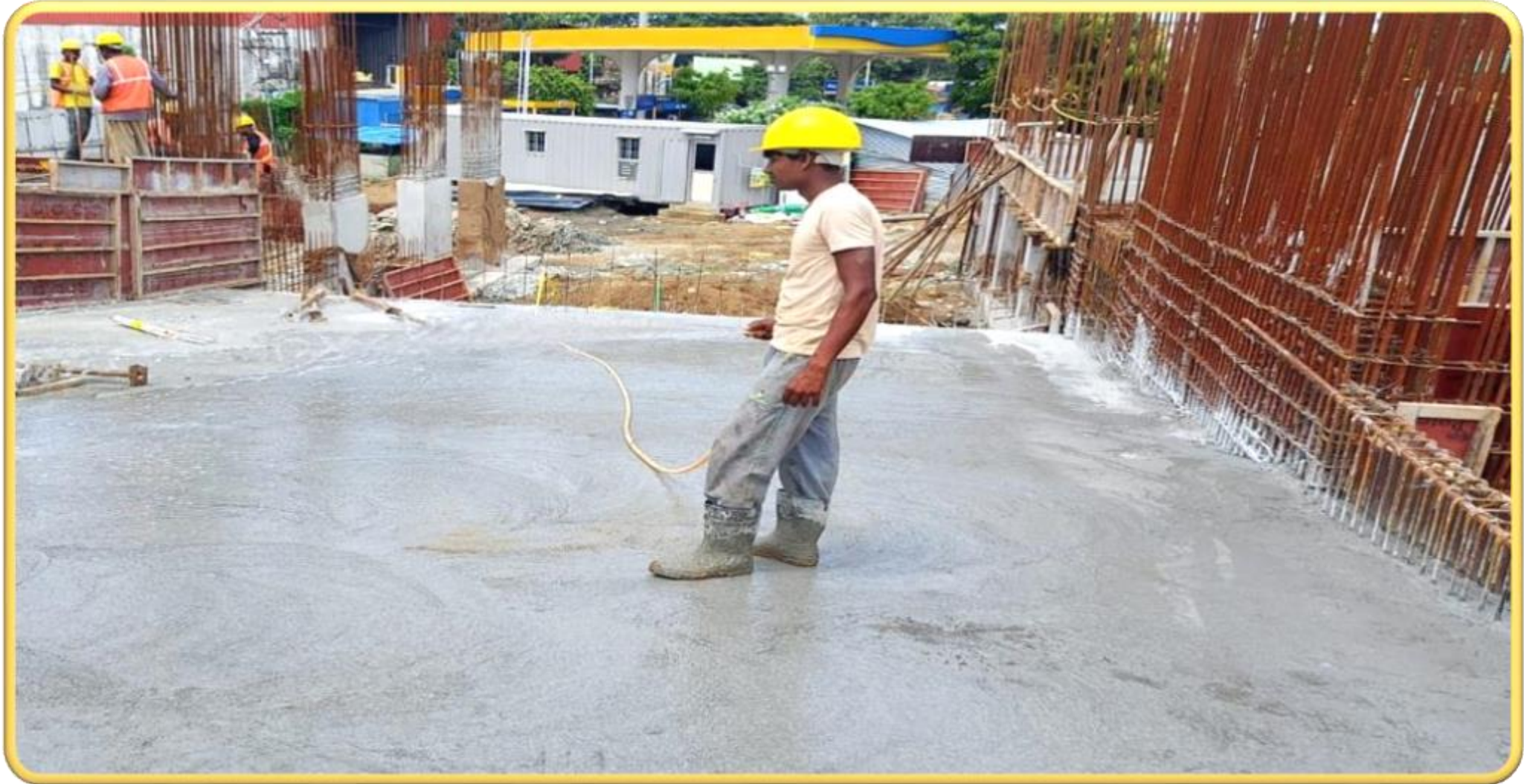
Main building – Ramp beam & slab concrete 50% completed
