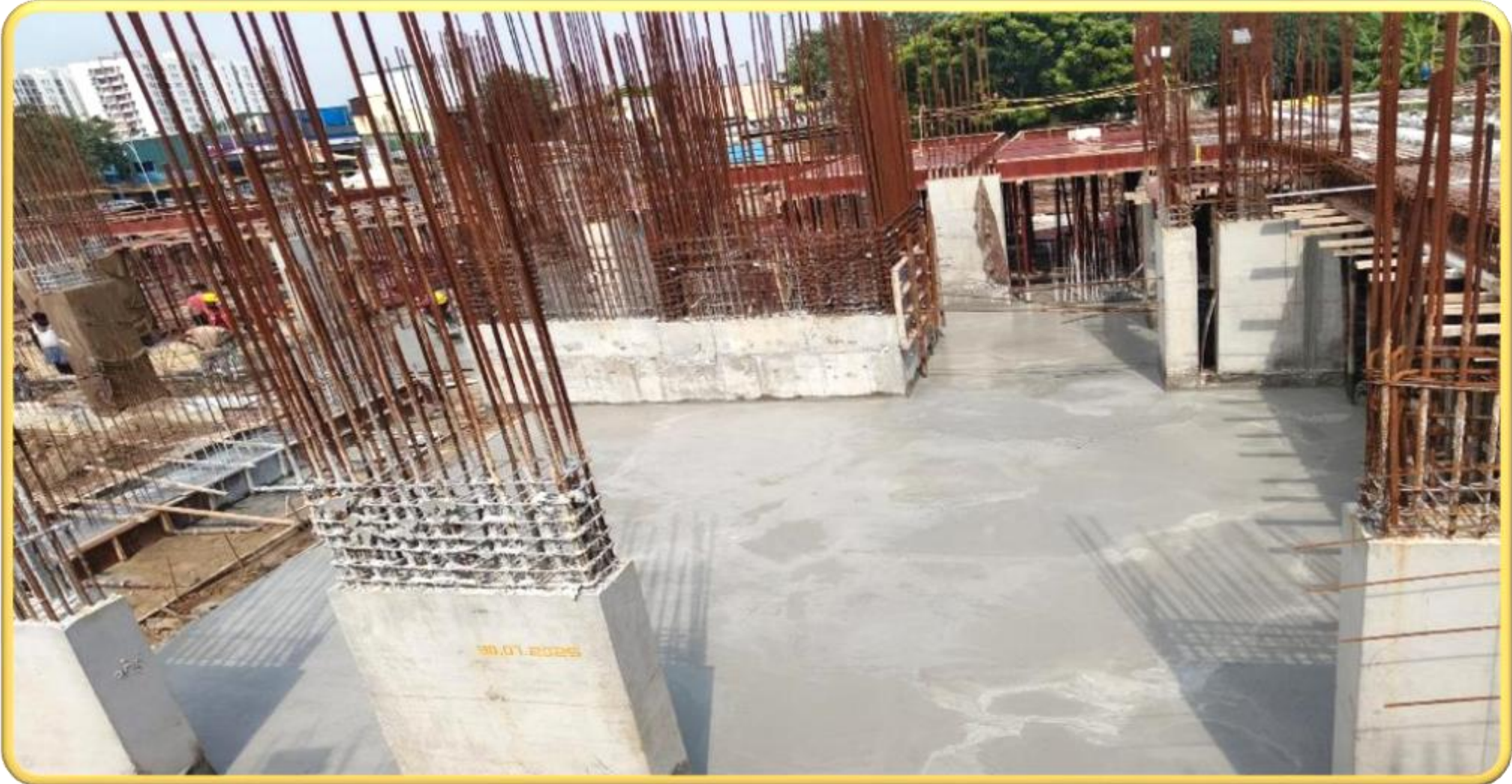
Main Building – Pour 2 grade slab PCC Completed
