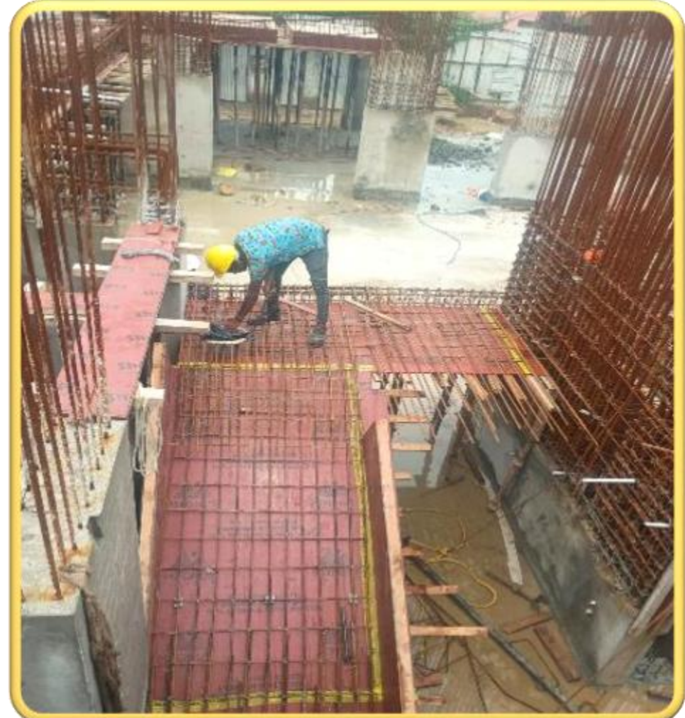
Main building – Staircase Mid landing shuttering & reinforcement work in progress
