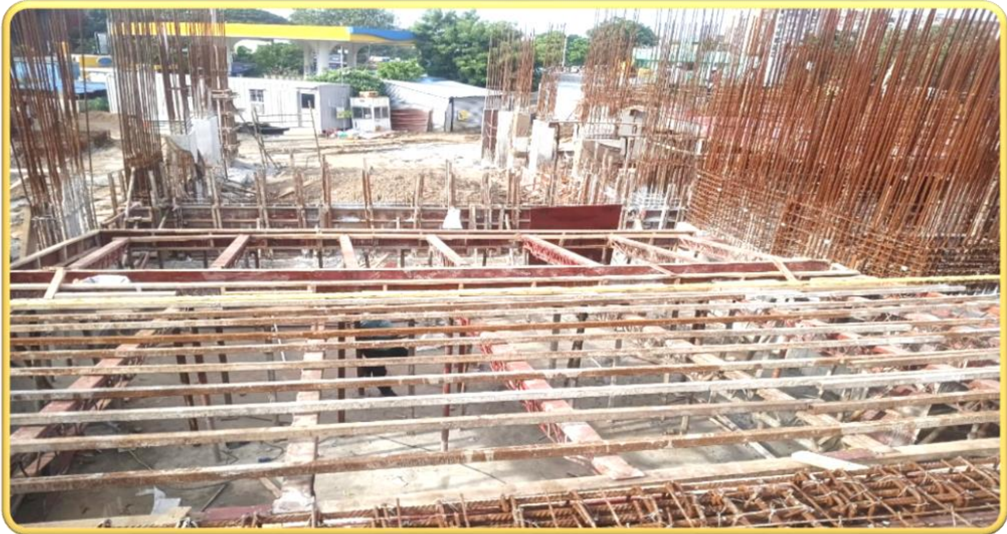
Main building – Ramp Slab Shuttering Work
