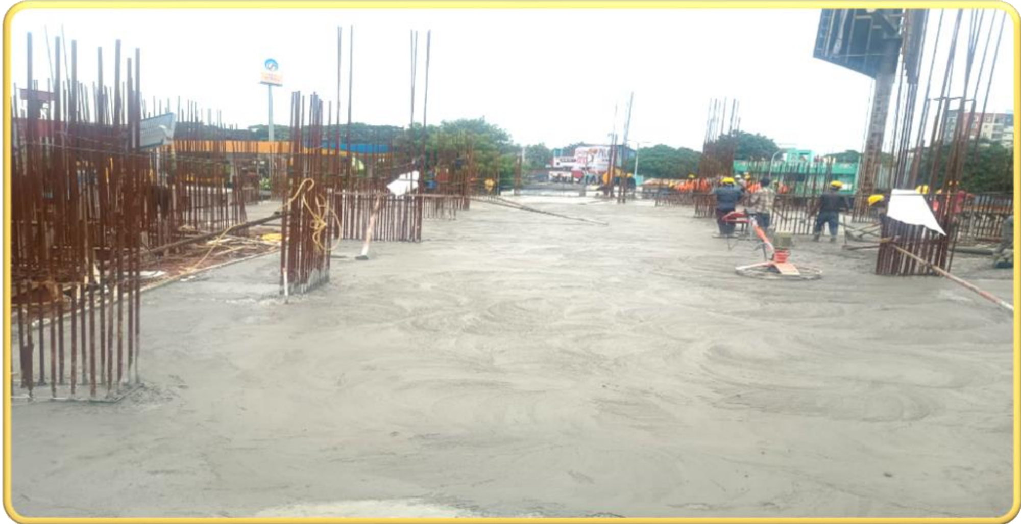
Main building – Pour 2 slab concrete work in progress
