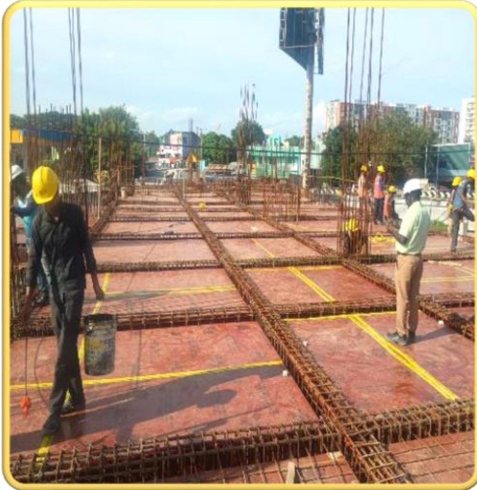
Main building – Pour 2 Stilt floor roof beam and slab reinforcement work completed
