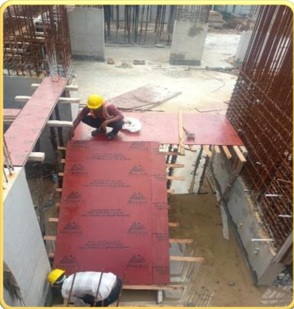
Main building – Staircase Mid landing shuttering & reinforcement work in progress
