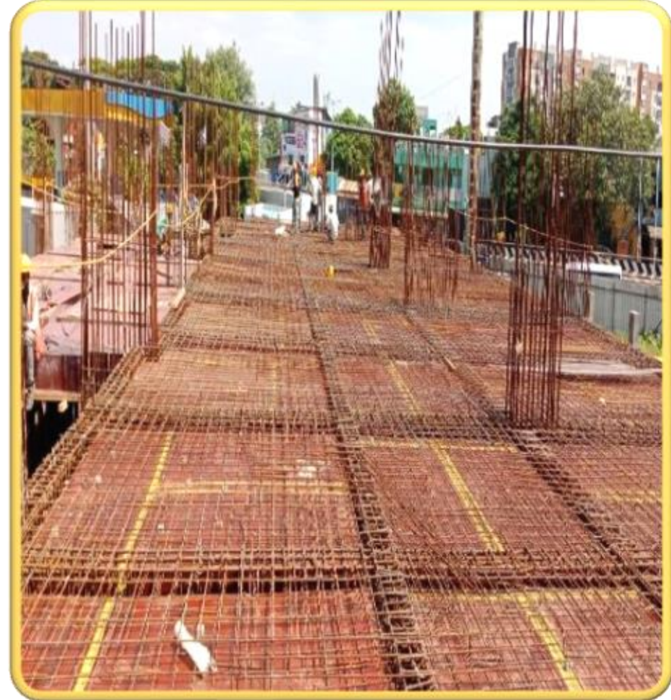
Main building – Pour 2 Stilt floor roof beam and slab reinforcement work completed
