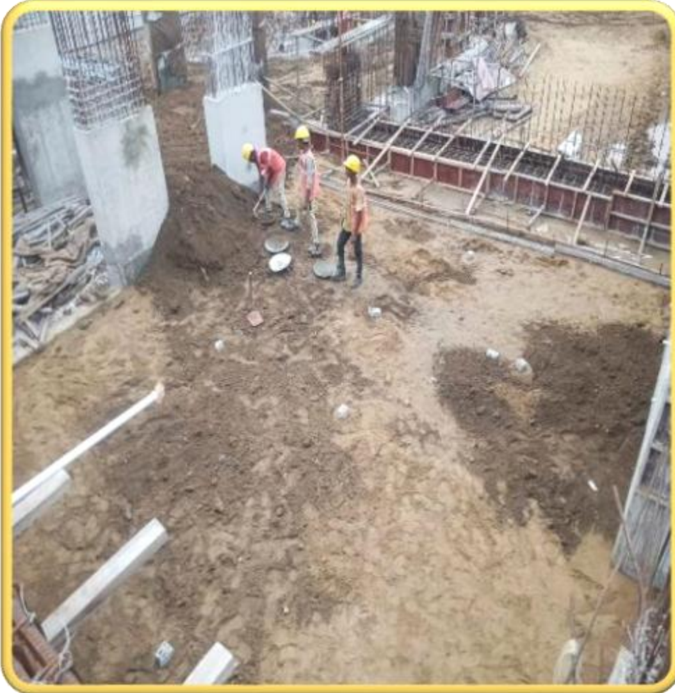
Main Building – Pour 2 Basement Backfilling and Consolidation work Completed
