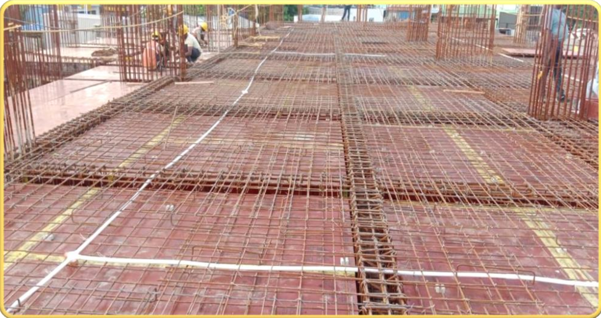
Main building – Stilt floor roof pour 2 Electrical Work
