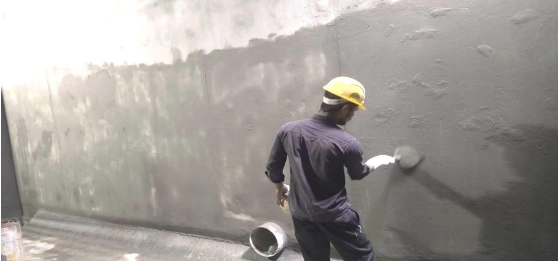
Main building – UG sump waterproofing work in progress
