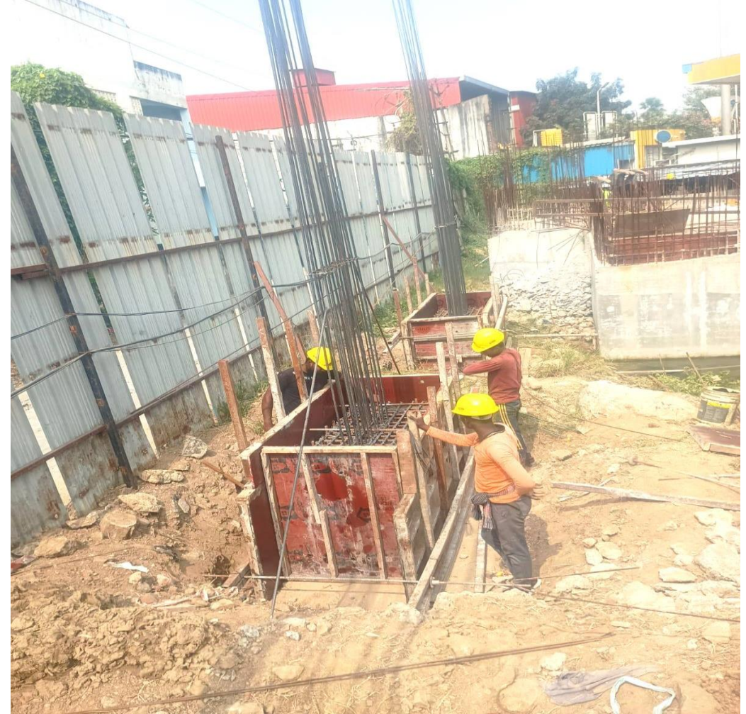
Amenity Block - Pile cap reinforcement and shuttering work in progress
