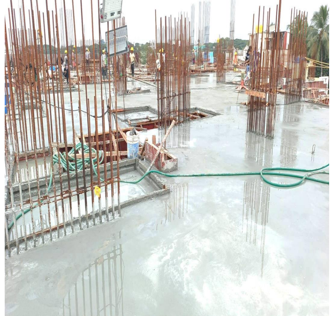
Main building – 2 nd floor roof slab concrete completed
