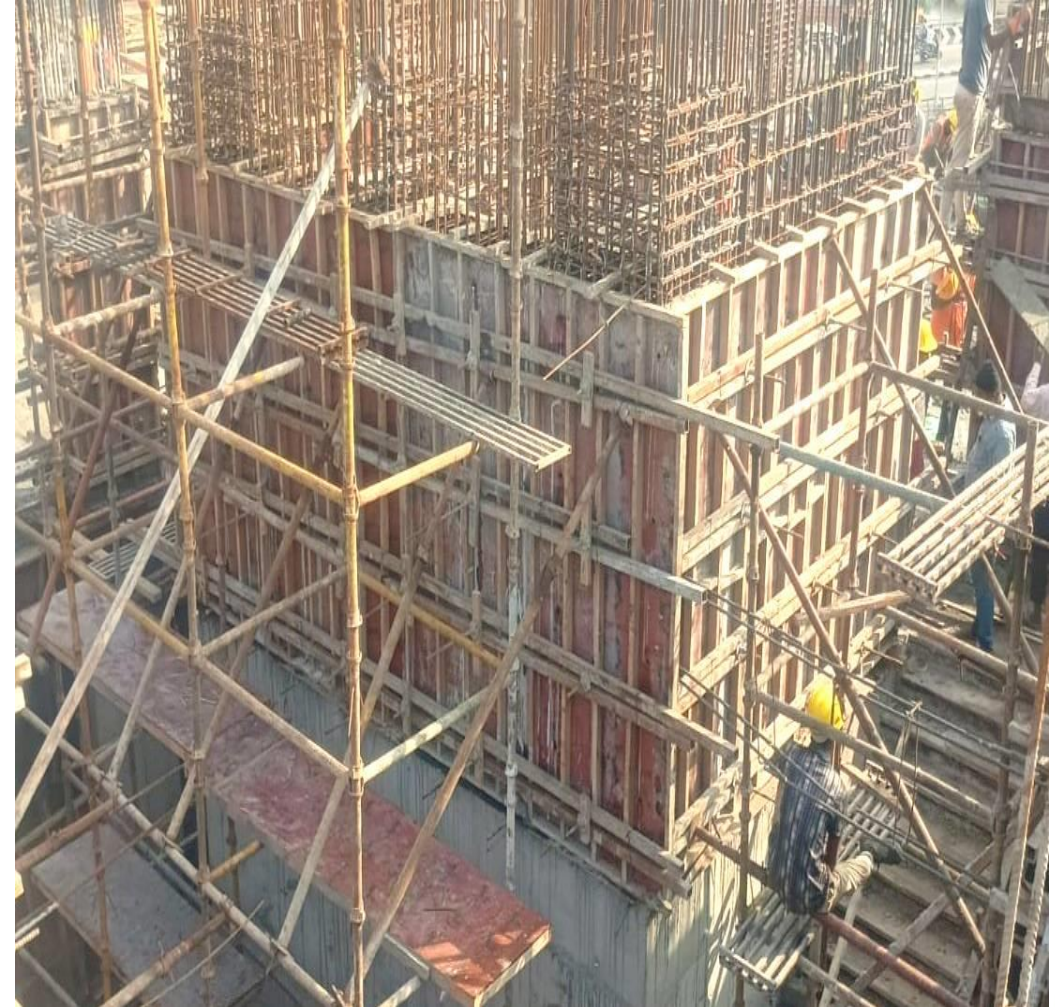
Main building - 3rd floor Lift wall and columns shuttering work completed
