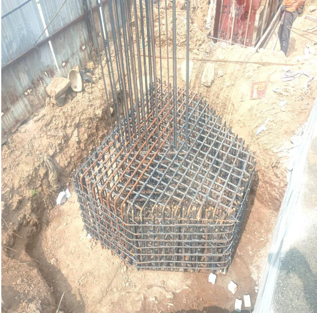
Amenity Block - Pile cap reinforcement and shuttering work in progress
