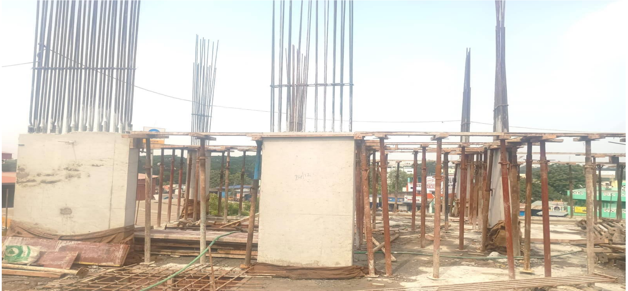
Main building – 3 rd floor roof slab shuttering work in progress
