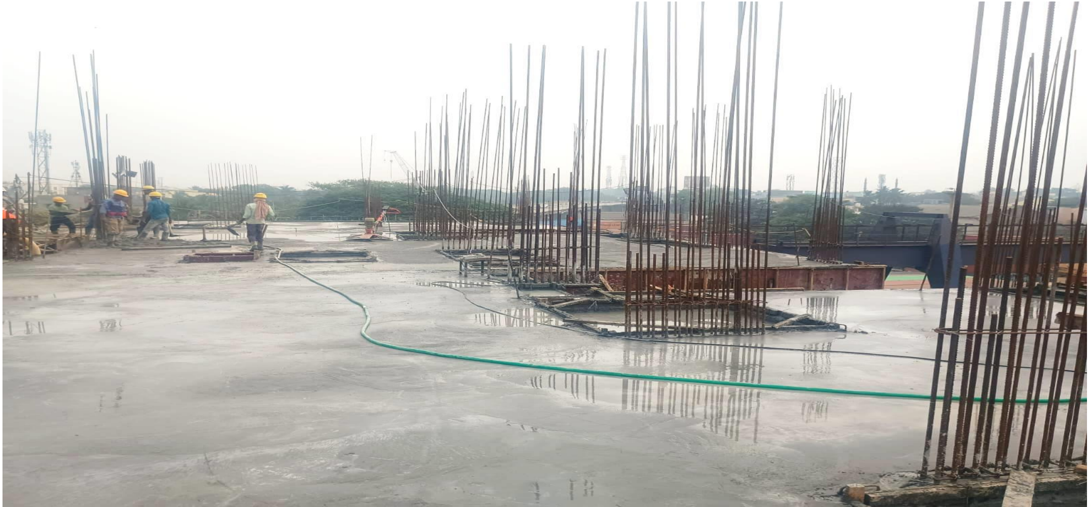
Main building – 3 rd floor roof slab concrete completed
