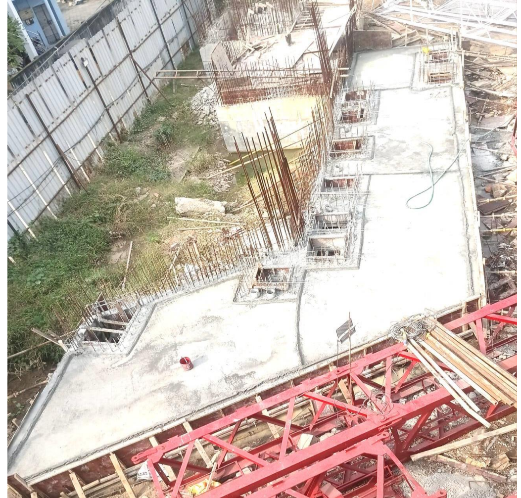
STP Cover slab reinforcement and concrete completed
