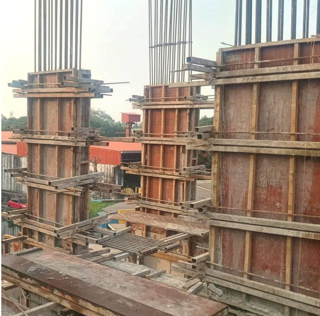
Main building - 3rd floor Lift wall and columns shuttering work completed
