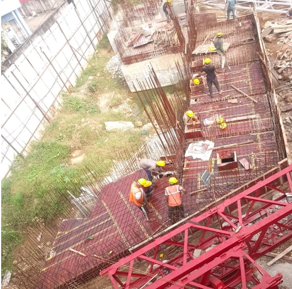
STP Cover slab reinforcement and concrete completed
