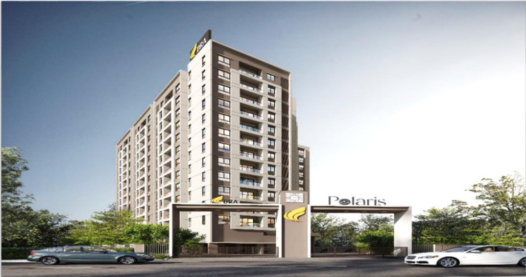
DRA POLARIS Construction update photos – March 2026
