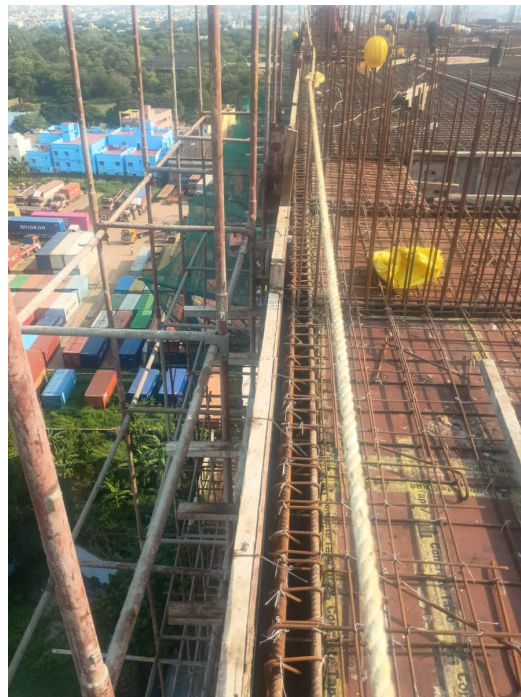
Thirteenth Floor P2 - Roof Slab Shuttering
