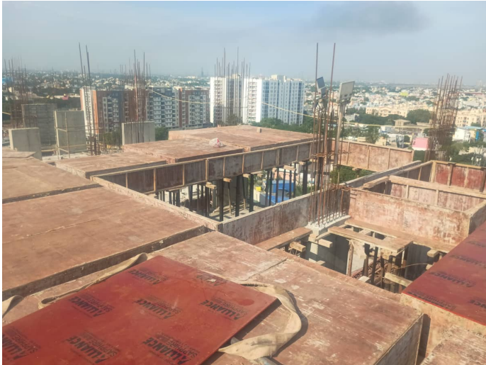
Thirteenth Floor P2 - Roof Slab Shuttering
