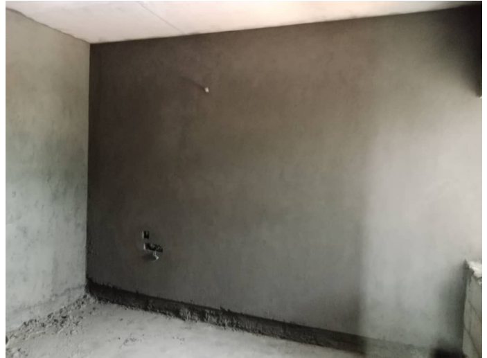
7F - Flat Internal Plastering
