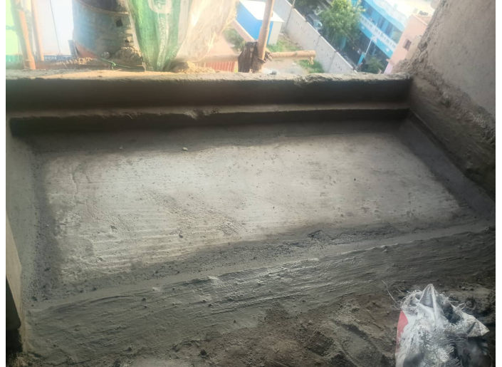
6F - Balcony Waterproofing
