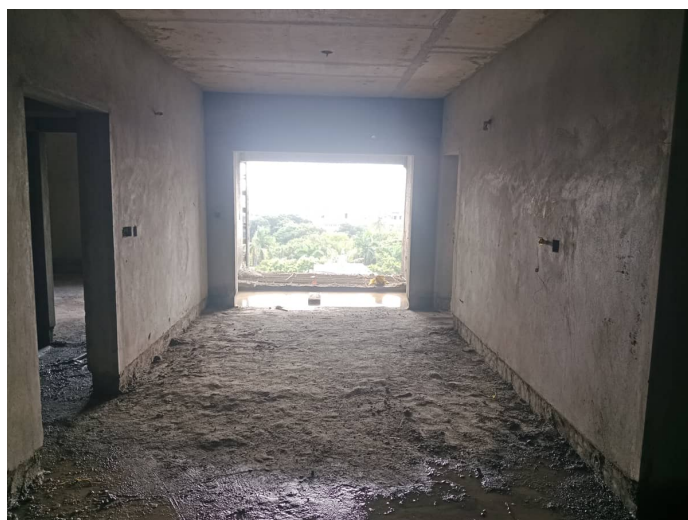
On Completion of Plastering - 6th Floor - 601
