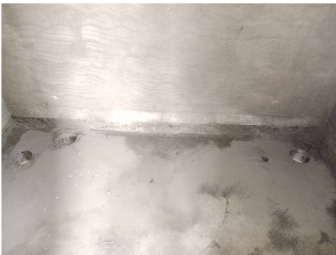
8F - Core & Wall Cutting - Civil
