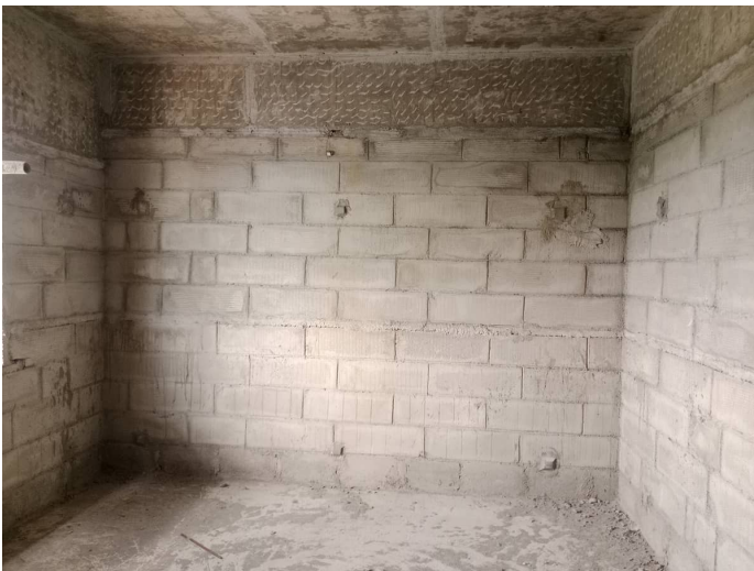
On Completion of Blockwork - 9th Floor - 907
