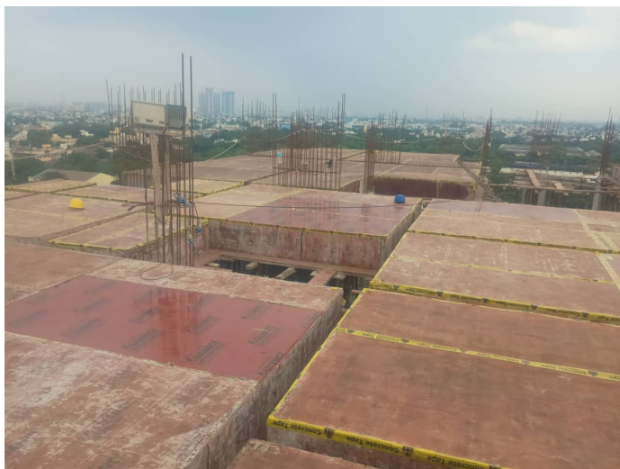
Thirteenth Floor P2 - Roof Slab Shuttering
