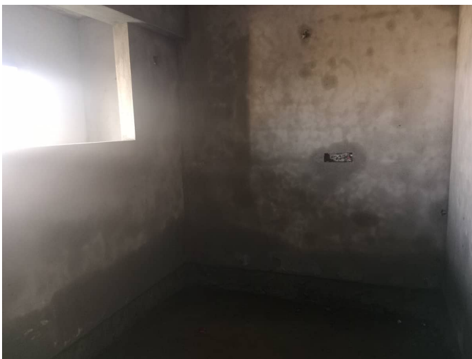
On Completion of Plastering - 6th Floor - 605
