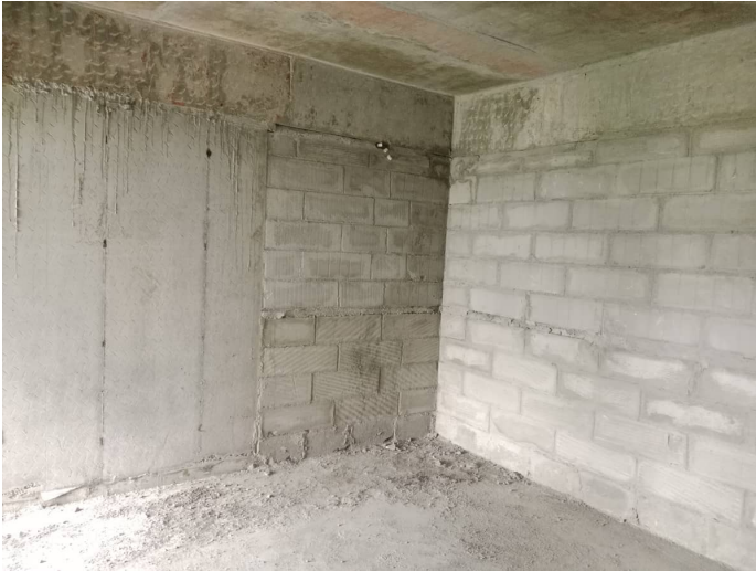
On Completion of Blockwork - 9th Floor - 904
