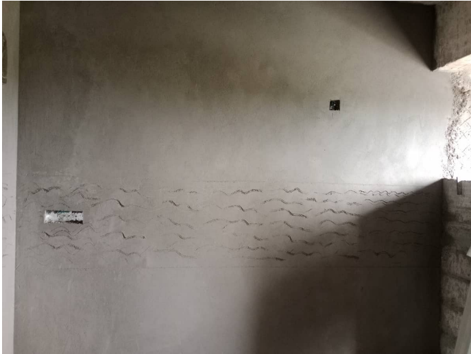
7F - Flat Internal Plastering
