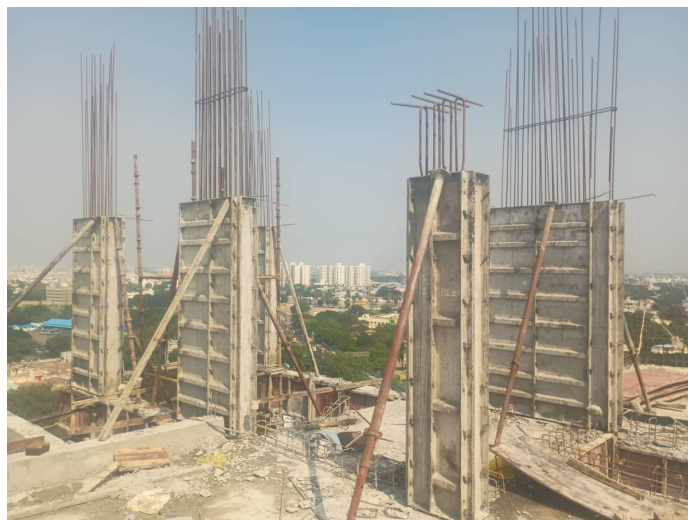
SHR - Column Shuttering
