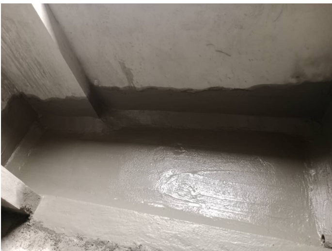
6F - Balcony Waterproofing
