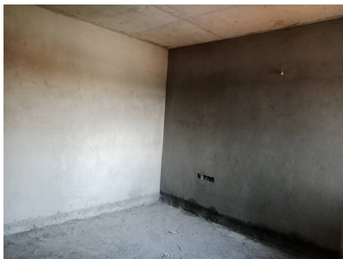
On Completion of Plastering - 6th Floor - 607
