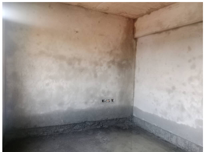
On Completion of Plastering - 6th Floor - 605
