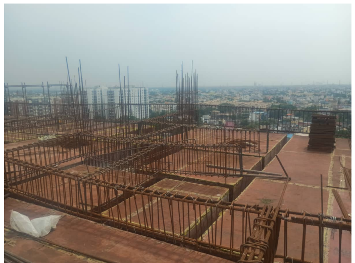
Thirteenth Floor P2 - Slab & Beam Reinforcement
