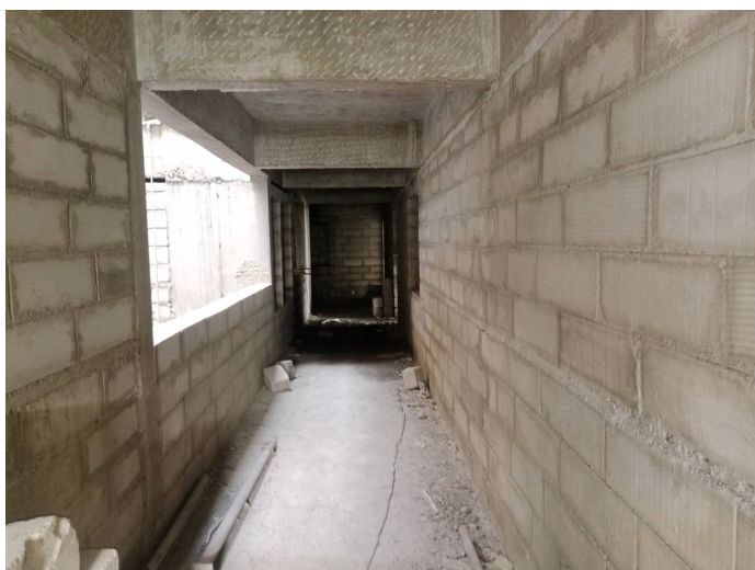
BW - Corridor - Ninth Floor
