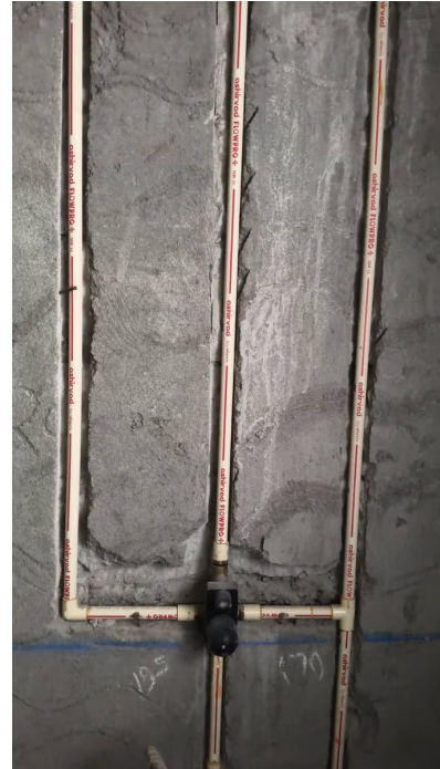
3F - Wall Concealed Pipe laying& Suspended Line
