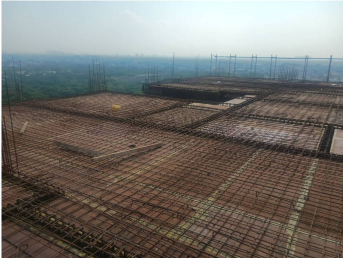
Thirteenth Floor P1 - Slab & Beam Reinforcement
