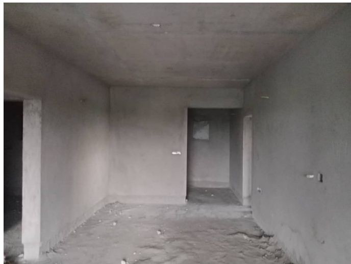
On Completion of Plastering - 6th Floor - 608
