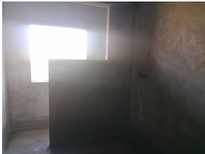
On Completion of Plastering - 6th Floor - 603
