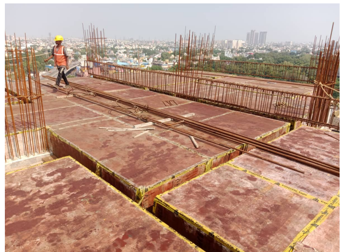
Thirteenth Floor P1 - Roof Slab Shuttering
