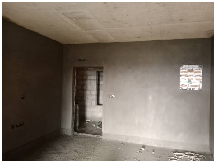
7F - Flat Internal Plastering
