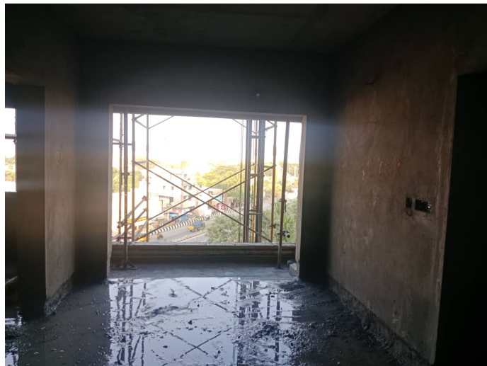
On Completion of Plastering - 6th Floor - 603
