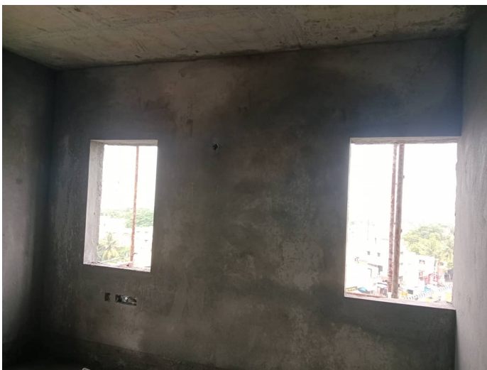
7F - Flat Internal Plastering
