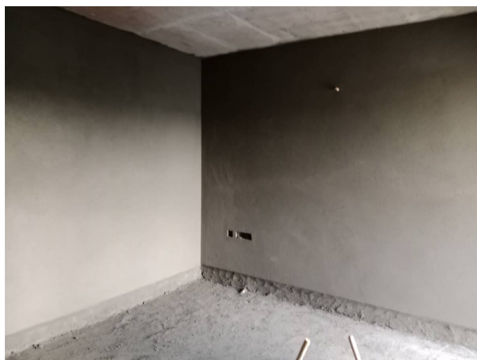
7F - Flat Internal Plastering
