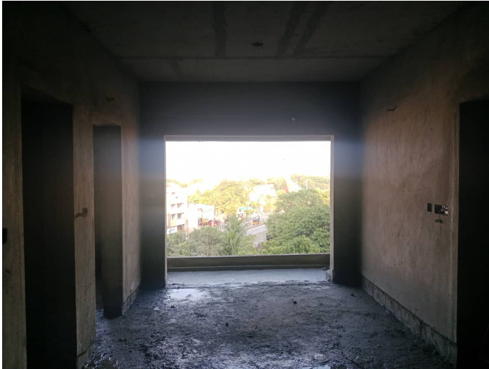
On Completion of Plastering - 6th Floor - 604
