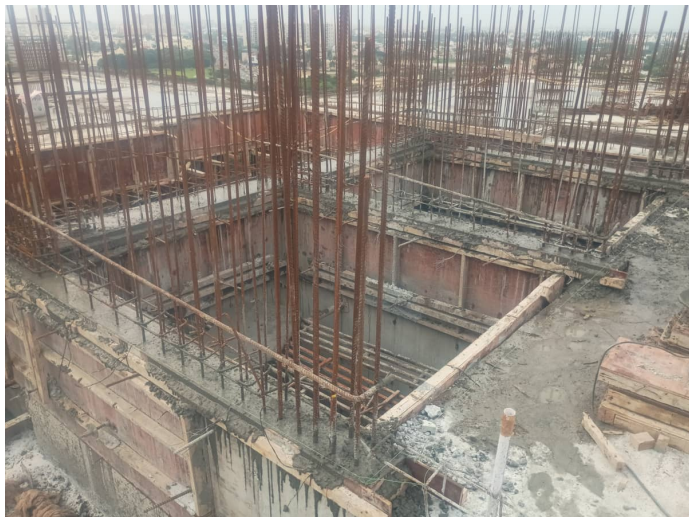
SHR - Col Marking & Reinforcement
