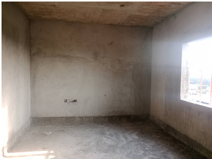
On Completion of Plastering - 6th Floor - 608
