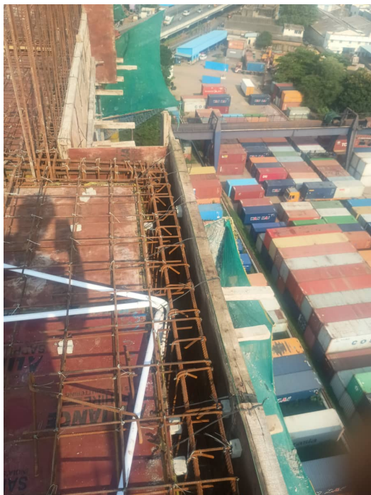
Thirteenth Floor P1 - Roof Slab Shuttering
