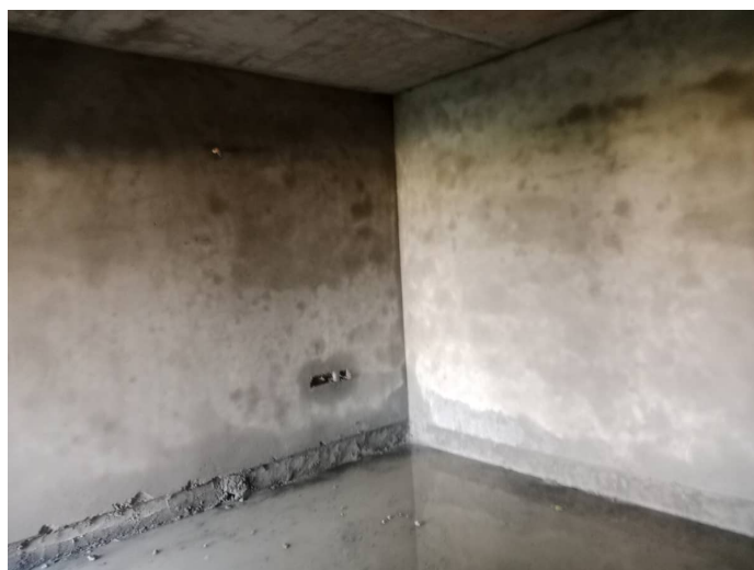
On Completion of Plastering - 6th Floor - 604
