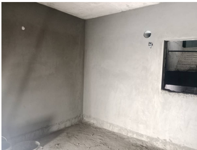
7F - Flat Internal Plastering
