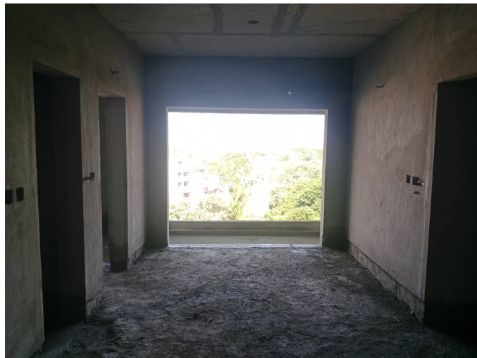
On Completion of Plastering - 6th Floor - 604
