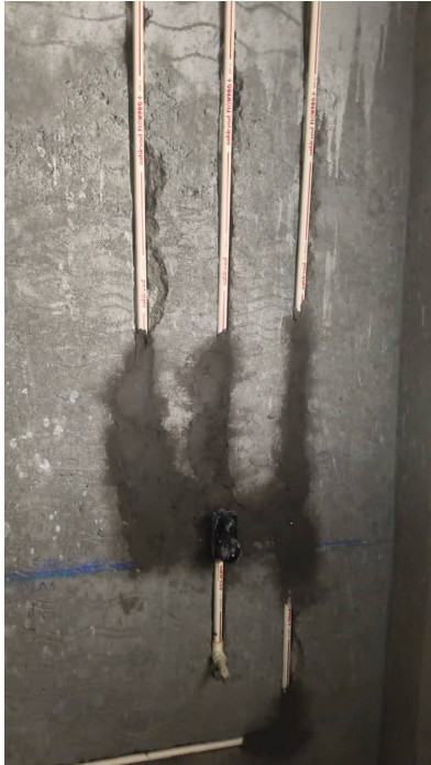
4F - Wall Concealed Pipe laying & Suspended Line
