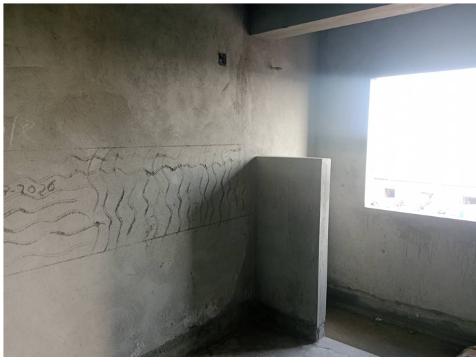
On Completion of Plastering - 6th Floor - 607
