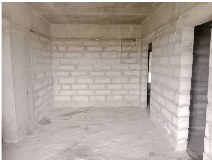
On Completion of Blockwork - 9th Floor - 903
