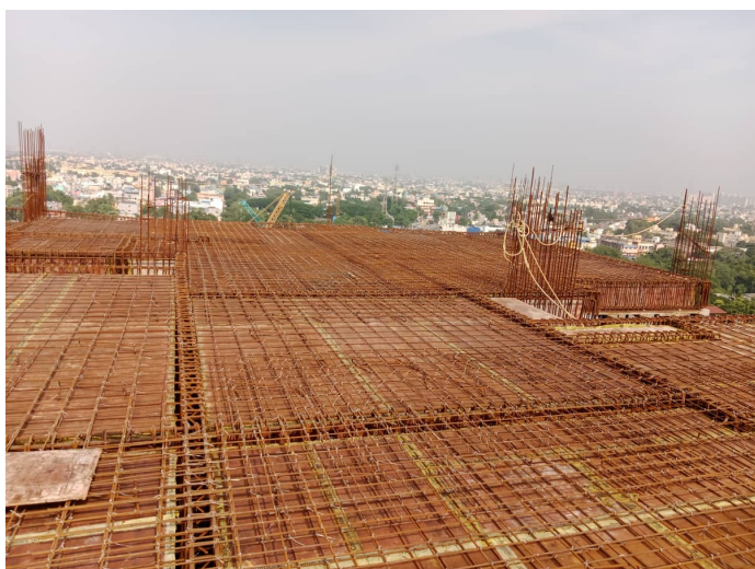
Thirteenth Floor P1 - Slab & Beam Reinforcement
