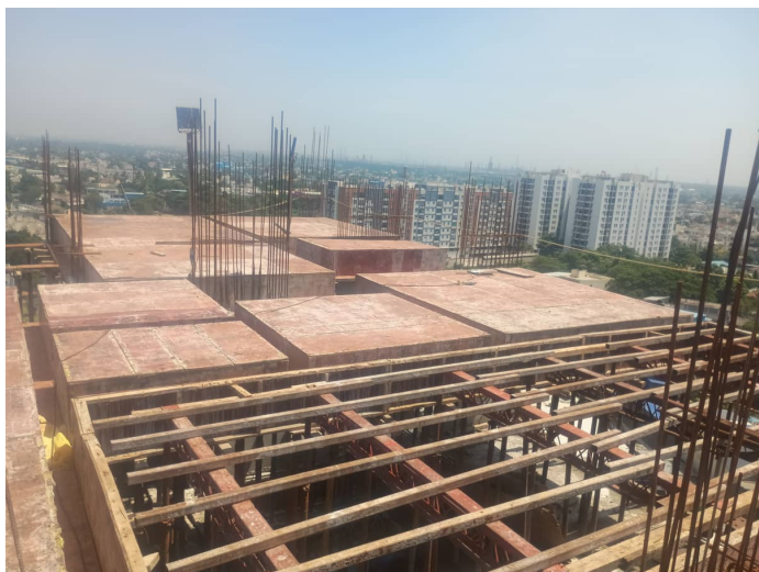
Thirteenth Floor P2 - Roof Slab Shuttering
