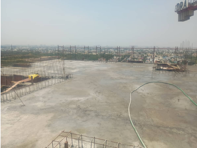
Thirteenth Floor P1 - Roof Slab Concreting
