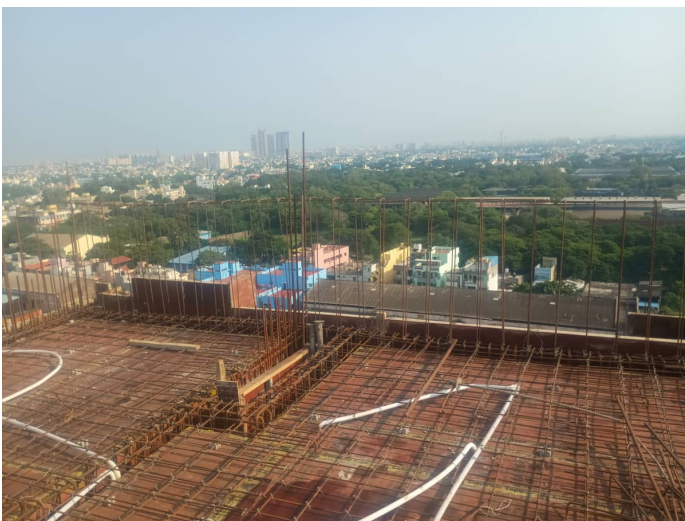
Thirteenth Floor P1 - Slab & Beam Reinforcement
