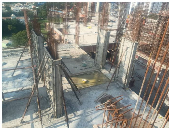
Thirteenth Floor P2 - Column Shuttering
