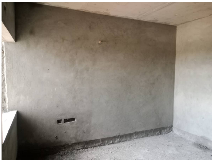
On Completion of Plastering - 6th Floor - 606
