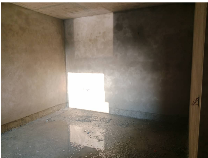
On Completion of Plastering - 6th Floor - 601
