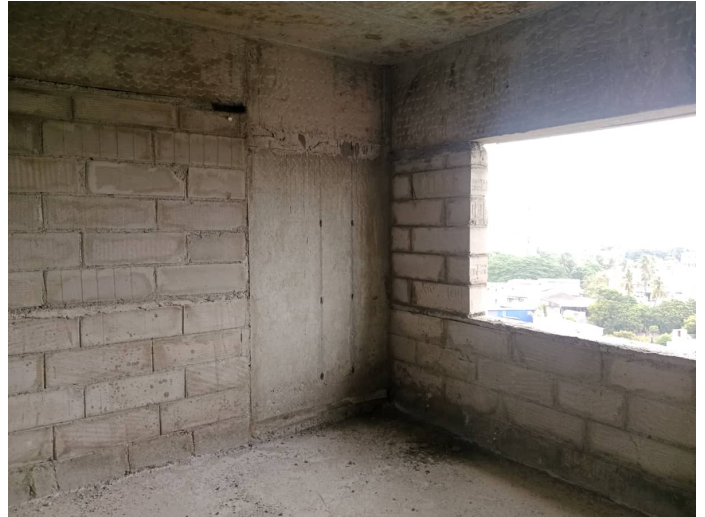
On Completion of Blockwork - 9th Floor - 904
