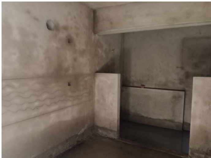
On Completion of Plastering - 6th Floor - 601
