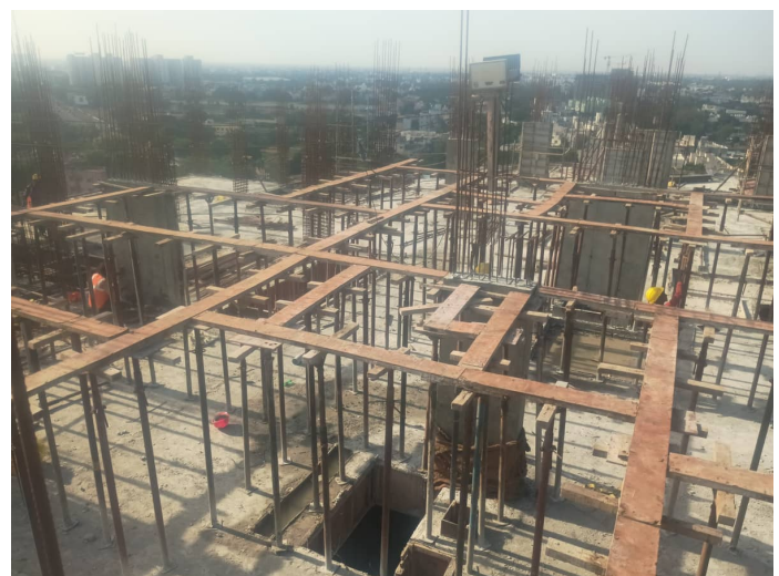
Thirteenth Floor P2 - Roof Slab Shuttering
