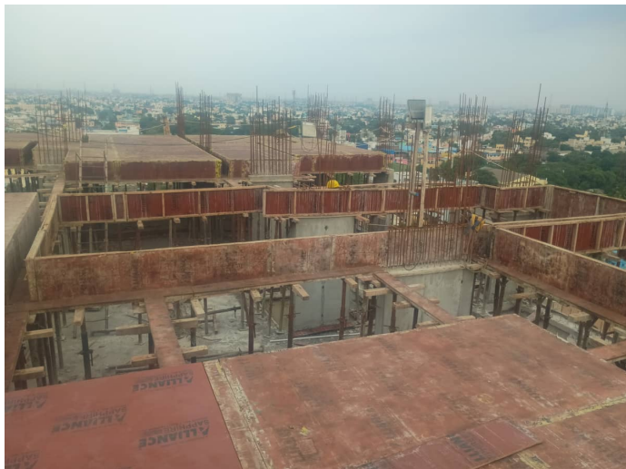
Thirteenth Floor P1 - Roof Slab Shuttering
