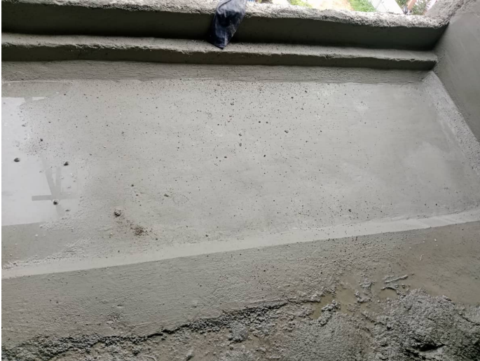
6F - Balcony Waterproofing
