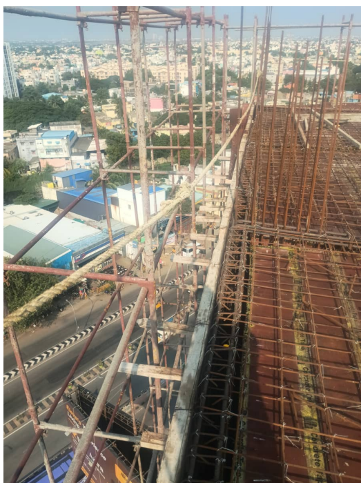
Thirteenth Floor P2 - Roof Slab Shuttering
