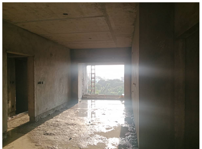
On Completion of Plastering - 6th Floor - 601
