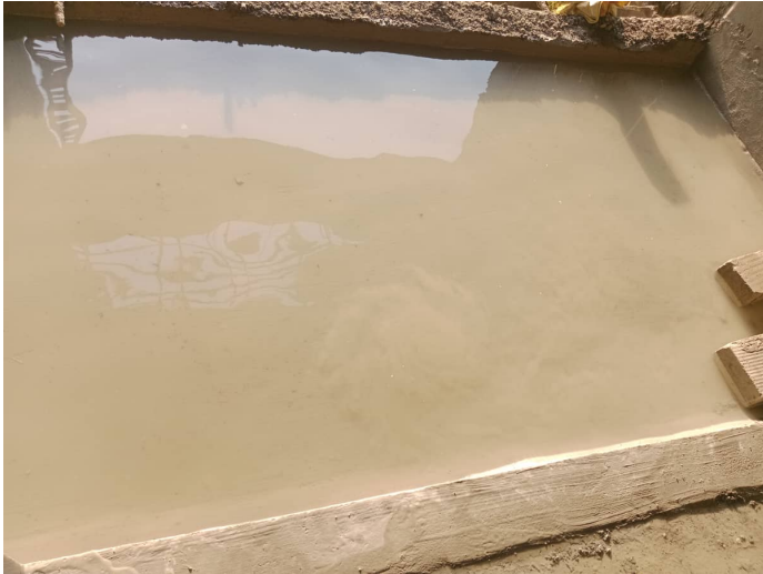
6F - Balcony Water Bond Test
