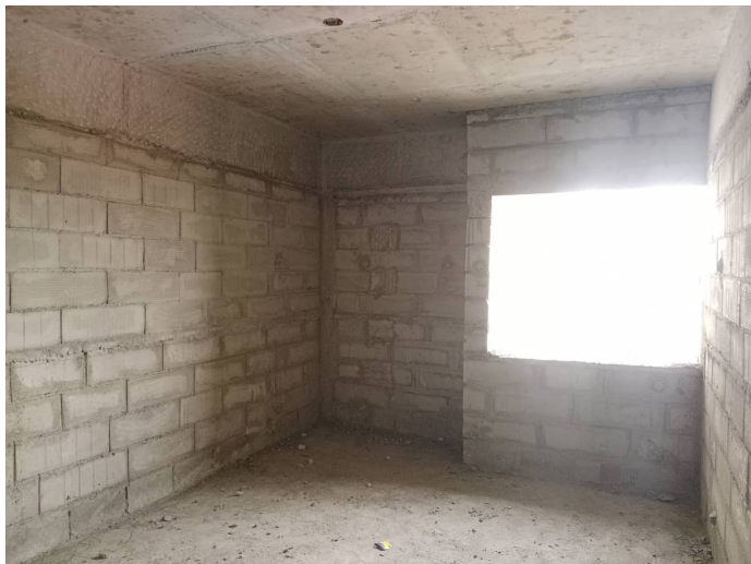
On Completion of Blockwork - 9th Floor - 901
