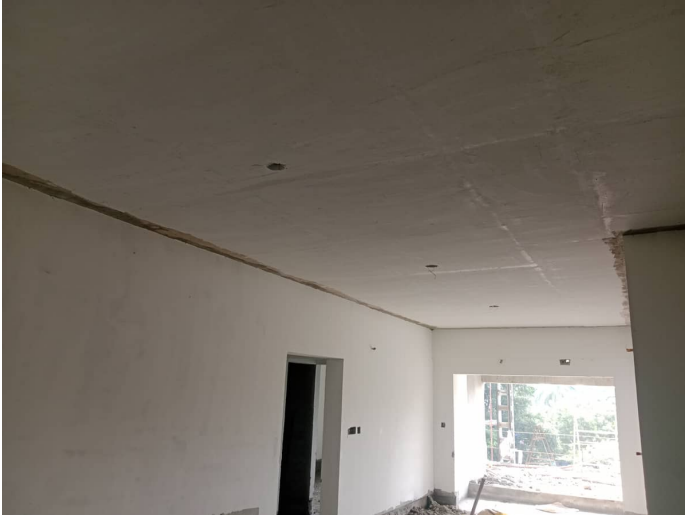
2F - Putty 1st Coat
