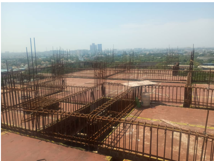
Thirteenth Floor P1 - Slab & Beam Reinforcement
