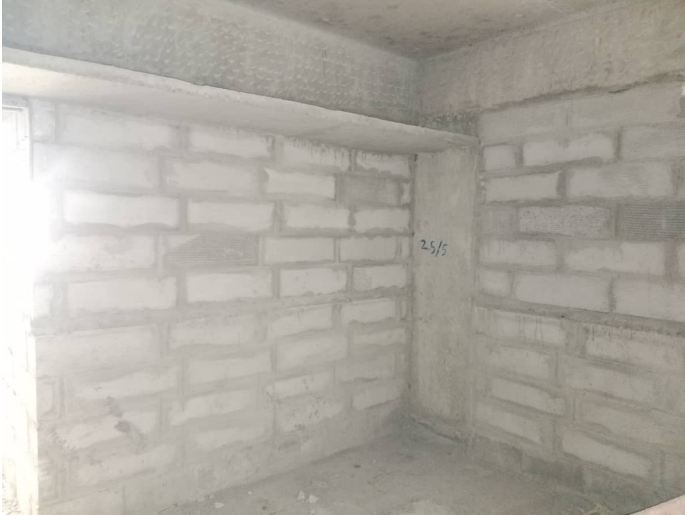
On Completion of Blockwork - 9th Floor - 908
