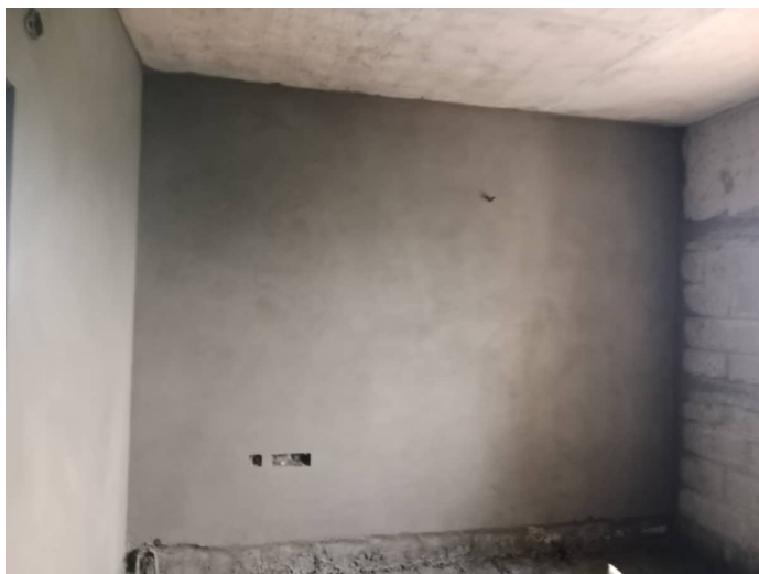
7F - Flat Internal Plastering
