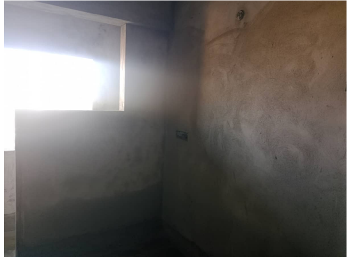
On Completion of Plastering - 6th Floor - 604
