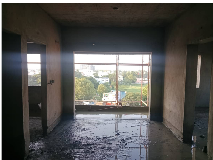
On Completion of Plastering - 6th Floor - 602
