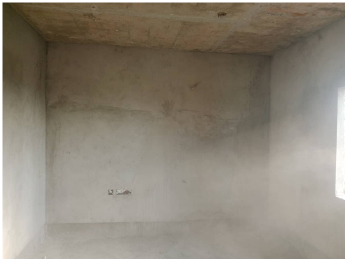
On Completion of Plastering - 6th Floor - 608
