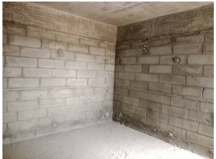
On Completion of Blockwork - 9th Floor - 907
