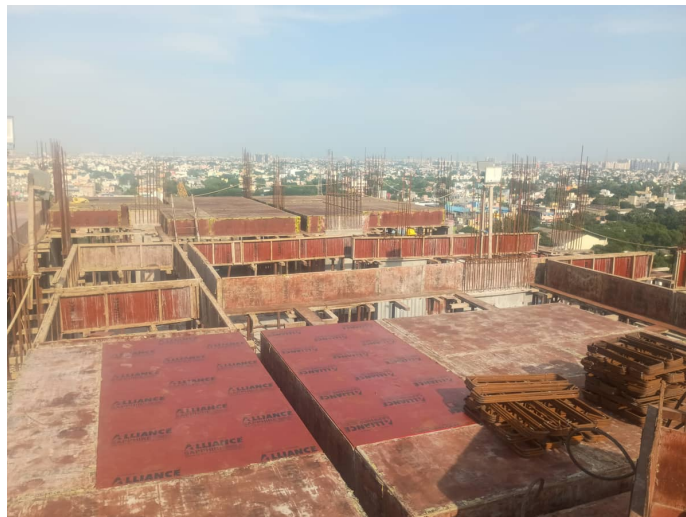
Thirteenth Floor P1 - Roof Slab Shuttering
