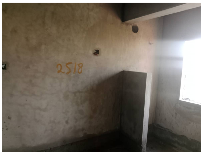
On Completion of Plastering - 6th Floor - 602
