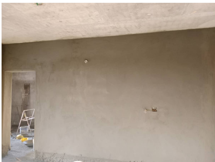
7F - Flat Internal Plastering
