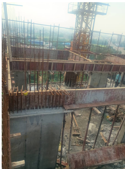
Thirteenth Floor P1 - Roof Slab Shuttering
