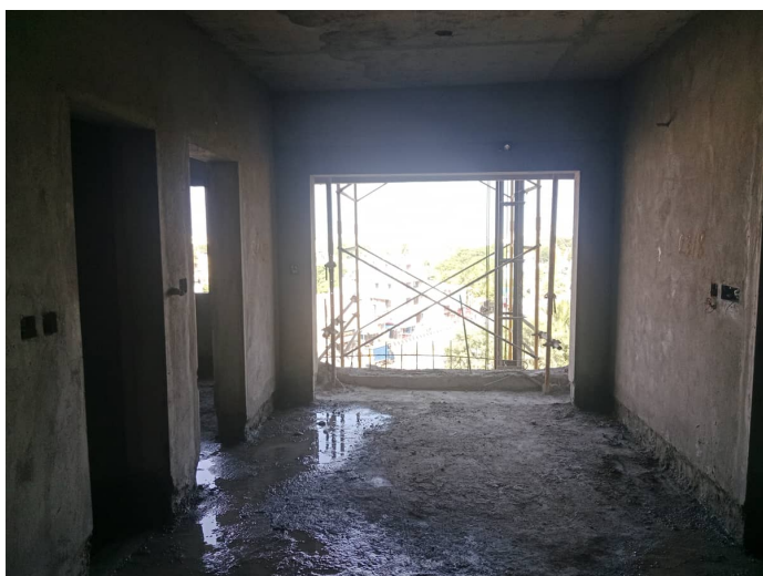
On Completion of Plastering - 6th Floor - 603
