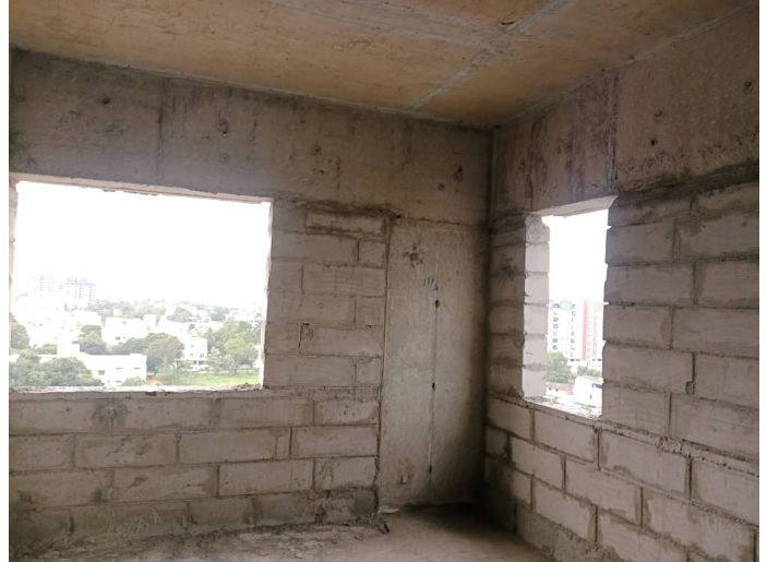
On Completion of Blockwork - 9th Floor - 902
