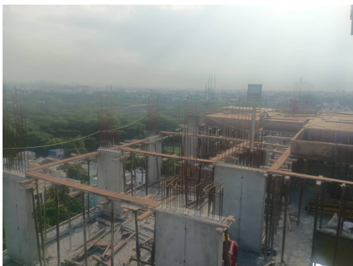
Thirteenth Floor P1 - Roof Slab Shuttering
