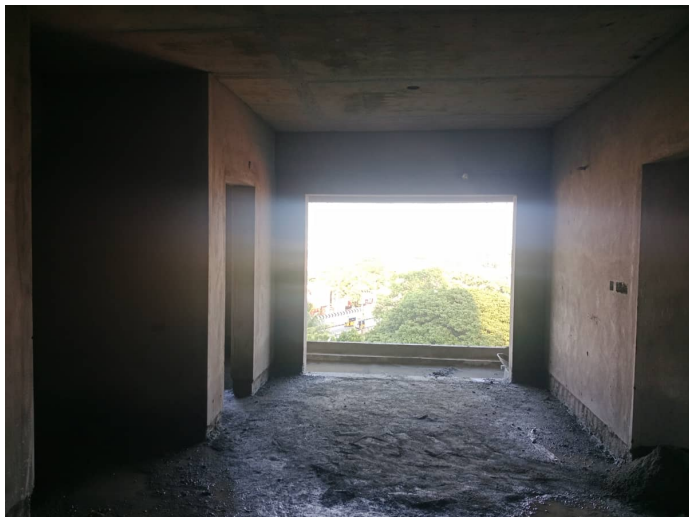
On Completion of Plastering - 6th Floor - 605
