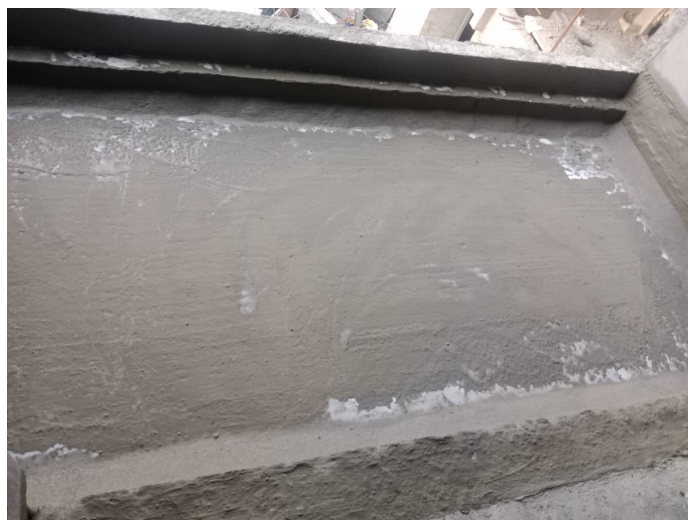
6F - Waterproofing - Civil
