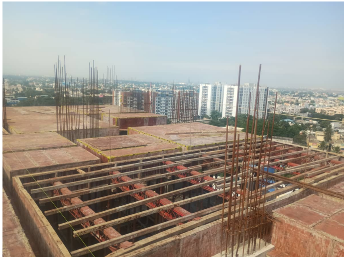
Thirteenth Floor P2 - Roof Slab Shuttering
