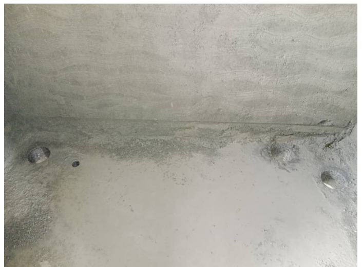
8F - Core & Wall Cutting - Civil
