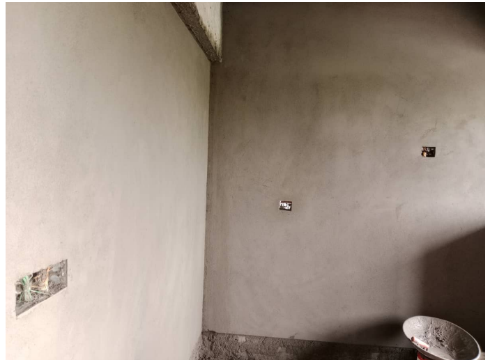
7F - Flat Internal Plastering
