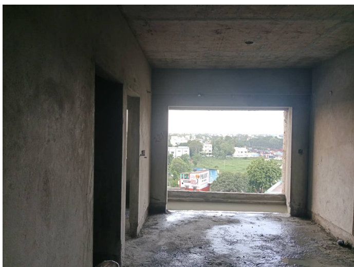
On Completion of Plastering - 6th Floor - 602
