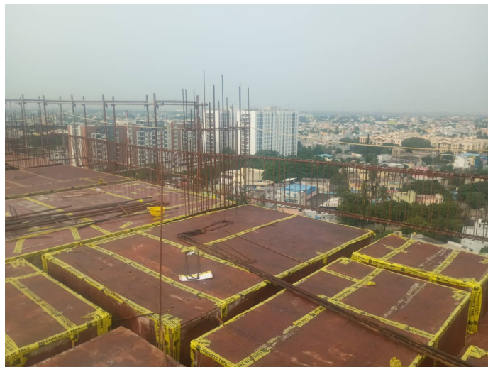
Thirteenth Floor P2 - Slab & Beam Reinforcement
