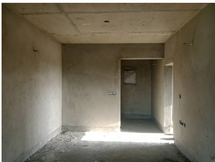
On Completion of Plastering - 6th Floor - 608
