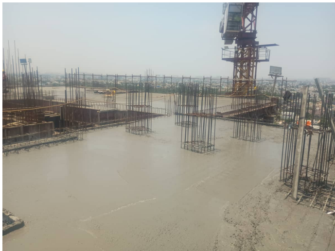
Thirteenth Floor P2 - Roof Slab Concreting
