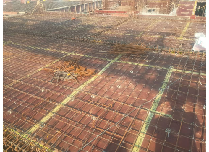
Thirteenth Floor P1 - Slab & Beam Reinforcement
