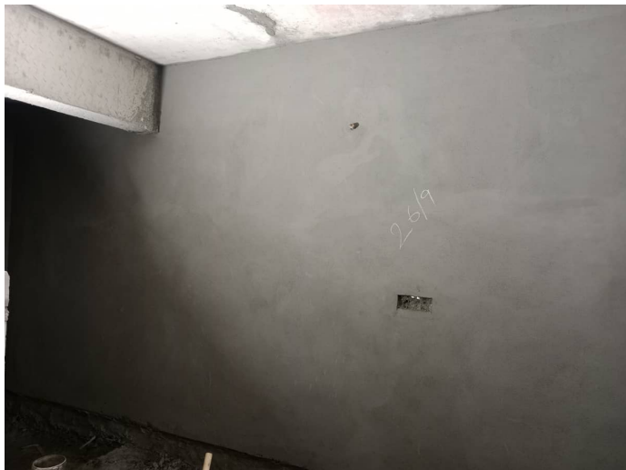
7F - Flat Internal Plastering
