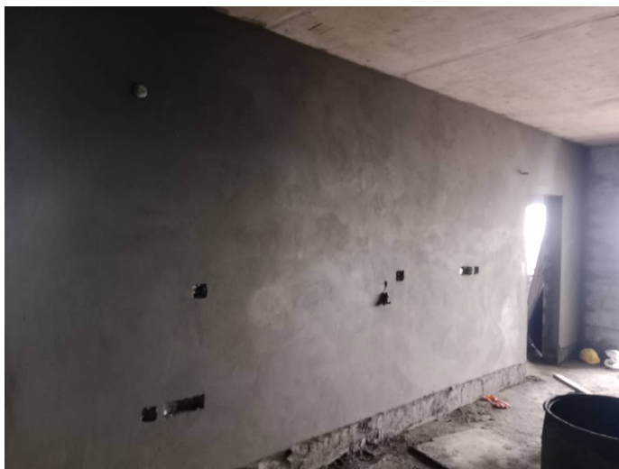
7F - Flat Internal Plastering
