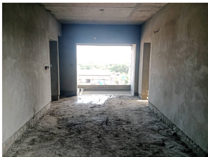
On Completion of Plastering - 6th Floor - 607
