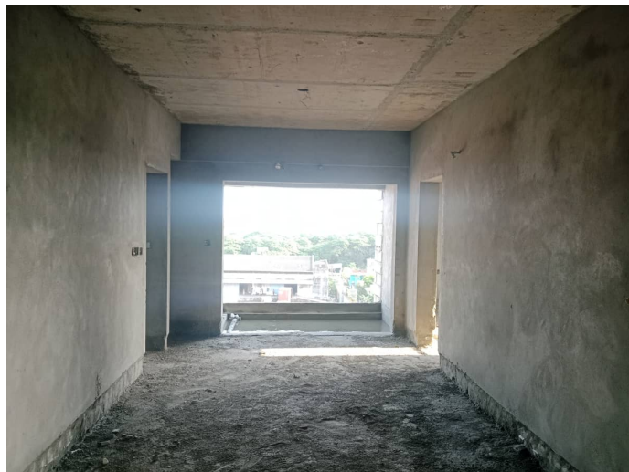
On Completion of Plastering - 6th Floor - 607
