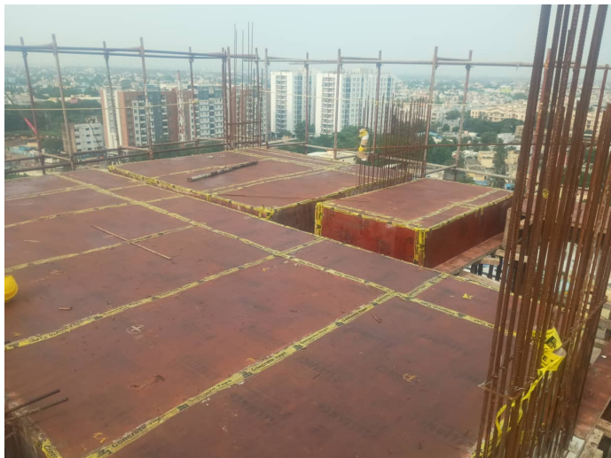
Thirteenth Floor P2 - Roof Slab Shuttering
