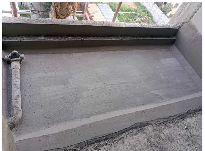
6F - Balcony Waterproofing
