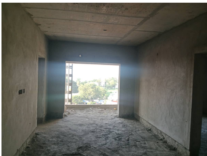
On Completion of Plastering - 6th Floor - 608
