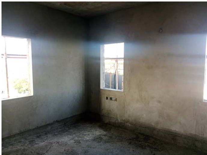
On Completion of Plastering - 6th Floor - 602
