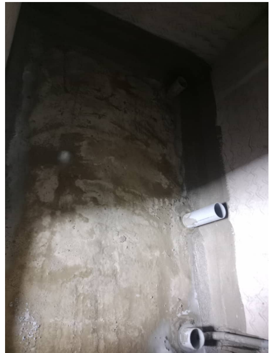
6F - Waterproofing - Civil
