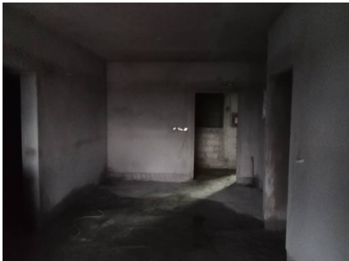
On Completion of Plastering - 6th Floor - 606
