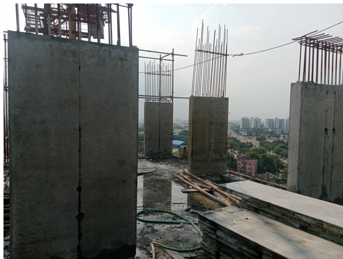
Thirteenth Floor P2 - Column Concrete
