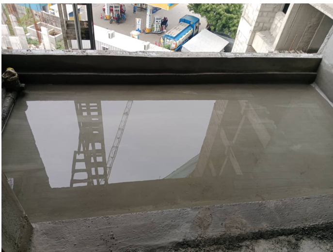
5F - Balcony Water Bond Test
