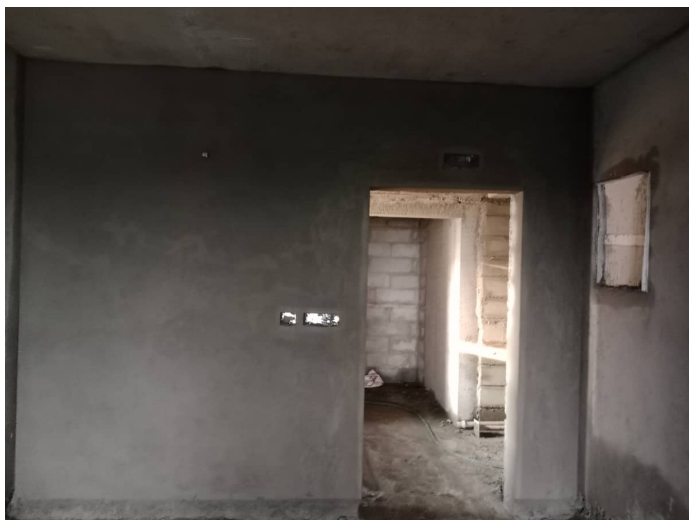
7F - Flat Internal Plastering
