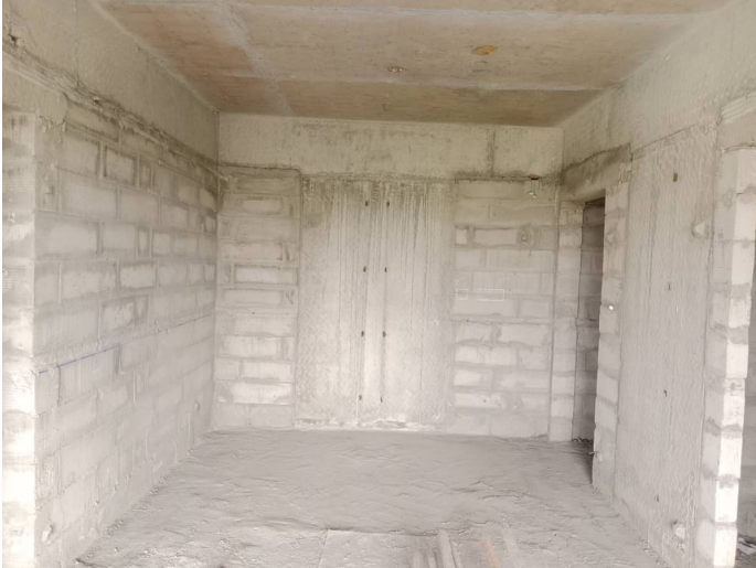
On Completion of Blockwork - 9th Floor - 902
