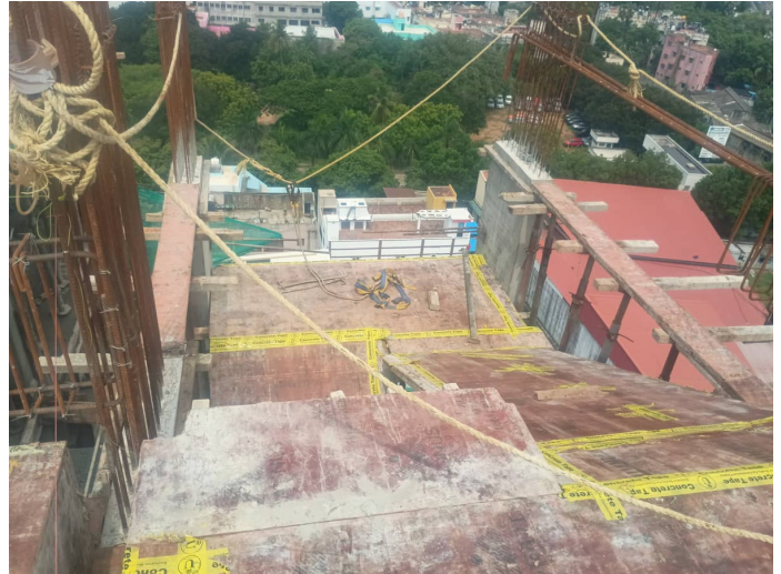
Thirteenth Floor P2 - Roof Slab Shuttering
