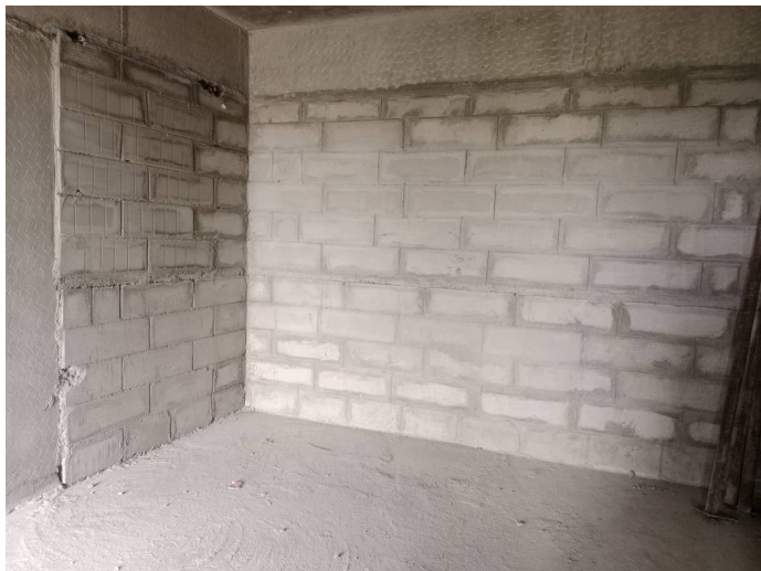
On Completion of Blockwork - 9th Floor - 903
