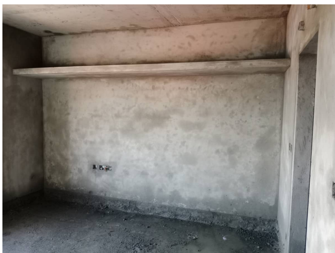
On Completion of Plastering - 6th Floor - 606
