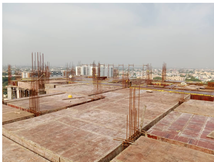
Thirteenth Floor P2 - Roof Slab Shuttering
