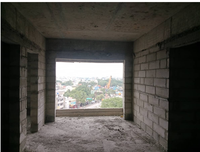
On Completion of Blockwork - 9th Floor - 904
