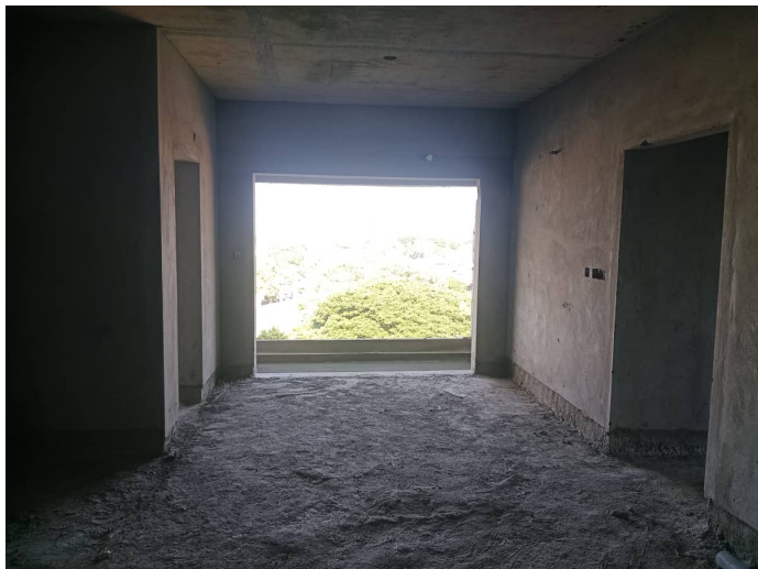
On Completion of Plastering - 6th Floor - 605
