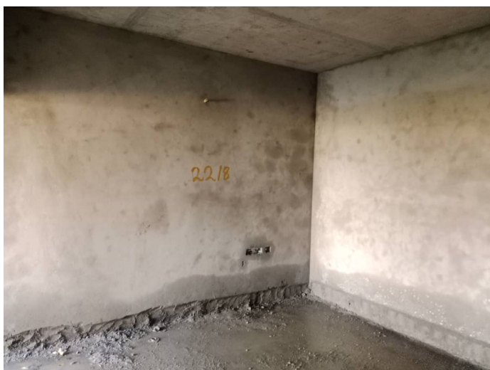
On Completion of Plastering - 6th Floor - 603
