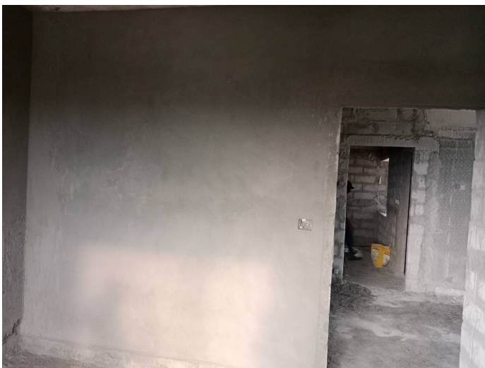
7F - Flat Internal Plastering
