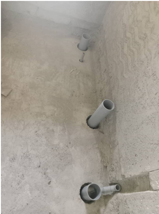
7F - Core & Wall Cutting - Civil
