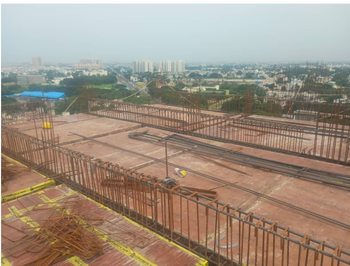
Thirteenth Floor P2 - Slab & Beam Reinforcement
