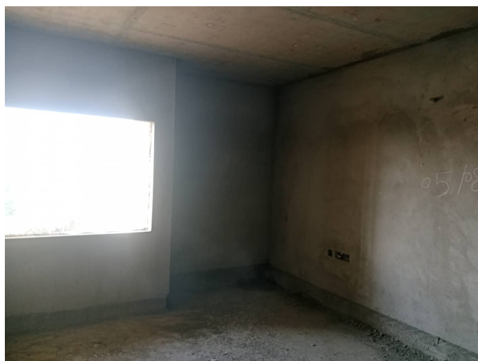
On Completion of Plastering - 6th Floor - 608
