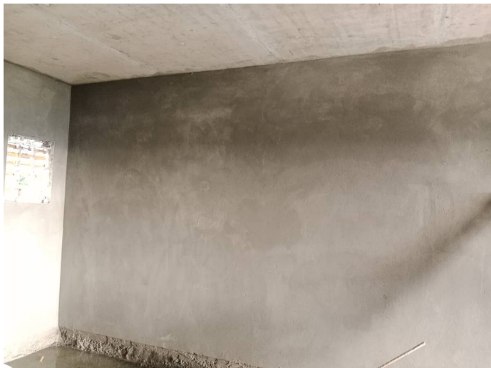
7F - Flat Internal Plastering
