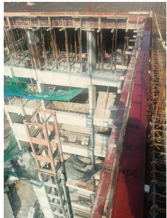
Thirteenth Floor P1 - Roof Slab Shuttering
