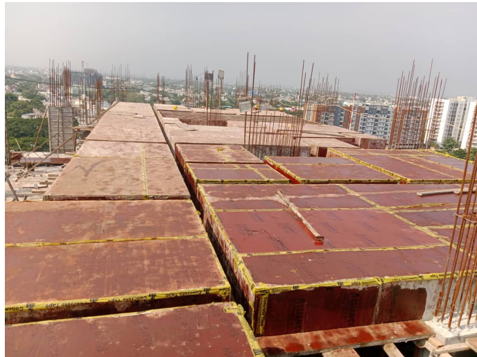
Thirteenth Floor P2 - Roof Slab Shuttering
