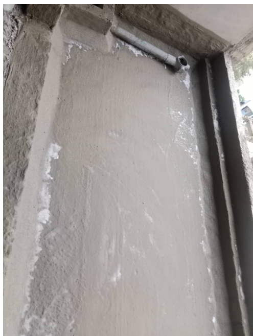
6F - Waterproofing - Civil
