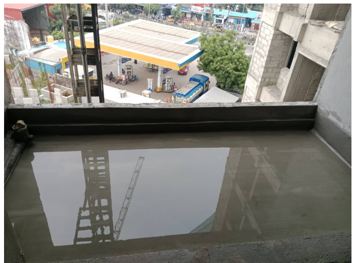
5F - Balcony Waterproofing
