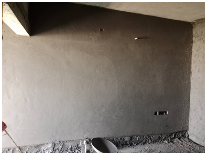
7F - Flat Internal Plastering
