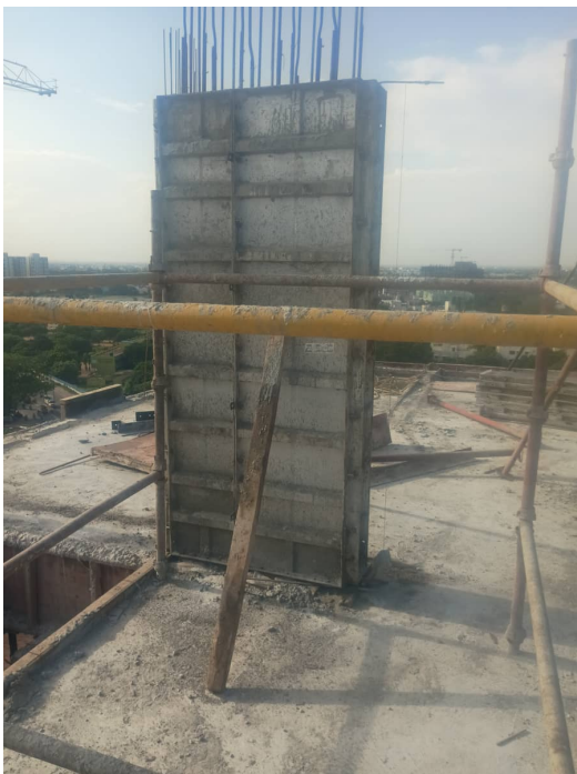
Thirteenth Floor P2 - Column Shuttering
