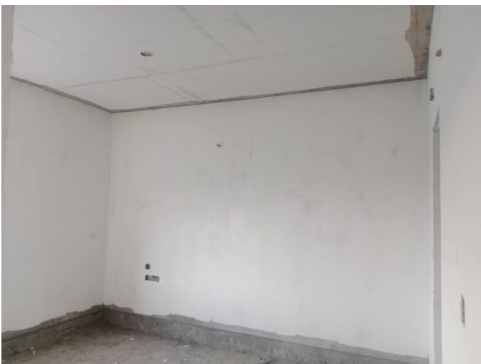
2F - Putty 1st Coat
