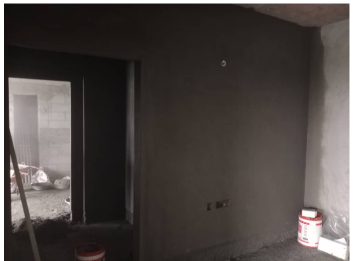
7F - Flat Internal Plastering
