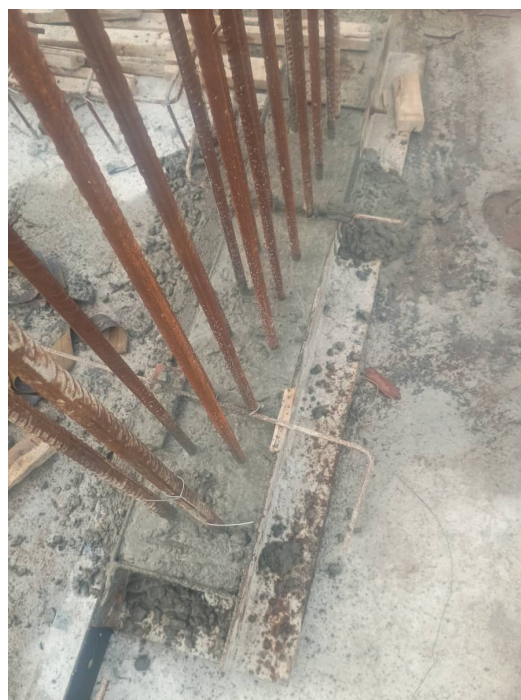
SHR - Col Marking & Reinforcement
