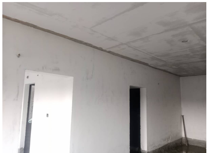
2F - Putty 1st Coat
