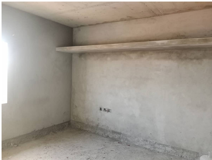
On Completion of Plastering - 6th Floor - 606
