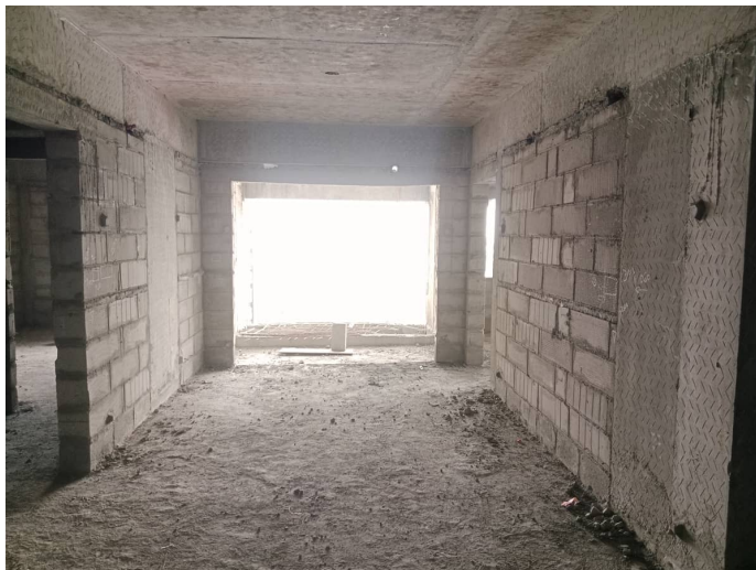
On Completion of Blockwork - 9th Floor - 901
