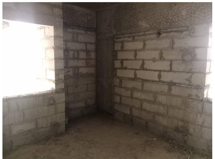
On Completion of Blockwork - 9th Floor - 901
