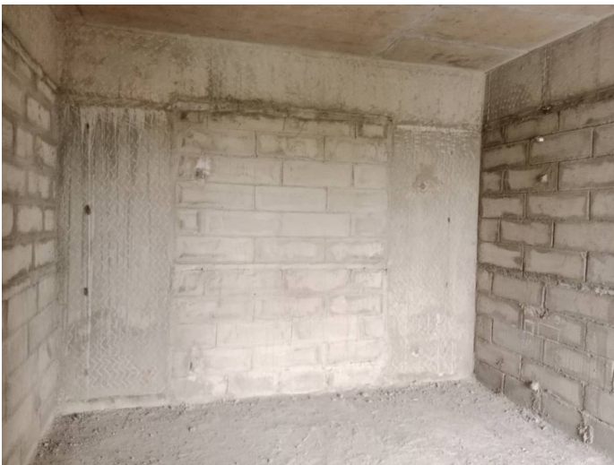
On Completion of Blockwork - 9th Floor - 902
