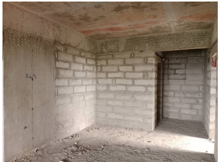
On Completion of Blockwork - 9th Floor - 908
