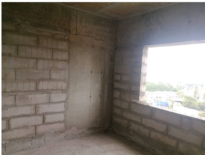
On Completion of Blockwork - 9th Floor - 903
