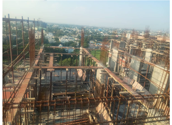
Thirteenth Floor P1 - Roof Slab Shuttering
