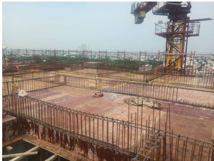
Thirteenth Floor P1 - Slab & Beam Reinforcement
