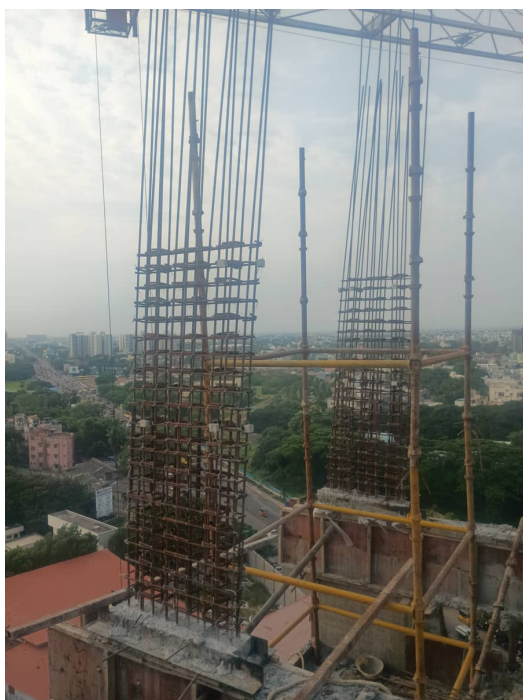
SHR - Col Marking & Reinforcement
