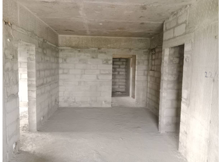
On Completion of Blockwork - 9th Floor - 907
