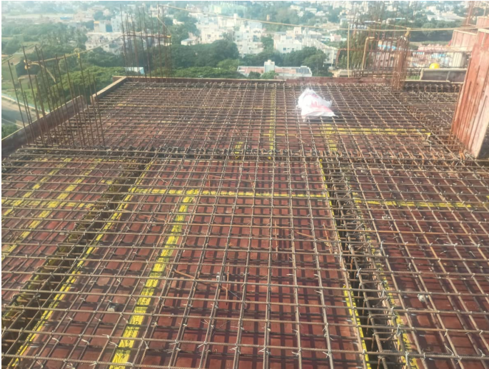
Thirteenth Floor P2 - Slab & Beam Reinforcement
