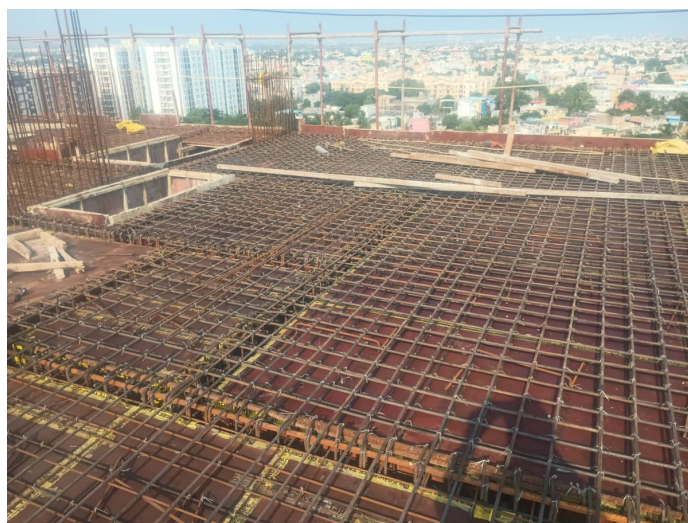
Thirteenth Floor P2 - Slab & Beam Reinforcement
