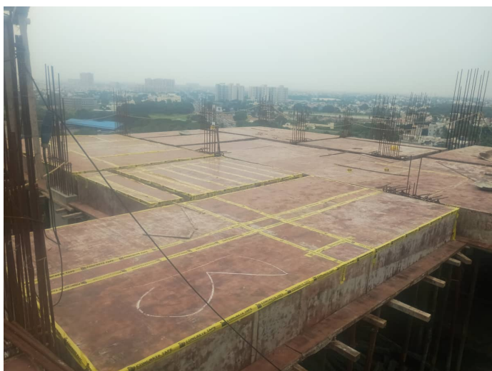
Thirteenth Floor P2 - Roof Slab Shuttering
