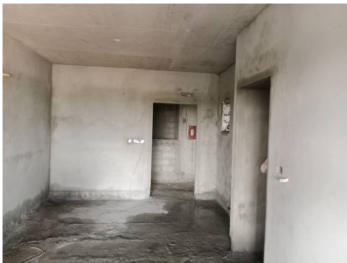
On Completion of Plastering - 6th Floor - 606
