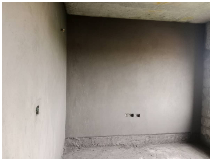
7F - Flat Internal Plastering
