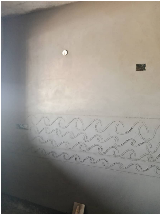
7F - Flat Internal Plastering
