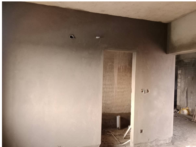
7F - Flat Internal Plastering
