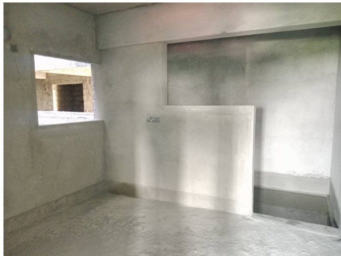
On Completion of Plastering - 6th Floor - 608
