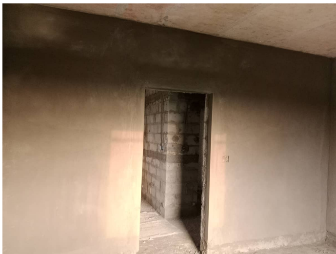
7F - Flat Internal Plastering
