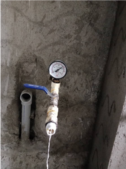
3F - Water Testing
