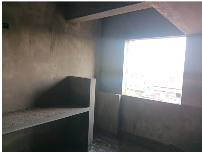
On Completion of Plastering - 6th Floor - 606
