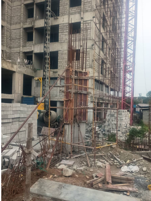
AM - Ground Floor - Column Concrete
