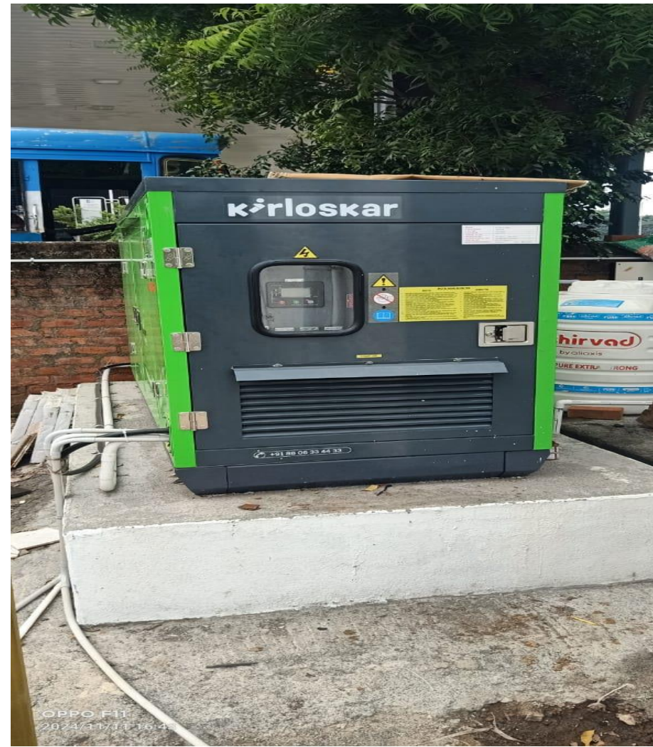
DRA Polaris - DG commissioning work completed
