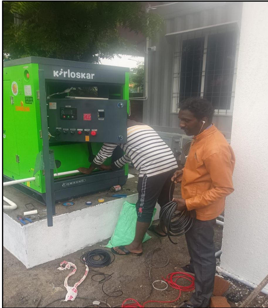
DRA Polaris - DG commissioning work completed
