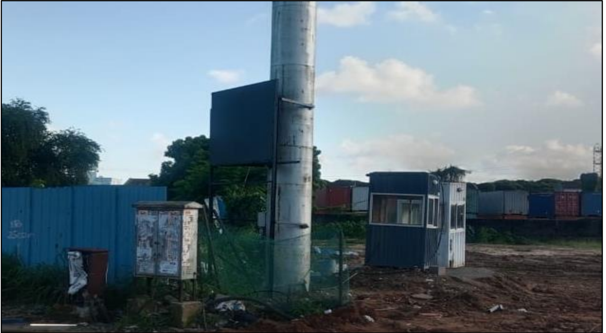
Timeline meter erection work completed
