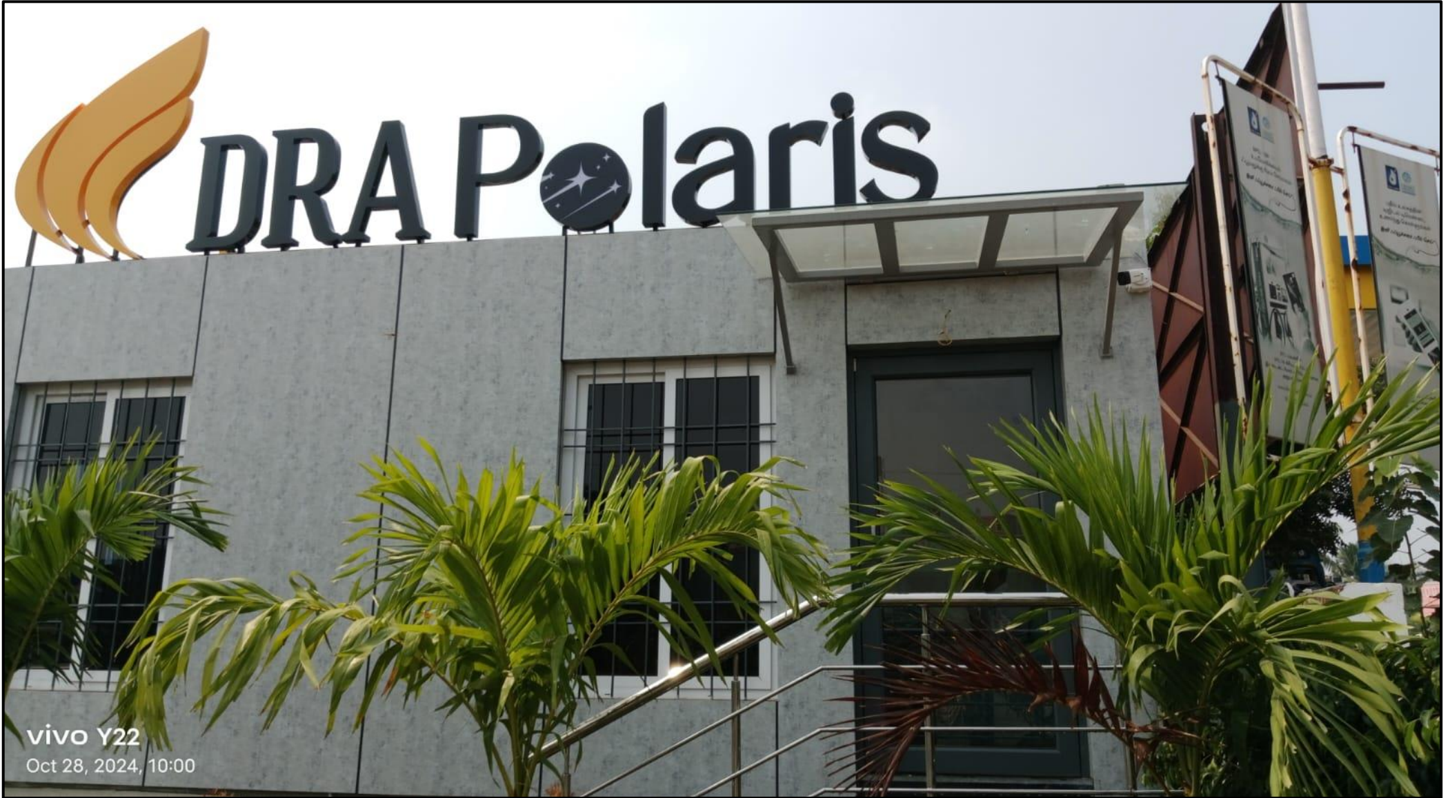
Sales office canopy glass installation work completed
