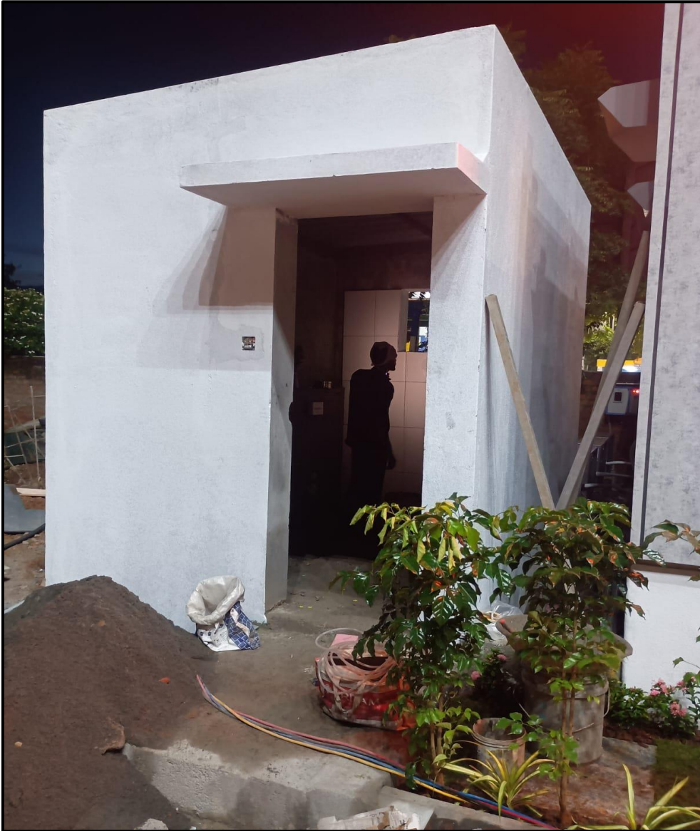
Toilet primer and texture putty work completed
