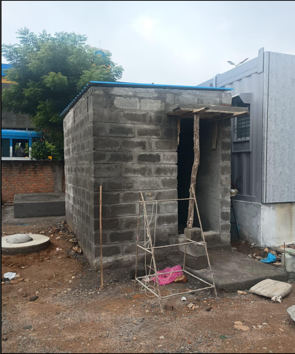
Toilet roof GI sheet installation work completed
