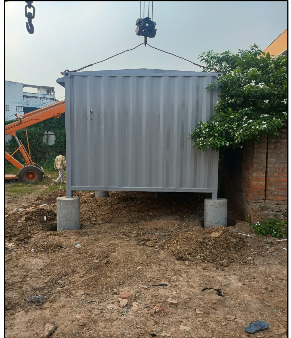
Site office foundation work & erection work completed
