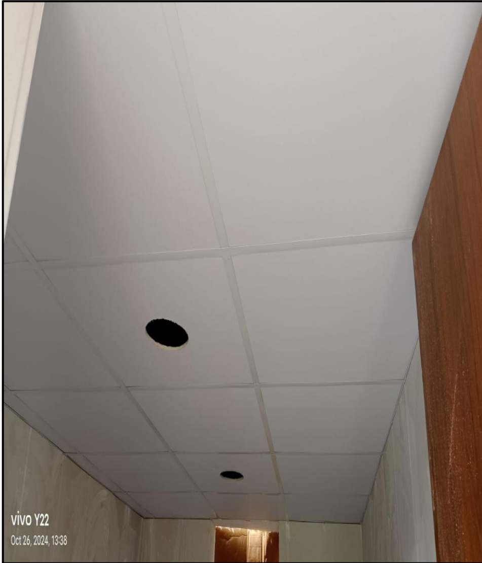
Toilet false ceiling work completed
