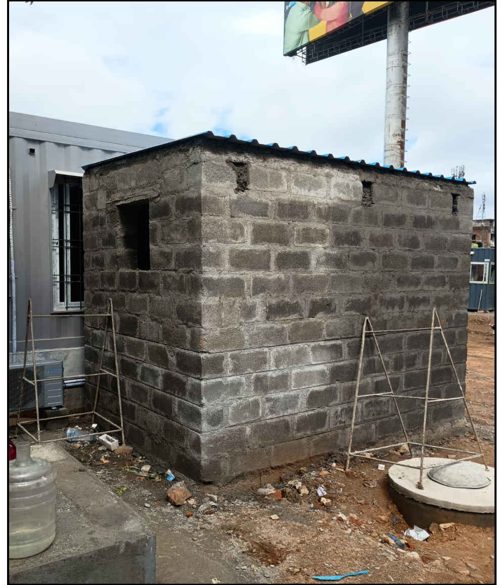
Toilet roof GI sheet installation work completed
