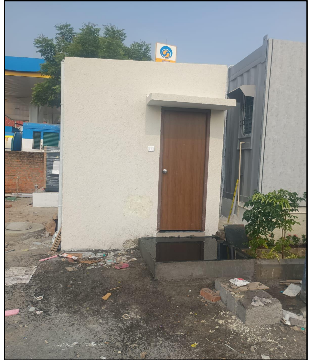
Toilet primer and texture putty work completed
