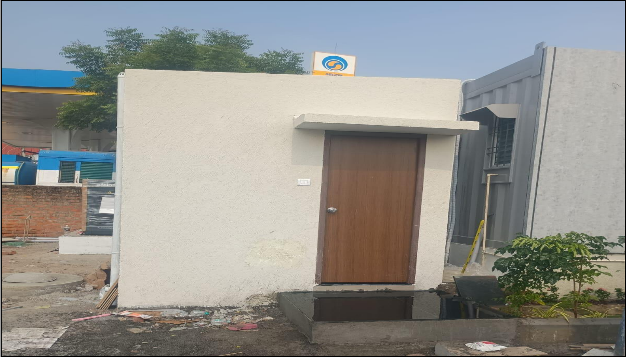
Toilet door installation work completed
