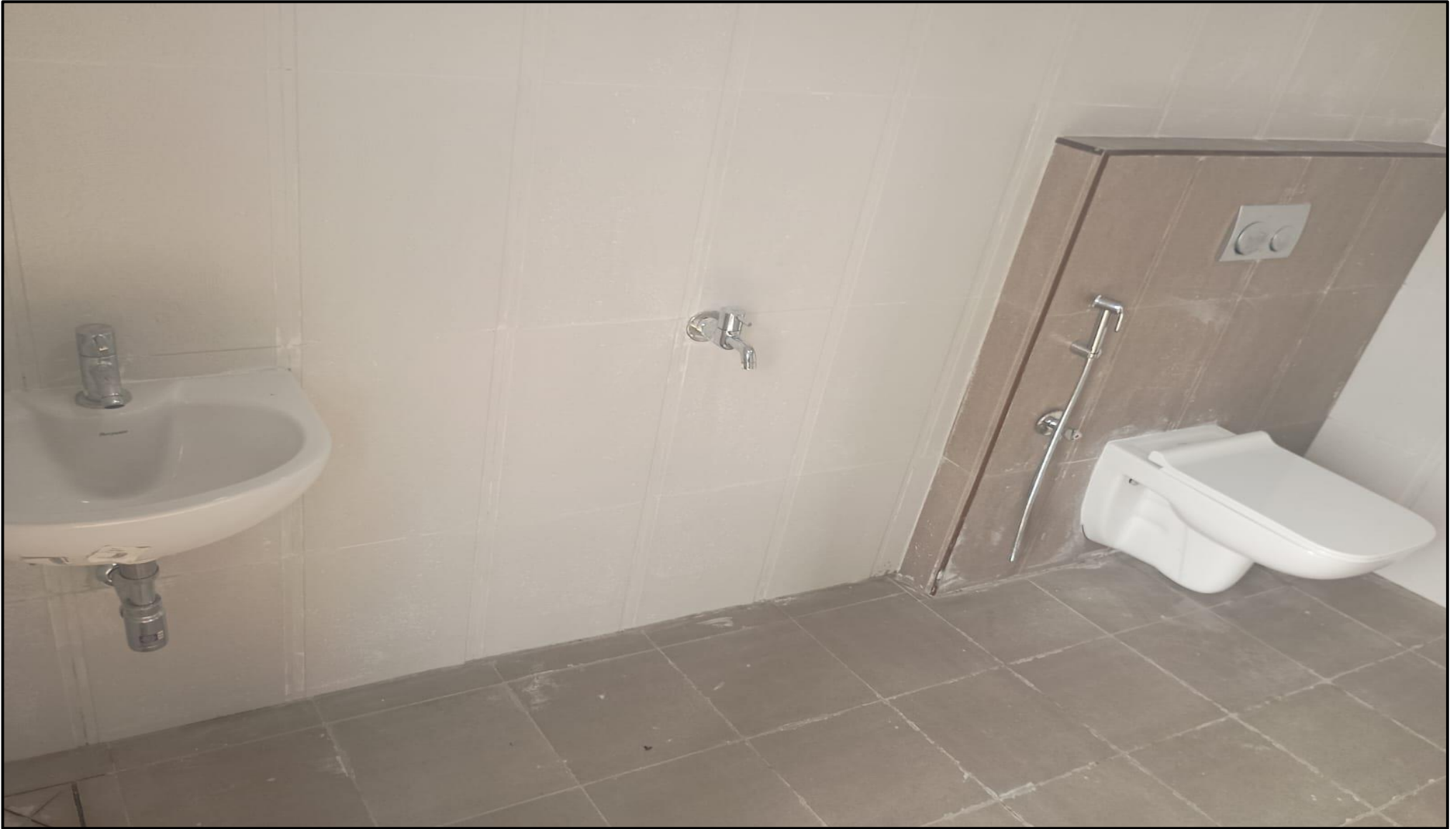
Toilet CP fittings work completed
