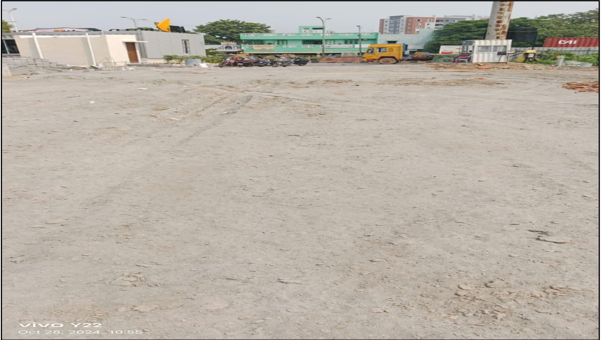
Site office pooja area dust levelling work completed
