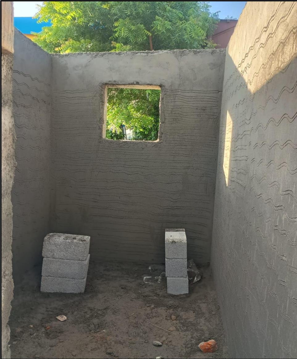
Toilet inner & external plastering work completed
