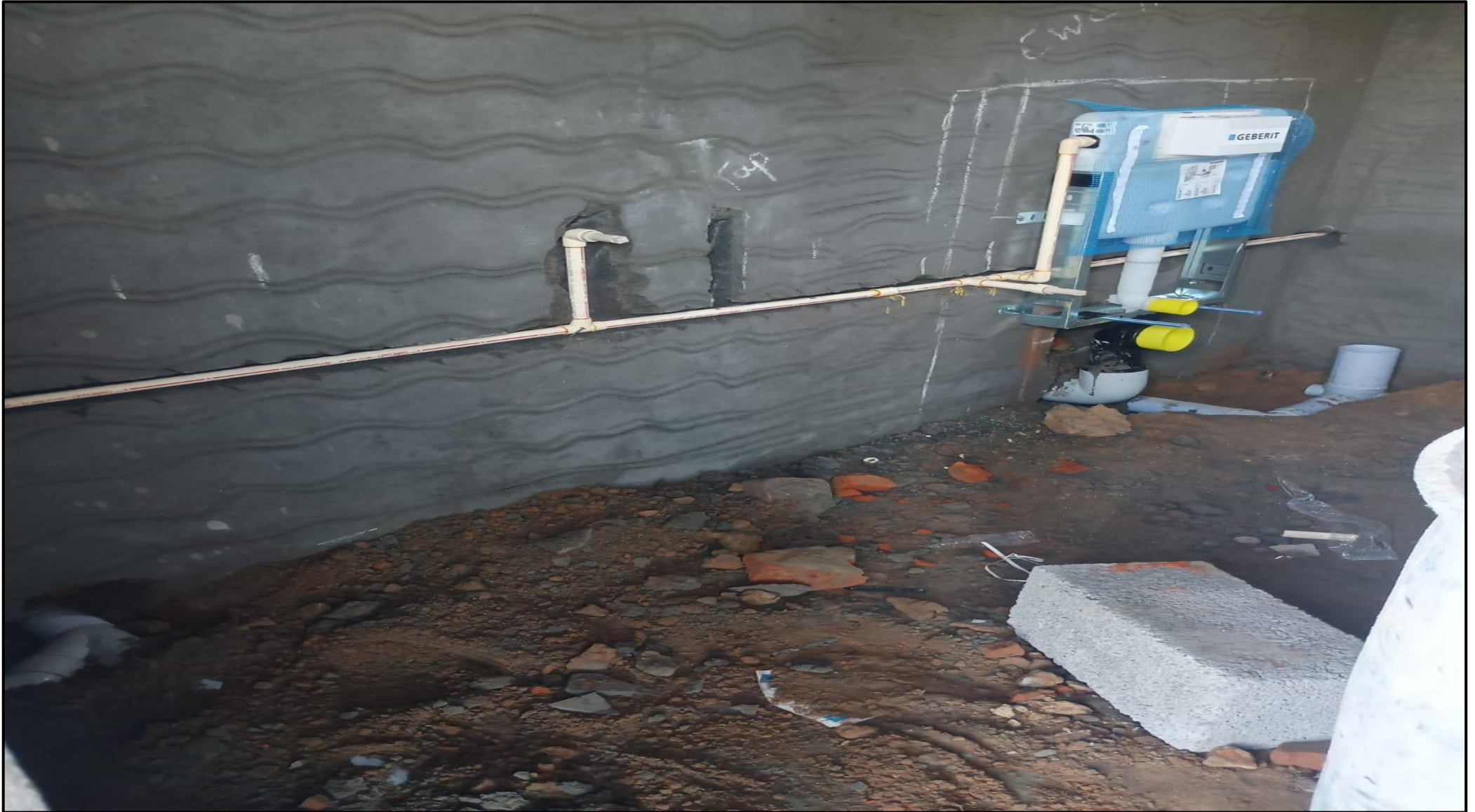
Toilet plumbing concealed work completed
