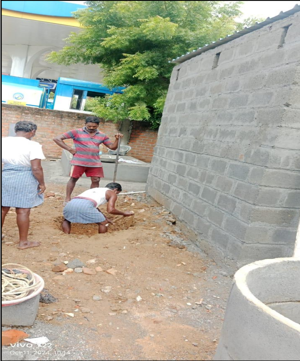
Toilet soak pit installation work completed
