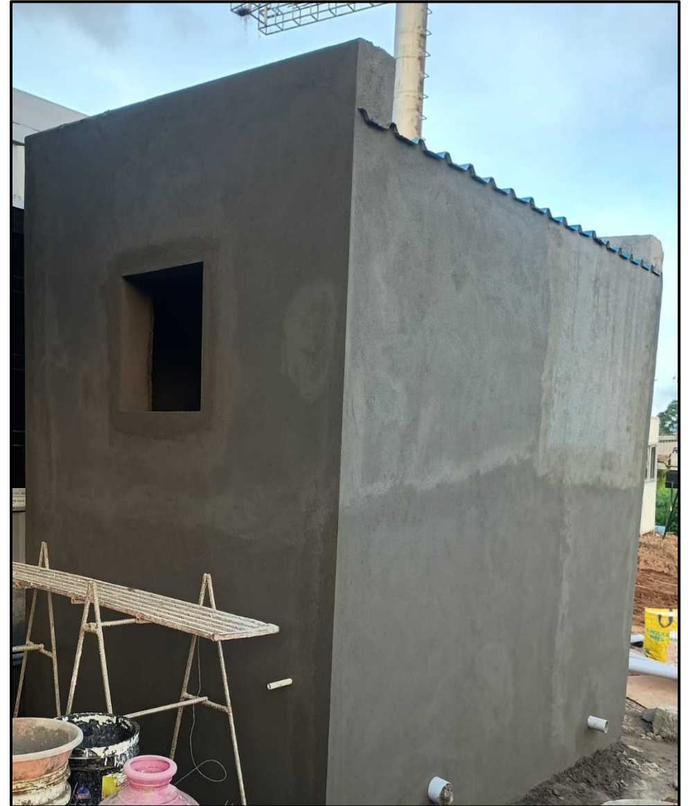
Toilet inner & external plastering work completed
