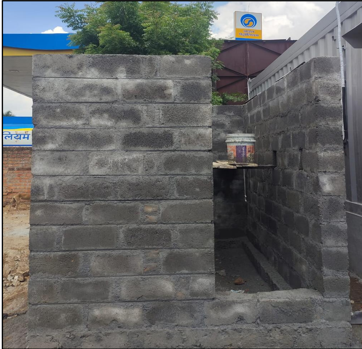
Sales Office Toilet Lintel level Blockwork in progress.
