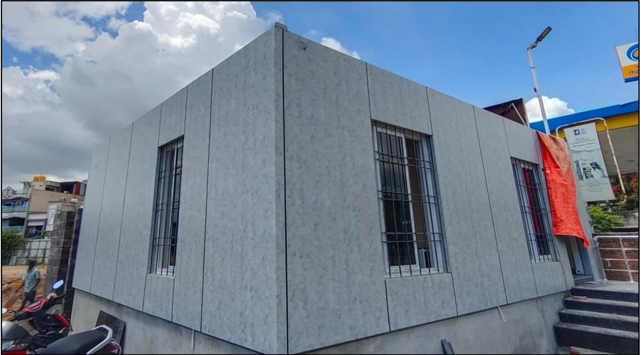
Sales Office ACP Cladding Completed
