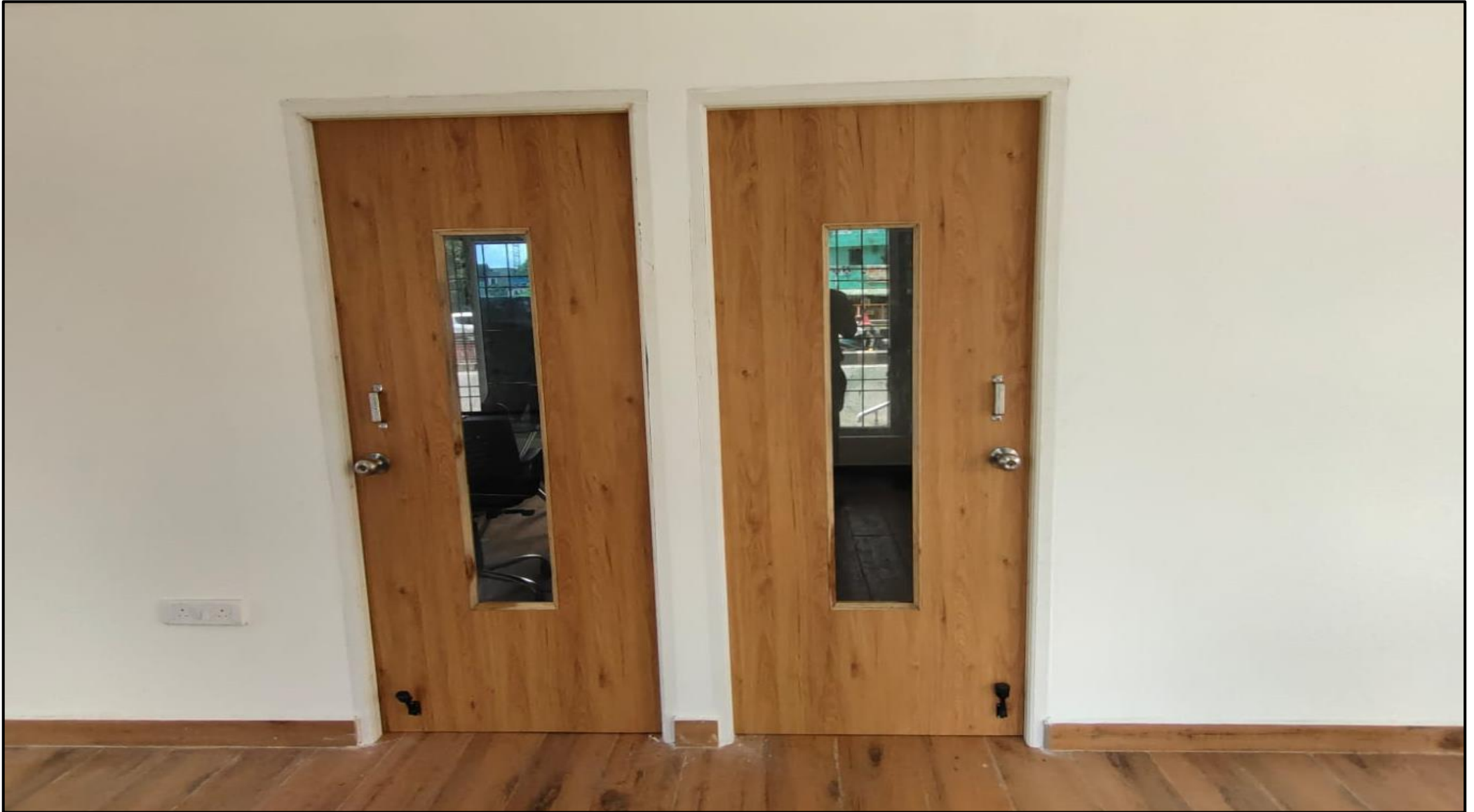
Sales Office Internal door fixing work Completed.
