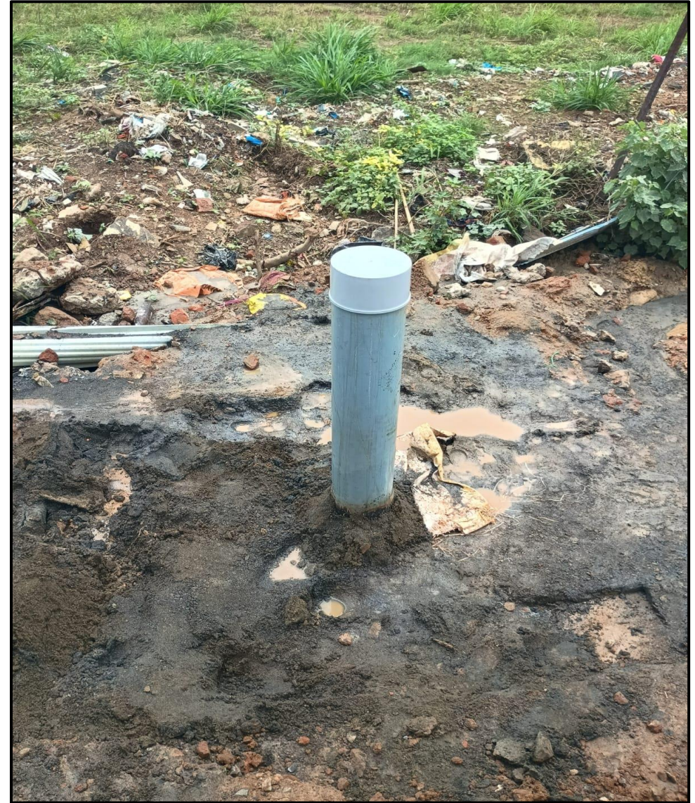
Borewell Drilling 1nos work Completed.
