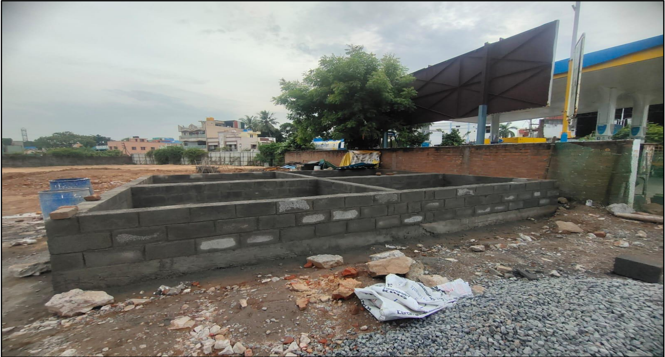
Sales Office Plinth beam above Blockwork completed.
