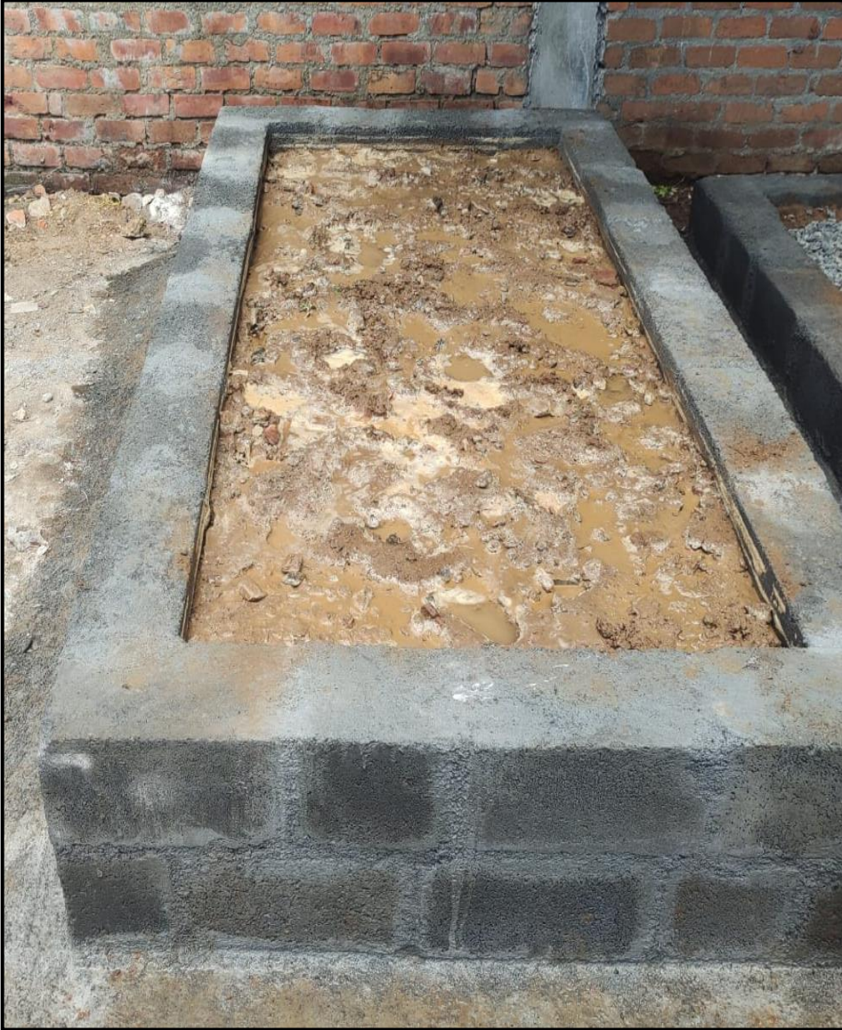
Sales Office DG Bed, Water Tank & Booster Pump Pedestal work in progress.
