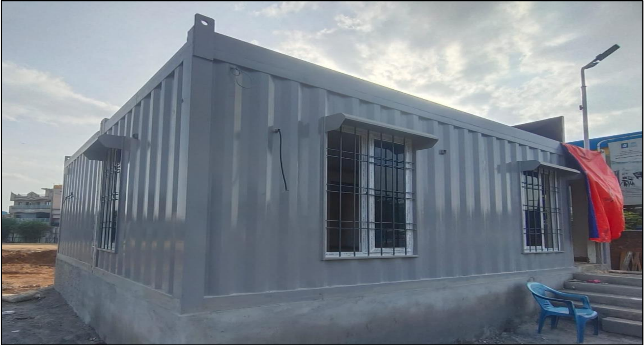
Sales Office Shifting & Erection work Completed.
