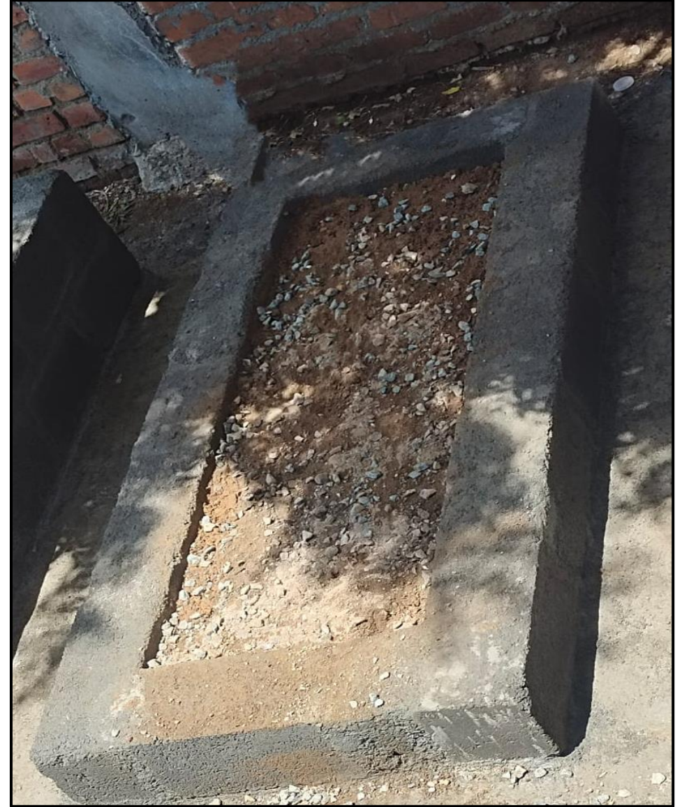
Sales Office DG Bed, Water Tank & Booster Pump Pedestal work in progress.
