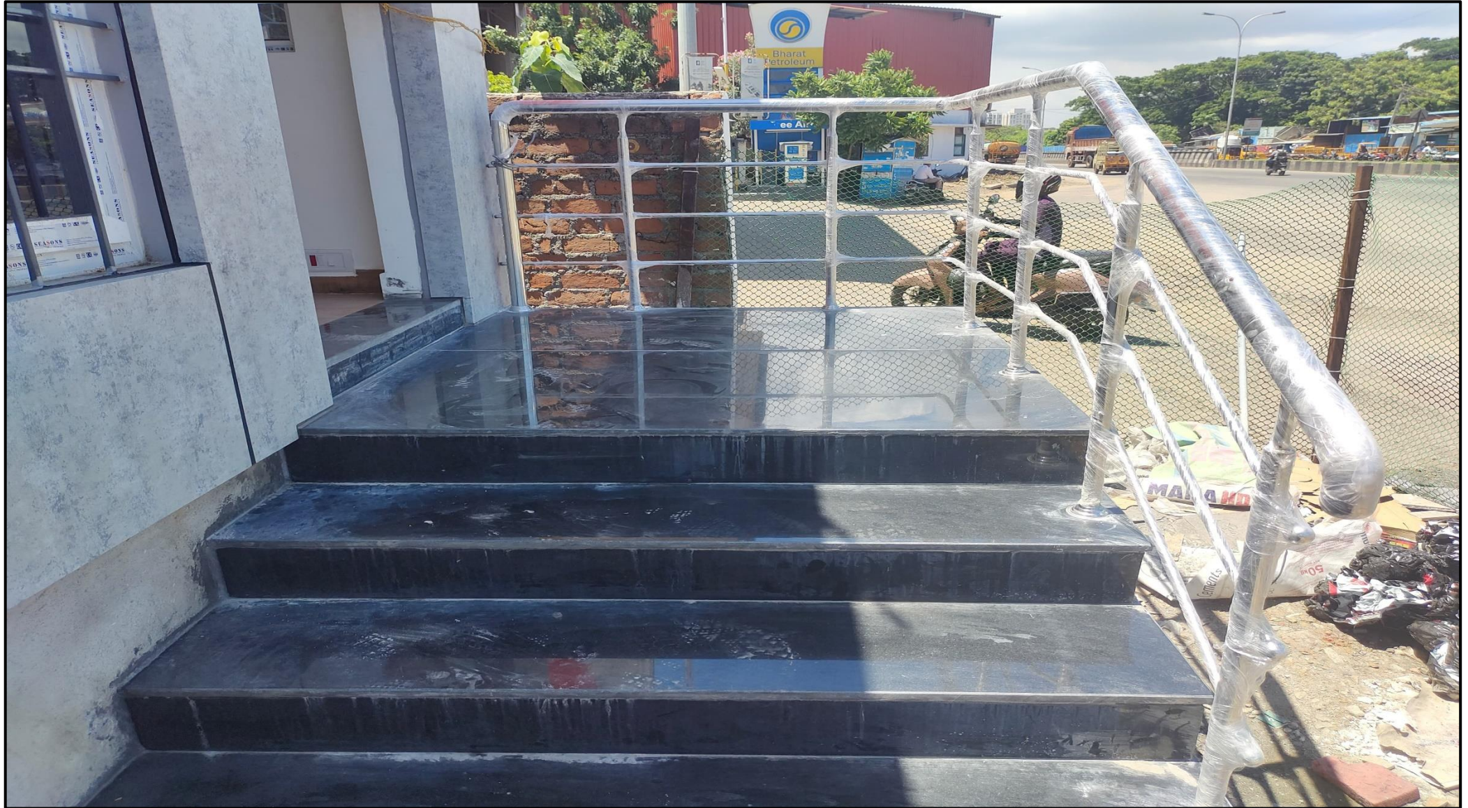
Sales office Staircase Granite & Handrail work Completed.
