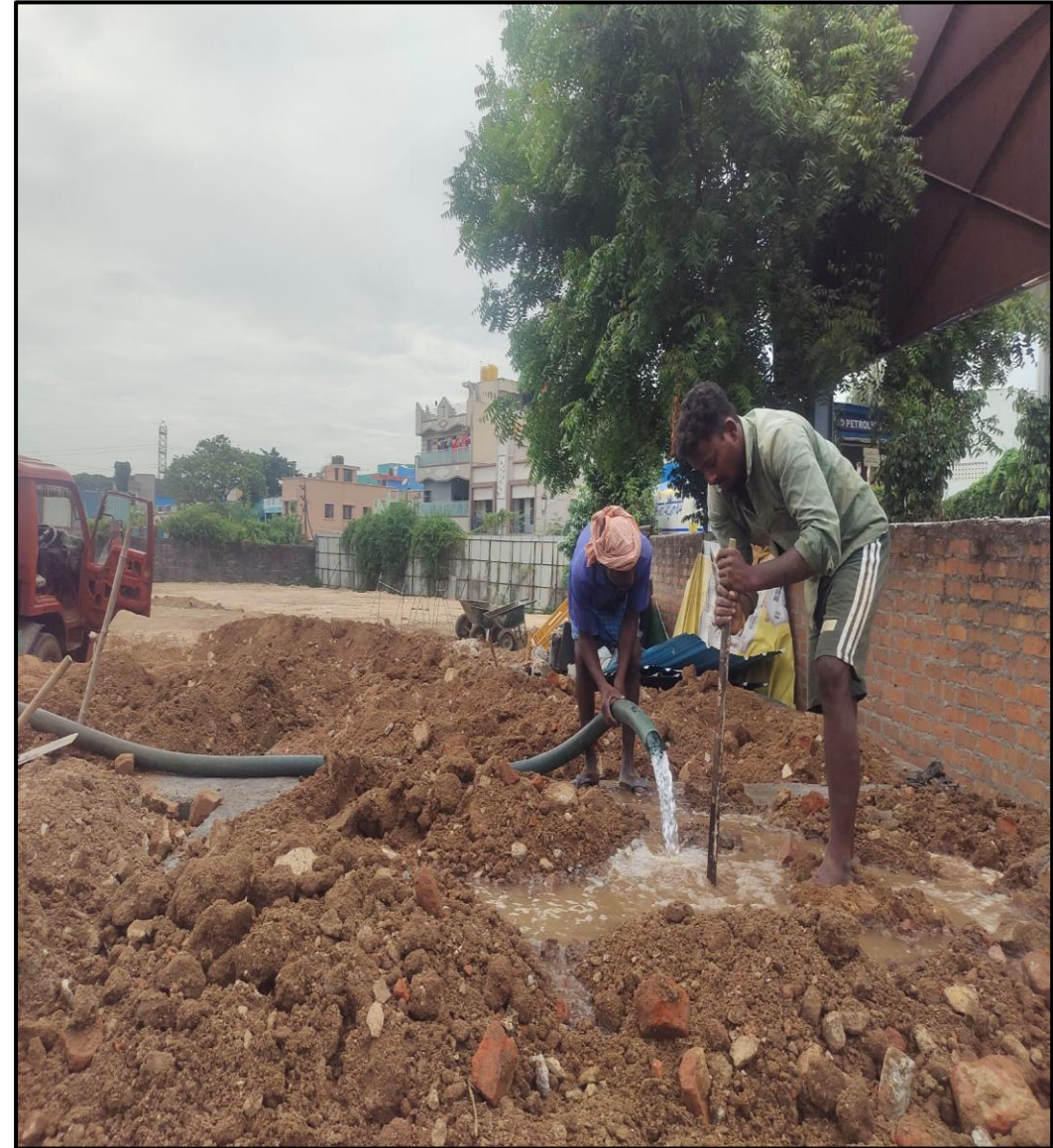
Sales Office Blockwork Inside Soil filling and Consolidation work completed.
