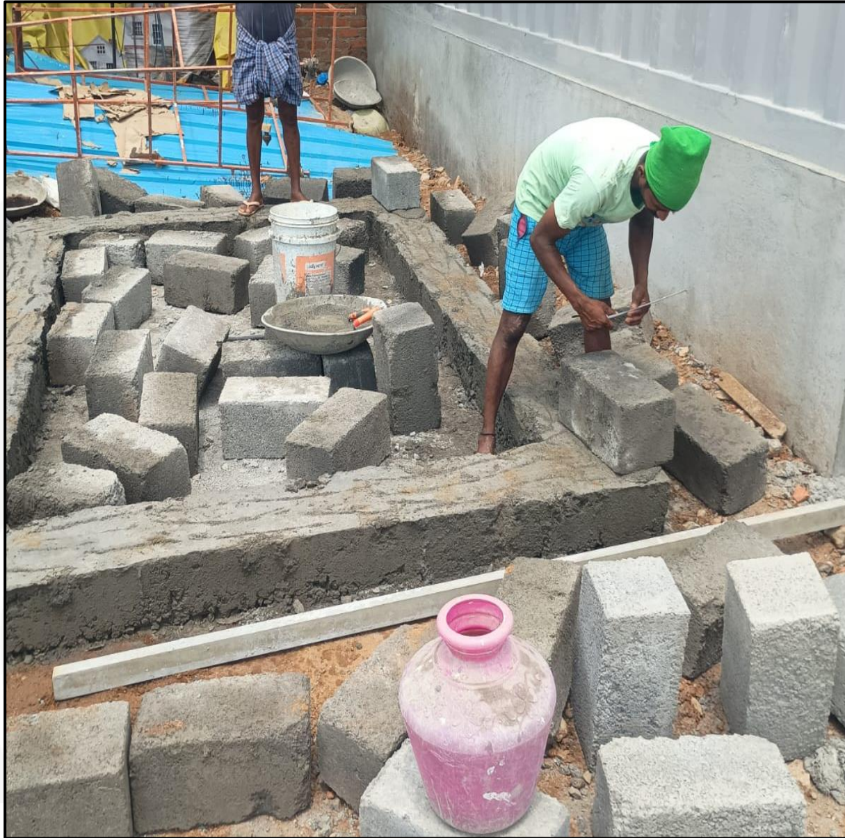
Sales Office Toilet Plinth Beam work Completed & Blockwork in progress.
