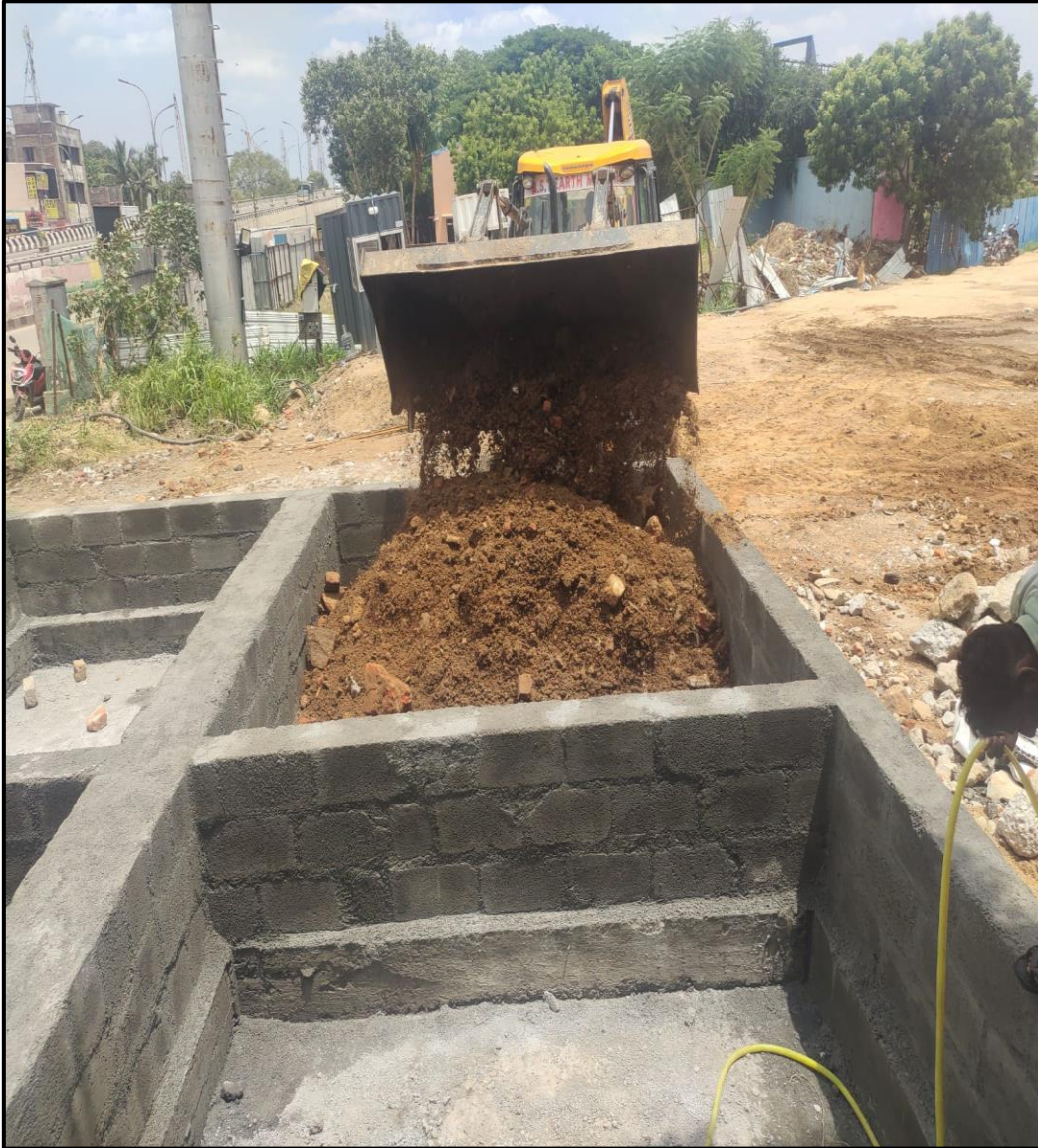
Sales Office Blockwork Inside Soil filling and Consolidation work completed.
