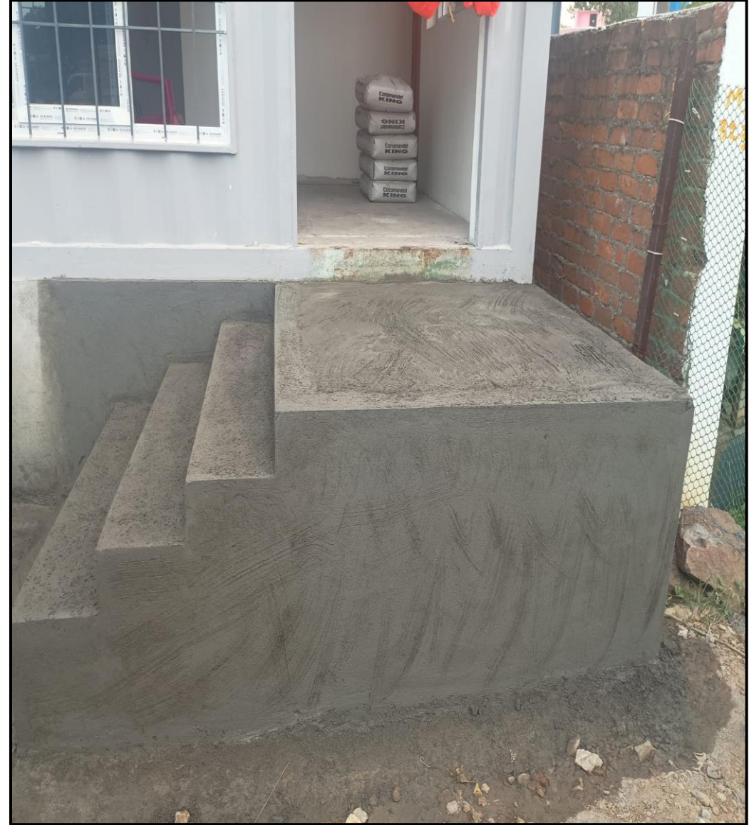
Sales Office Staircase Blockwork & Plastering work Completed.
