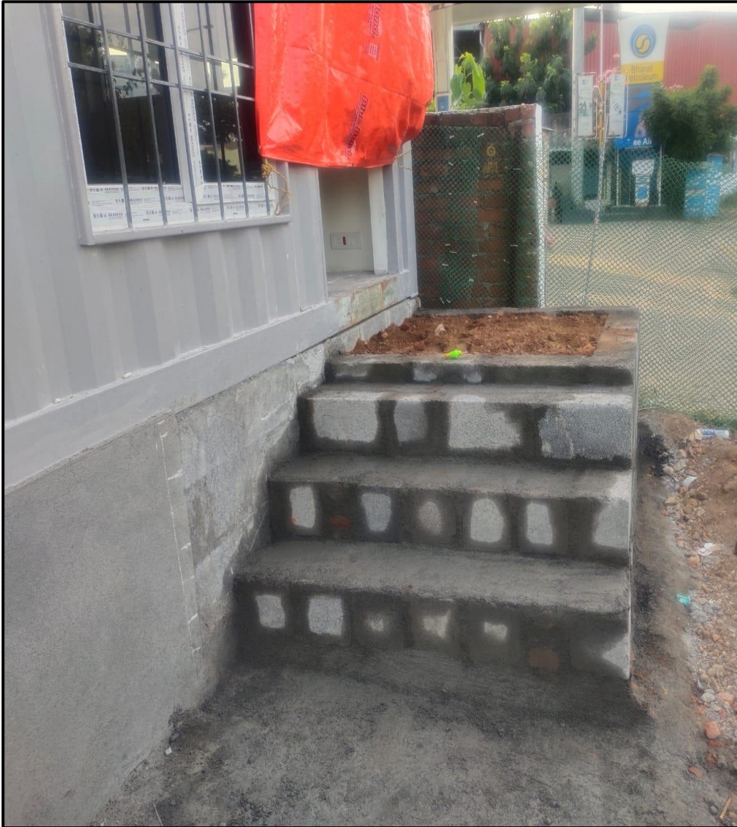
Sales Office Staircase Blockwork & Plastering work Completed.
