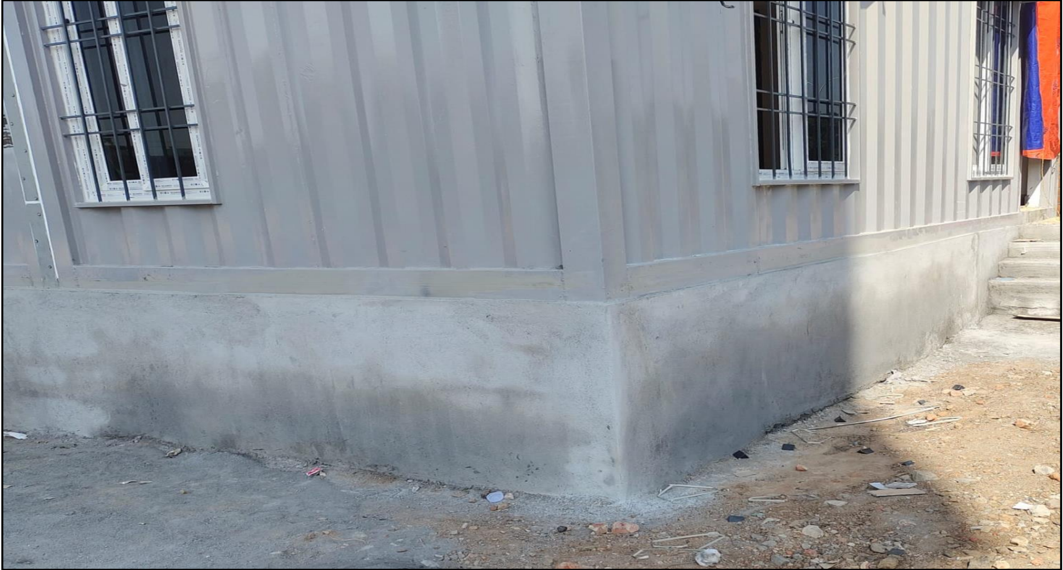
Sales Office External Below Blockwork Plastering work Completed.
