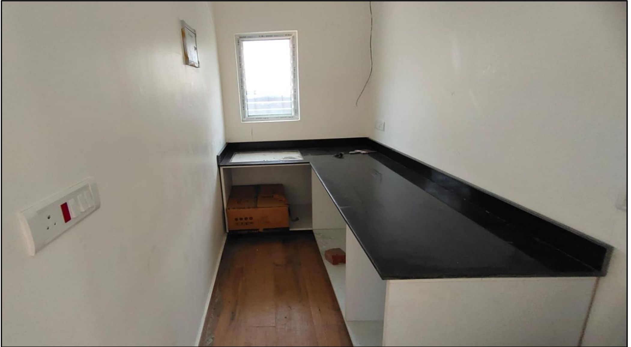
Sales Office Pantry Interior work in progress.
