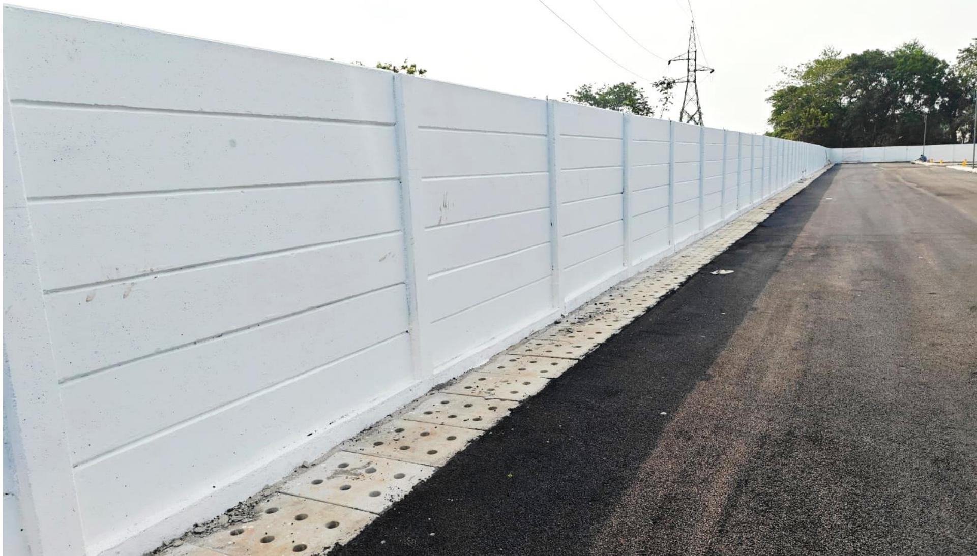
Pre-Cast Compound Wall Paint 2 nd Coat WIP
