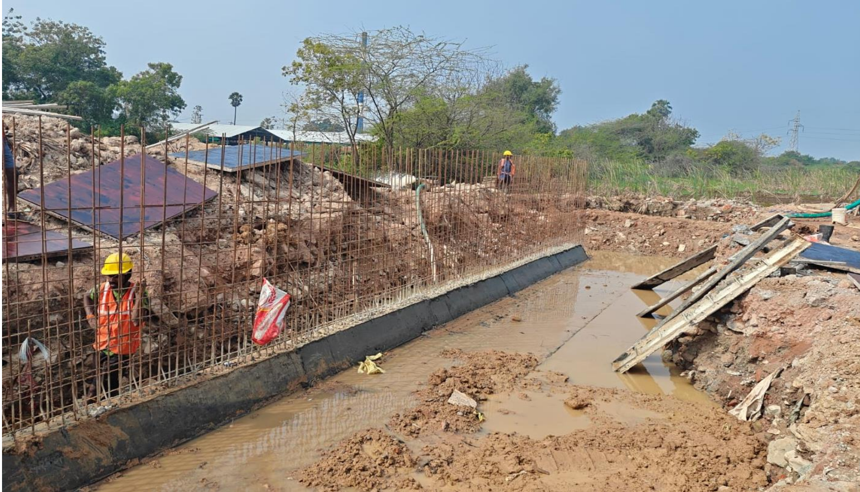
South Side Raft & Haunch Work In Progress
