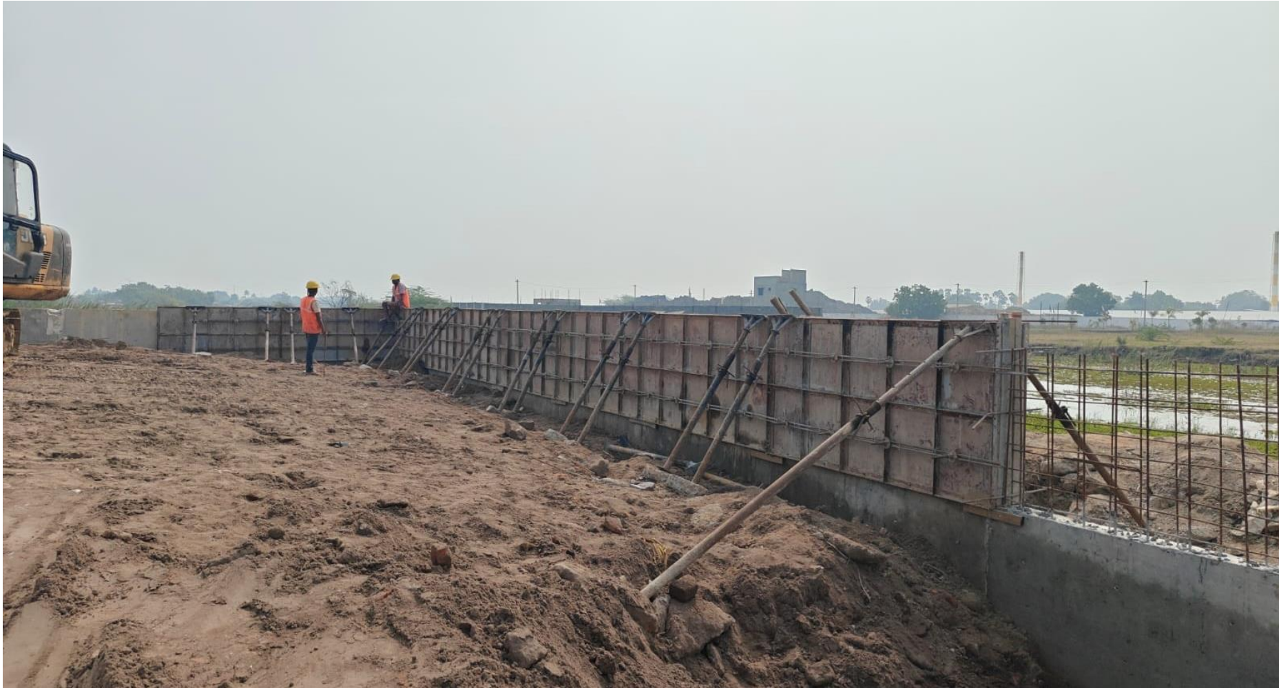
South Side 2 nd Lift Concrete WIP
