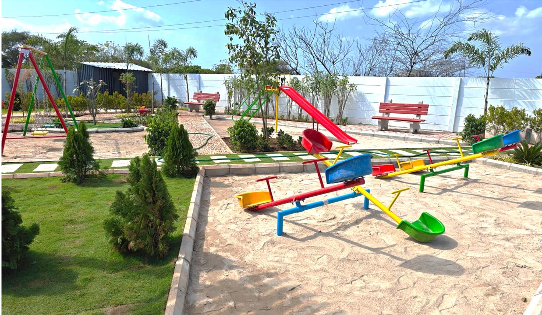
OSR Works Completed
