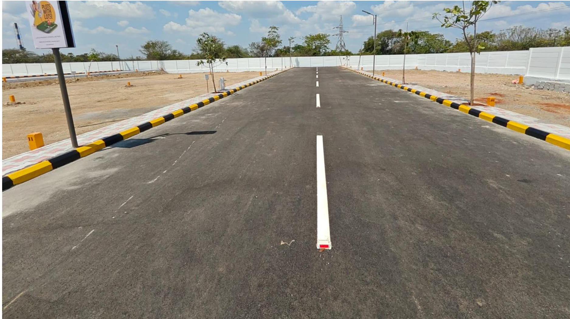
Bliss Street Works Completed
