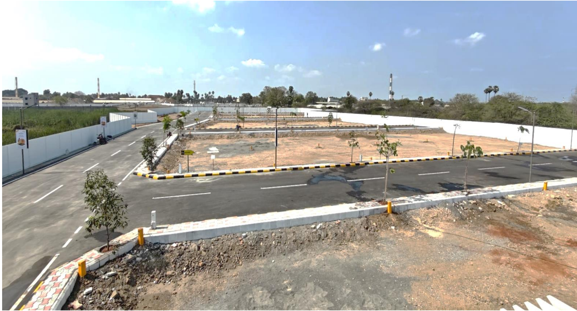
PHASE-II AERIAL VIEW
