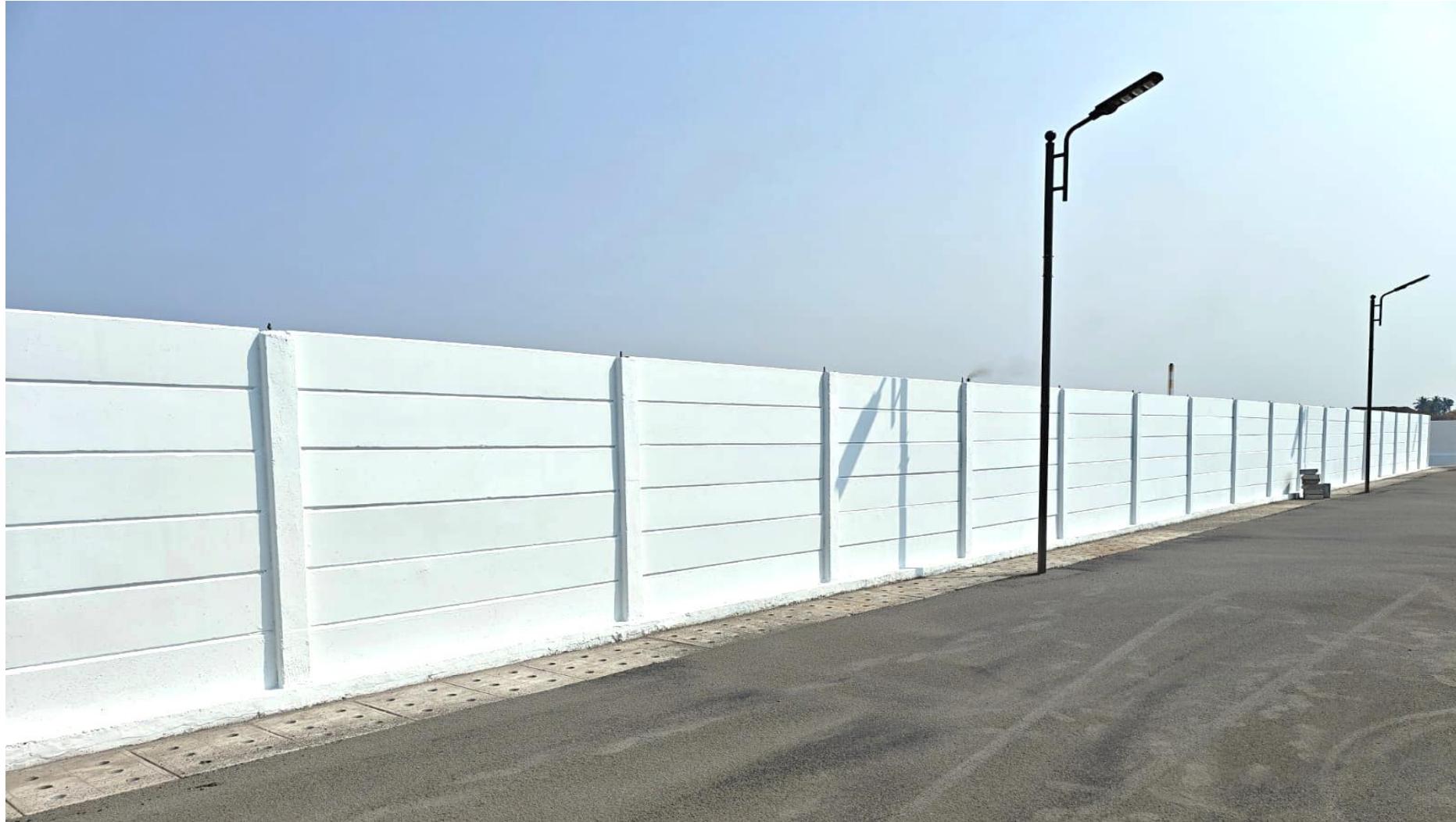
Pre-Cast Compound Wall Painting Works Completed
