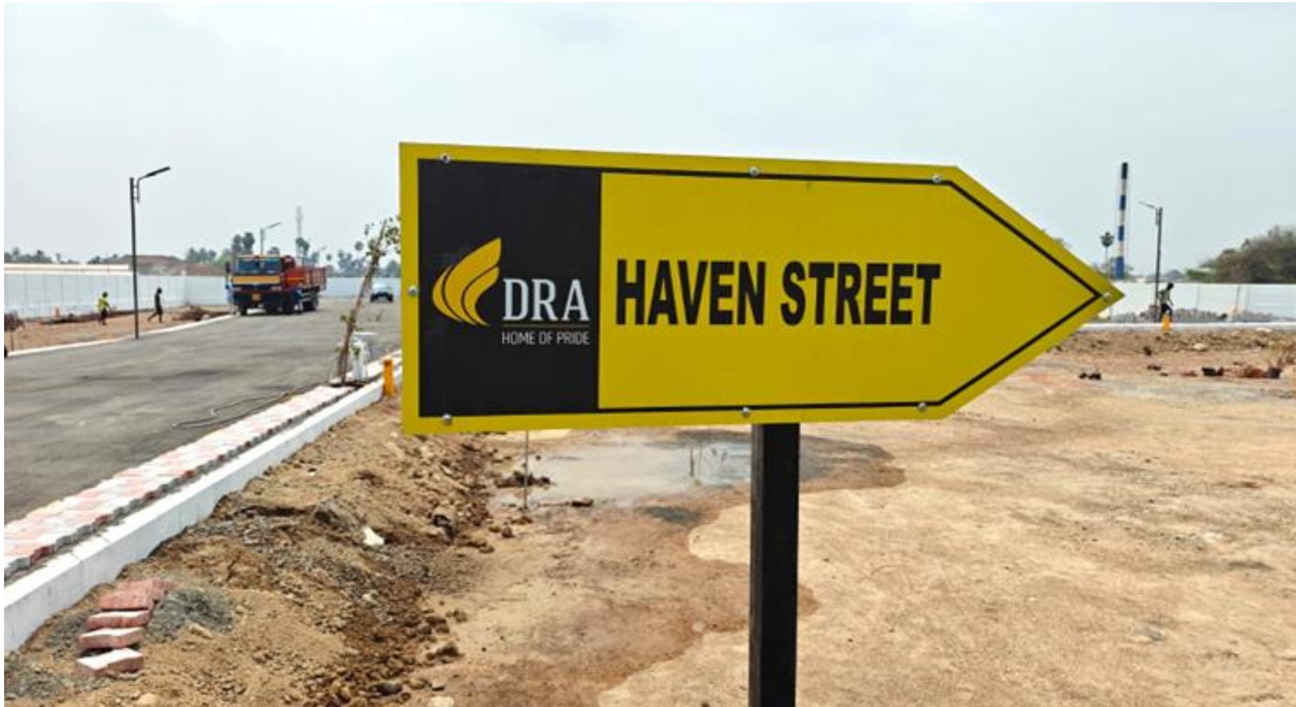
Street Board Erection Works Completed
