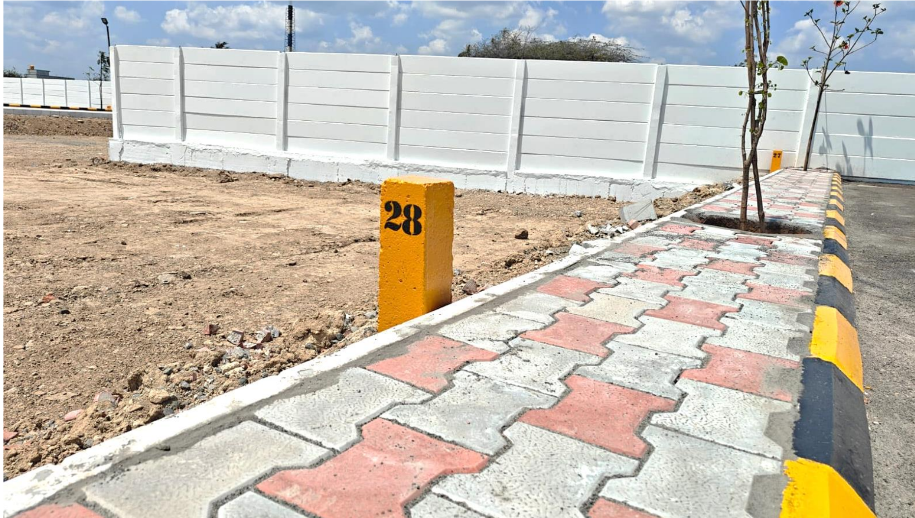
Plot Stone Painting & Numbering Works Completed
