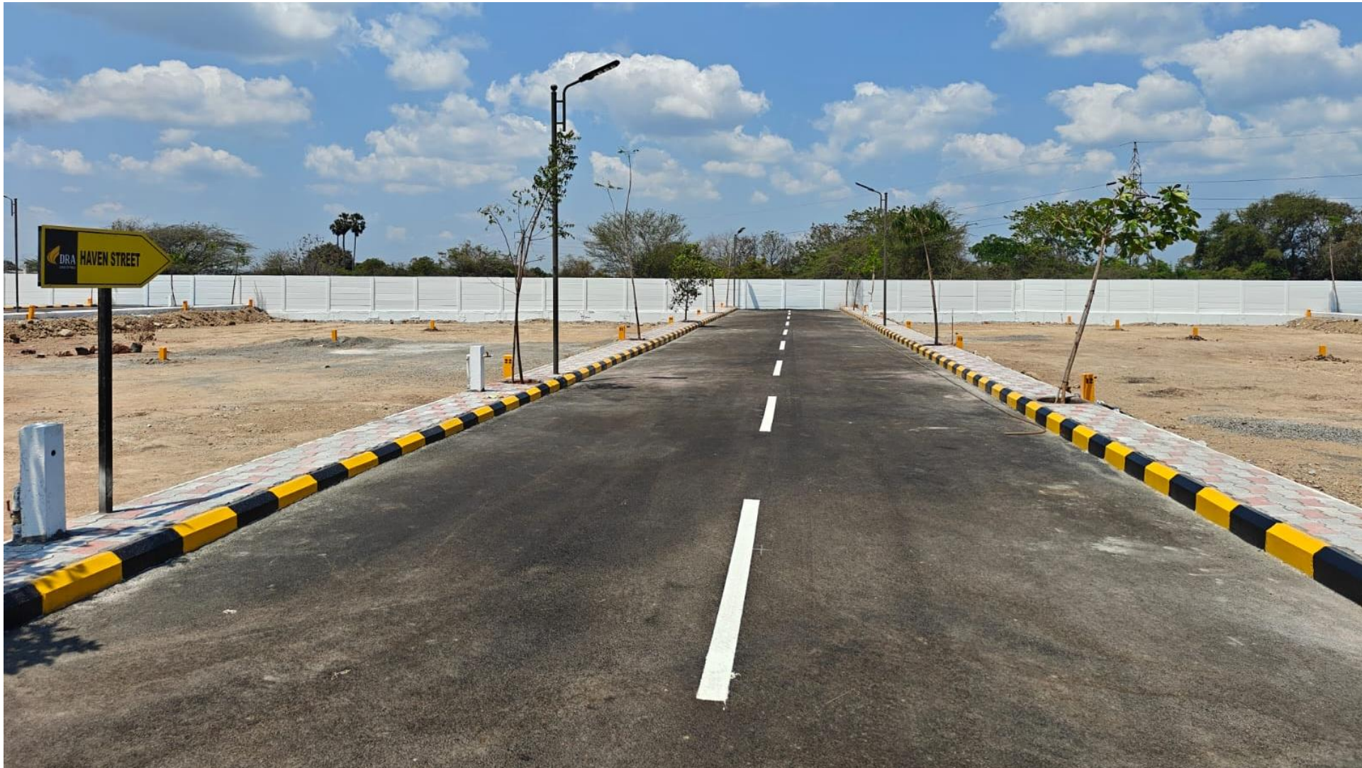
Haven Street Works Completed
