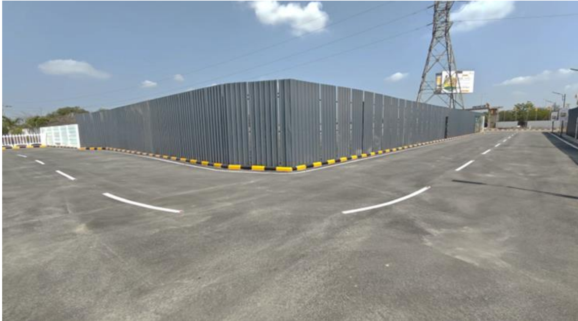
Connecting Road Barricade Works Completed
