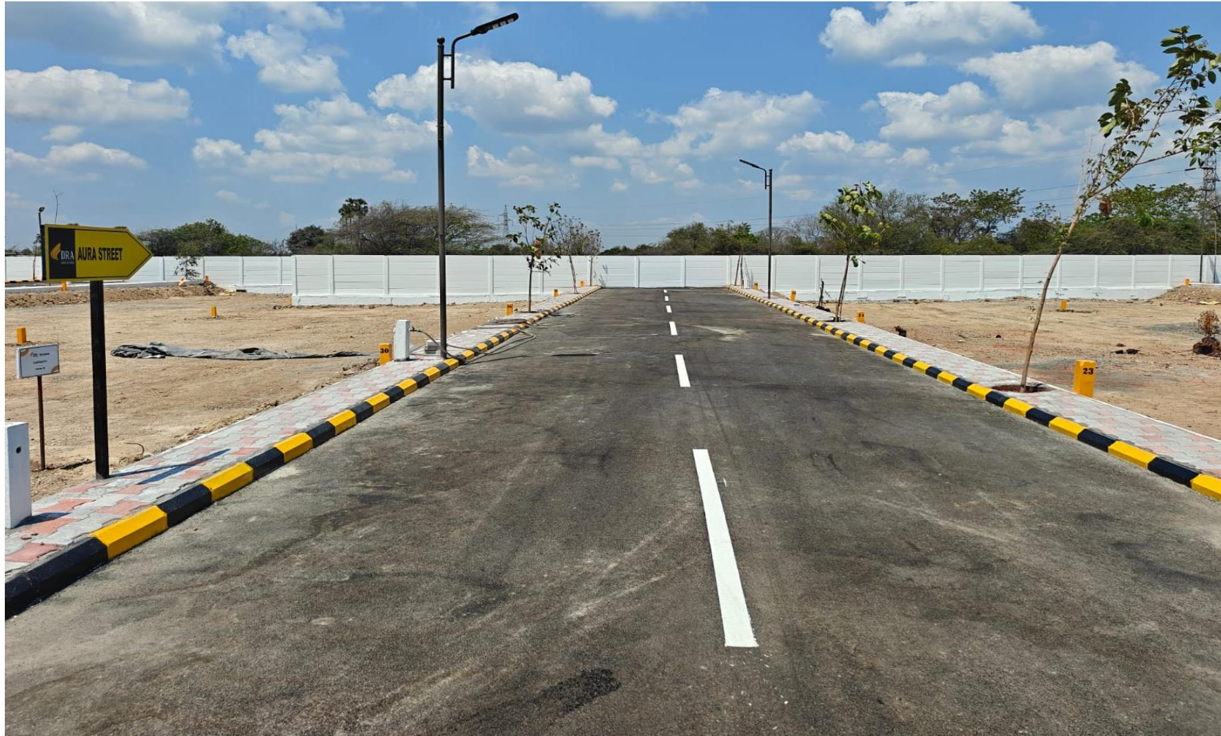
Aura Street Works Completed
