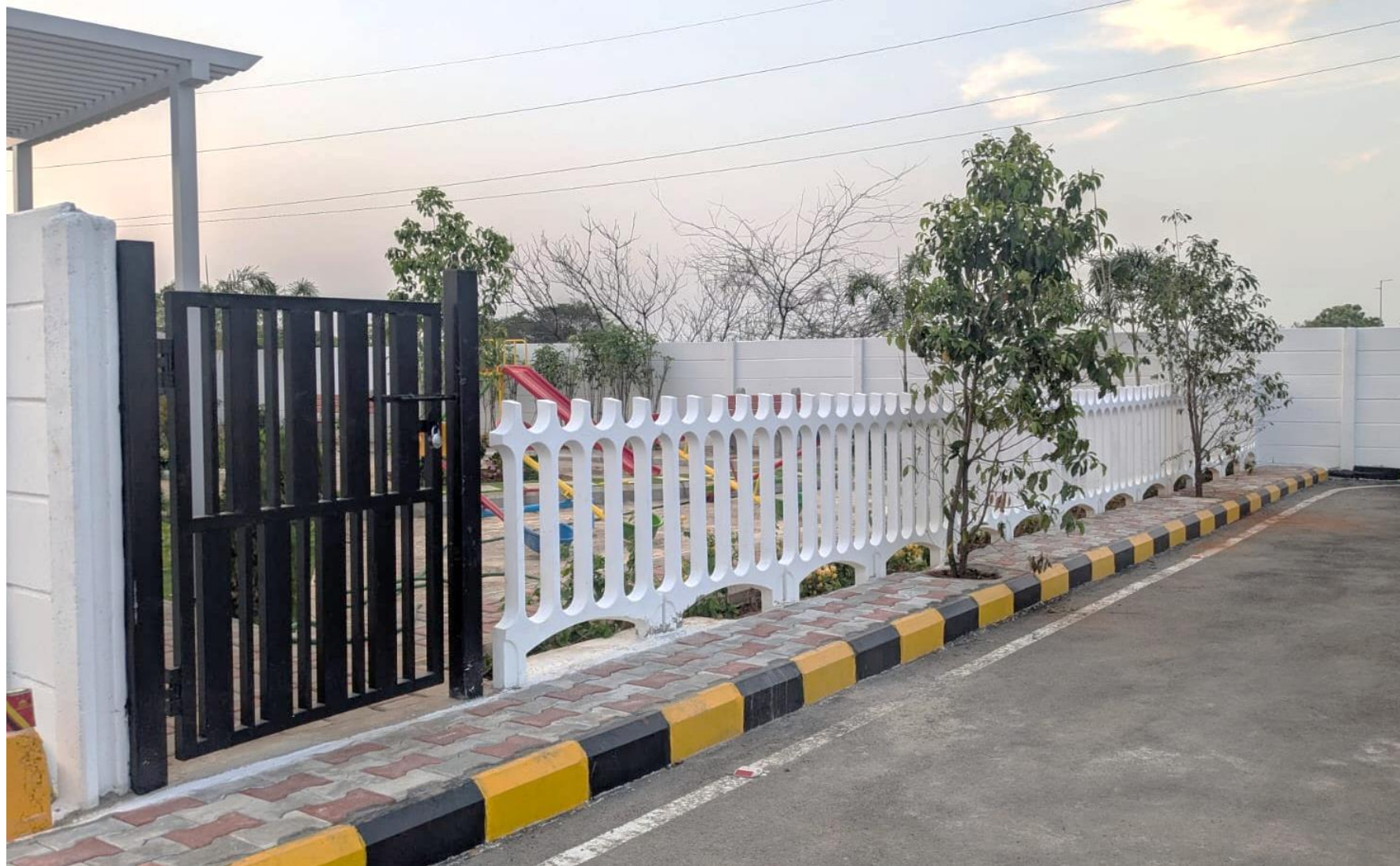
OSR Picket Fencing Works Completed
