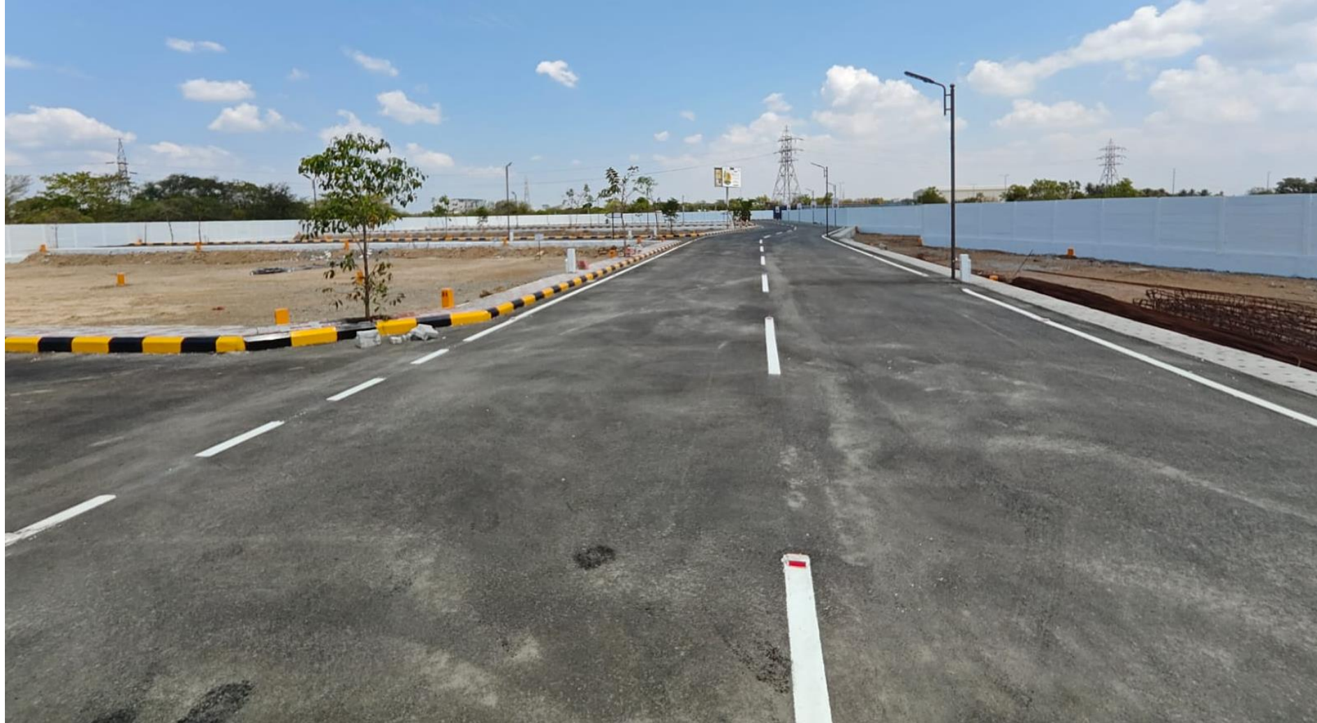
Eden Street Works Completed
