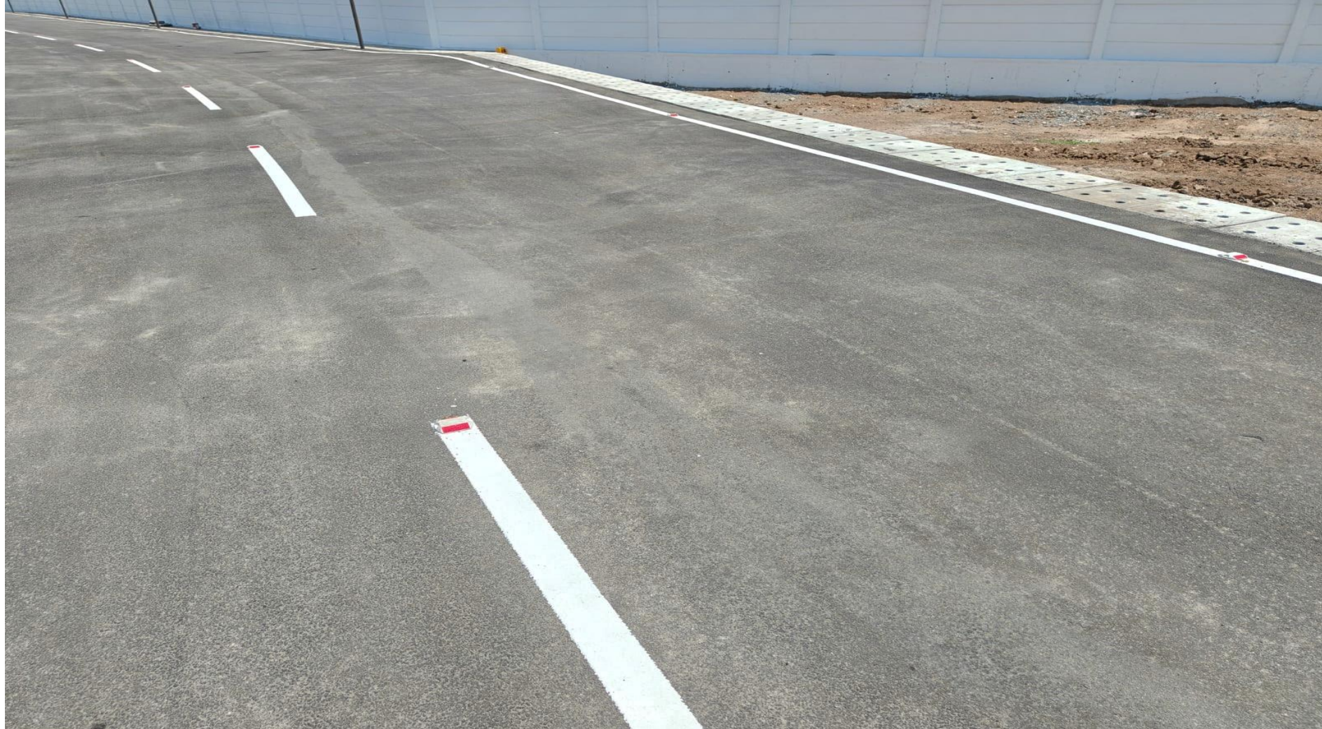
Thermoplast Painting & Reflective Studs Works Completed
