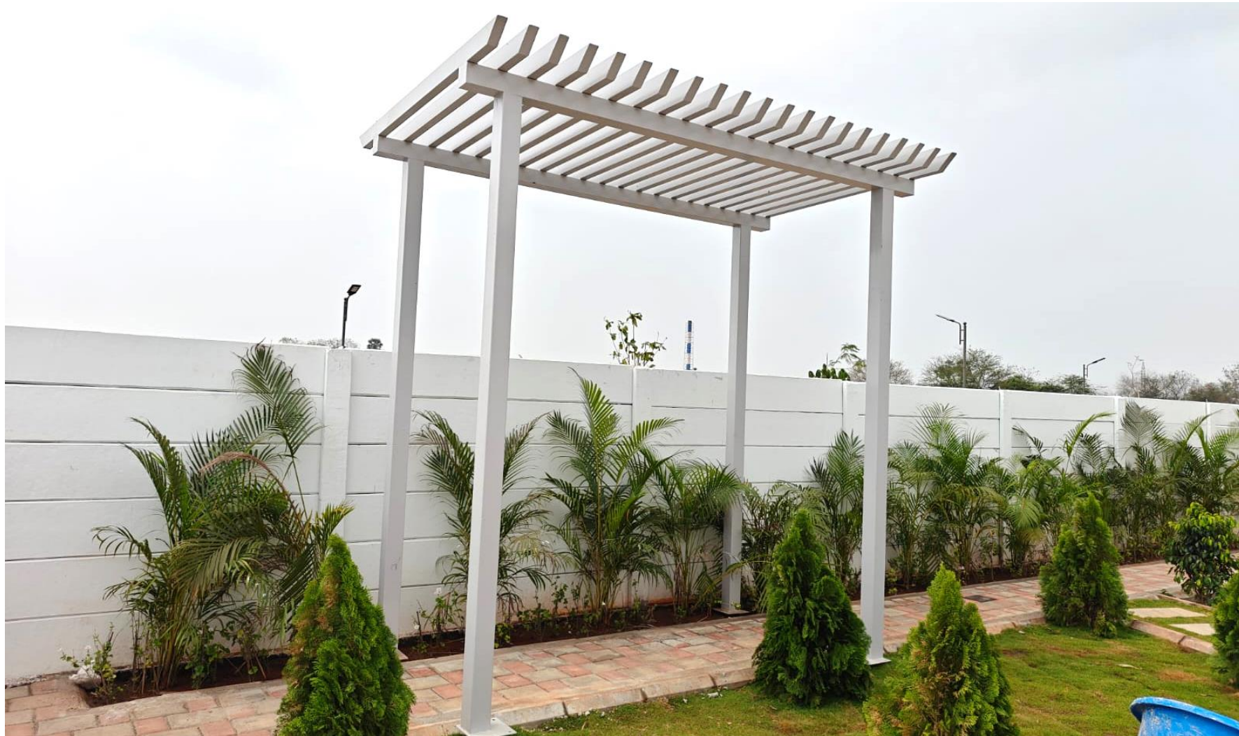
OSR MS Pergola Works Completed
