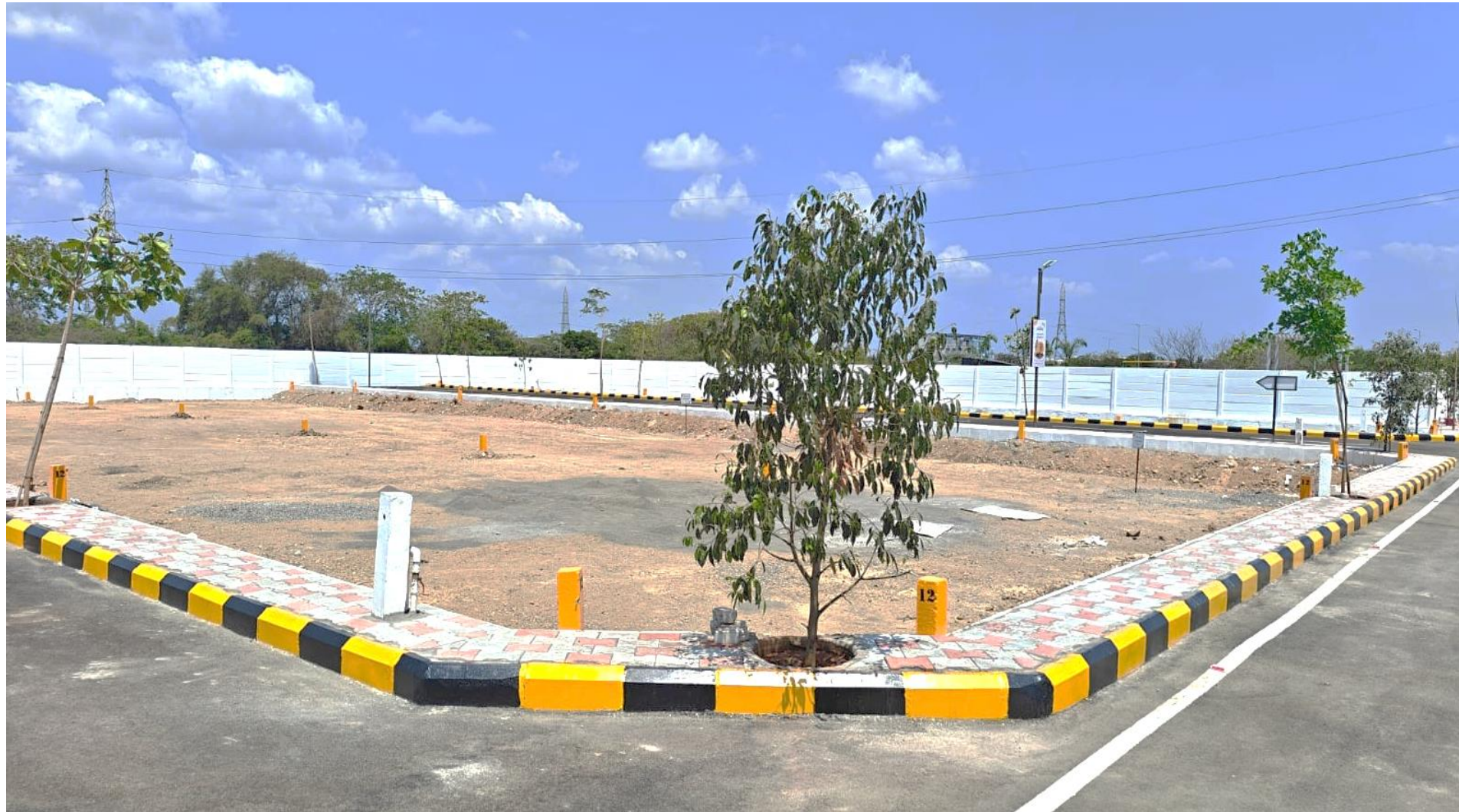
Pathway Landscape Works Completed
