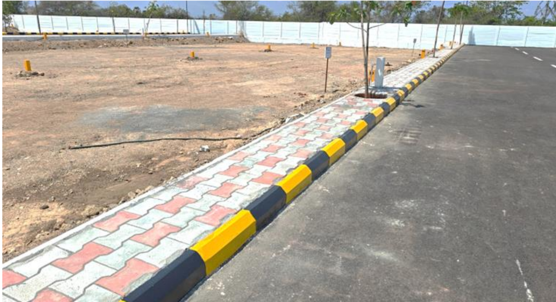
Pathway Works Completed
