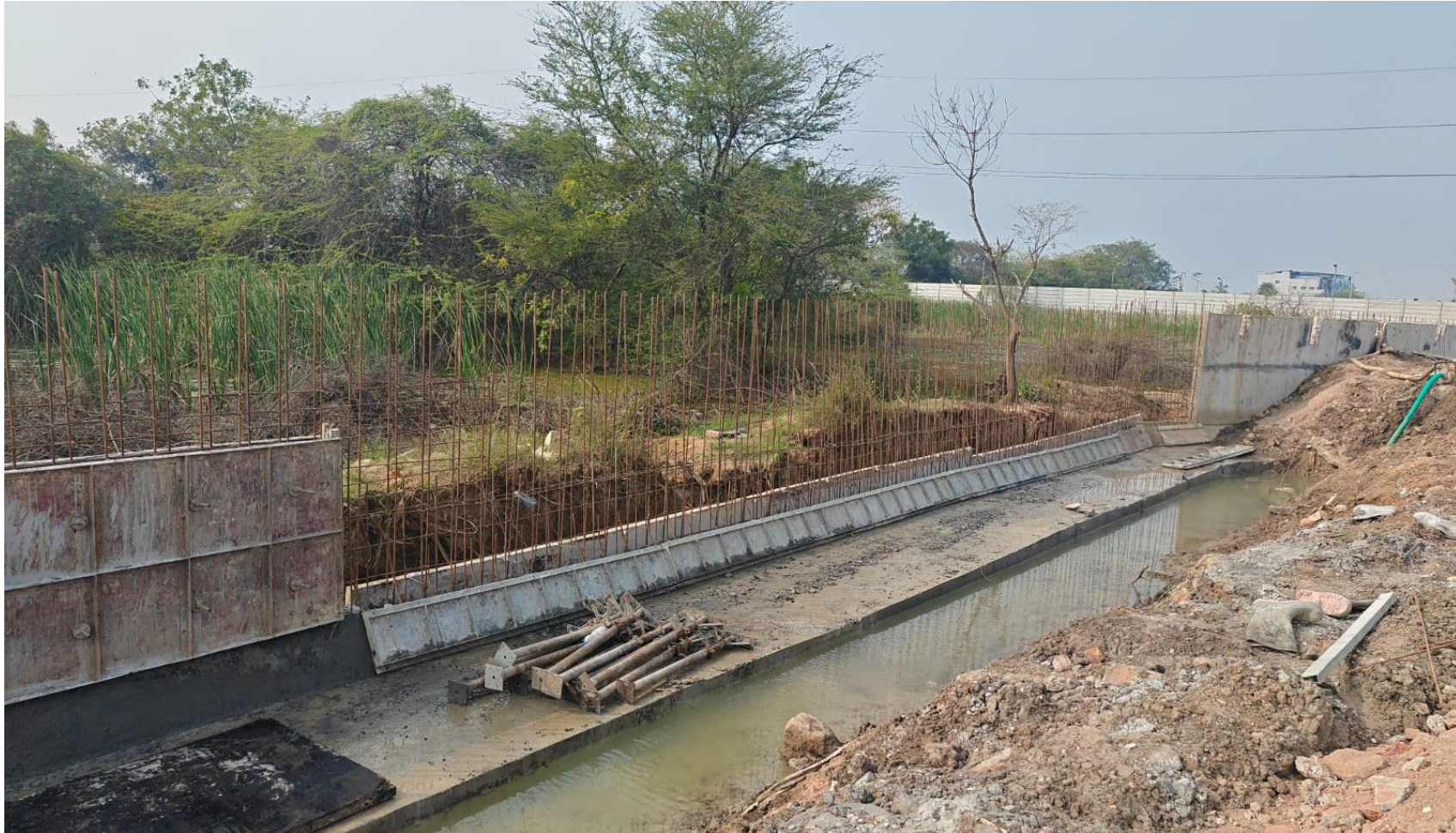
West Side Raft & Haunch Work In Completed
