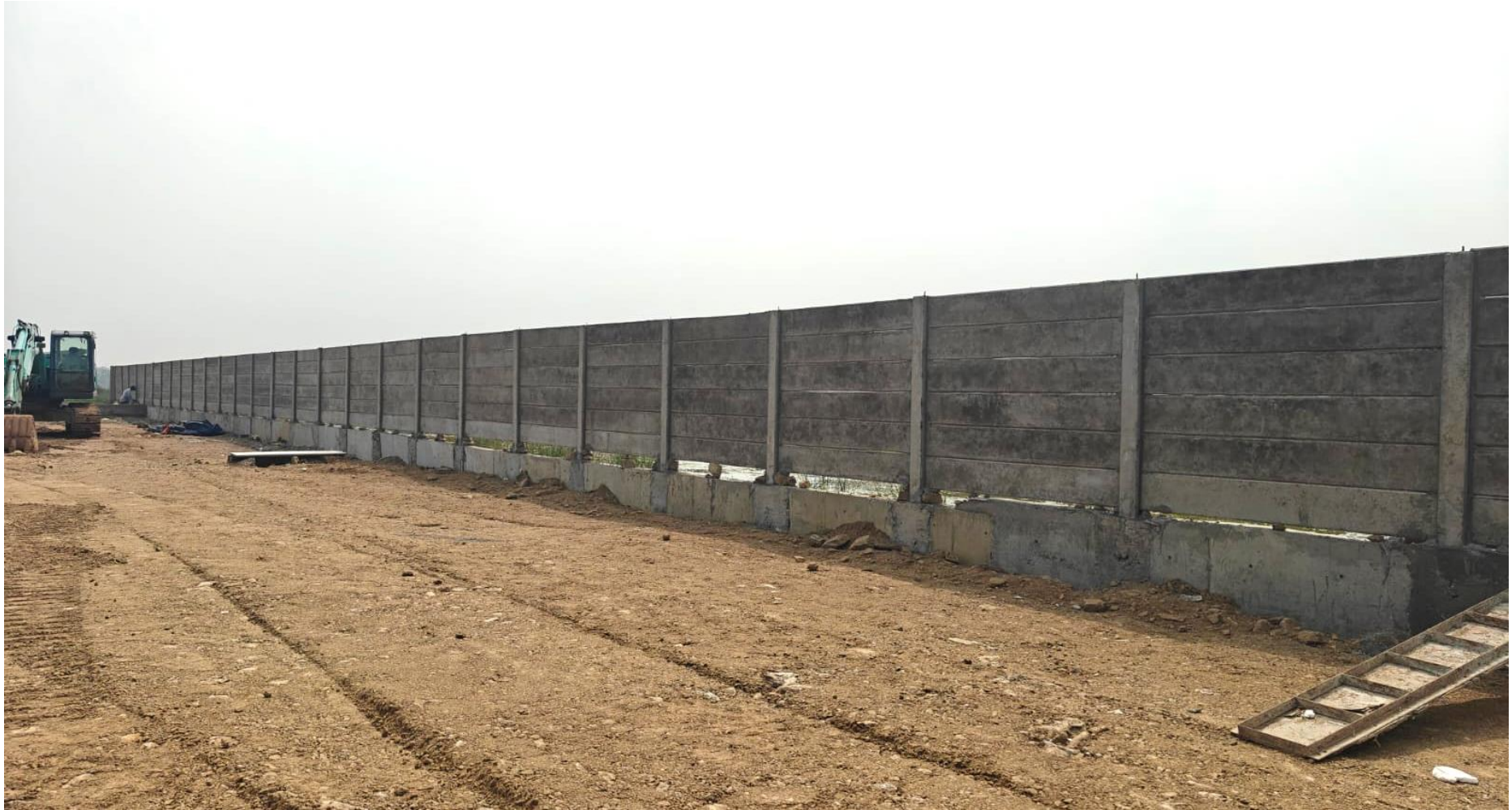
South Side Pre-cast Compound Slab Fixing Completed
