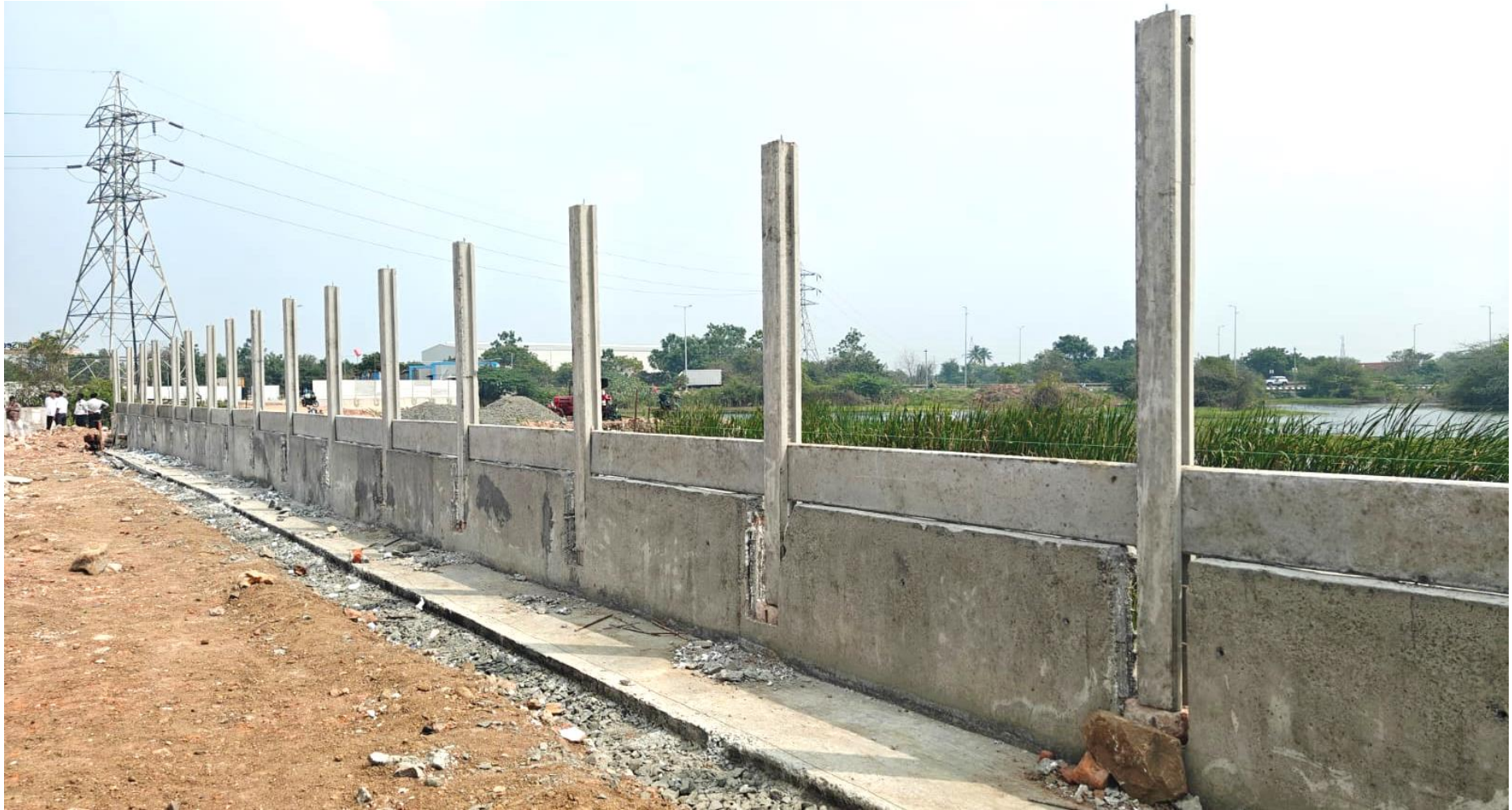
East Side Pre-cast Compound Post Fixing WIP
