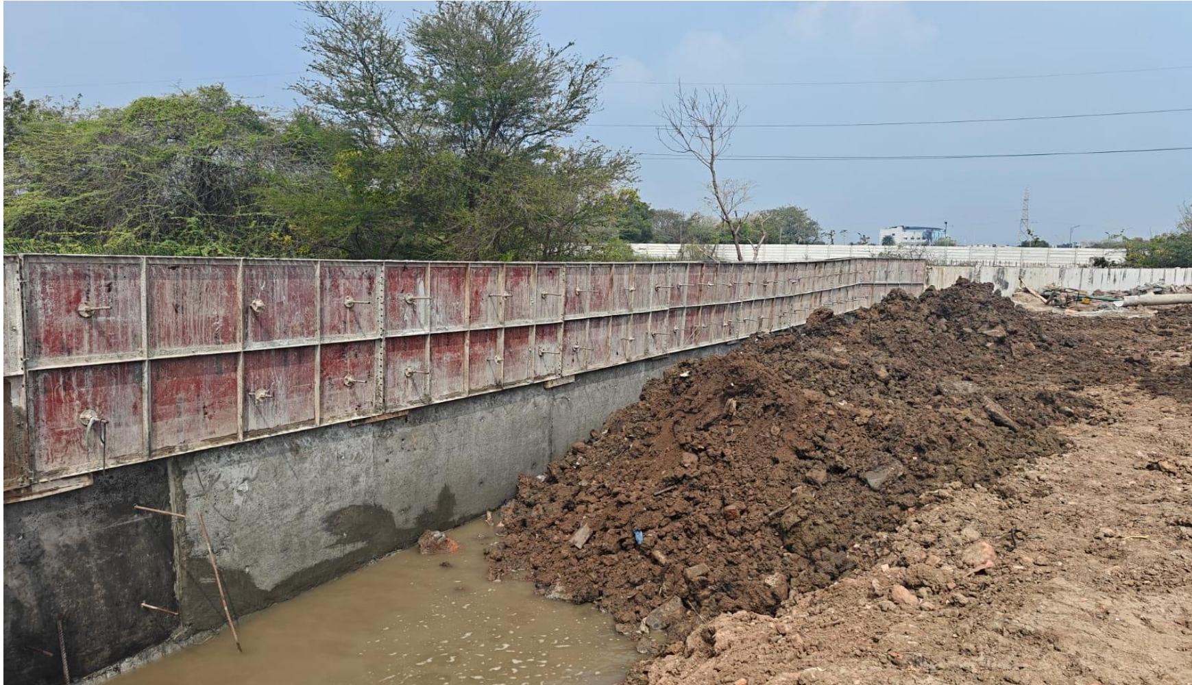
South Side 2 nd Lift Concrete WIP
