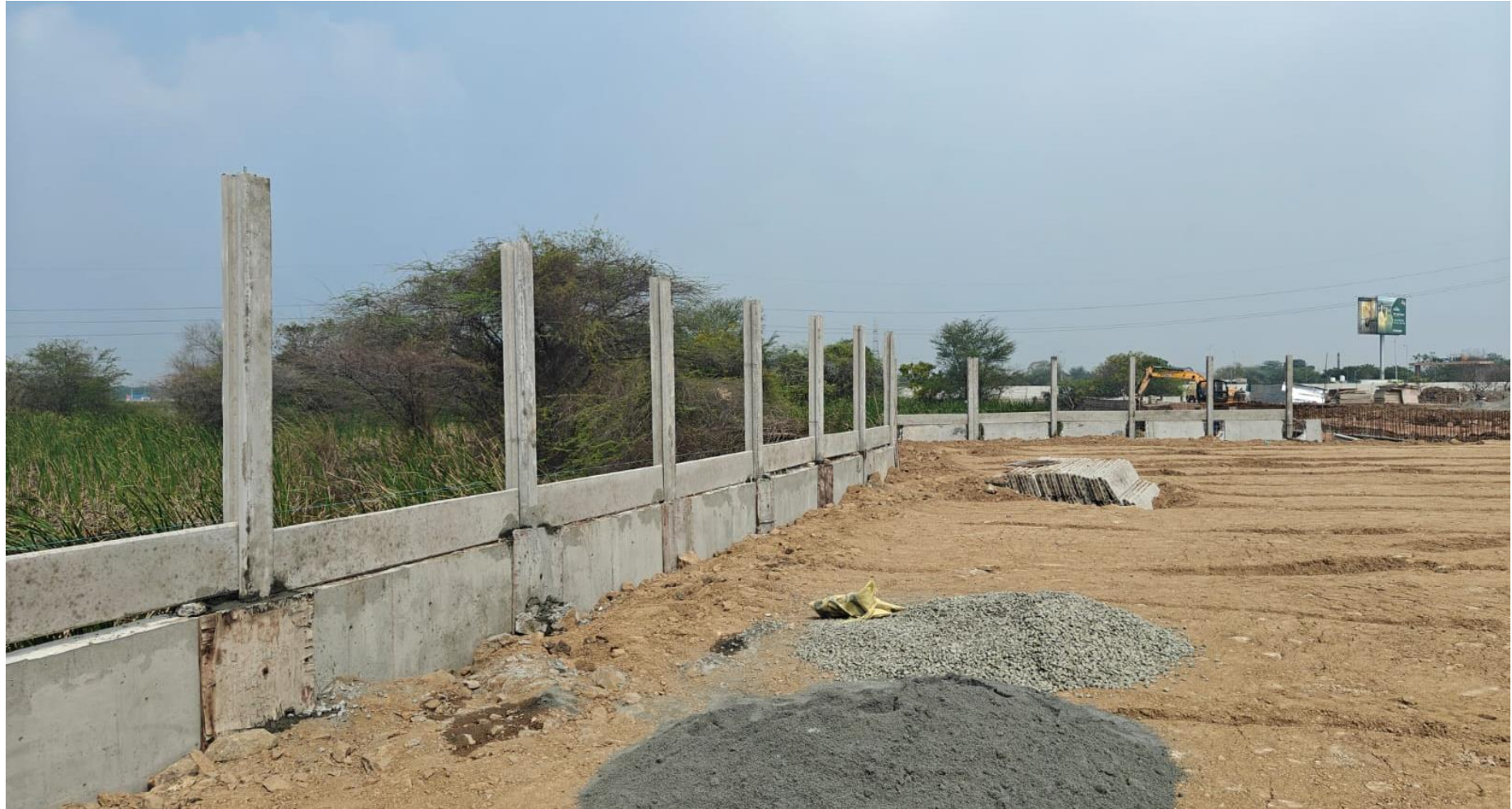
West Side Pre-cast Compound Post Fixing & Concrete WIP
