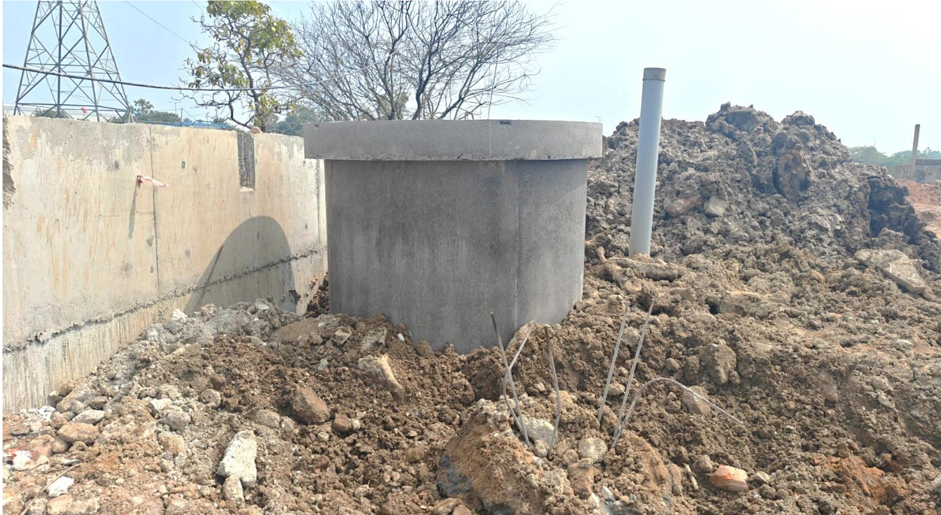
OSR Bore Pipeline and UG Sump Fixing Completed
