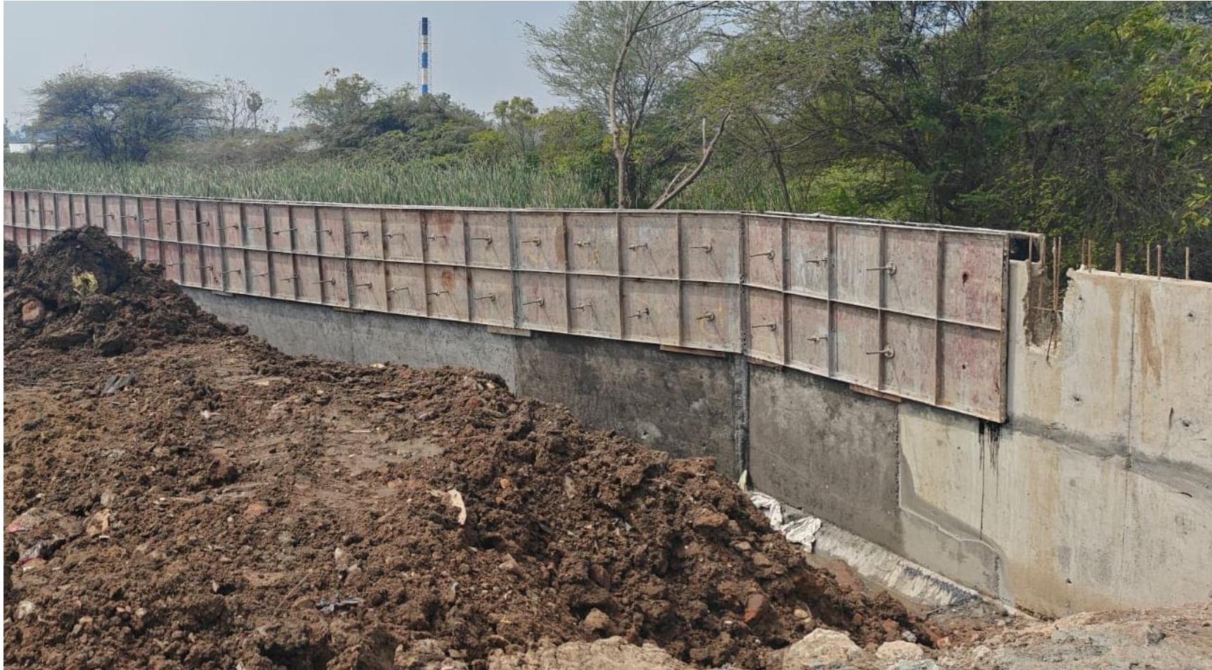
South Side 1 st Lift Concrete Works Completed
