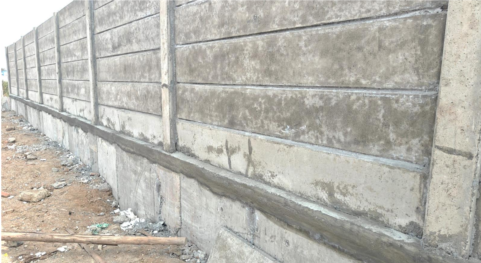
Retaining Wall Top Finishing WIP
