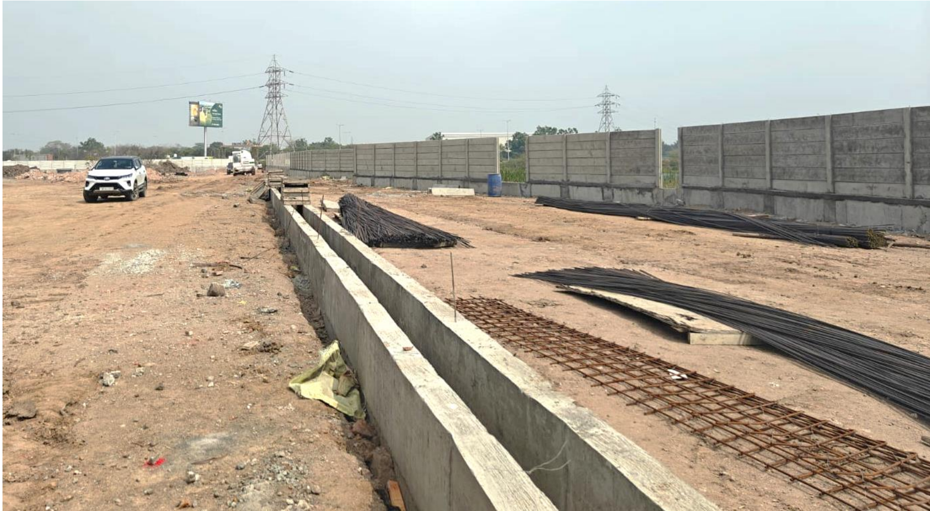
Trench Wall Concrete WIP
