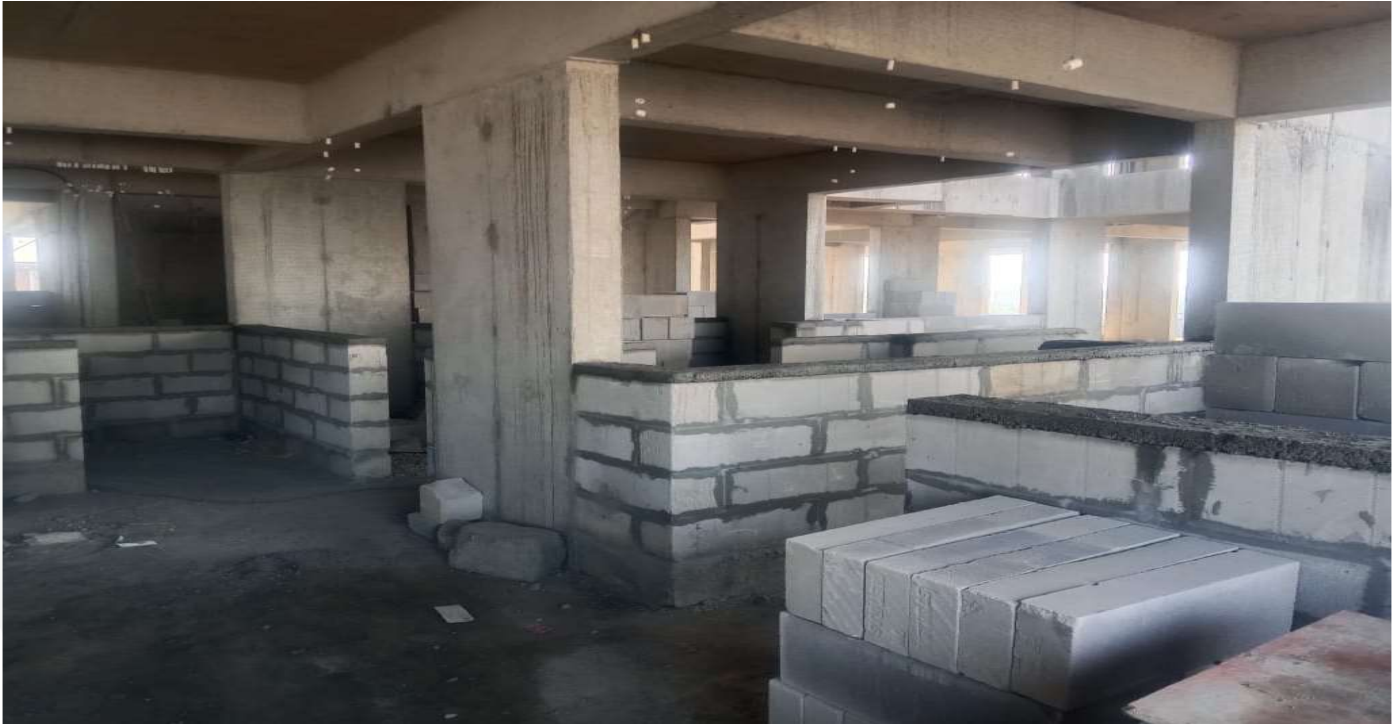
BLOCK 1 – SEVENTH FLOOR BLOCKWORK (SILL LEVEL) IN PROGRESS.
