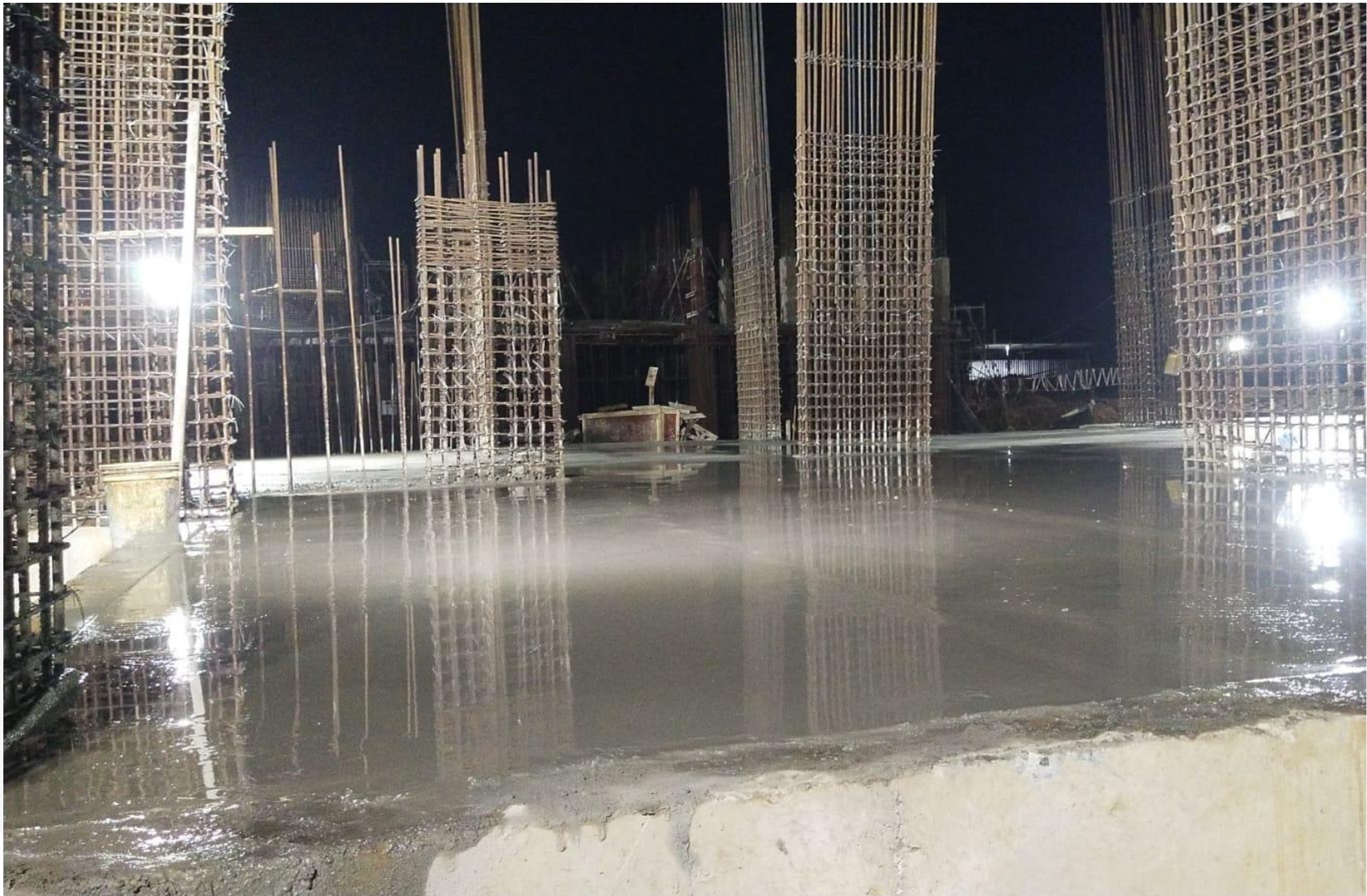
BLOCK 2 STILT FLOOR PCC WORK COMPLETED
