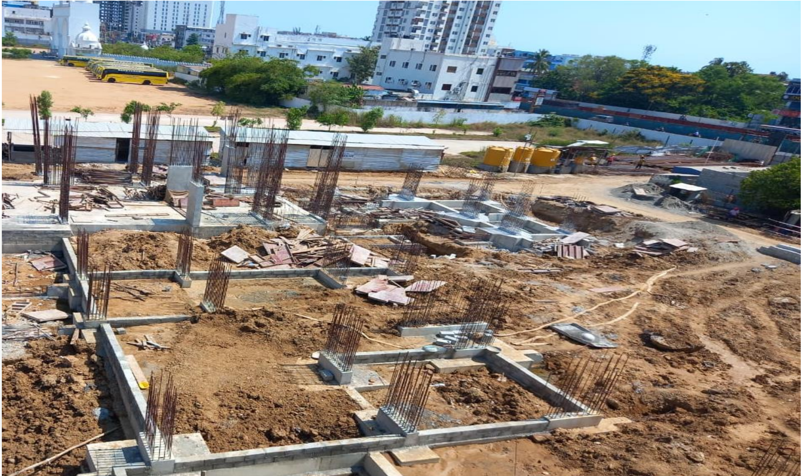
Block 2- Backfilling Work In Progress
