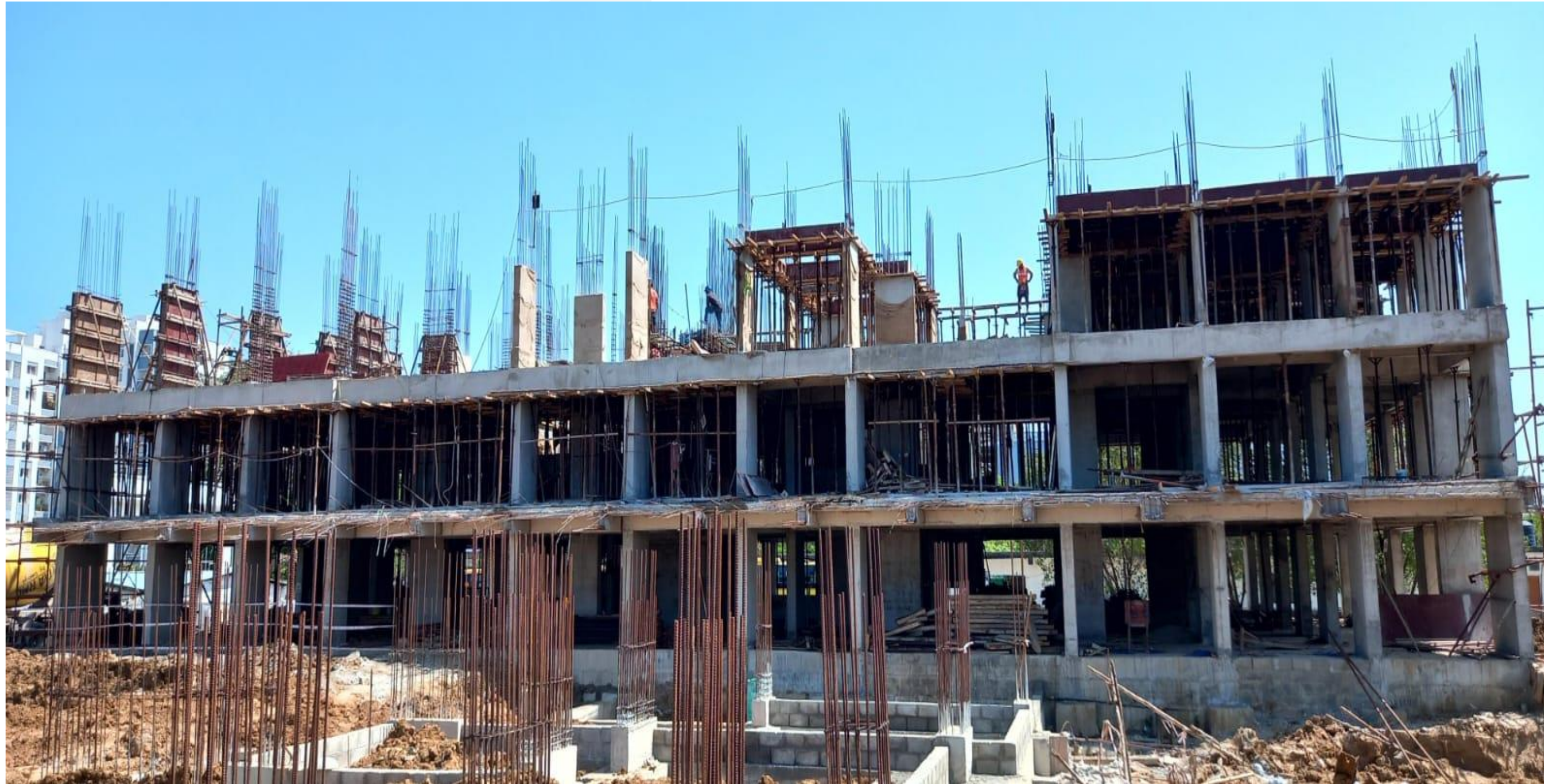
Block 1 – Second Floor Shuttering Work In Progress
