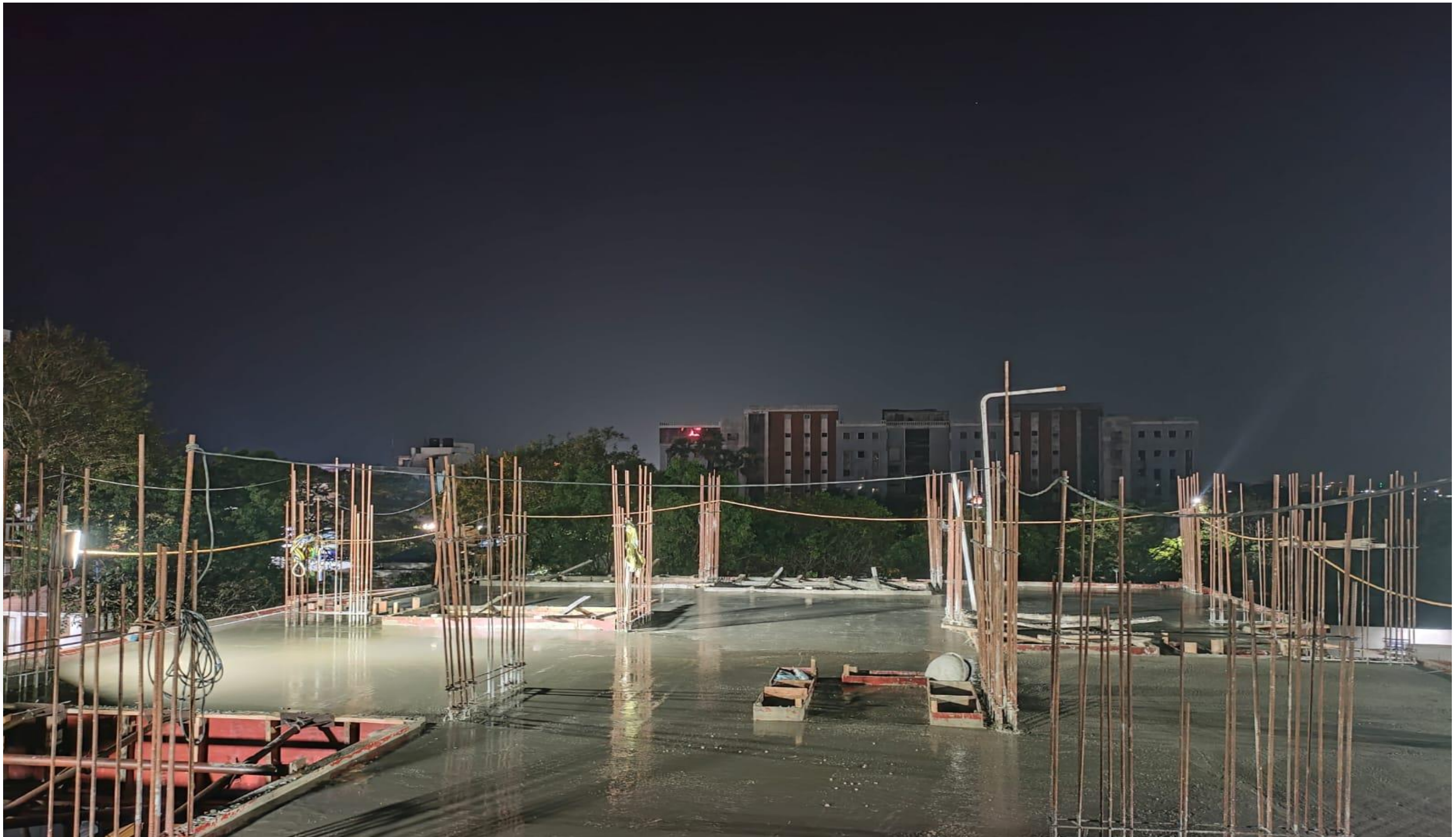
Block 1 - First Floor Roof Slab Work Completed
