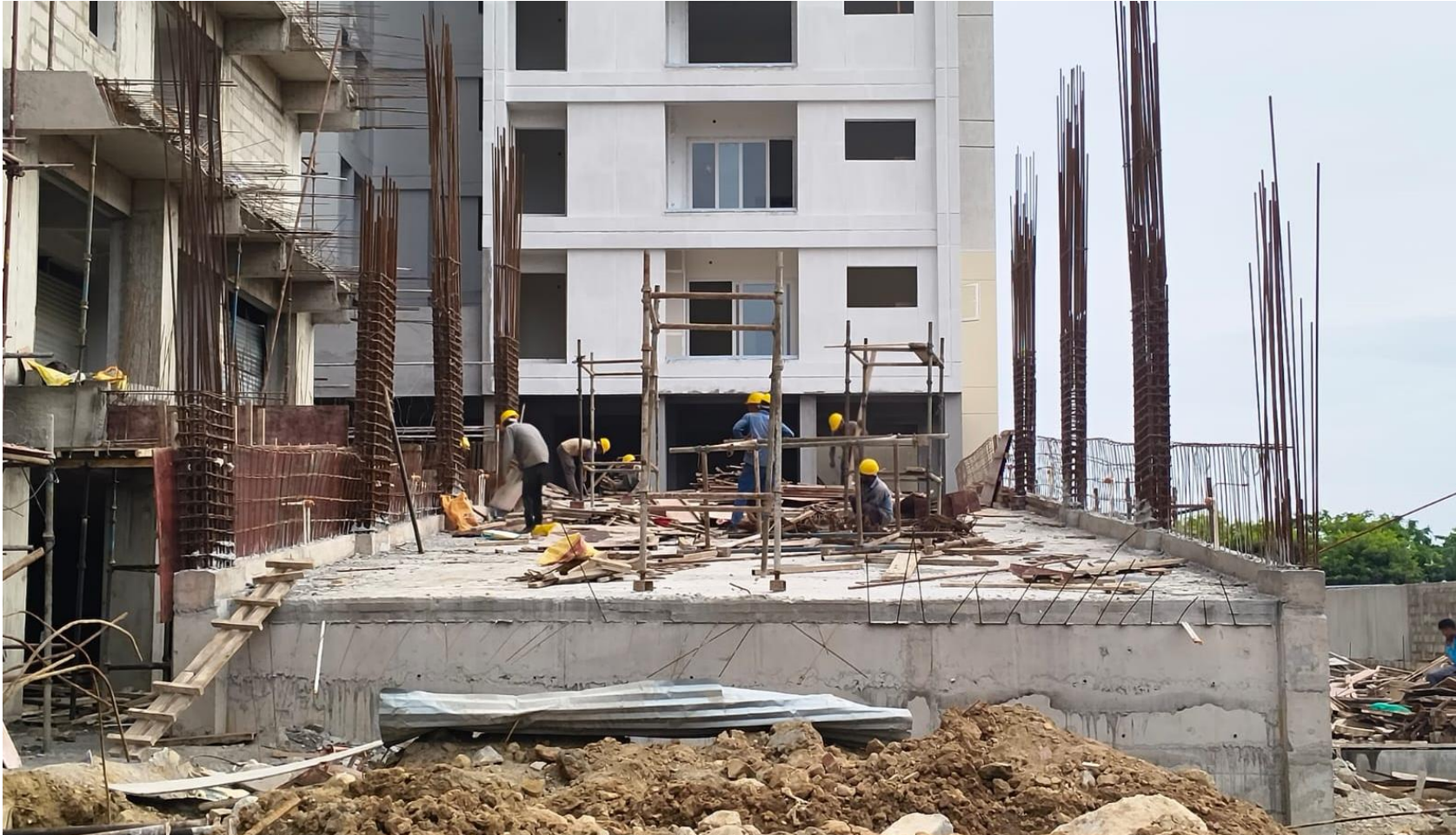
RAMP PARAPET WALL SHUTTERING & REINFORCEMENT WORK IN PROGRESS
