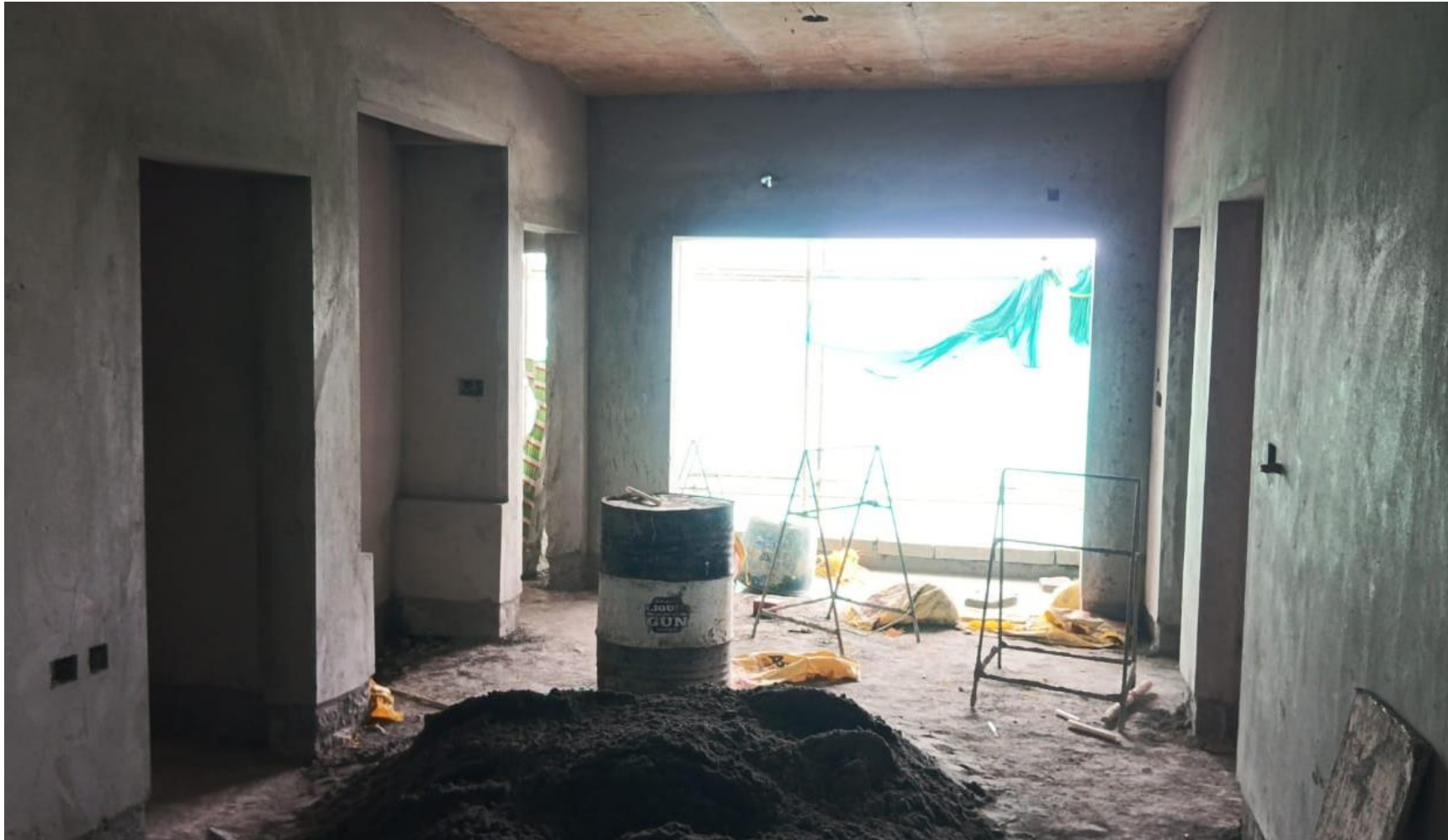
BLOCK 2 POUR 2 - TENTH FLOOR INTERNAL PLASTERING WORK IN PROGRESS
