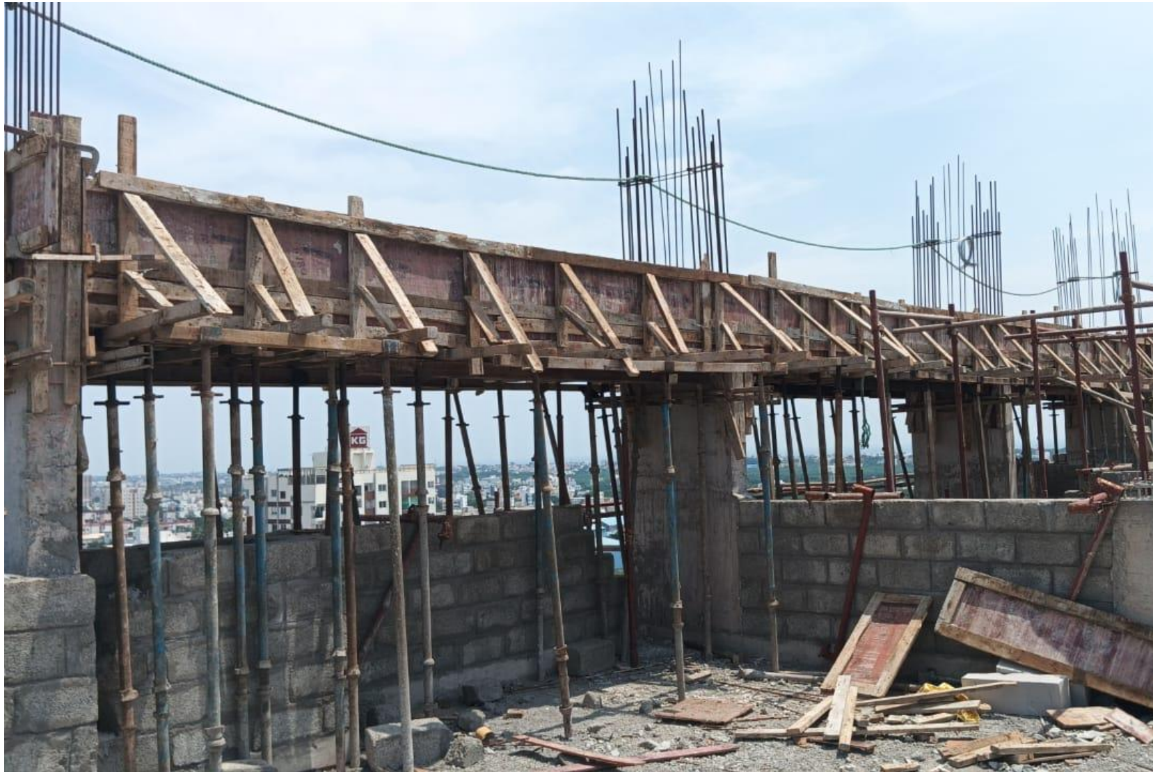
BLOCK 2 POUR 1 - TERRACE PERGOLA CONCRETE COMPLETED
