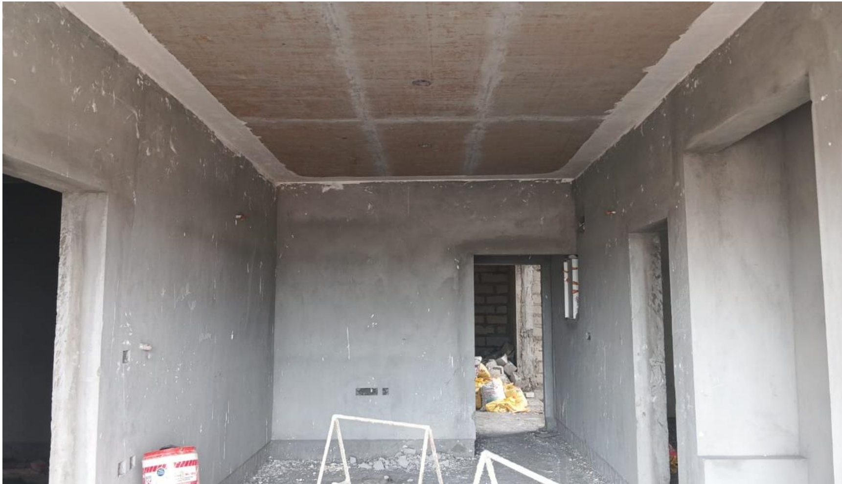
BLOCK 2 POUR 2 – EIGHTH FLOOR CORNER CORRECTION IN PROGRESS
