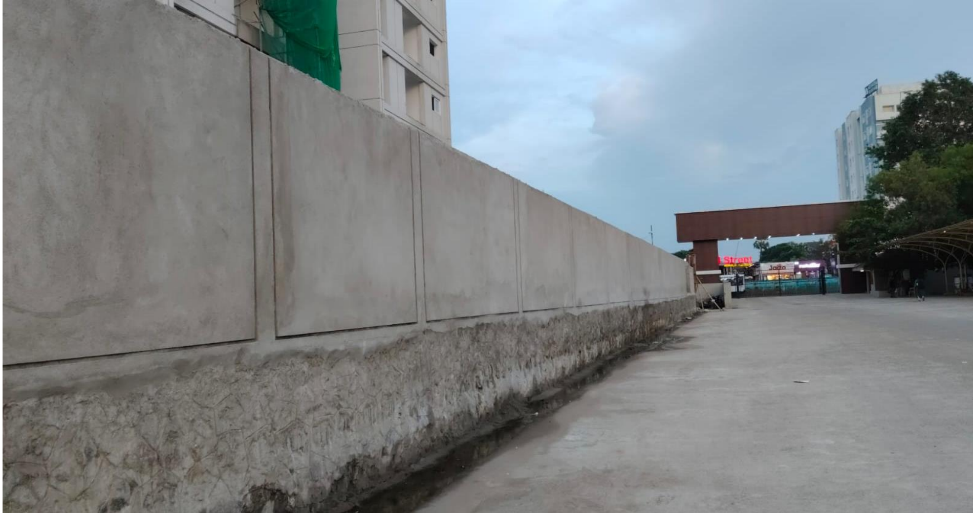
COMPOUND WALL EXTERNAL PLASTERING IN PROGRESS
