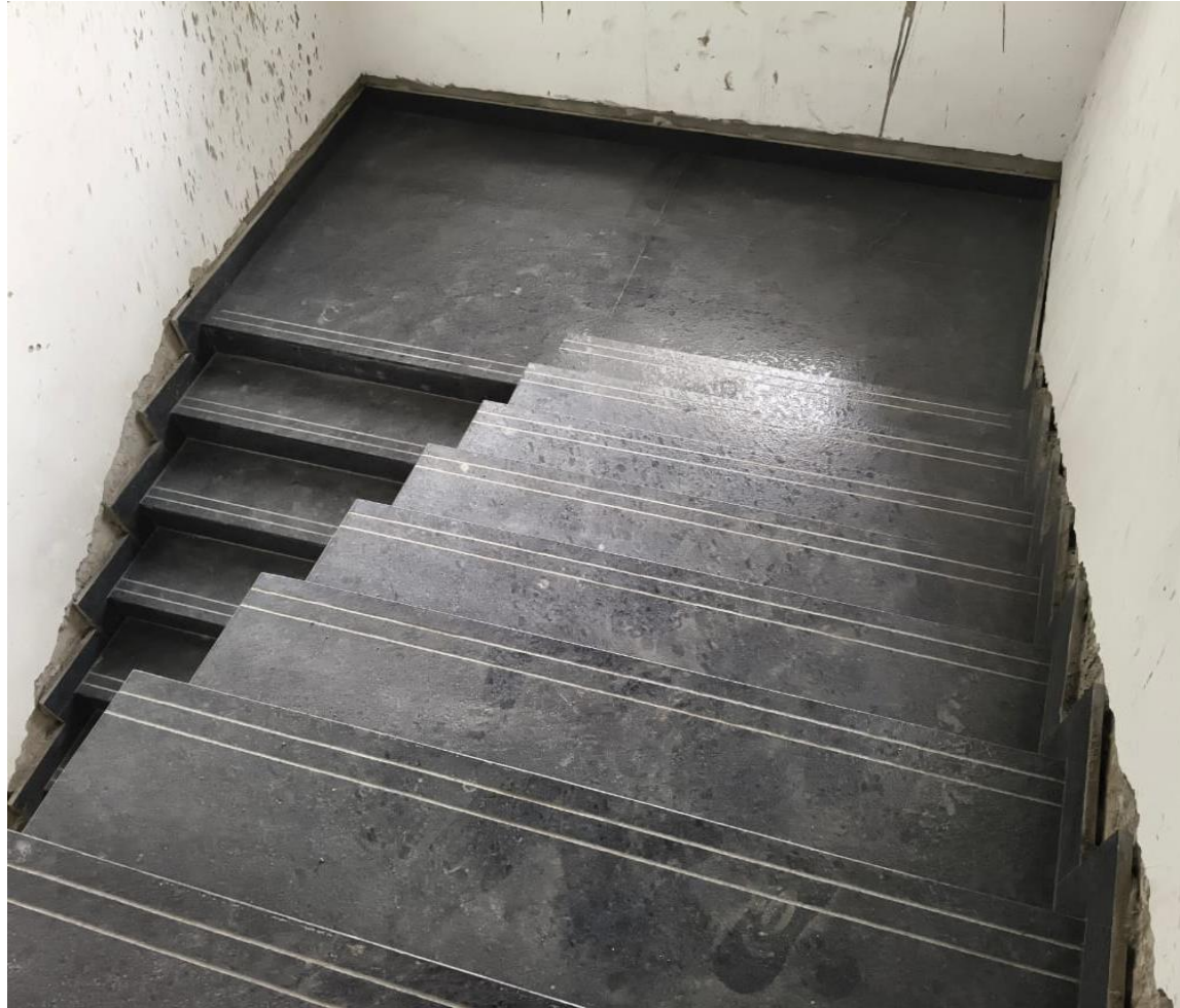
BLOCK 1 - STAIRCASE 2 GRANITE WORK IN PROGRESS
