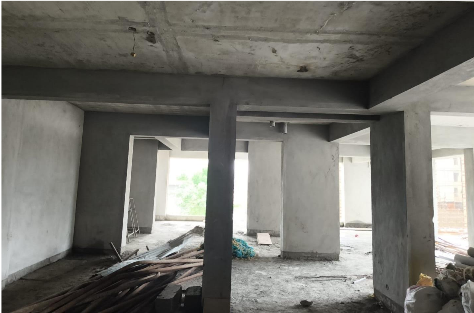
BLOCK 1 - FIRST FLOOR CAR PARKING PLASTERING WORK IN PROGRESS
