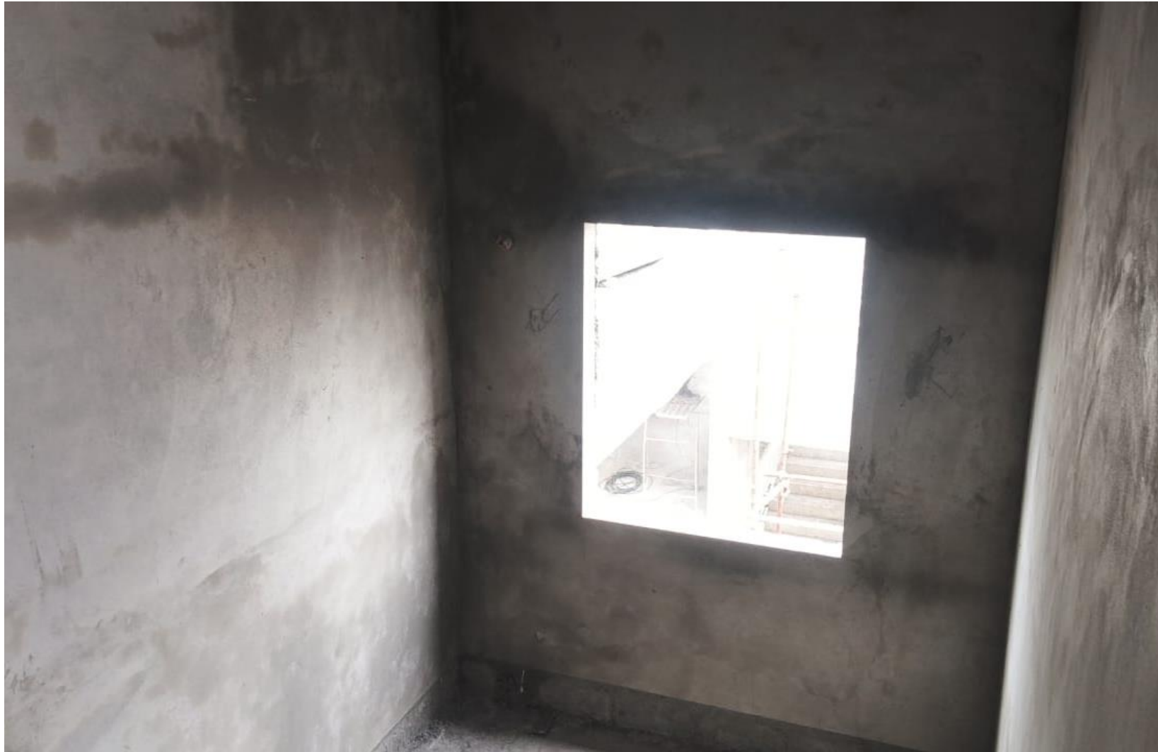
BLOCK 2 POUR 1 - HEADROOM PLASTERING WORK IN PROGRESS
