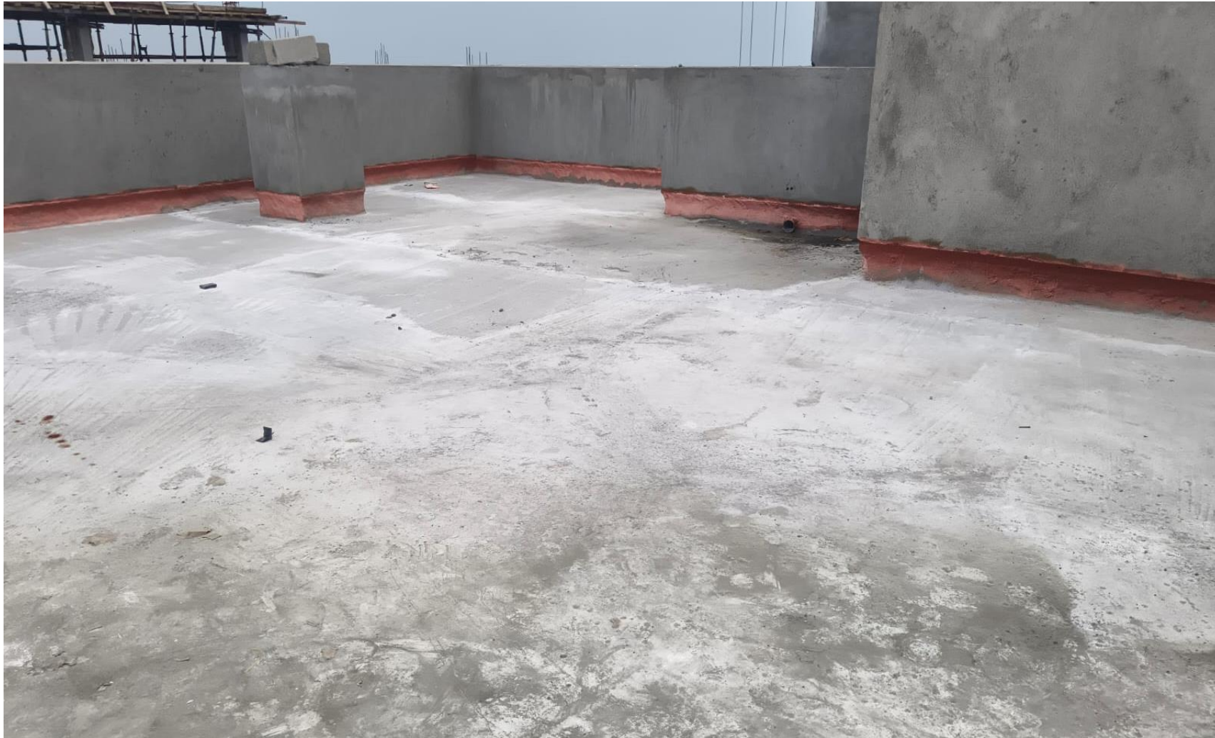
BLOCK 1 - TERRACE BAY 2 SCREED CONCRETE COMPLETED
