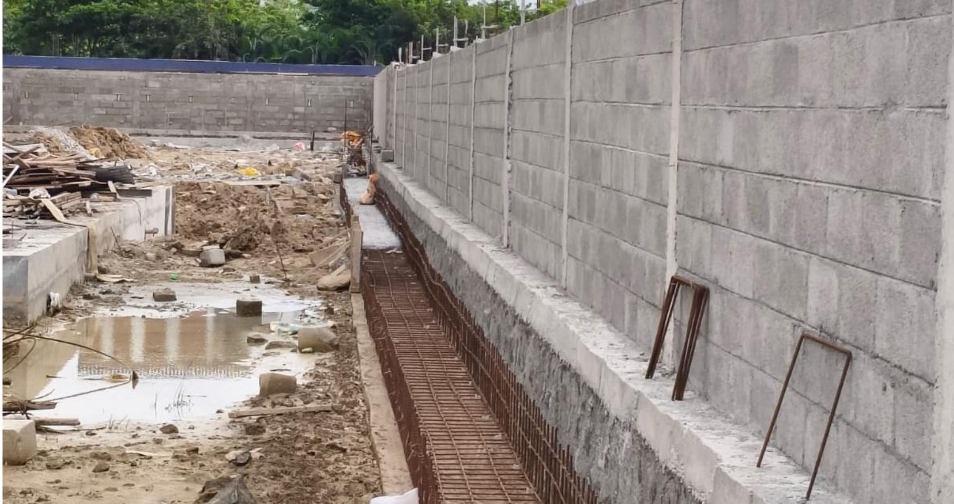
WEST SIDE TRENCH RAFT CONCRETE WORK IN PROGRESS
