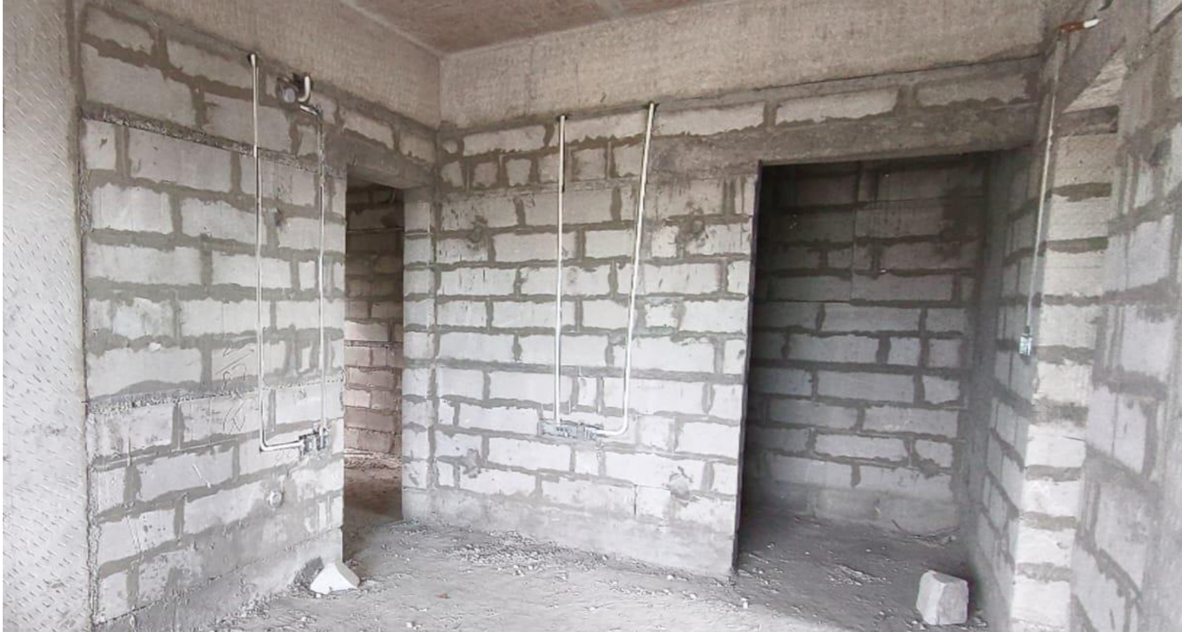
BLOCK 1 - THIRTEENTH FLOOR ELECTRICAL WALL CHASING WORK IN PROGRESS
