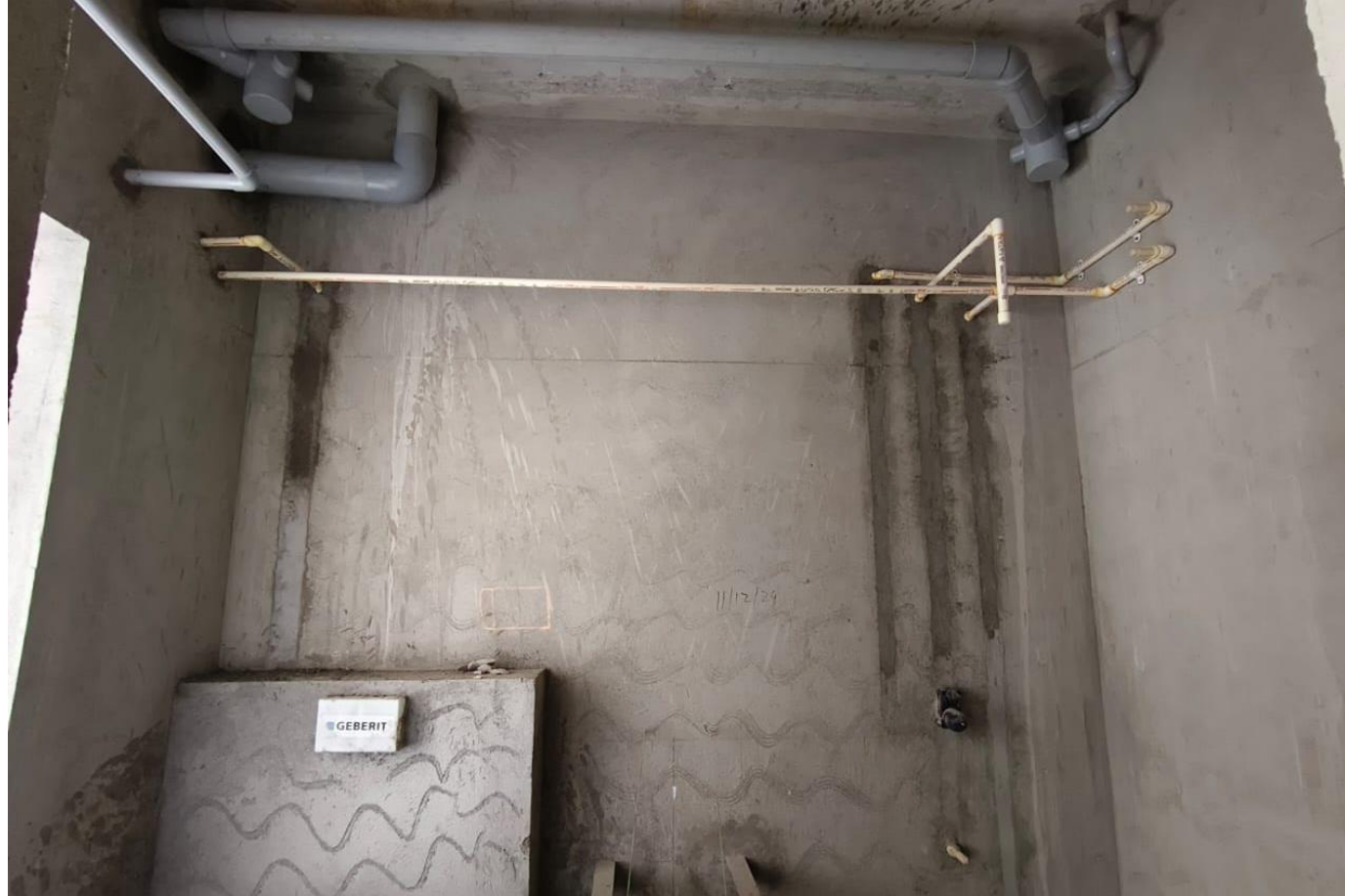
BLOCK 1 - SIXTH FLOOR PLUMBING SUSPENDED LINE WORK IN PROGRESS
