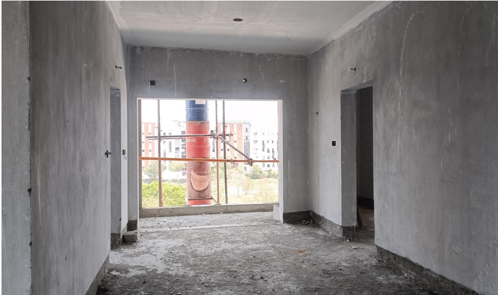
BLOCK 1 - FOURTH FLOOR CEILING & WALL PUTTY WORK IN PROGRESS
