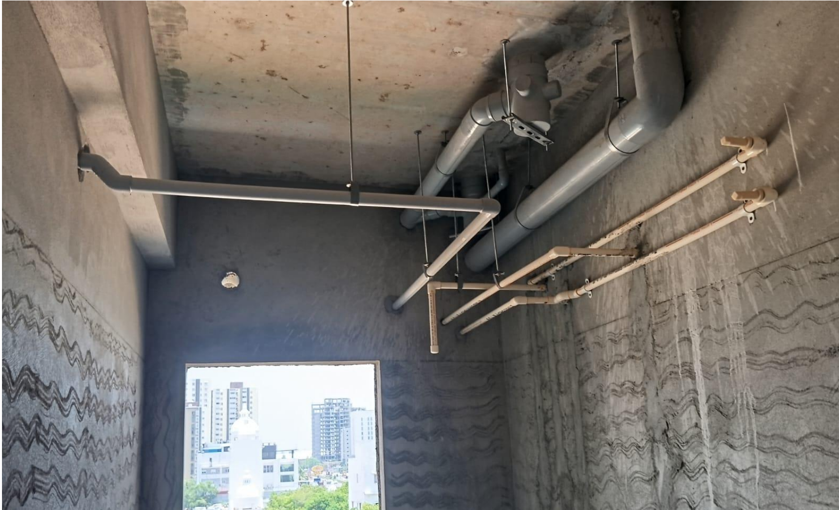
BLOCK 2 POUR 1 - FOURTH FLOOR TOILET SUSPENDED LINE WORK IN PROGRESS
