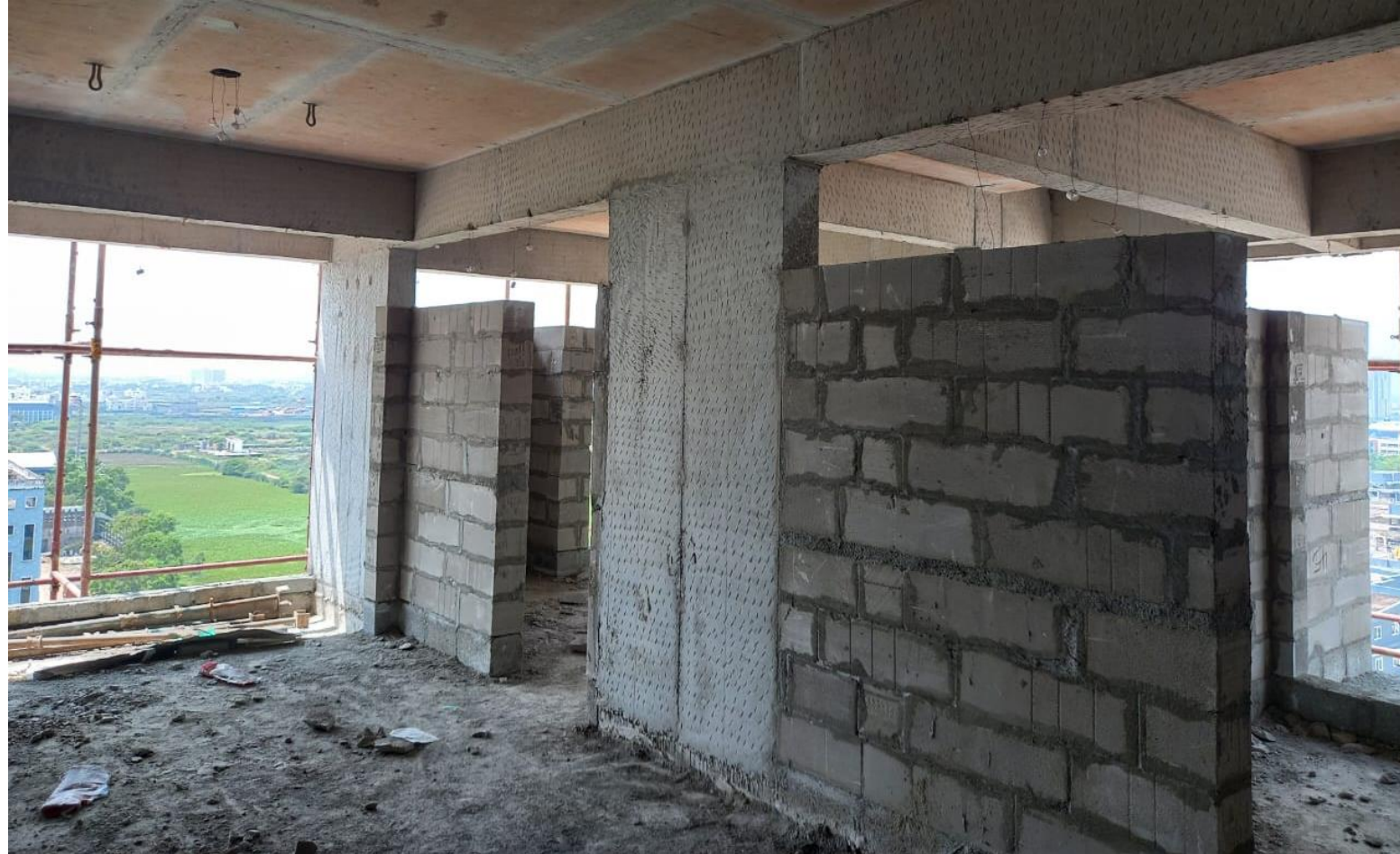
BLOCK 1 - TWELFTH FLOOR BLOCK WORK IN PROGRESS
