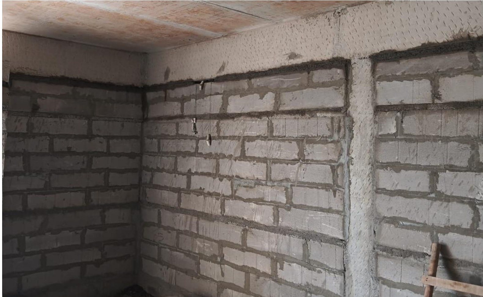
BLOCK 2 POUR 1 – SEVENTH FLOOR BLOCK WORK COMPLETED
