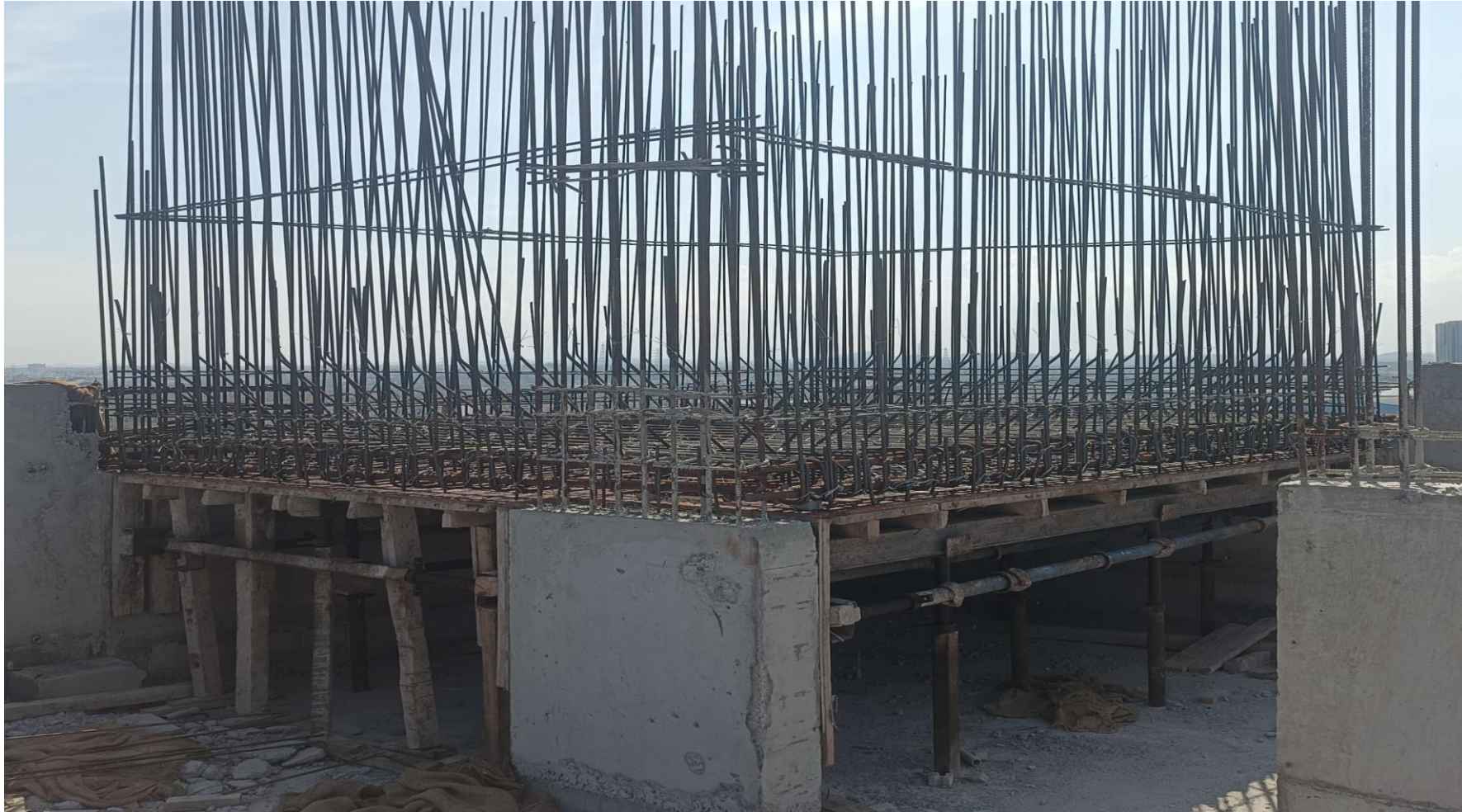
BLOCK 1 - TERRACE OHT WORK IN PROGRESS
