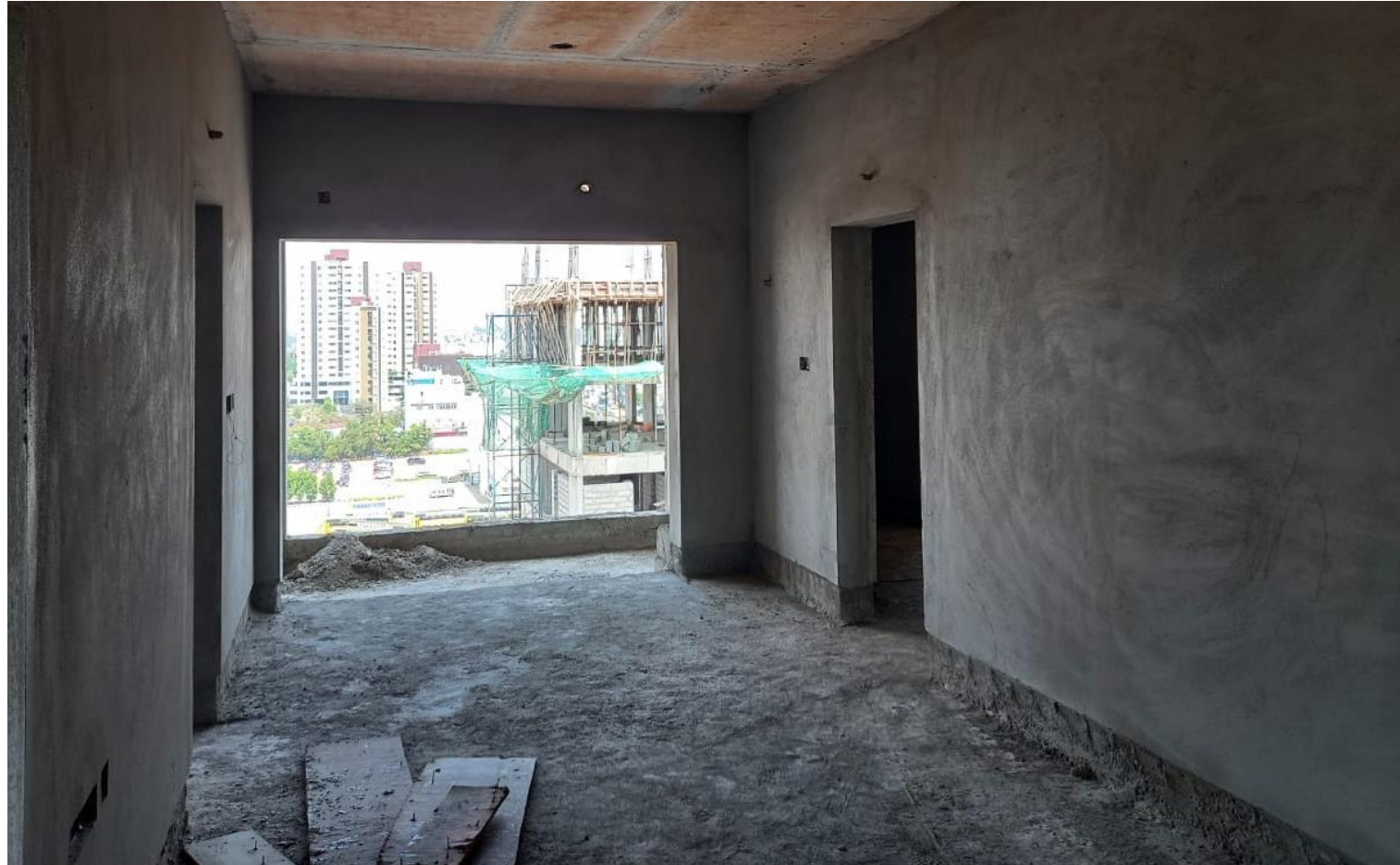
BLOCK 1 – TENTH FLOOR INTERNAL PLASTERING WORK IN PROGRESS
