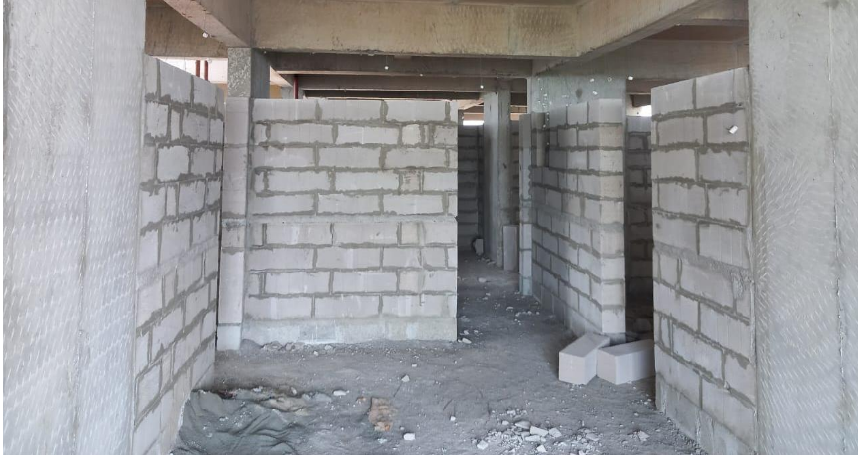
BLOCK 1 - ELEVENTH FLOOR BLOCK WORK IN PROGRESS
