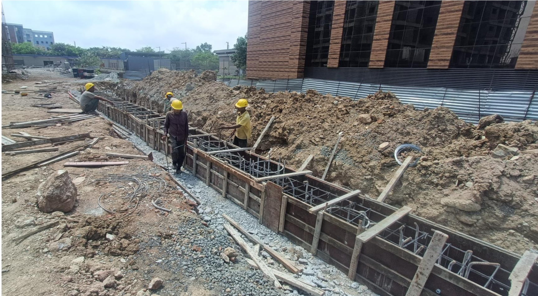
STP CONTIGUOUS PILE TIE BEAM REINFORCEMENT & SHUTTERING WORK IN PROGRESS
