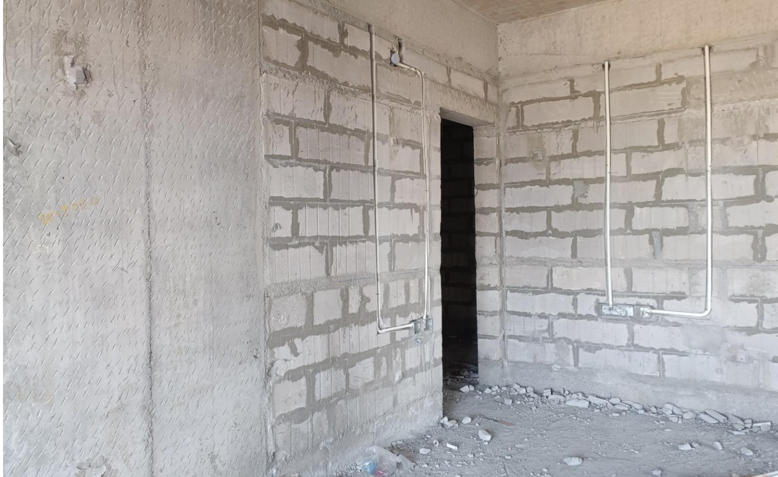
BLOCK 1 - NINTH FLOOR ELECTRICAL WALL CHASING WORK IN PROGRESS
