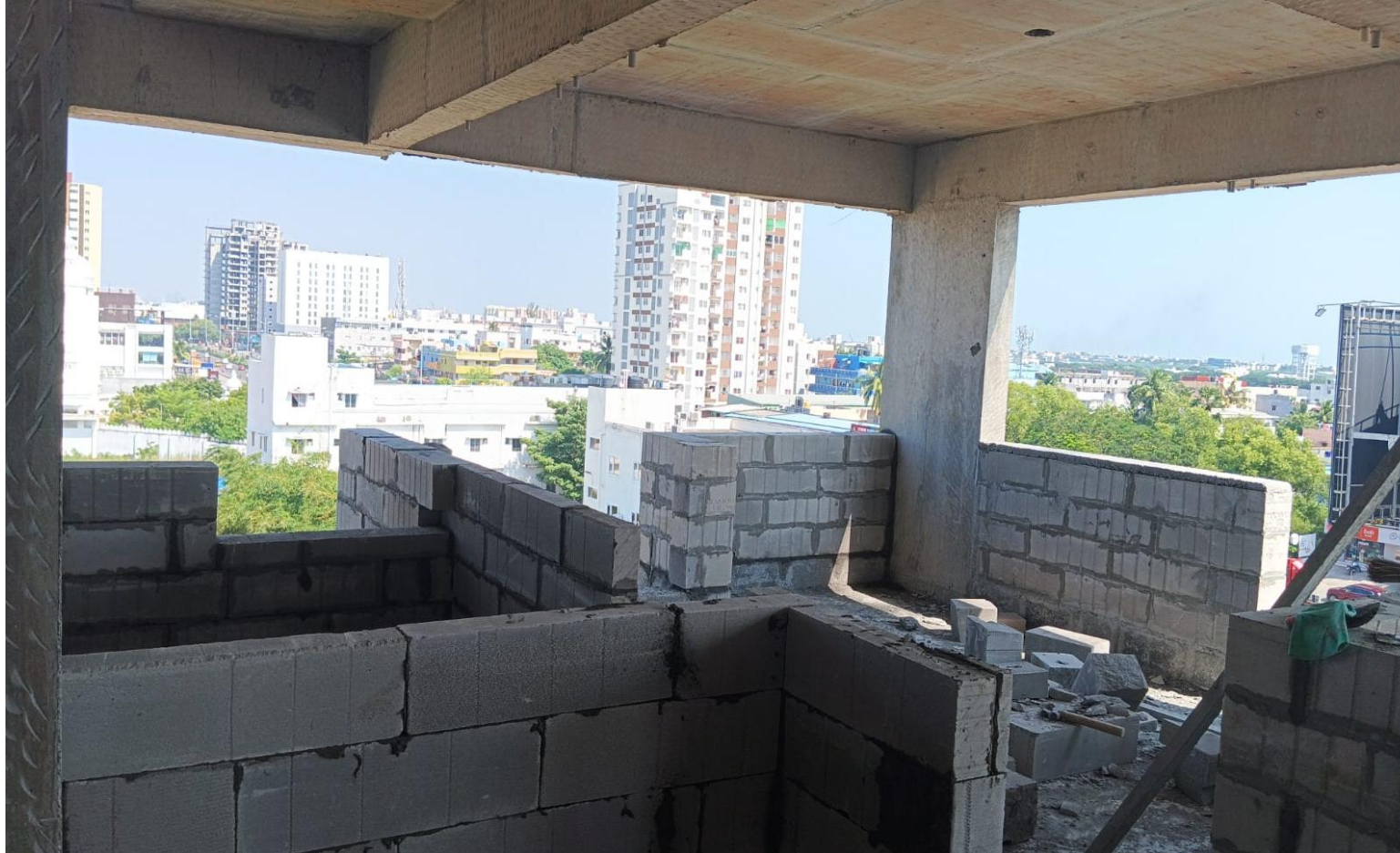
BLOCK 2 POUR 1 - SEVENTH FLOOR BLOCK WORK IN PROGRESS
