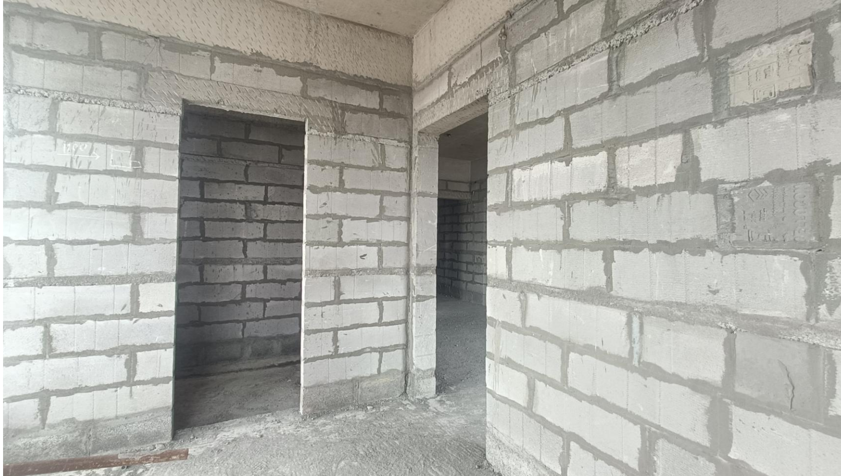
BLOCK 1 - TENTH FLOOR BLOCK WORK IN PROGRESS
