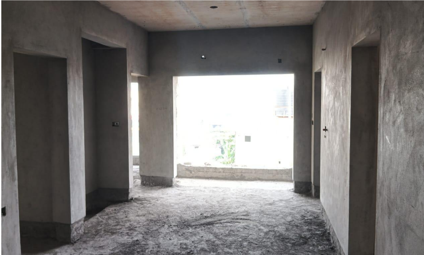
BLOCK 1 - EIGHTH FLOOR INTERNAL PLASTERING WORK COMPLETED
