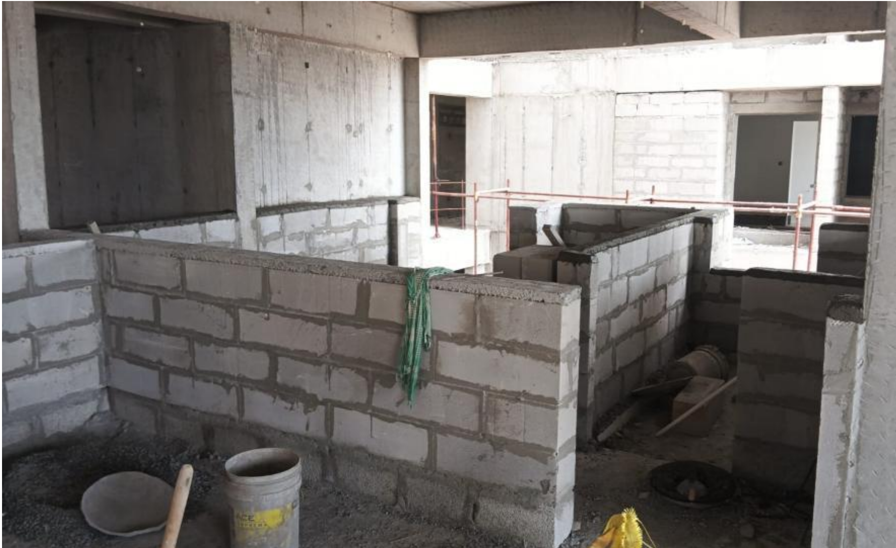
BLOCK 2 POUR 2 – SECOND FLOOR BLOCK WORK IN PROGRESS
