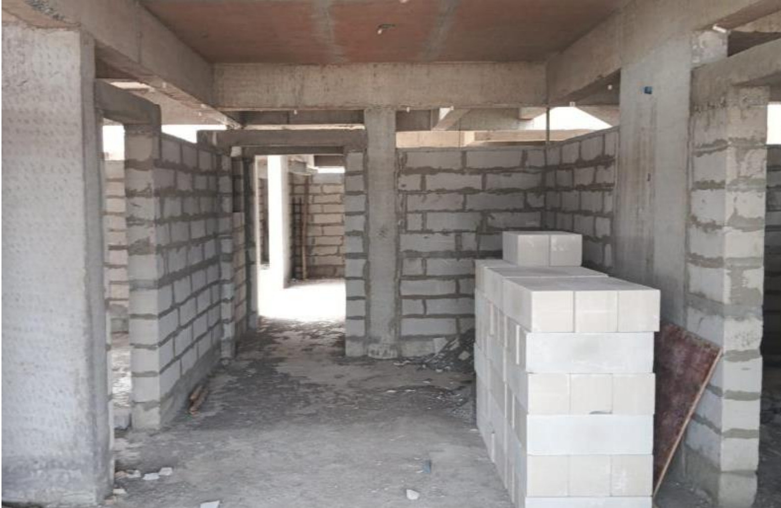
BLOCK 2 POUR 1 – THIRTEENTH BLOCK WORK IN PROGRESS
