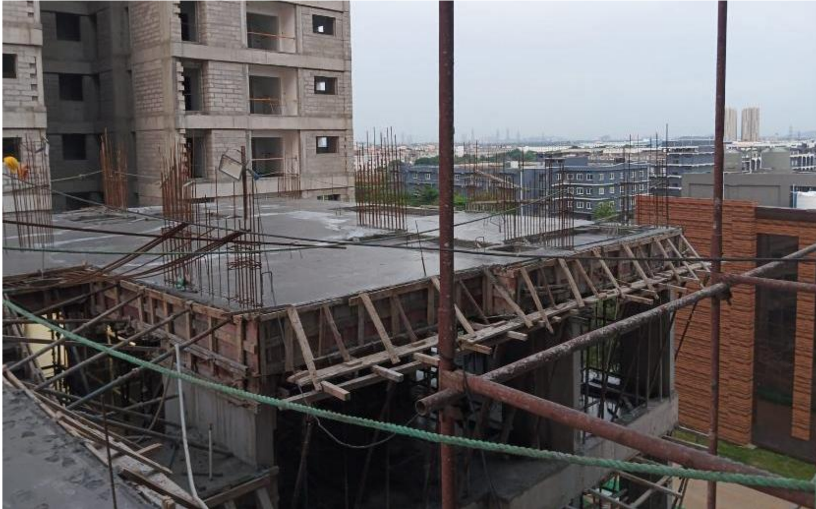
BLOCK 2 POUR 2 – FIFTH FLOOR ROOF SLAB CONCRETE COMPLETED
