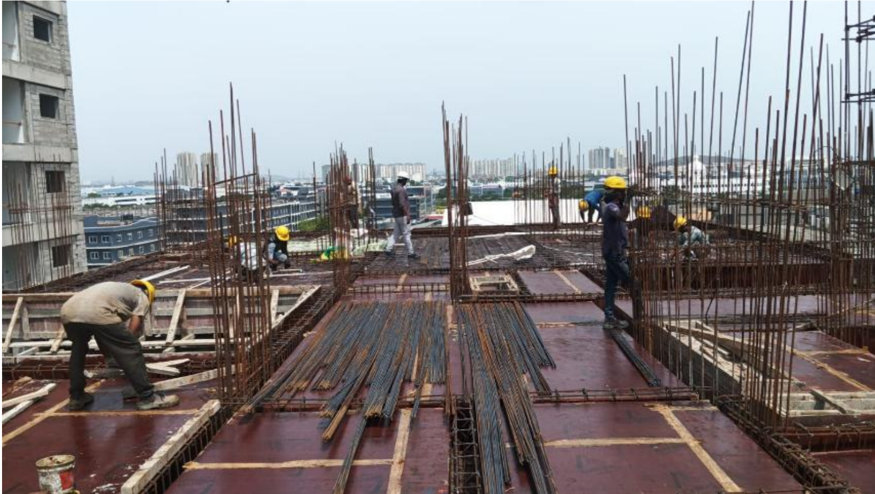
BLOCK 2 POUR 2 – SIXTH FLOOR ROOF SLAB REINFORCEMENT WORK IN PROGRESS
