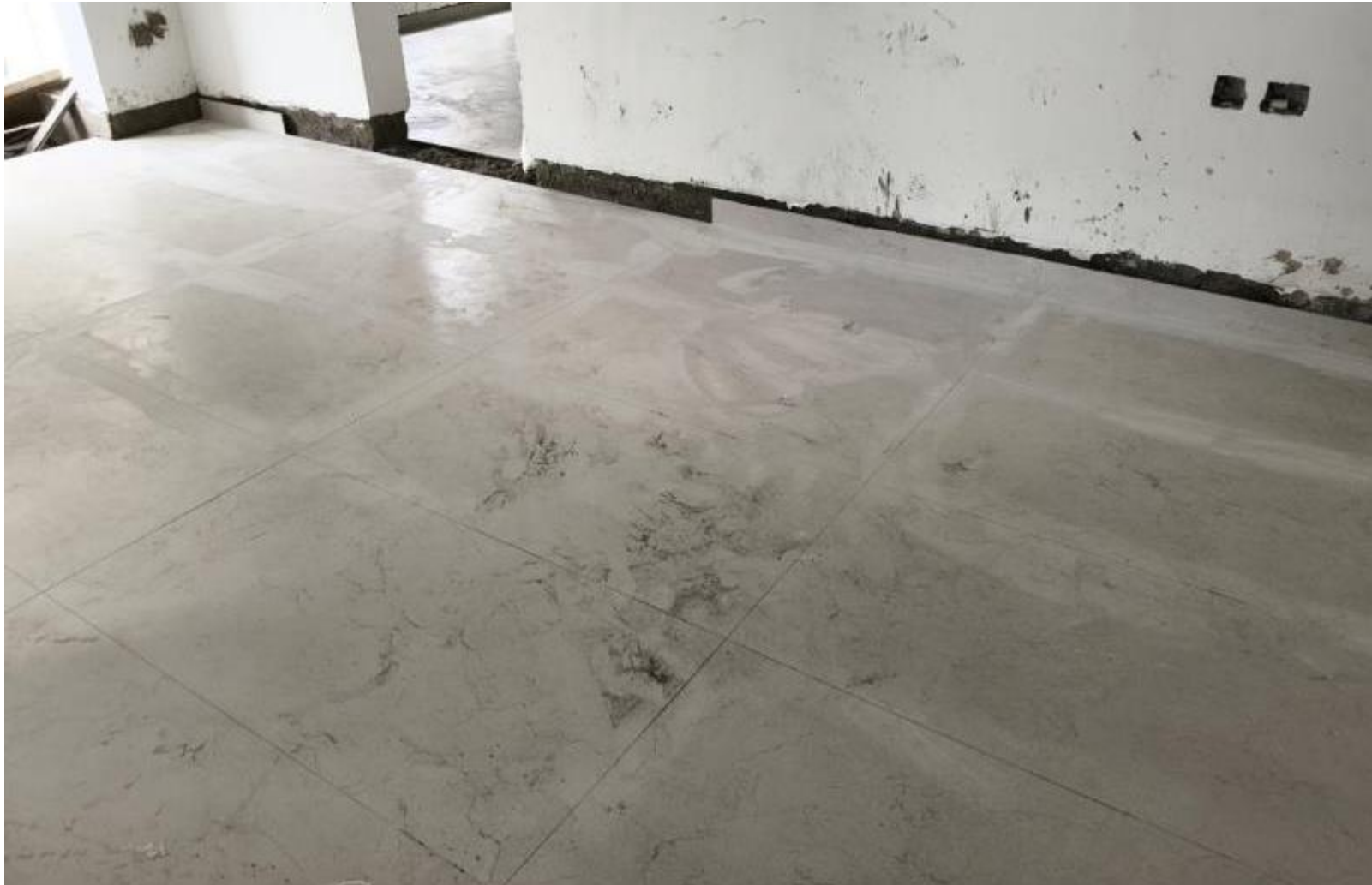
BLOCK 1 – SIXTH FLOOR TILES LAYING WORK IN PROGRESS
