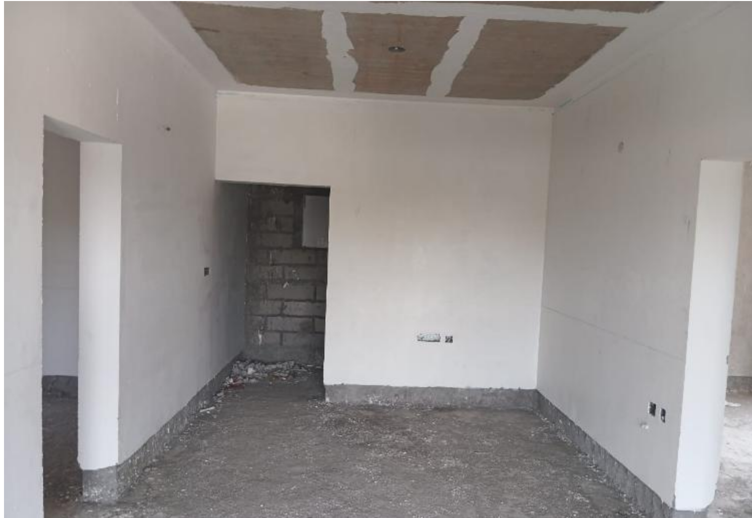
BLOCK 2 POUR 1 – SIXTH FLOOR WALL & CEILING PUTTY WORK IN PROGRESS
