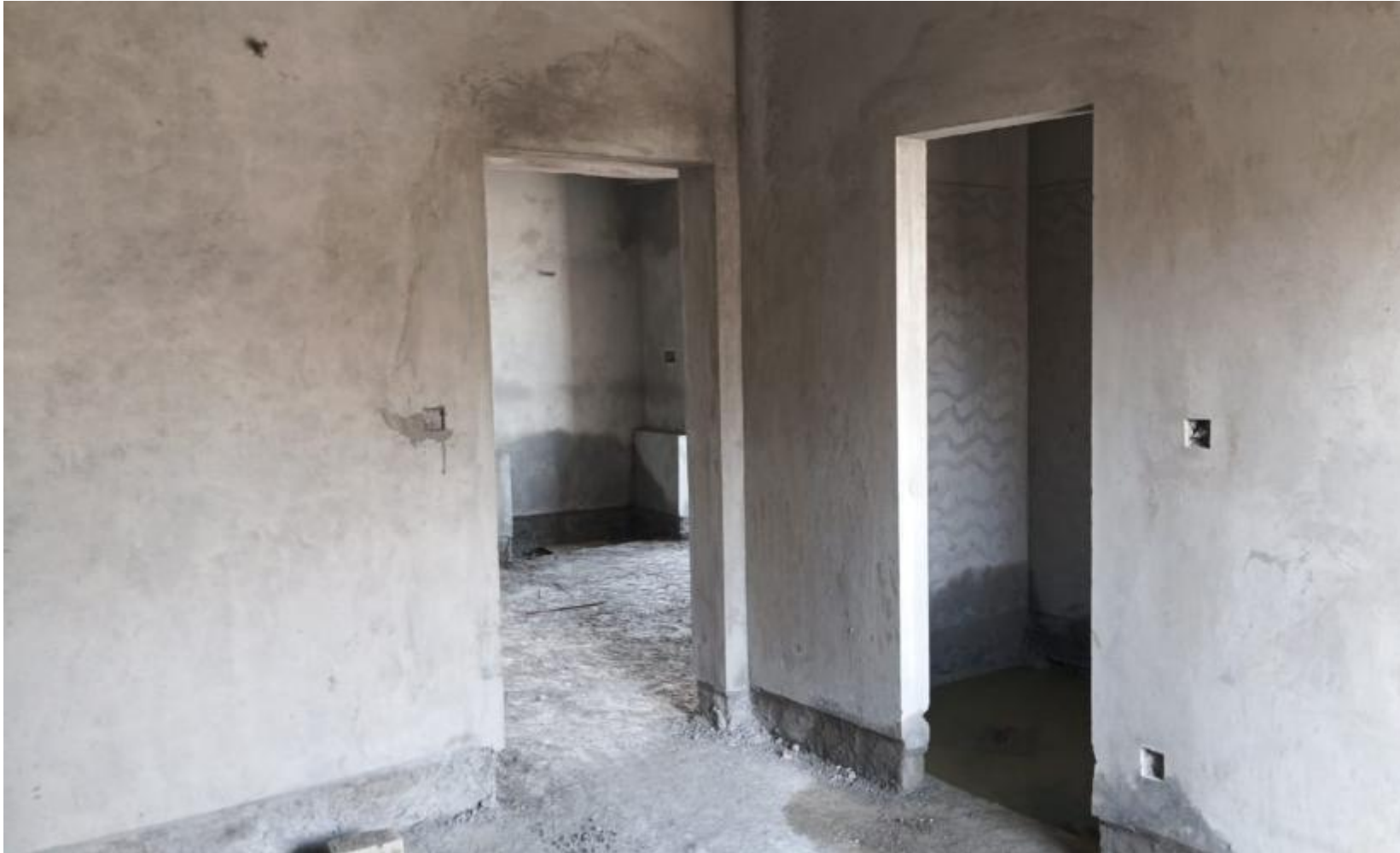
BLOCK 2 POUR 1 – TWELFTH FLOOR INNER PLASTERING COMPLETED
