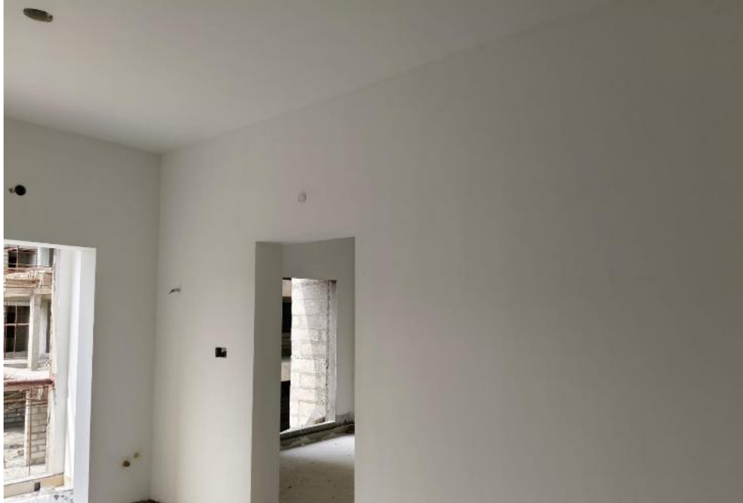
BLOCK 1 - SECOND FLOOR SECOND COAT PUTTY COMPLETED
