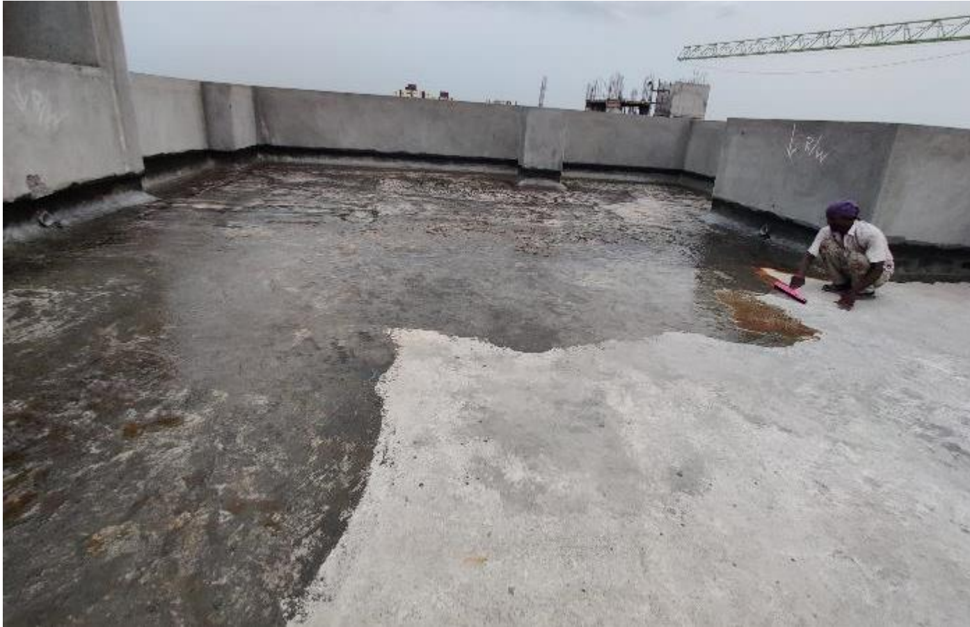
BLOCK 1 – TERRACE FLOOR WATERPROOFING WORK IN PROGRESS
