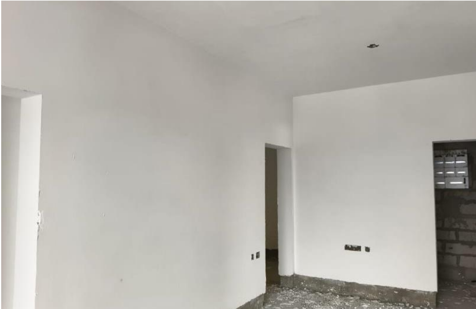
BLOCK 1 – ELEVENTH FLOOR CEILING & WALL FIRST COAT PUTTY WORK IN PROGRESS
