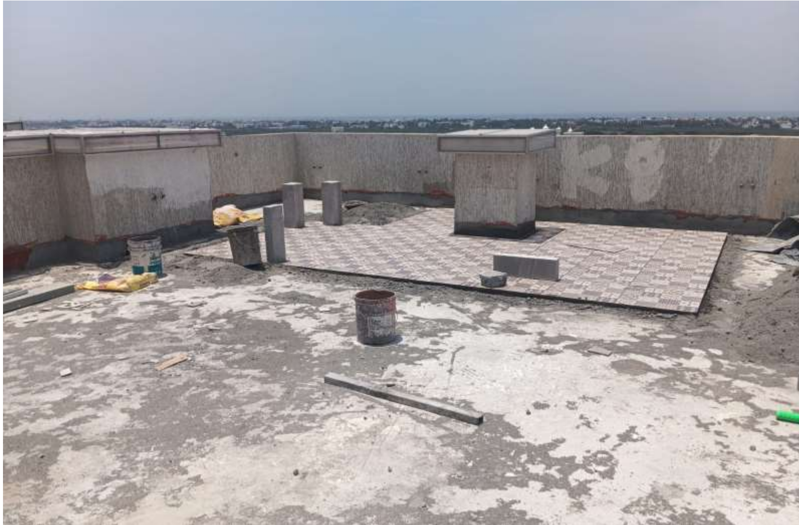
BLOCK 2 POUR 2 – TERRACE TILE LAYING WORK IN PROGRESS
