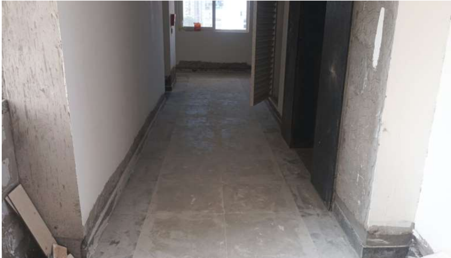
BLOCK 2 POUR 1 – CORRIDOR POP REMOVING COMPLETED
