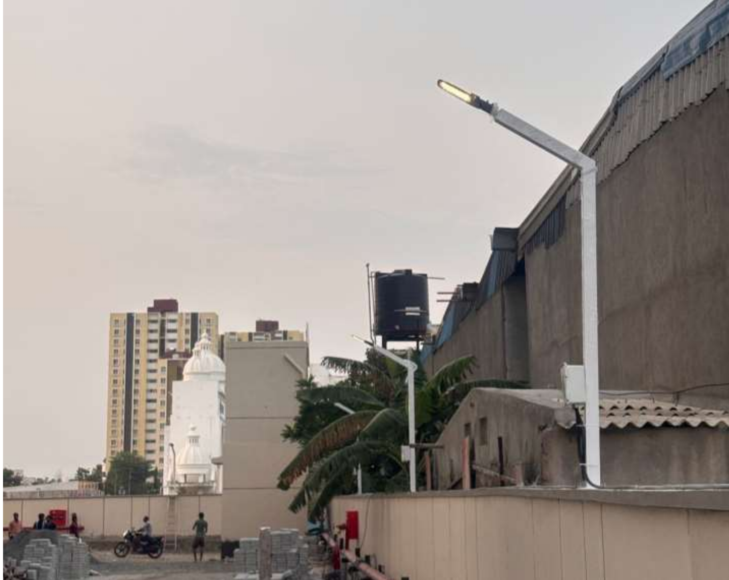
STREET LIGHT FIXING WORK IN PROGRESS
