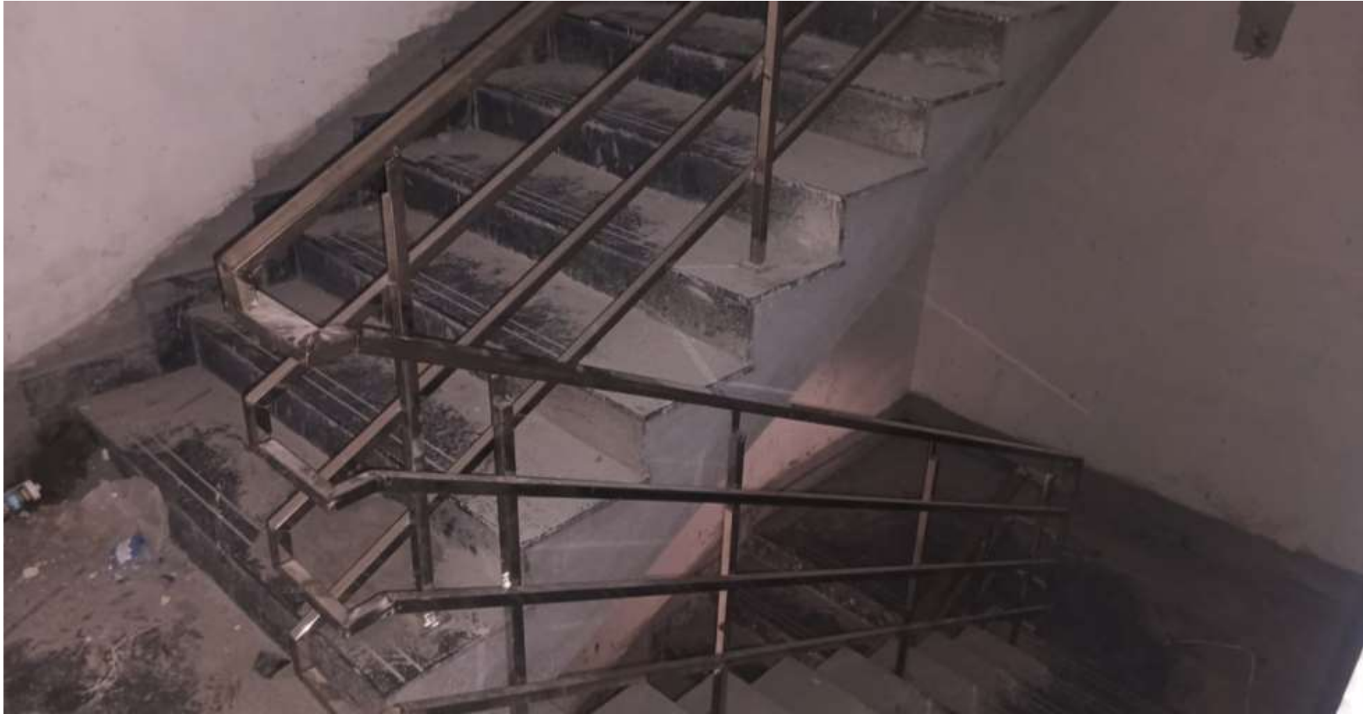
BLOCK 2 POUR 2 – SS HANDRAIL FINISHING WORK IN PROGRESS
