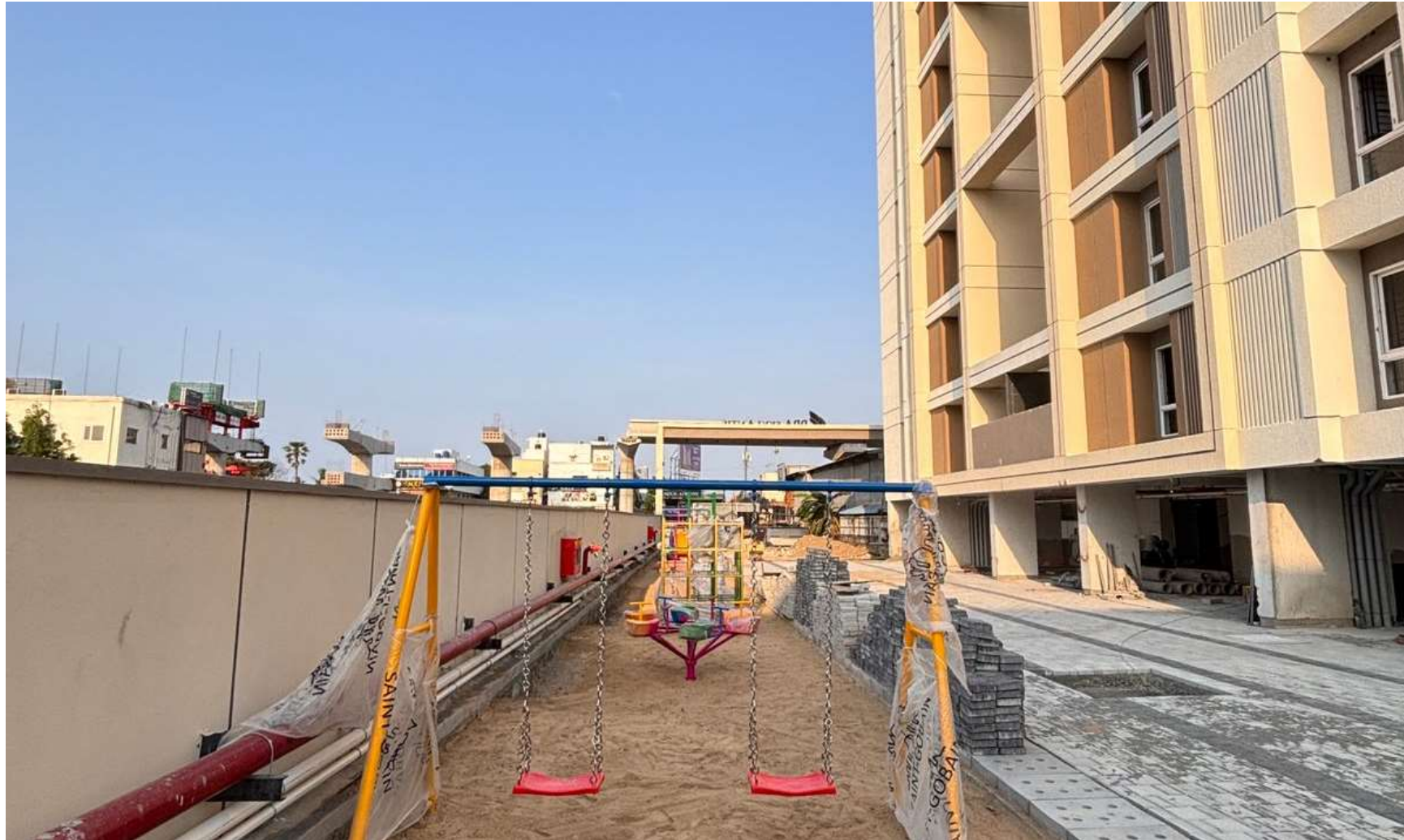
KIDS PLAY AREA SAND SEA FILLING IN PROGRESS
