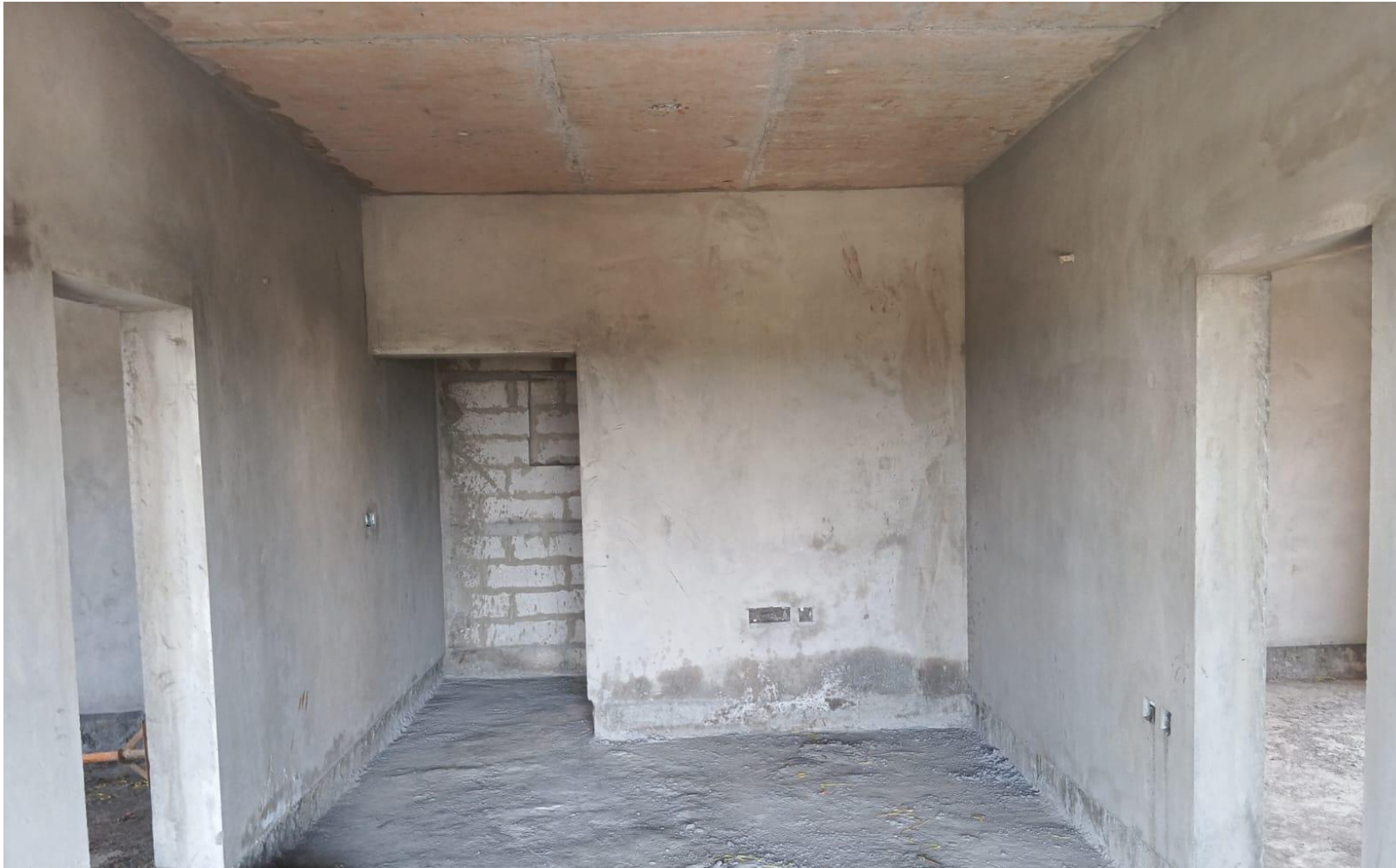
BLOCK 2 POUR 1 – ELEVENTH FLOOR INNER PLASTERING WORK IN PROGRESS
