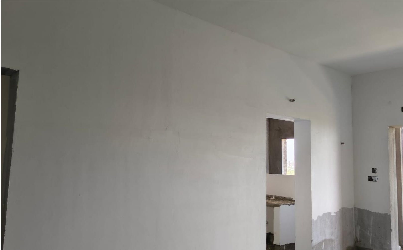
BLOCK 1 - NINTH FLOOR CEILING & WALL PUTTY WORK IN PROGRESS
