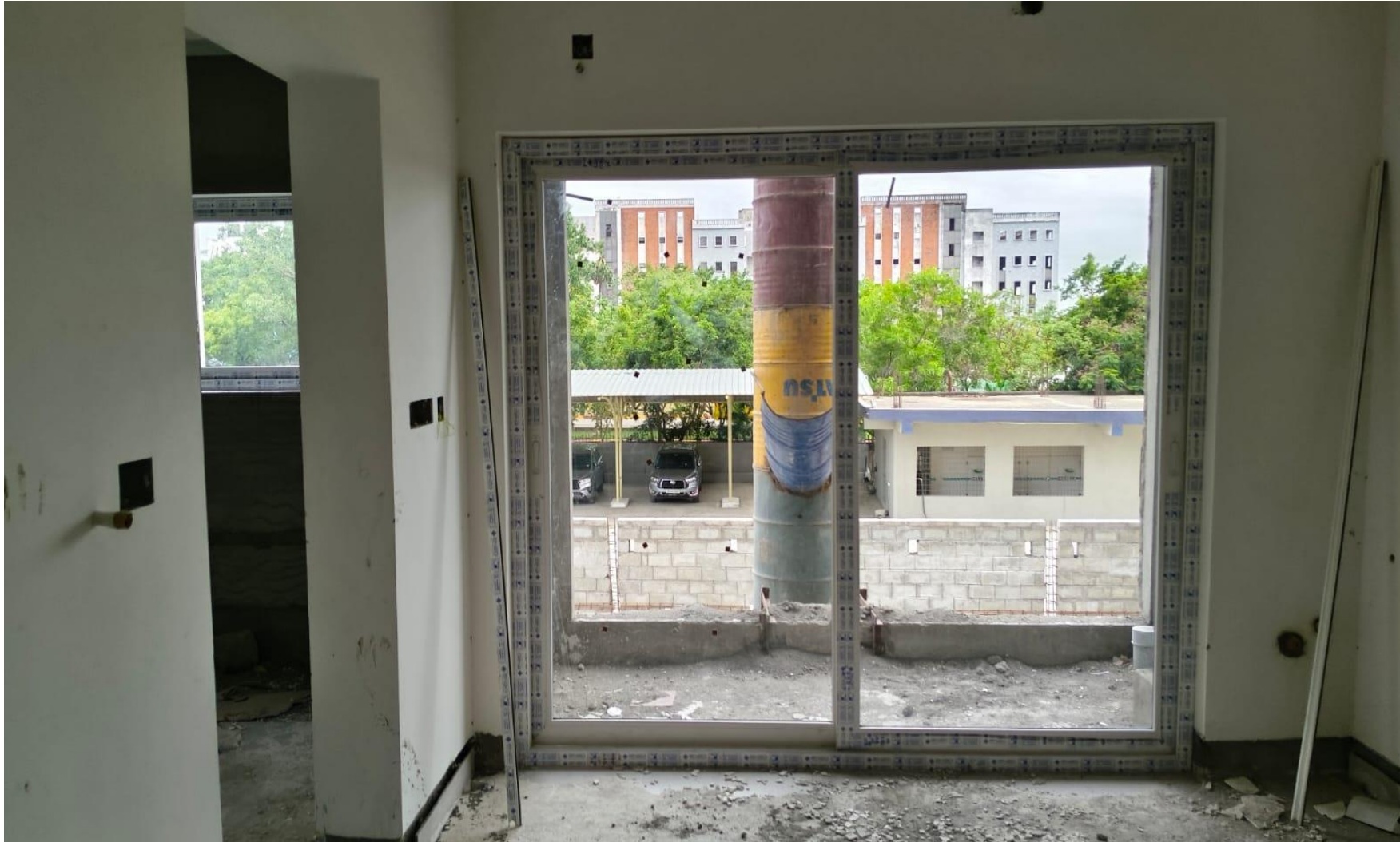
BLOCK 1 – FIRST FLOOR UPVC JOINERIES MOCK UP COMPLETED
