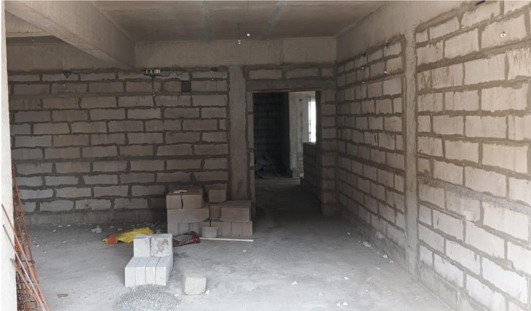
BLOCK 2 POUR 2 – FIRST FLOOR BLOCK WORK COMPLETED
