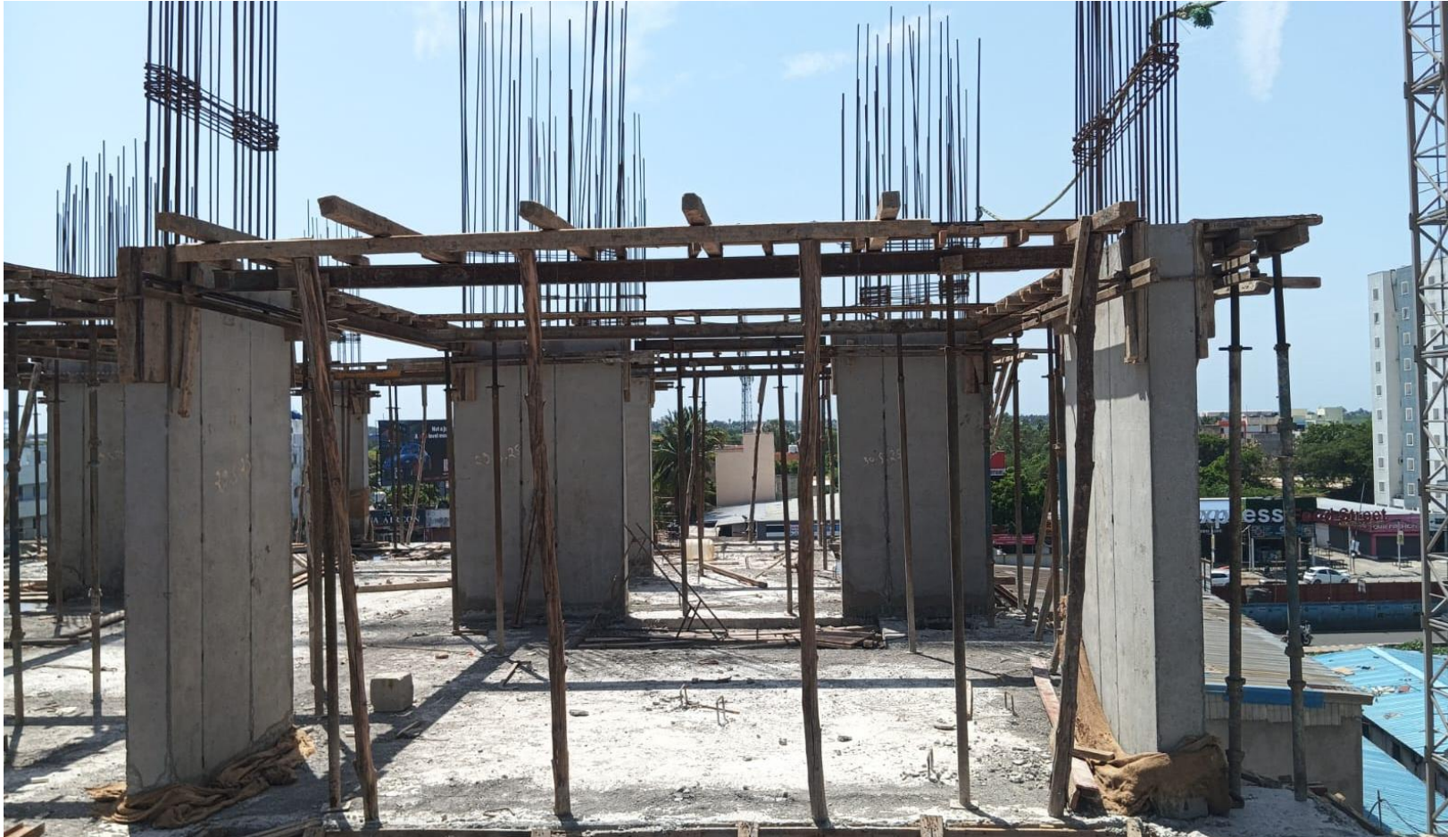
BLOCK 2 POUR 2 – FOURTH FLOOR ROOF SLAB SHUTTERING WORK IN PROGRESS
