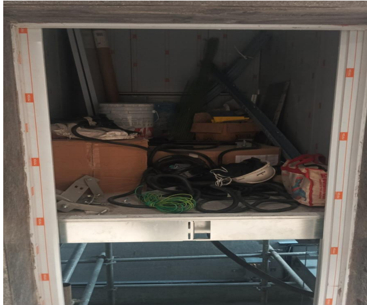
LIFT 004 CABIN ERECTION COMPLETED
