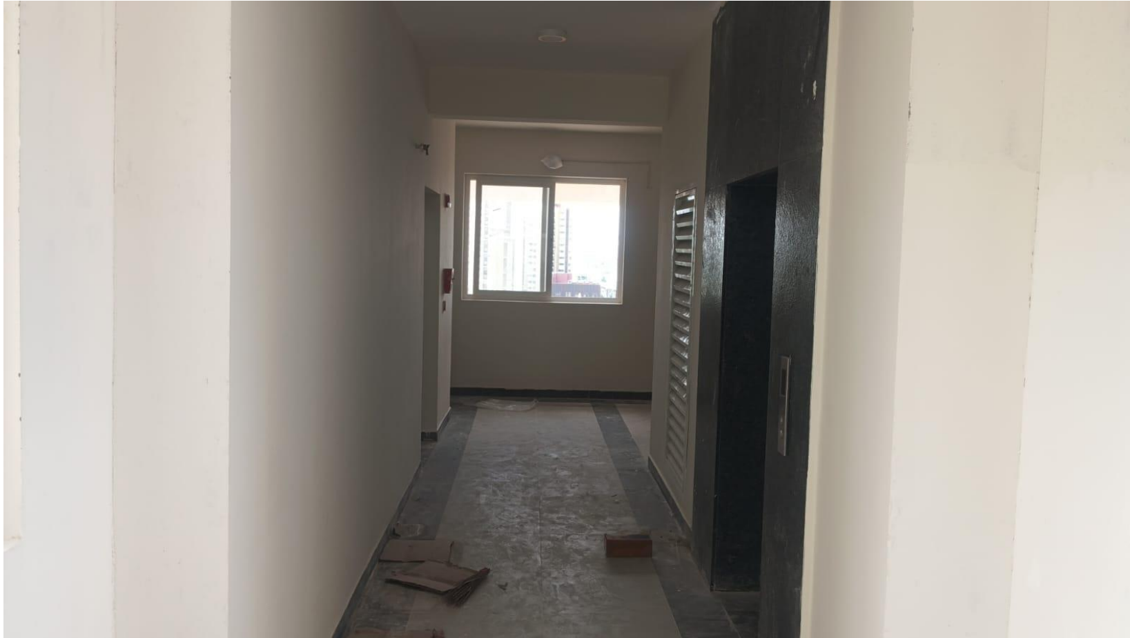
BLOCK 2 CORRIDOR PAINTING WORK IN PROGRESS
