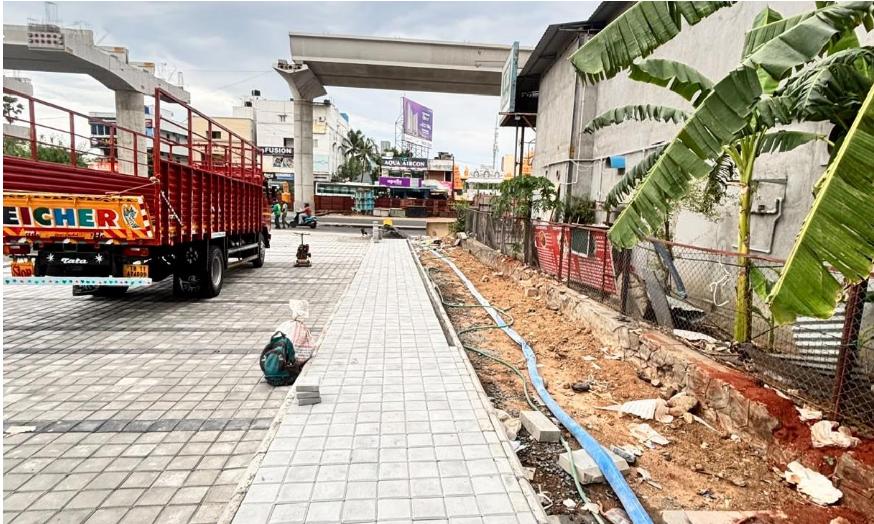
WALKWAY PAVER LAYING WORK IN PROGRESS
