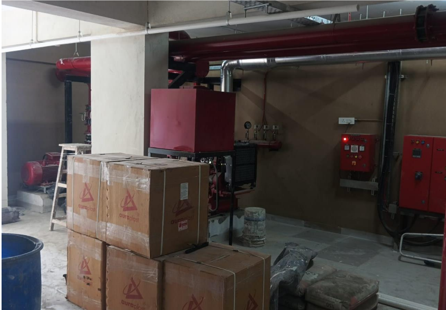
WTP PUMP ROOM PAINTING WORK COMPLETED
