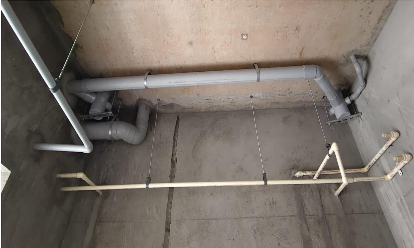
BLOCK 1 – TWELFTH FLOOR PLUMBING SUSPENDED LINE WORK COMPLETED
