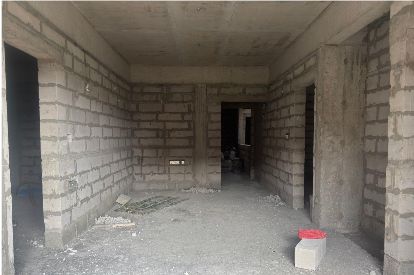
BLOCK 2 POUR 2 – SECOND FLOOR BLOCK WORK COMPLETED
