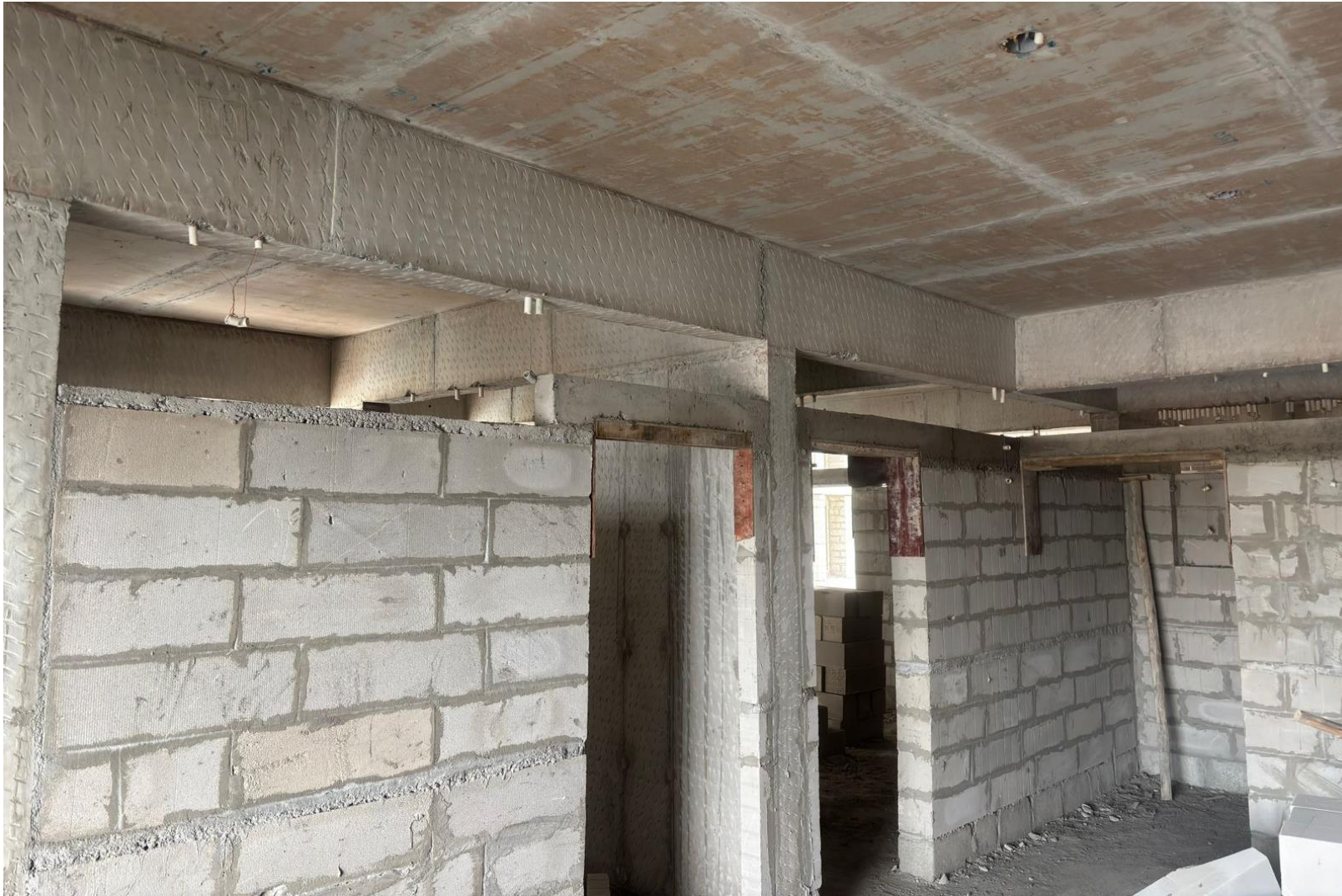
BLOCK 2 POUR 2 – FOURTH FLOOR BLOCK WORK IN PROGRESS
