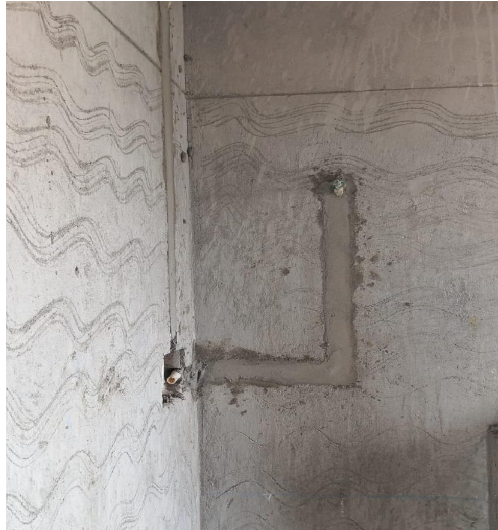
BLOCK 2 POUR 1 – NINTH FLOOR TOILET ELECTRICAL WORK IN PROGRESS
