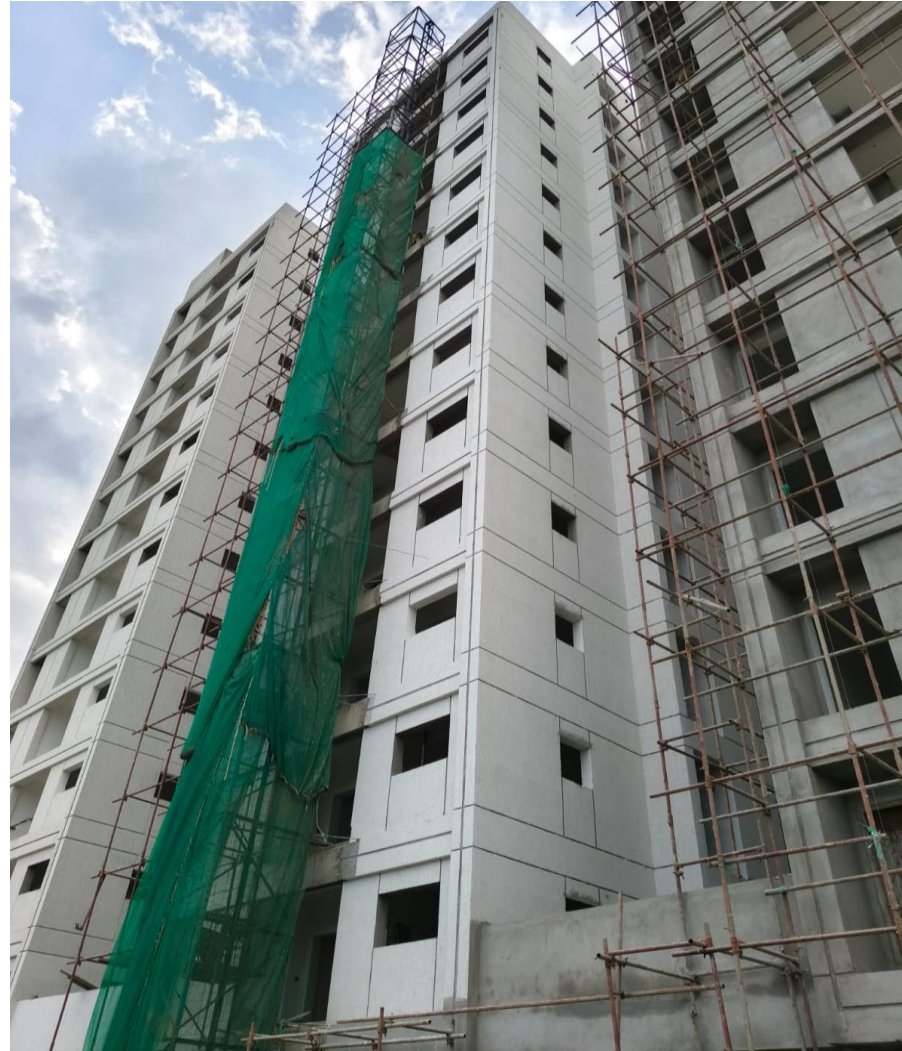
BLOCK 1 – SOUTH SIDE EXTRENAL TEXTURE WORK IN PROGRESS
