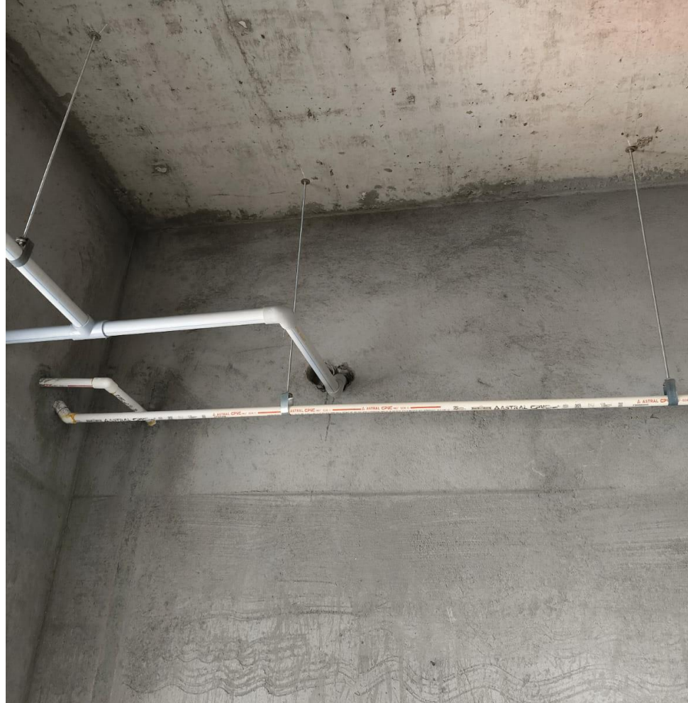
BLOCK 1 – THIRTEENTH FLOOR PLUMBING CONCEALED LINE COMPLETED
