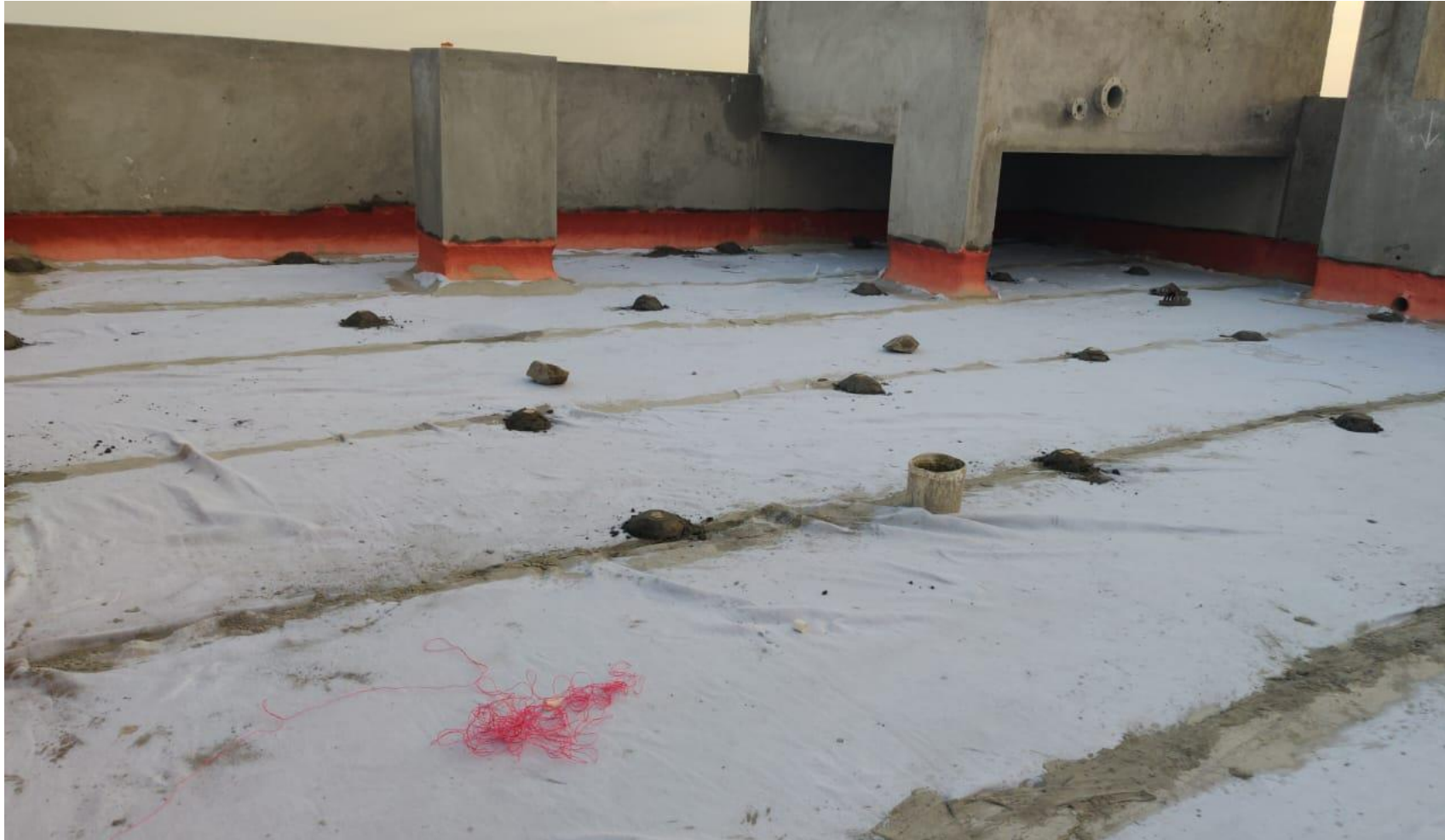
BLOCK 1 – TERRACE BAY 1 SCREED CONCRETE BUTTON MARK FIXING WORK IN PROGRESS
