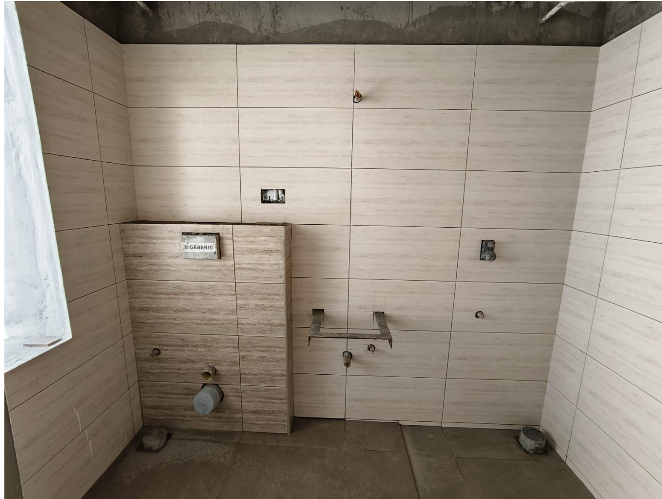
BLOCK 1 – NINTH FLOOR TOILET WALL TILES LAYING WORK IN PROGRESS
