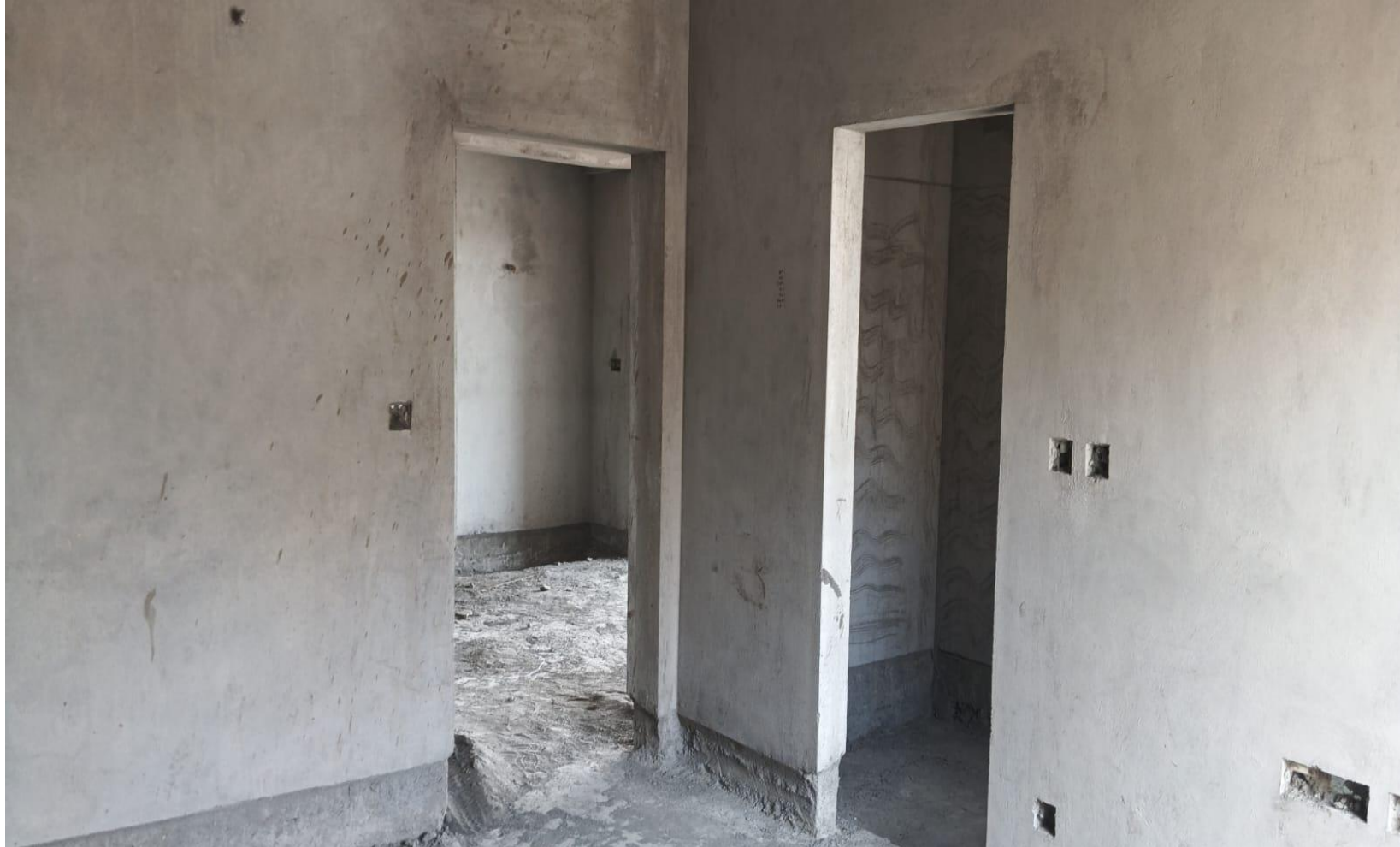
BLOCK 2 POUR 1 – THIRTEENTH FLOOR INNER PLASTERING COMPLETED
