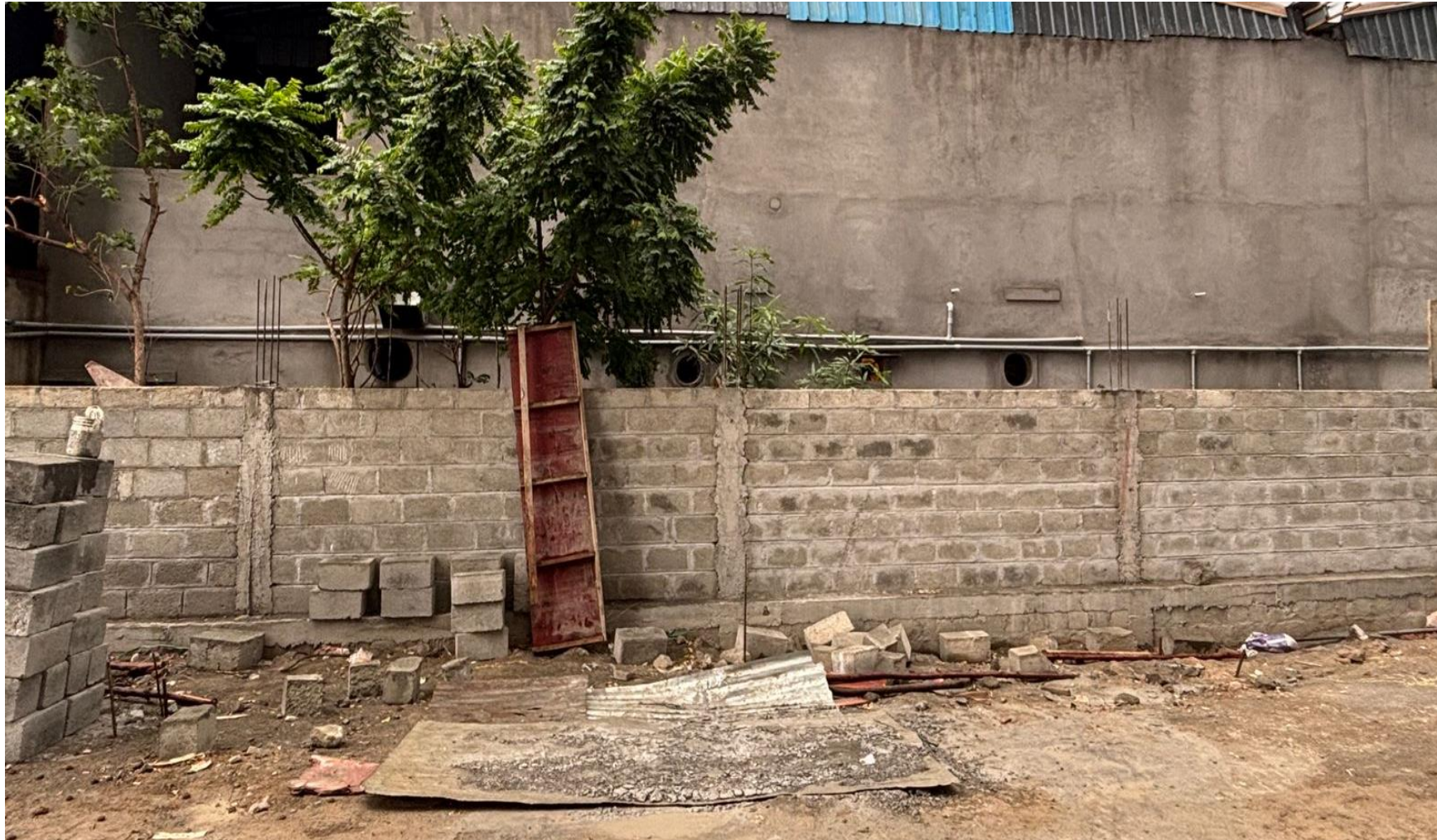
COMPOUND WALL EAST SIDE – BLOCK WORK IN PROGRESS
