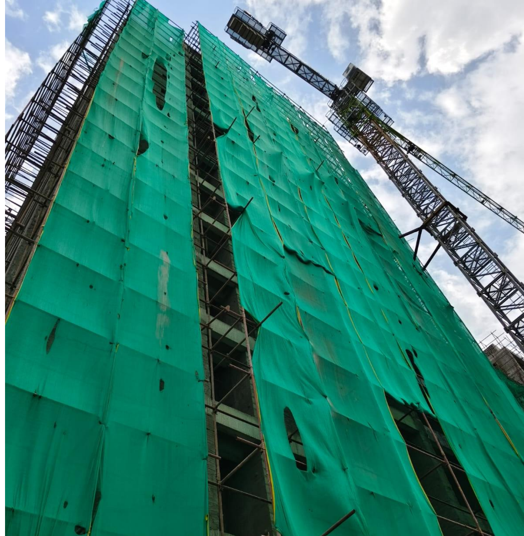
BLOCK 1 – EAST SIDE EXTERNAL PLASTERING WORK IN PROGRESS
