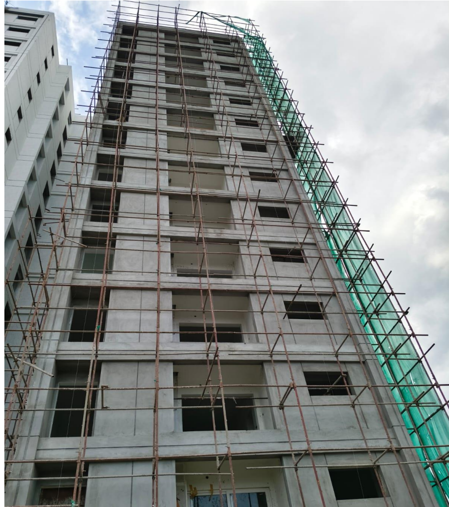
BLOCK 1 – SOUTH SIDE EXTRENAL PLASTERING WORK IN PROGRESS
