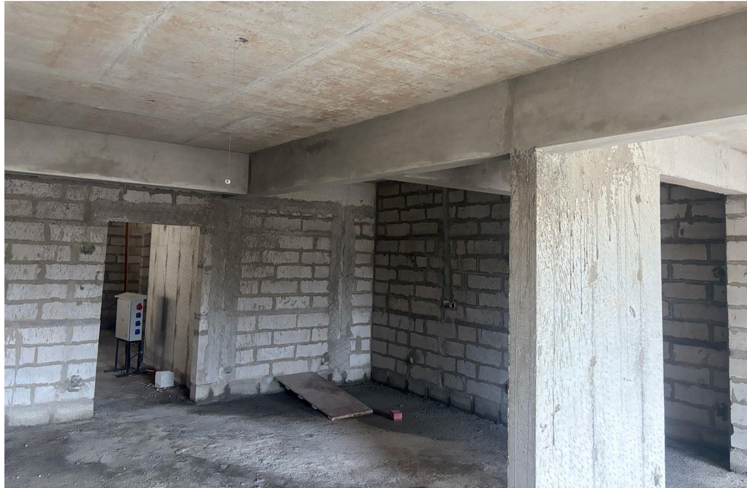
BLOCK 2 POUR 2 – FIRST FLOOR GYM INTERNAL PLASTERING WORK IN PROGRESS
