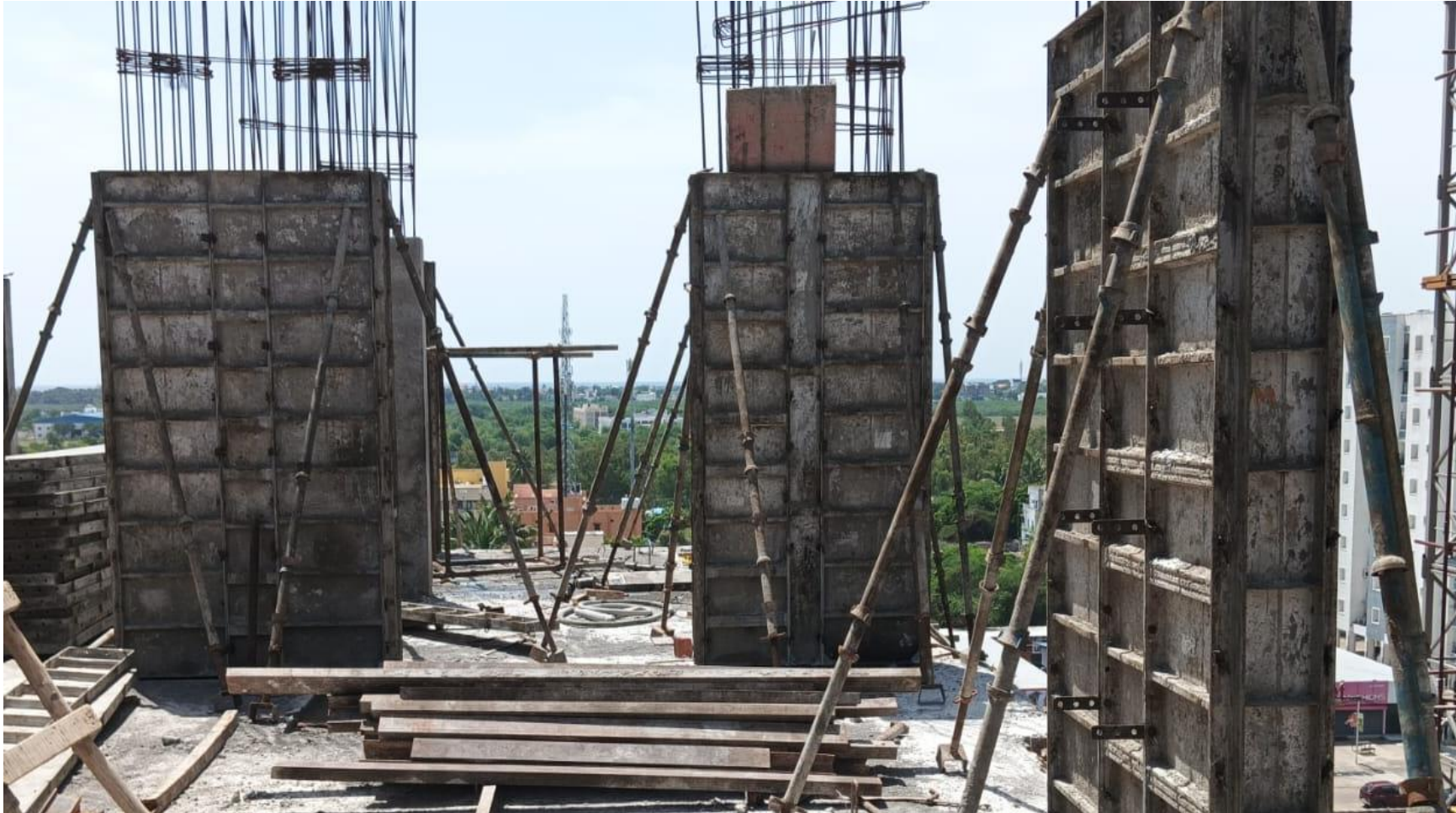
BLOCK 2 POUR 2 – TENTH FLOOR COLUMN CONCRETE IN PROGRESS
