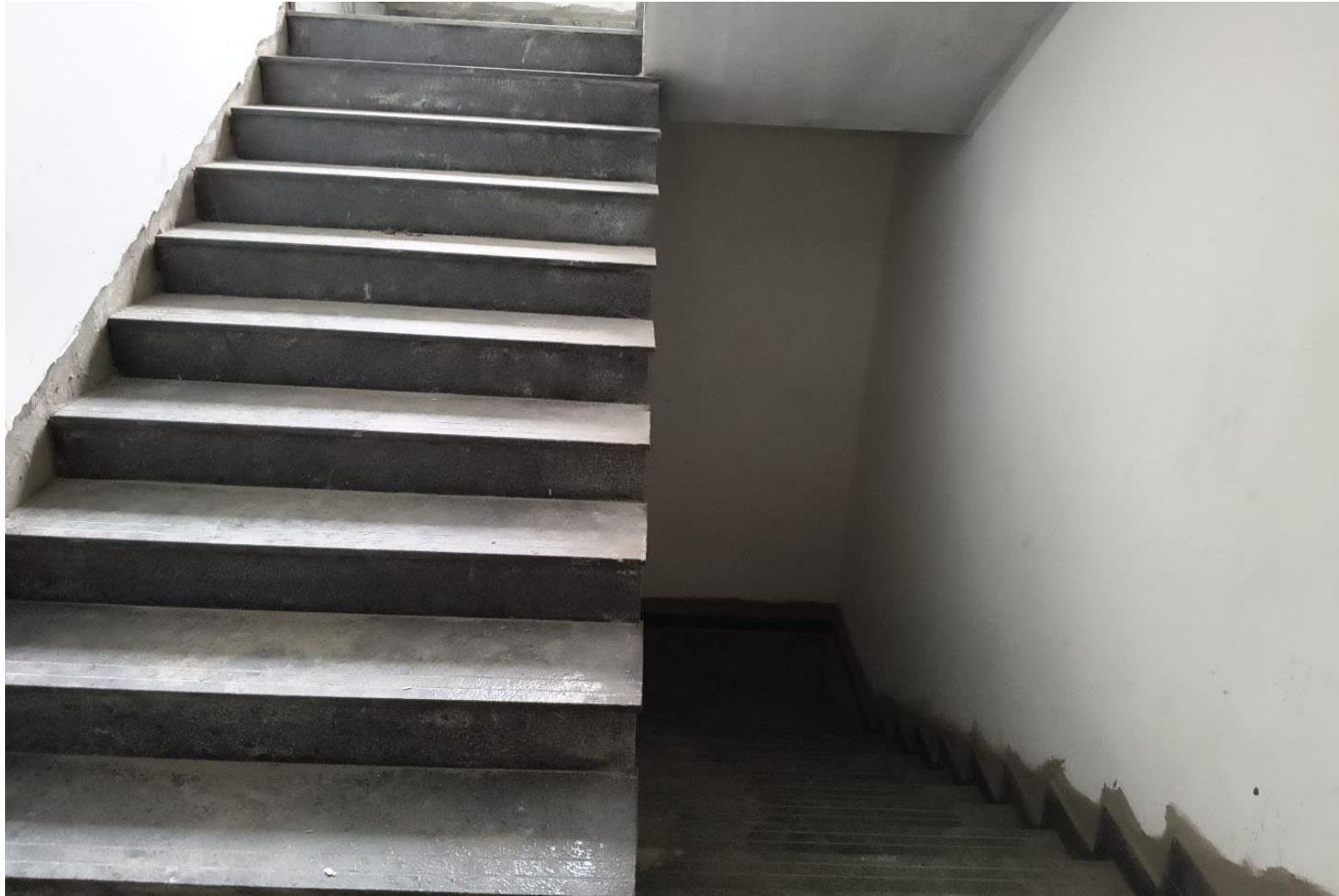
BLOCK 1 – FIFTH FLOOR STAIRACSE GRANITE LAYING WORK IN PROGRESS
