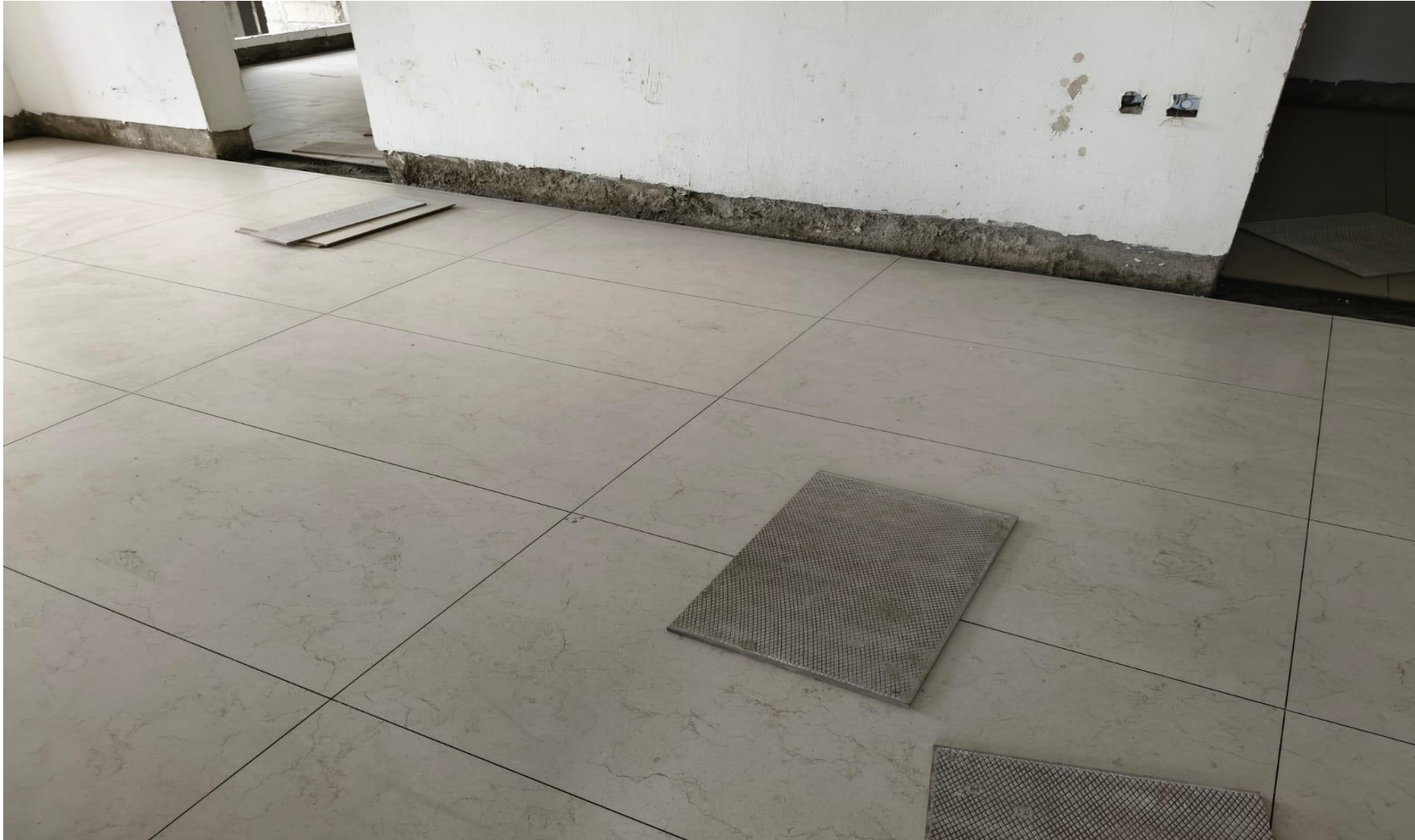
BLOCK 1 – EIGHTH FLOOR TILES LAYING WORK IN PROGRESS
