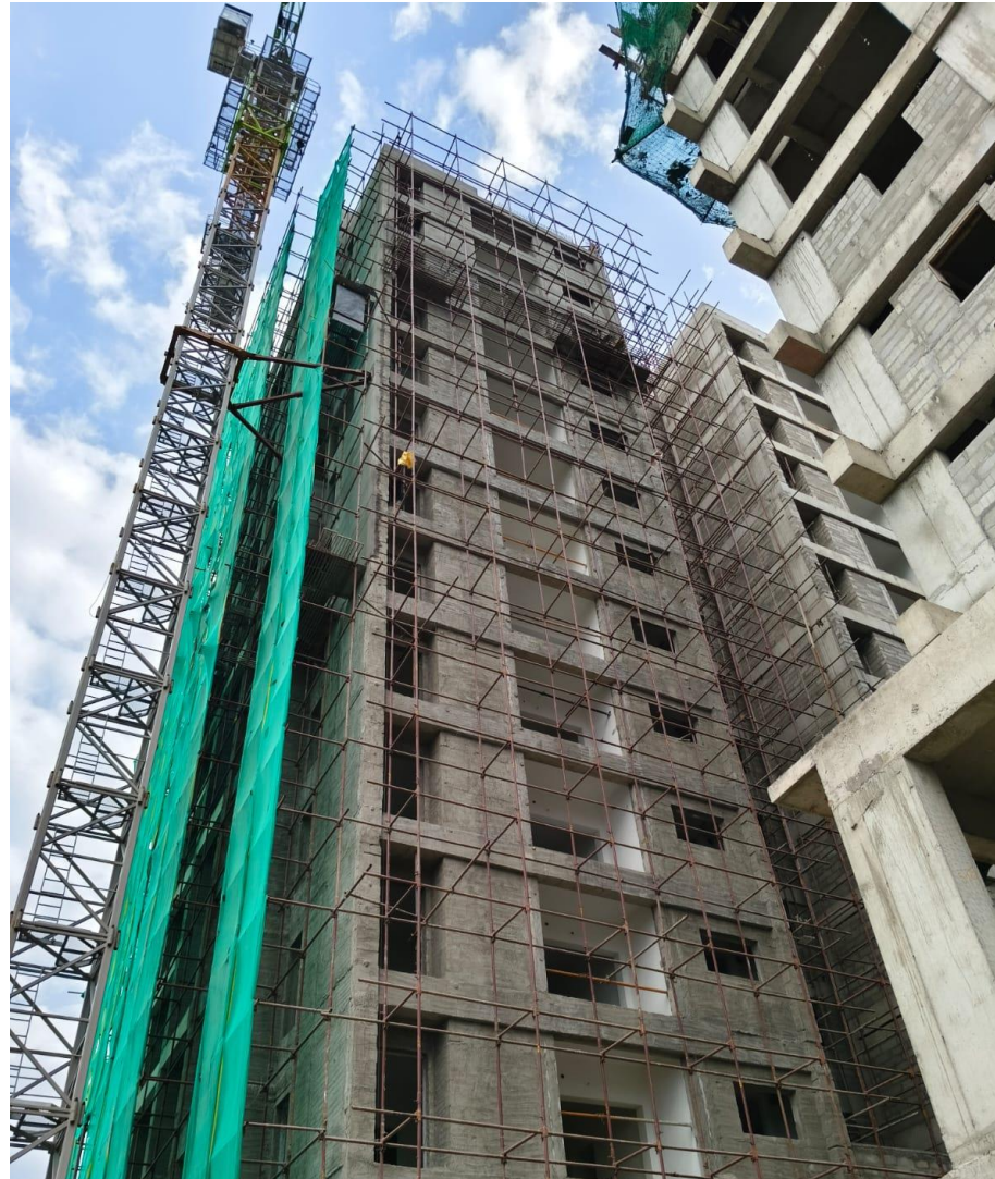
BLOCK 1 – NORTH SIDE EXTERNAL PLASTERING WORK IN PROGRESS
