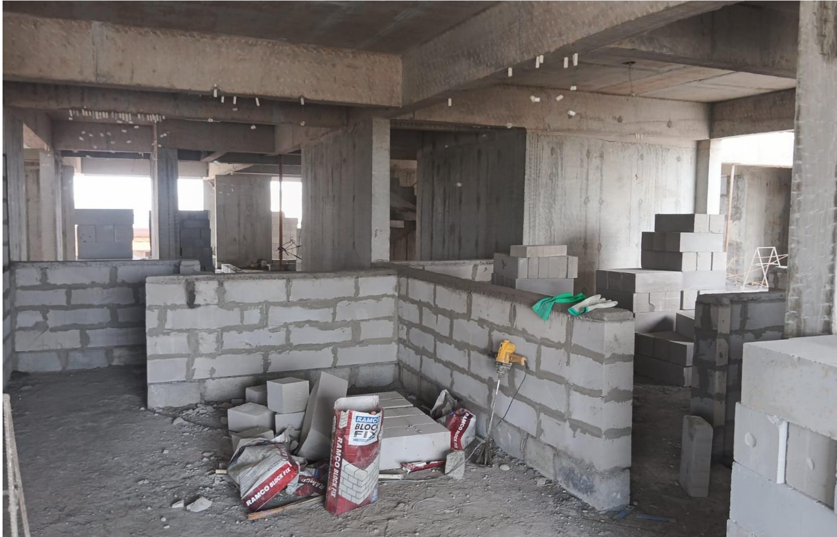
BLOCK 2 POUR 2 – FIFTH FLOOR BLOCK WORK IN PROGRESS
