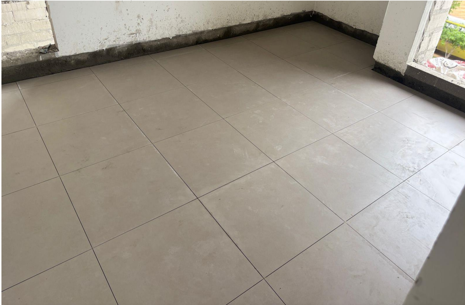
BLOCK 2 POUR 1 – FOURTH & FIFTH TILES LAYING WORK IN PROGRESS
