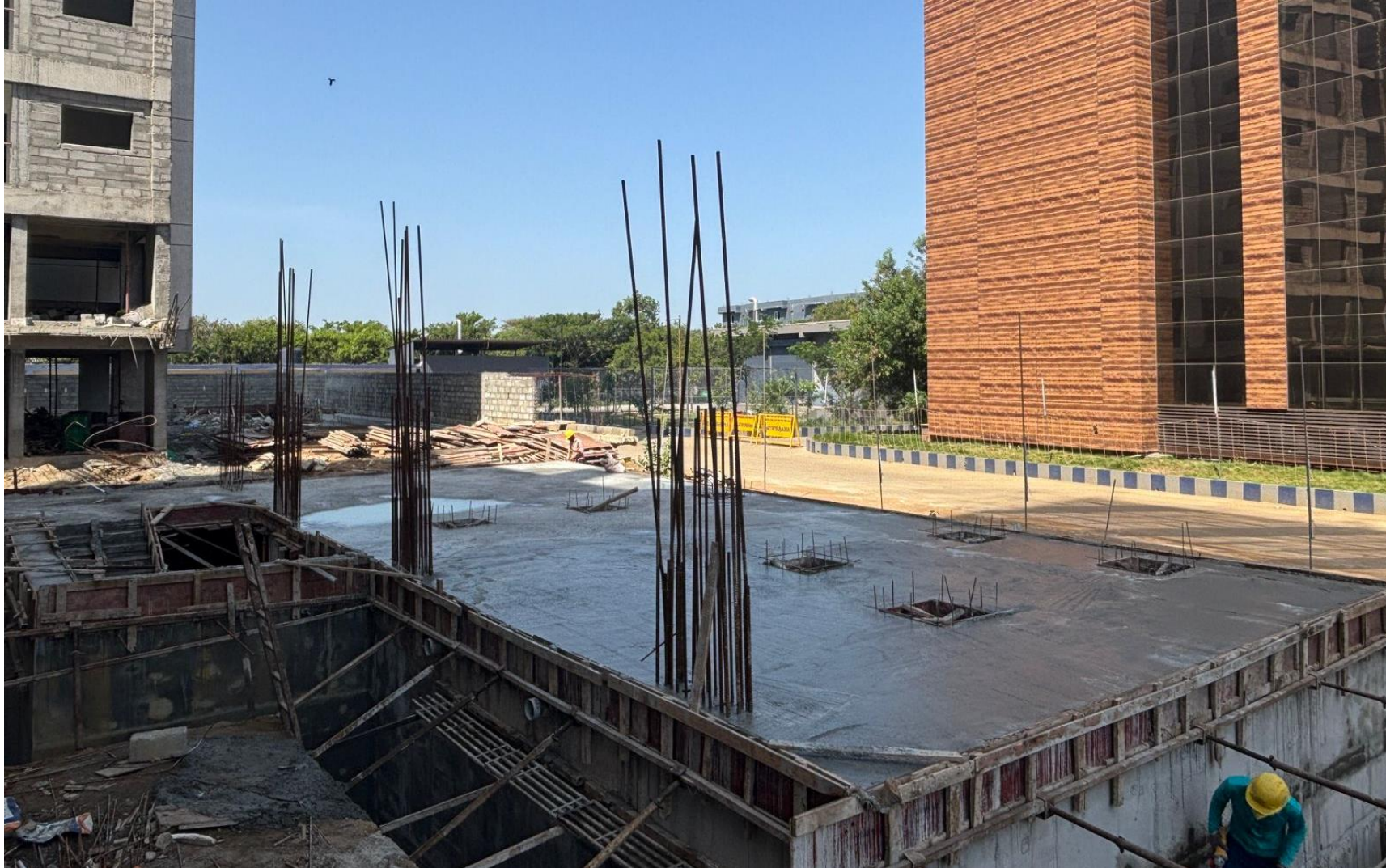
STP COVER SLAB CONCRETE COMPLETED
