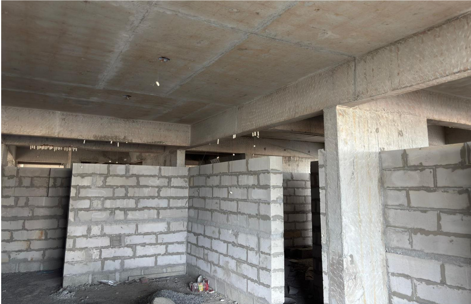
BLOCK 2 POUR 2 – THIRD FLOOR BLOCK WORK IN PROGRESS
