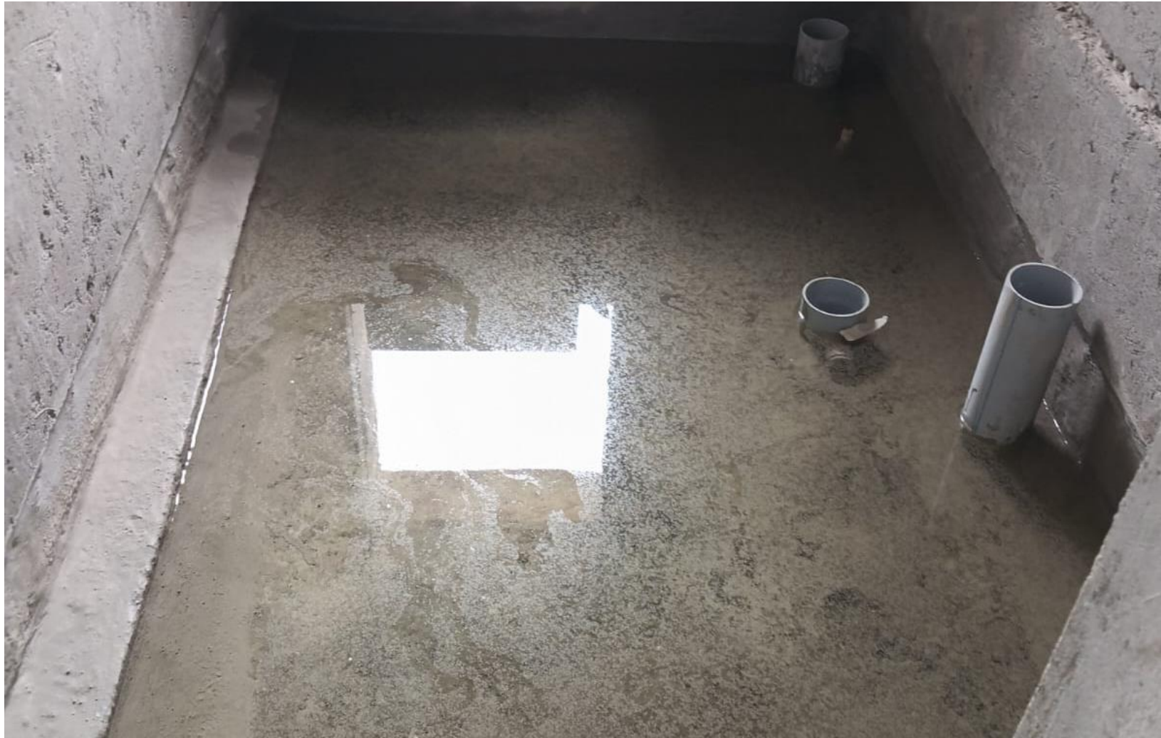
BLOCK 2 POUR 1 – TWELFTH SUNKEN WATER PROOFING WORK IN PROGRESS
