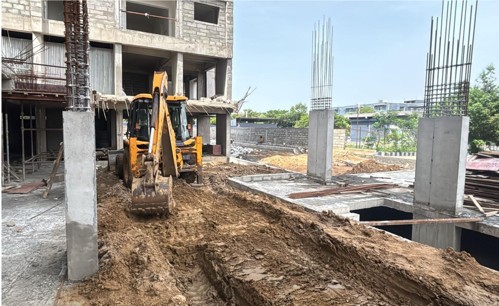
STP EXTERNAL BACK FILLING WORK IN PROGRESS
