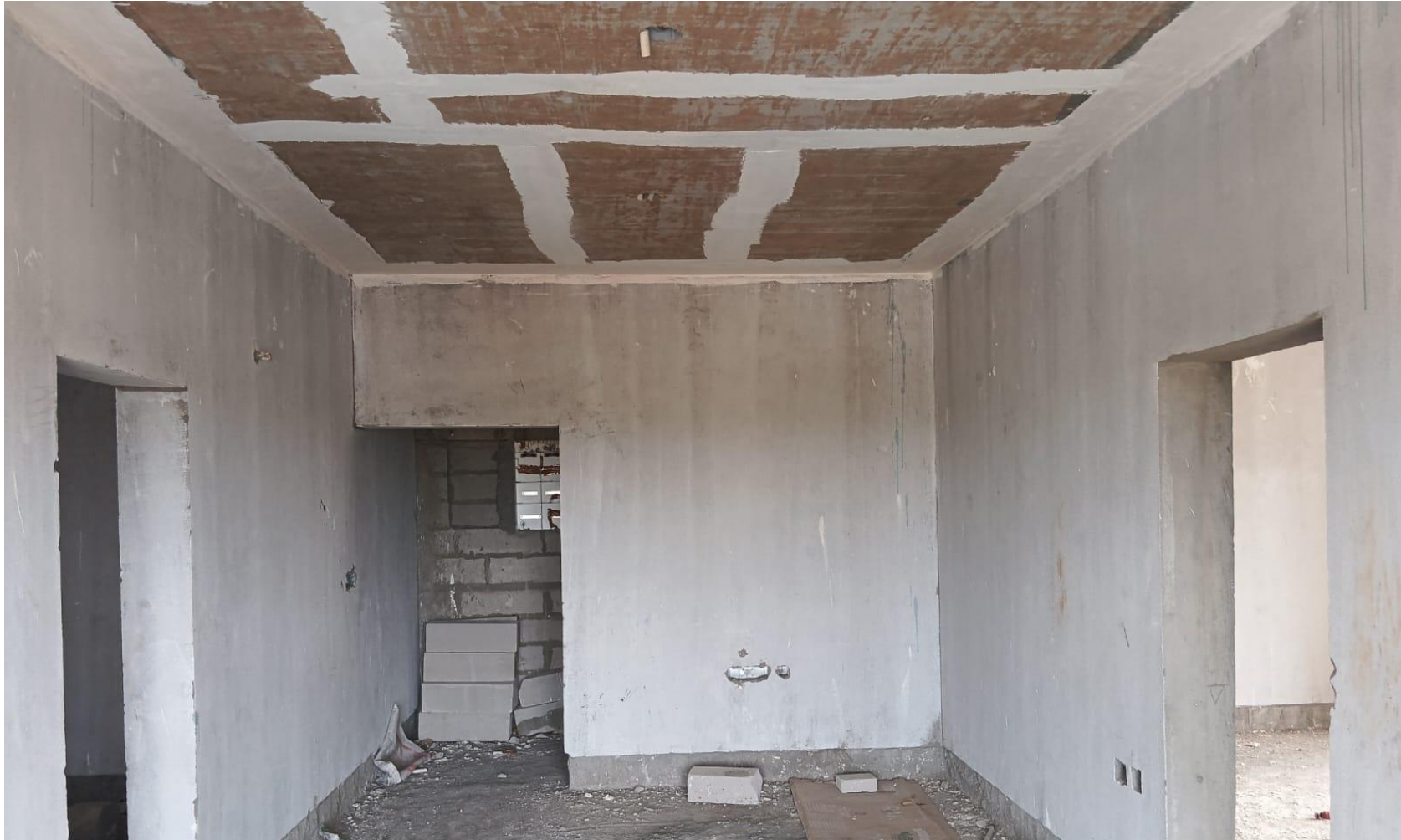
BLOCK 2 POUR 1 – SEVENTH & EIGHTH CEILING PUTTY WORK IN PROGRESS
