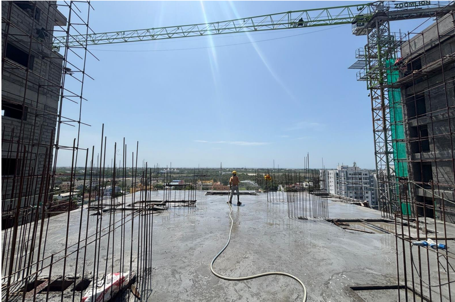
BLOCK 2 POUR 2 – NINTH FLOOR ROOF SLAB CONCRETE COMPLETED
