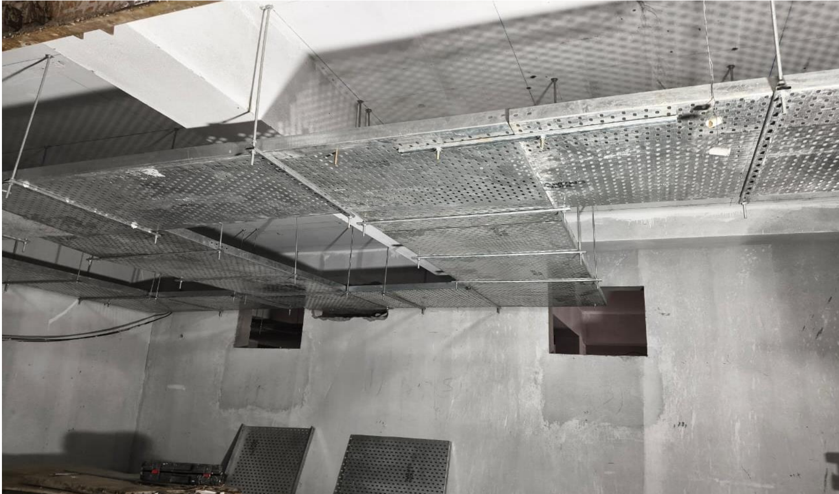
BLOCK 1 ELECTRICAL PANEL ROOM WORK IN PROGRESS
