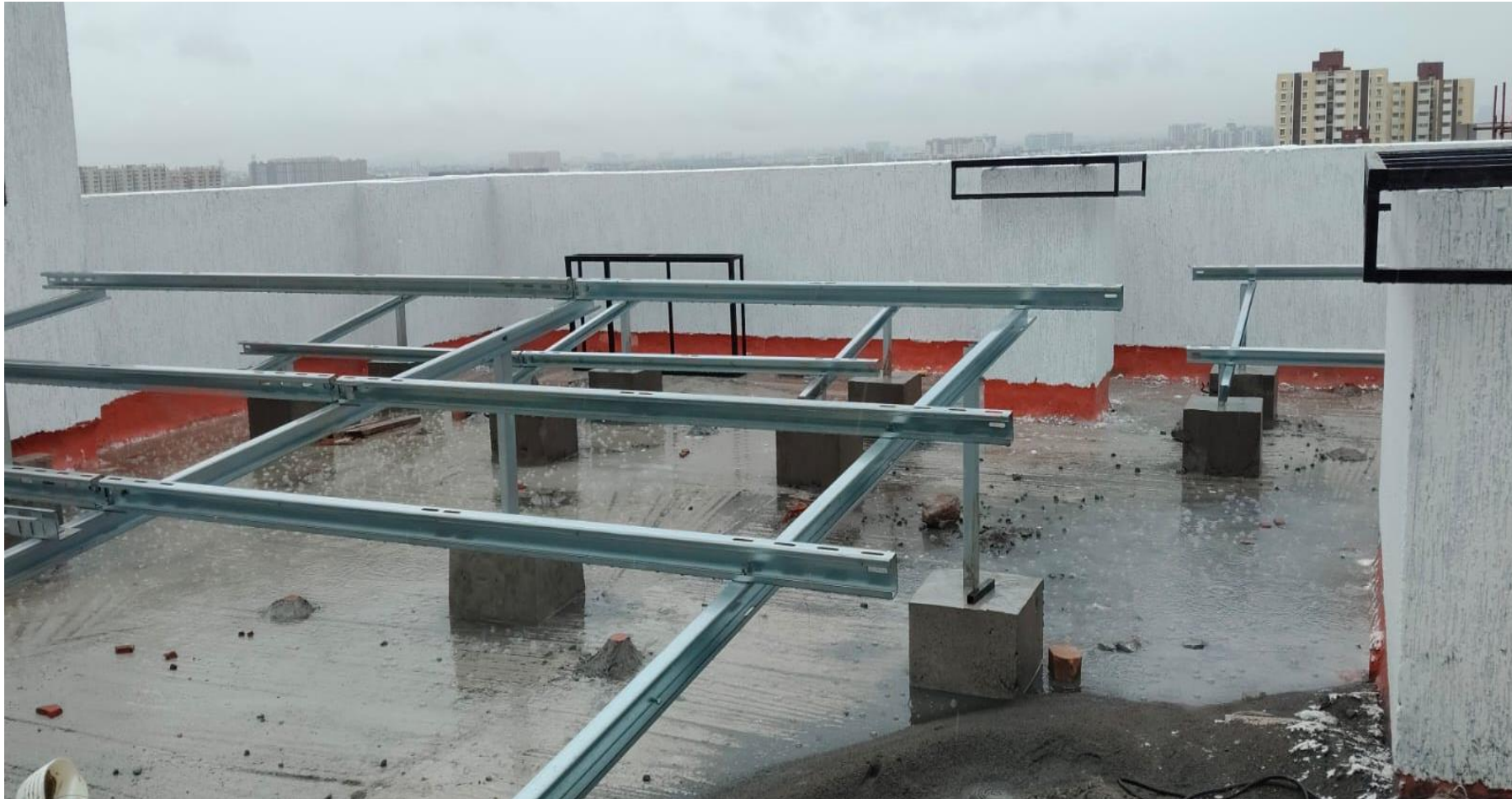
BLOCK 1- TERRACE OTS COVERING WORK IN PROGRESS
