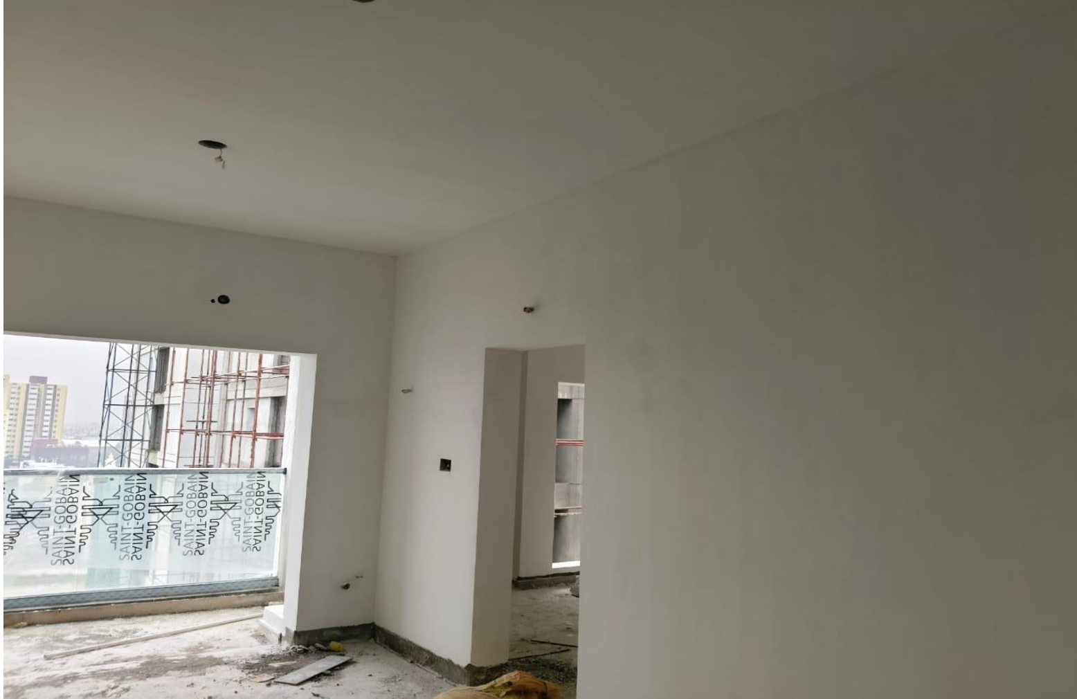
BLOCK 1 - 13 th FLOOR PRIMER WORK IN PROGRESS
