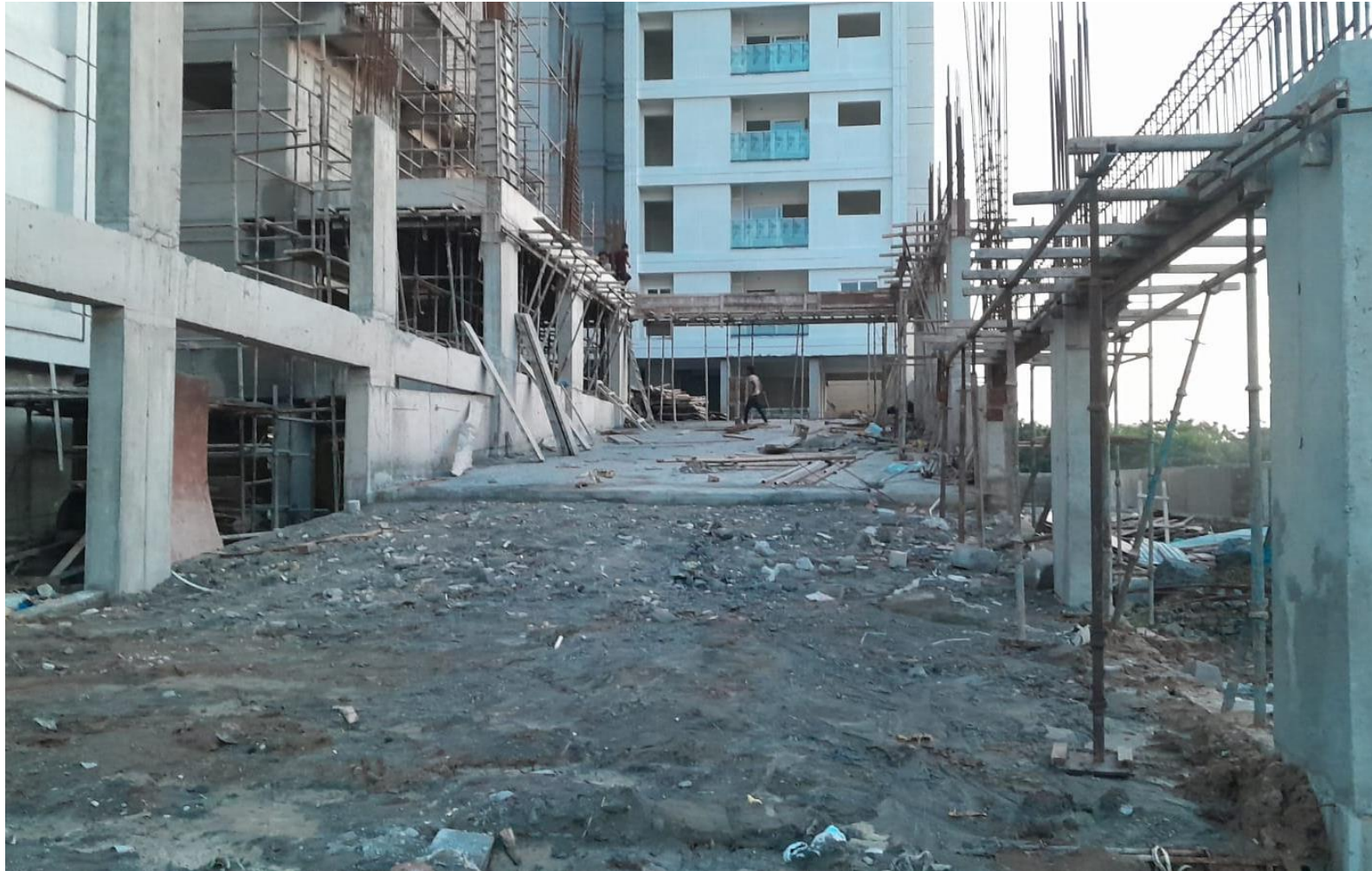
RAMP COLUMN & BEAM WORK IN PROGRESS
