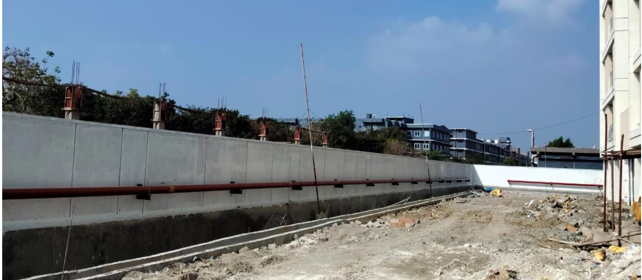
FIRE FIGHTING HYDRANT PIPE LAYING WORK IN PROGRESS
