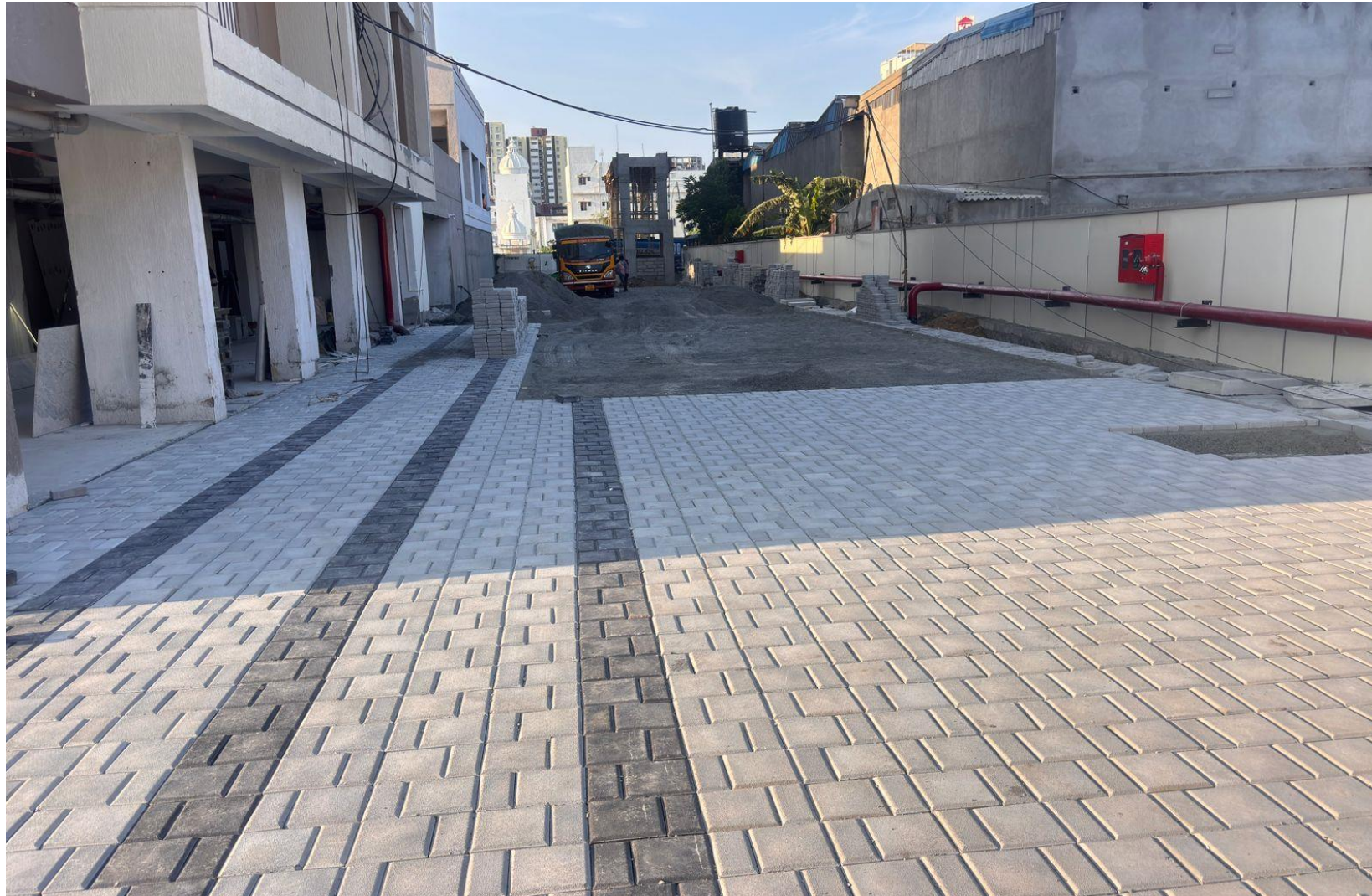
EAST SIDE PAVER BLOCK LAYING WORK IN PROGRESS
