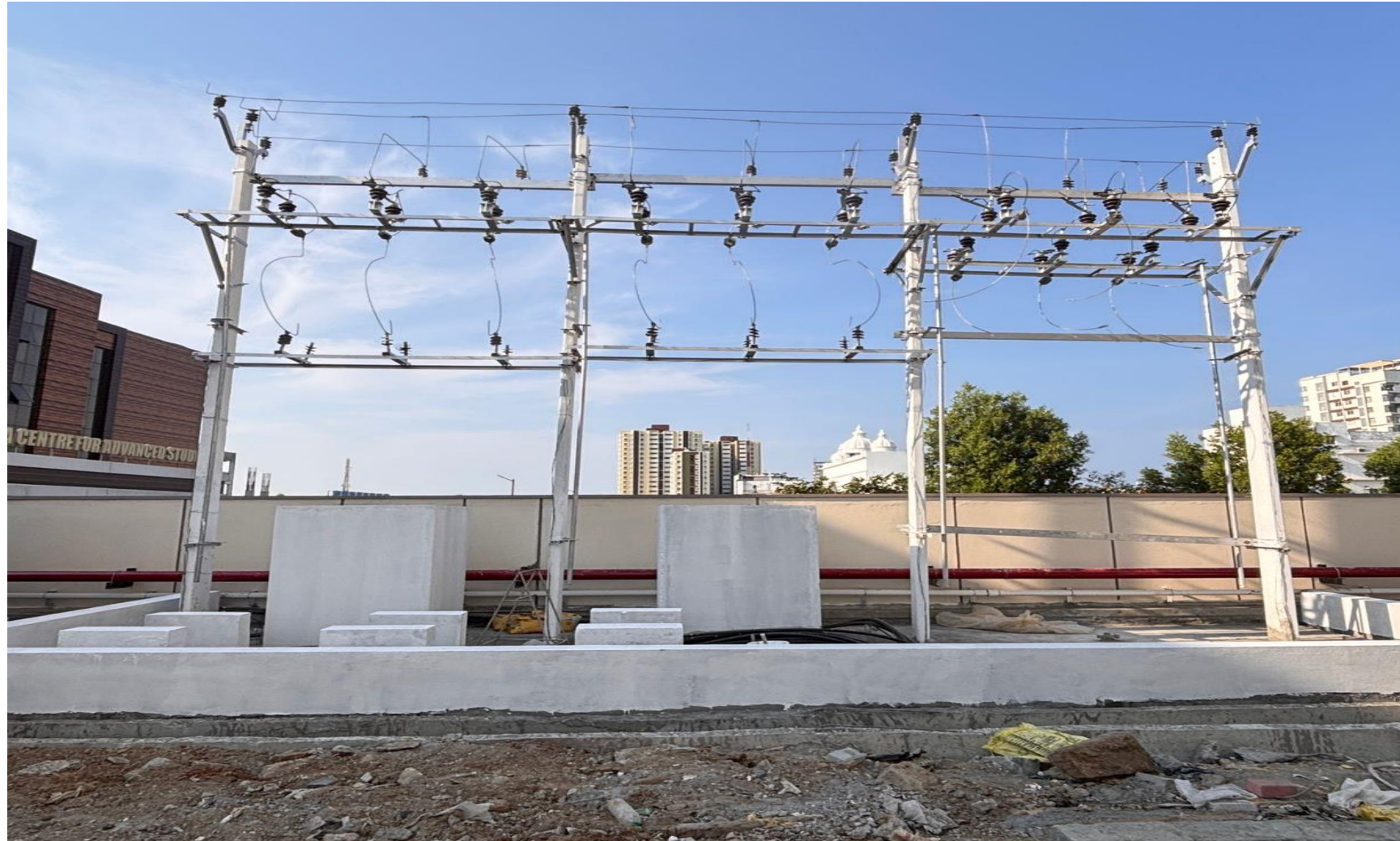
TRANSFORMER YARD CIVIL WORKS IN PROGRESS
