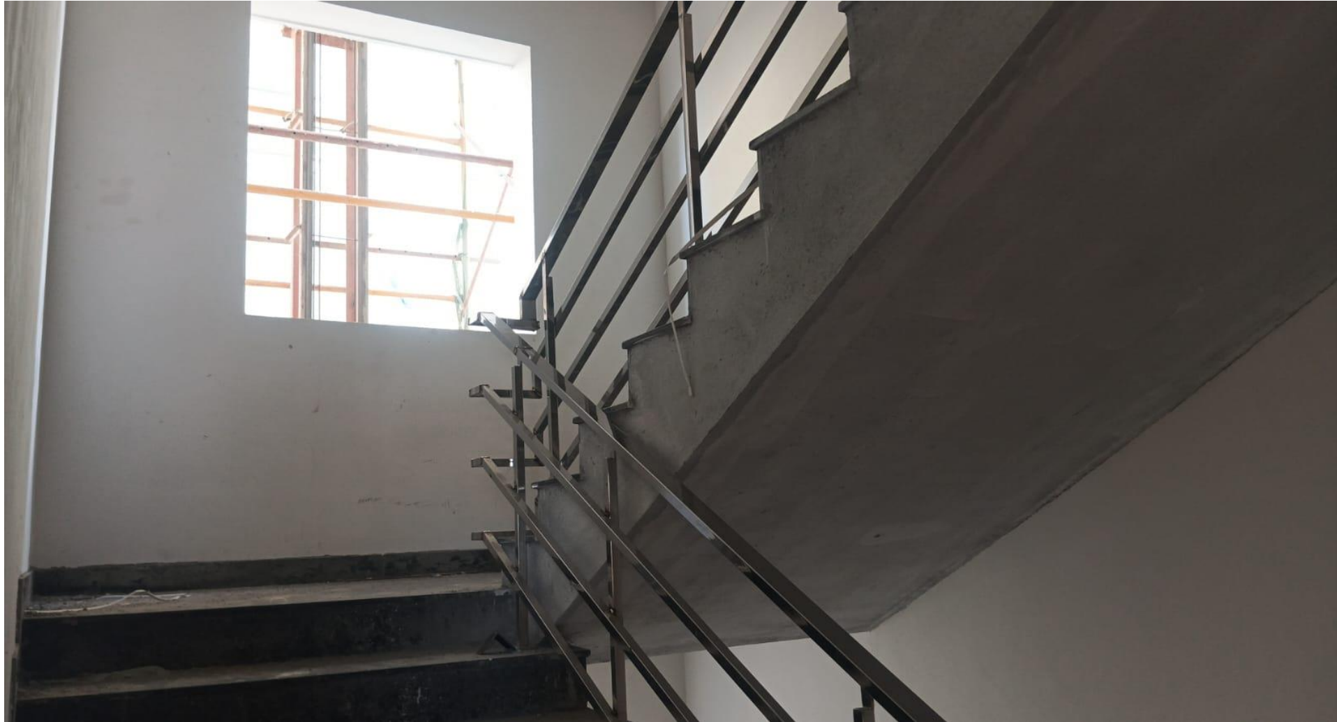
BLOCK 2 POUR 1 – STAIRCASE SS HANDRAIL FIXING WORK IN PROGRESS
