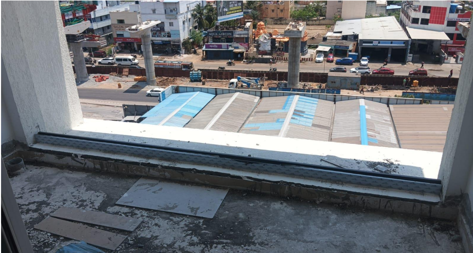
BLOCK 2 POUR 2 – BALCONY GLASS RAIL BOTTOM PROFILE FIXING IN PROGRESS
