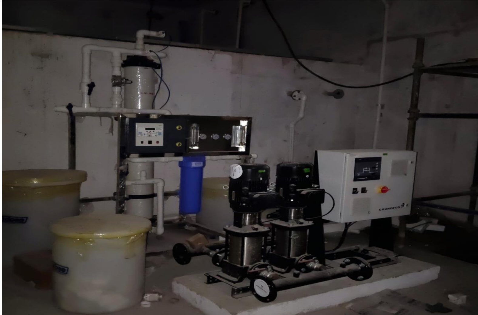
STP PUMP INSTALATION COMPLETED
