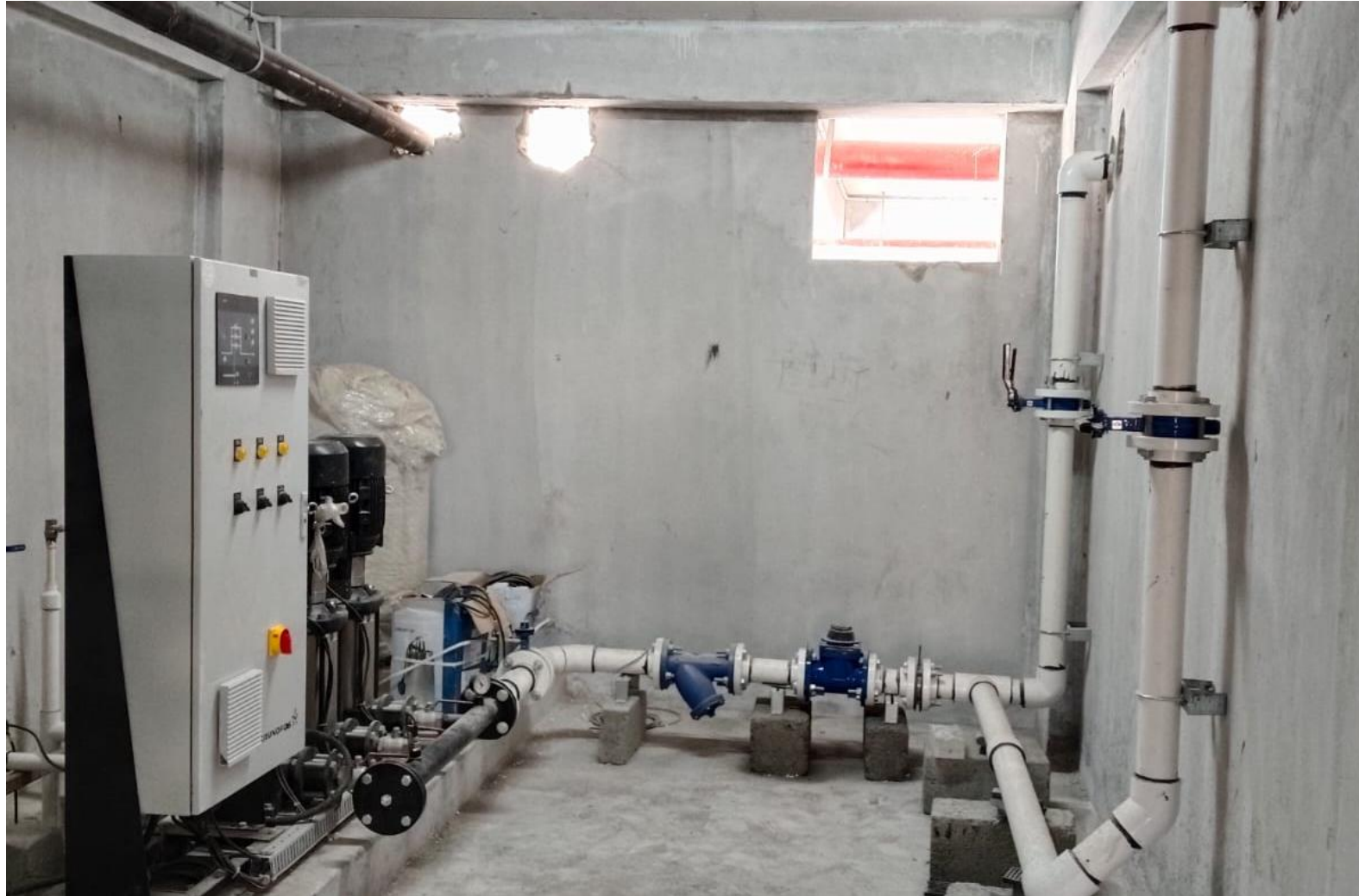
HNS PUMP INSTALATION COMPLETED
