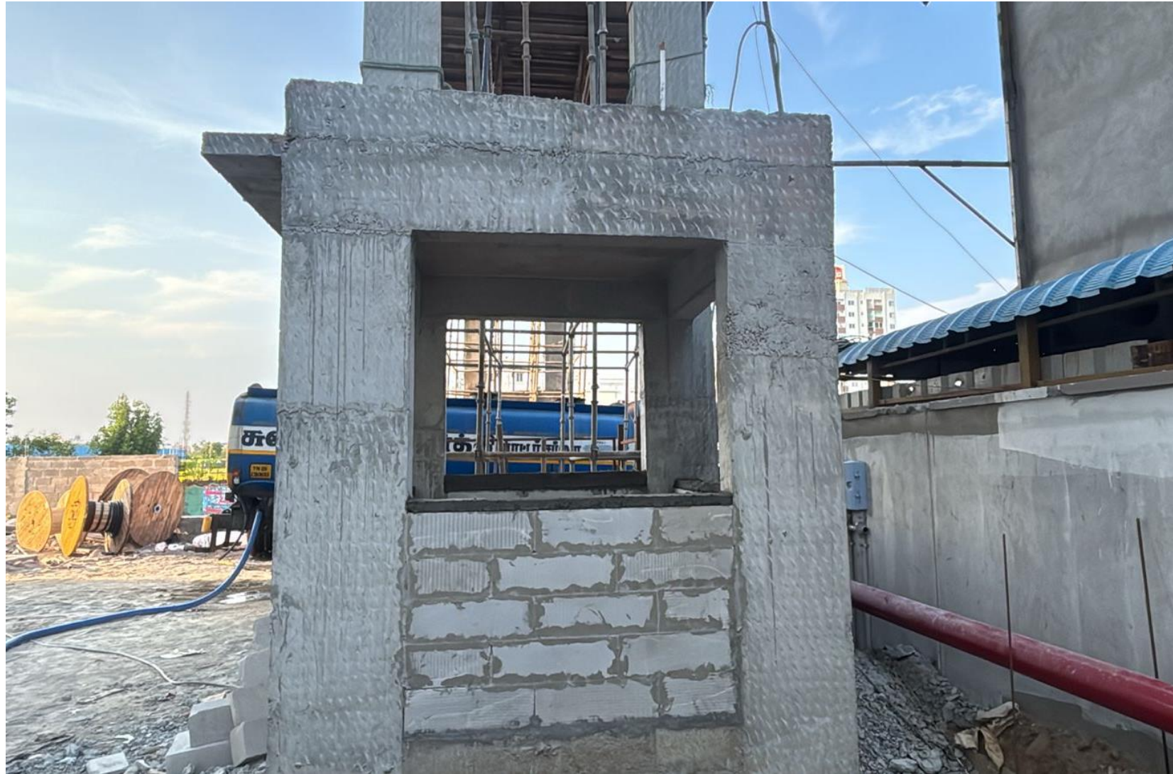
SECURITY CABIN BLOCKWORK IN PROGRESS
