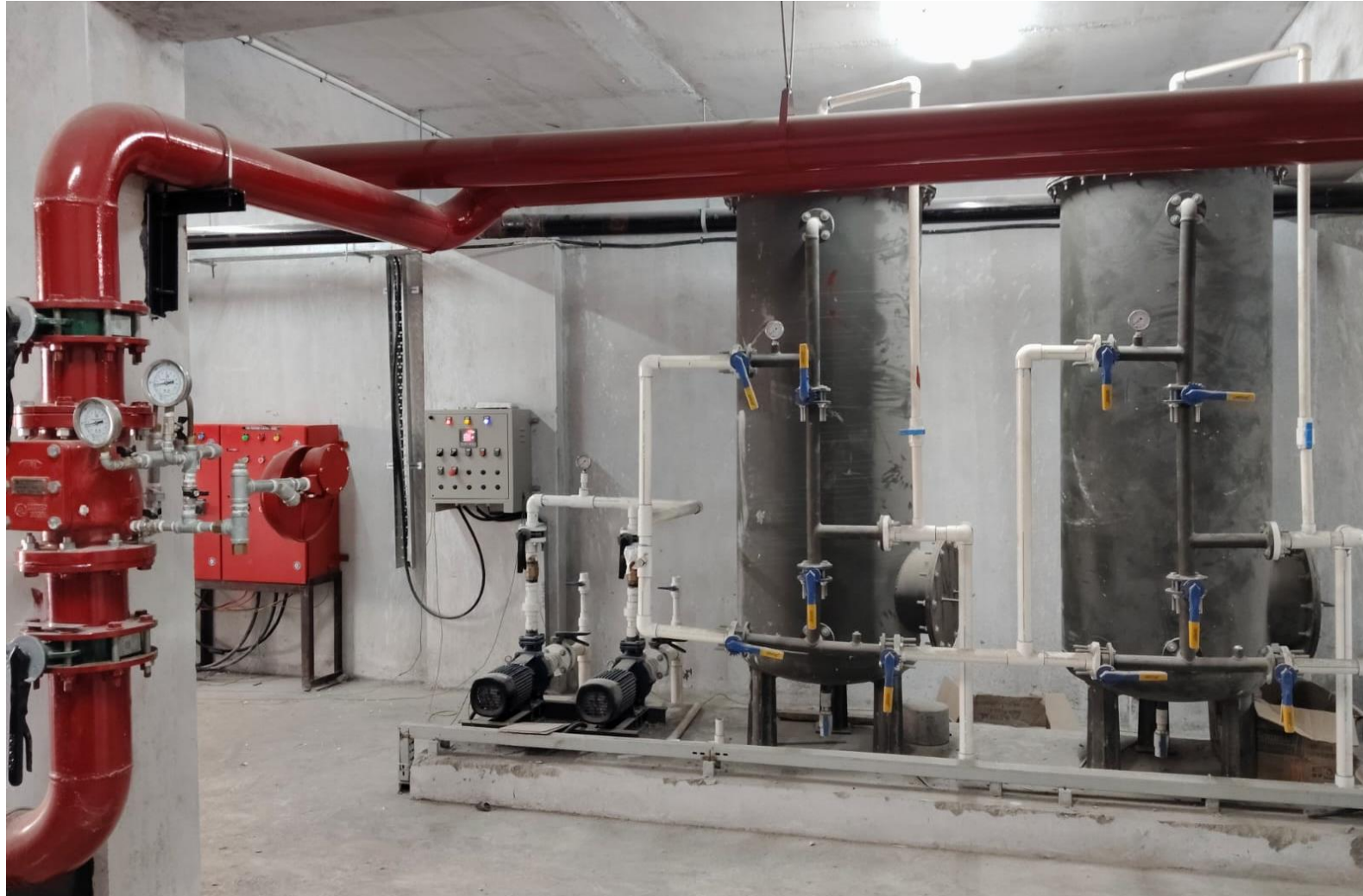
WTP & FIRE PUMP INSTALATION COMPLETED
