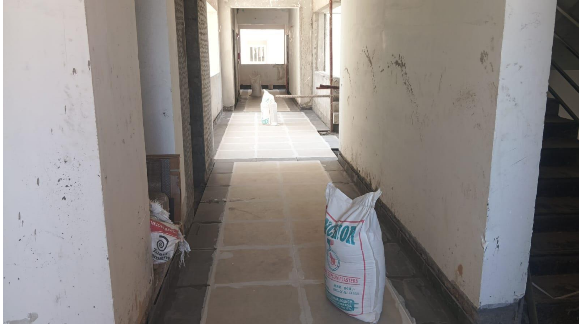
BLOCK 2 – CORRIDOR TILE LAYING COMPLETED
