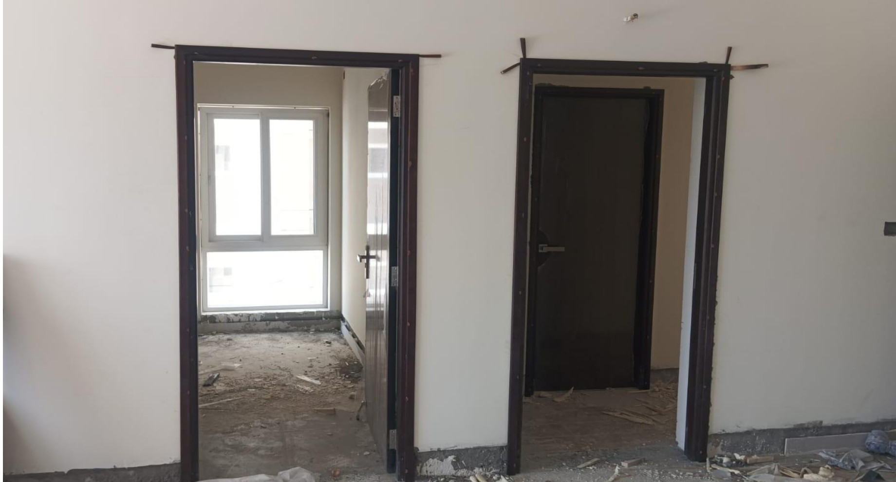
BLOCK 2 POUR 2 – 4 TH FLOOR DOOR FIXING WORK IN PROGRESS
