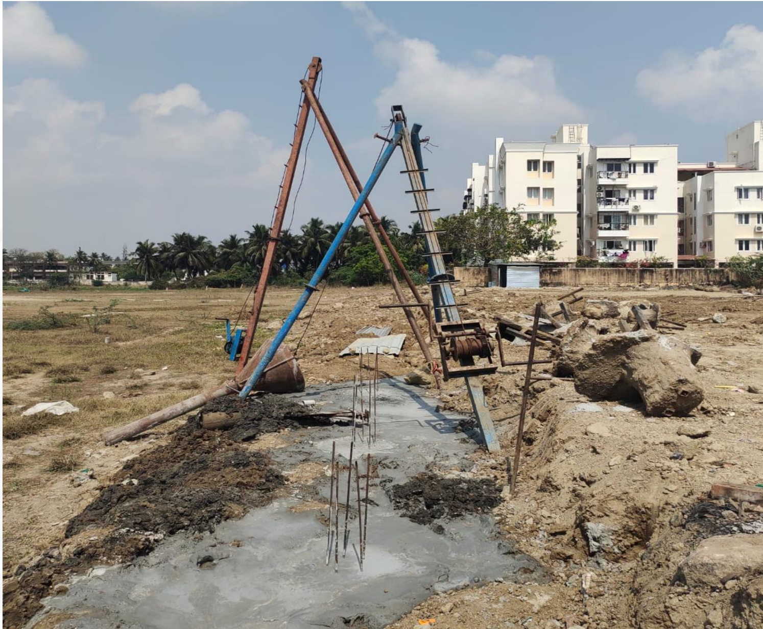
Compound Wall Pile Work In Progress
