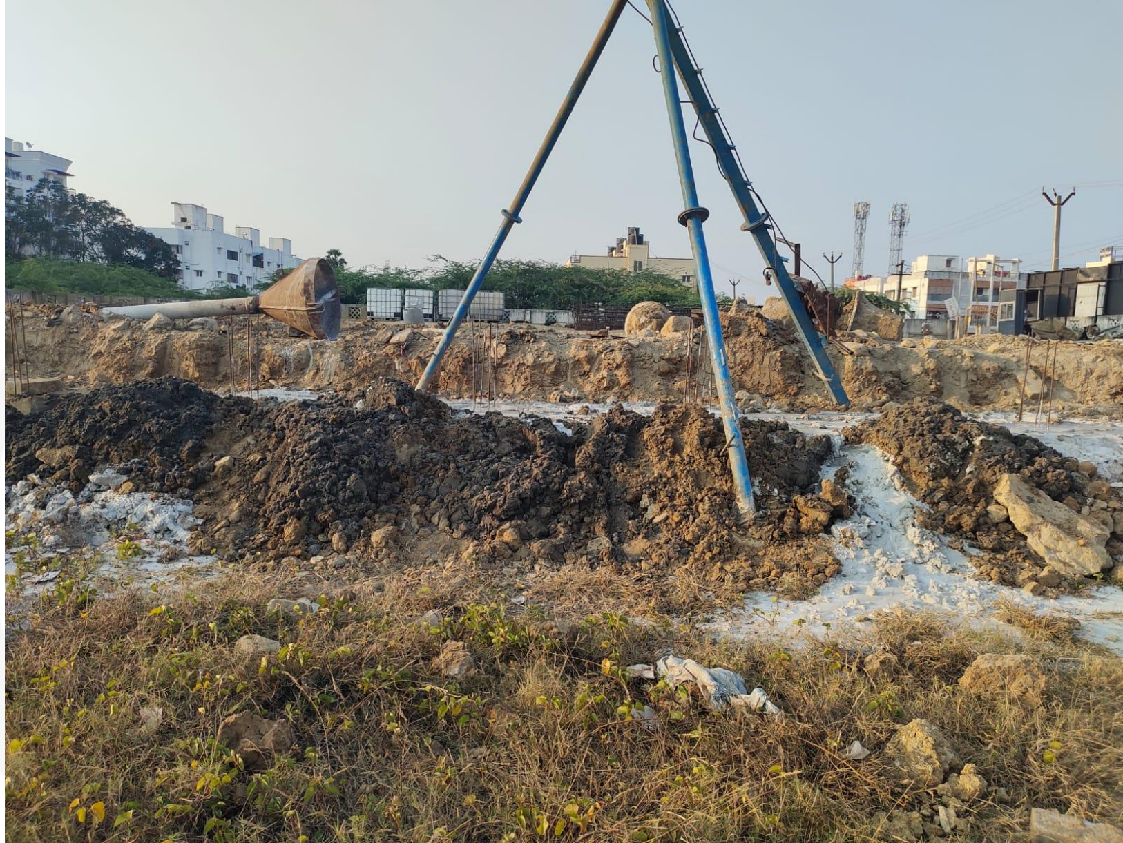
Compound Wall Pile Work In Progress
