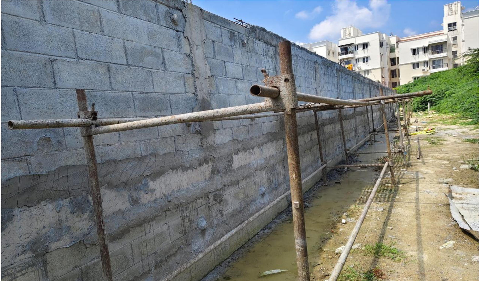
Compound Wall External Plastering North Side Work in progress.
