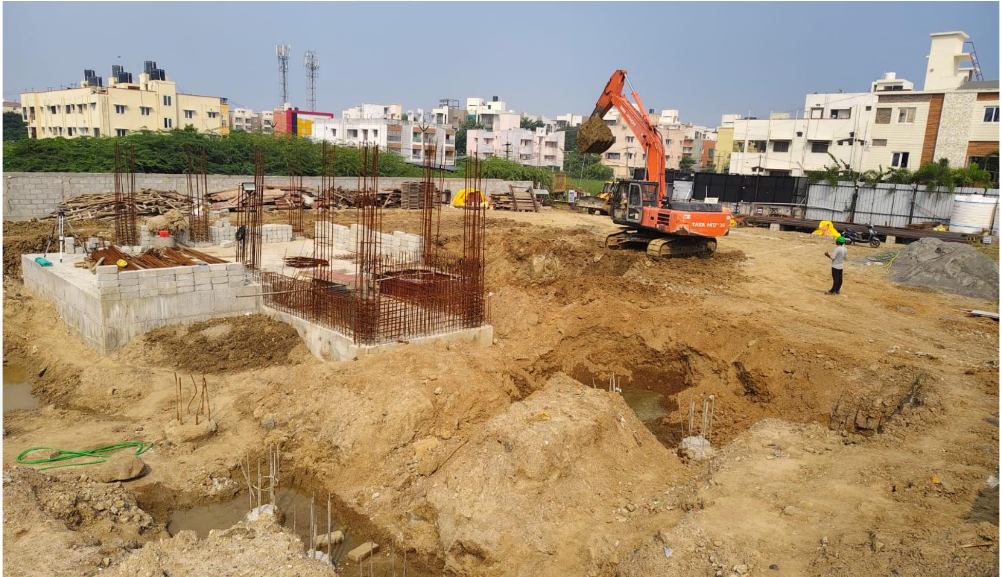
Overall Site View.
