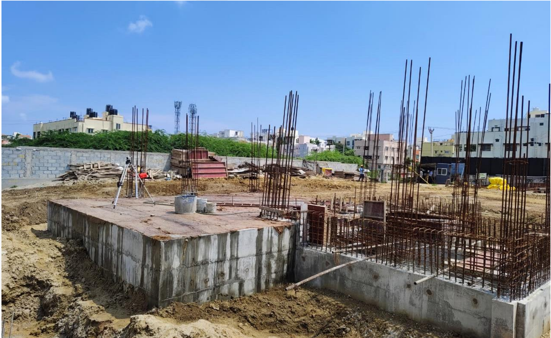
STP Cover Slab Concrete Work Completed.
