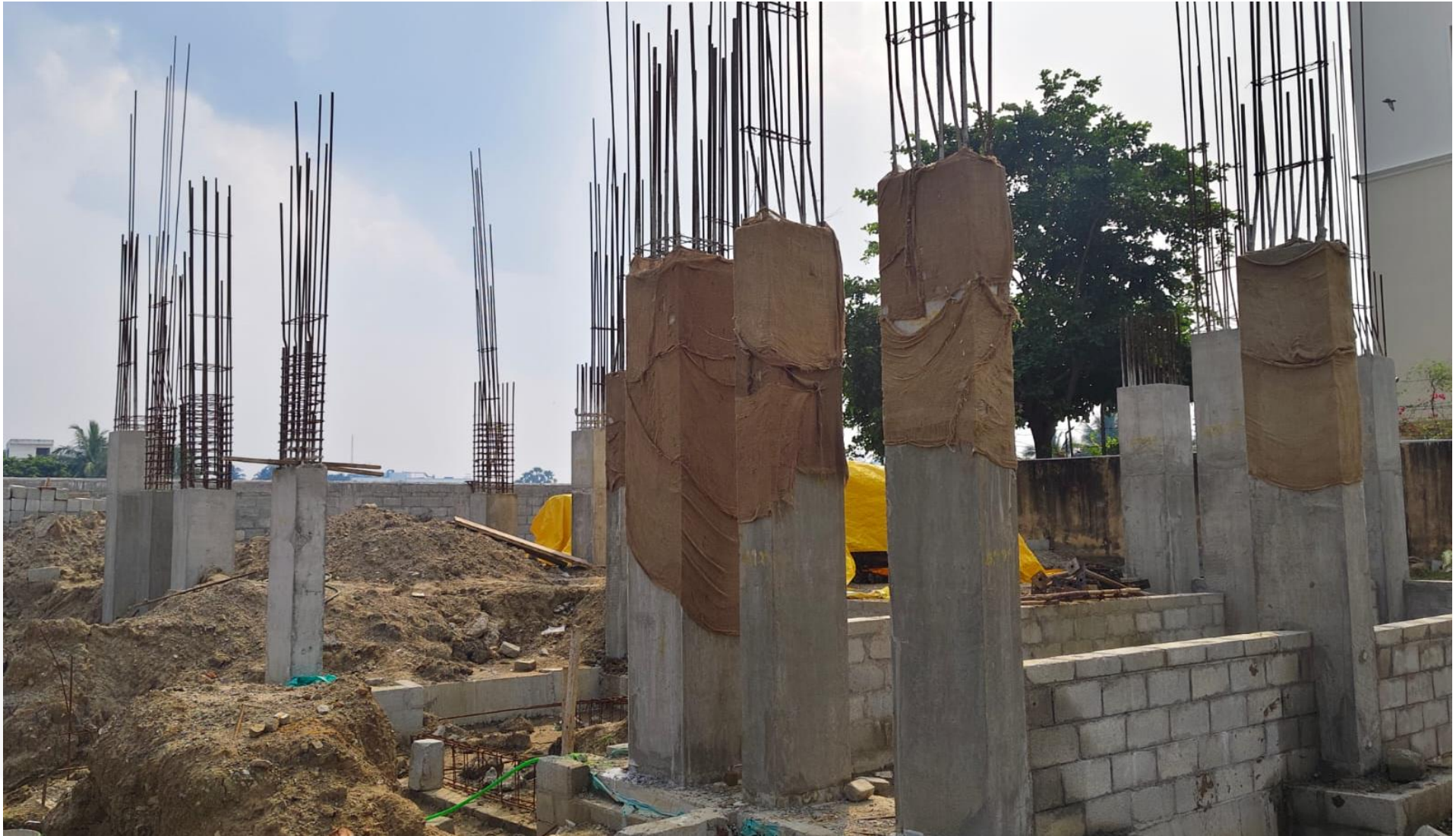
Main Building West Side Column 2 nd Lift Concrete work in progress.
