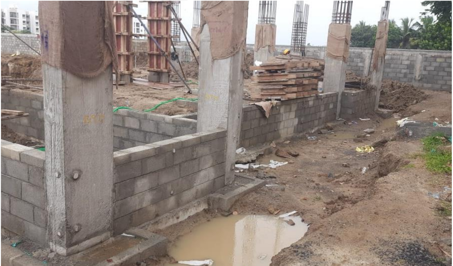
Main Building pile cap to stilt floor Plastering work in progress.
