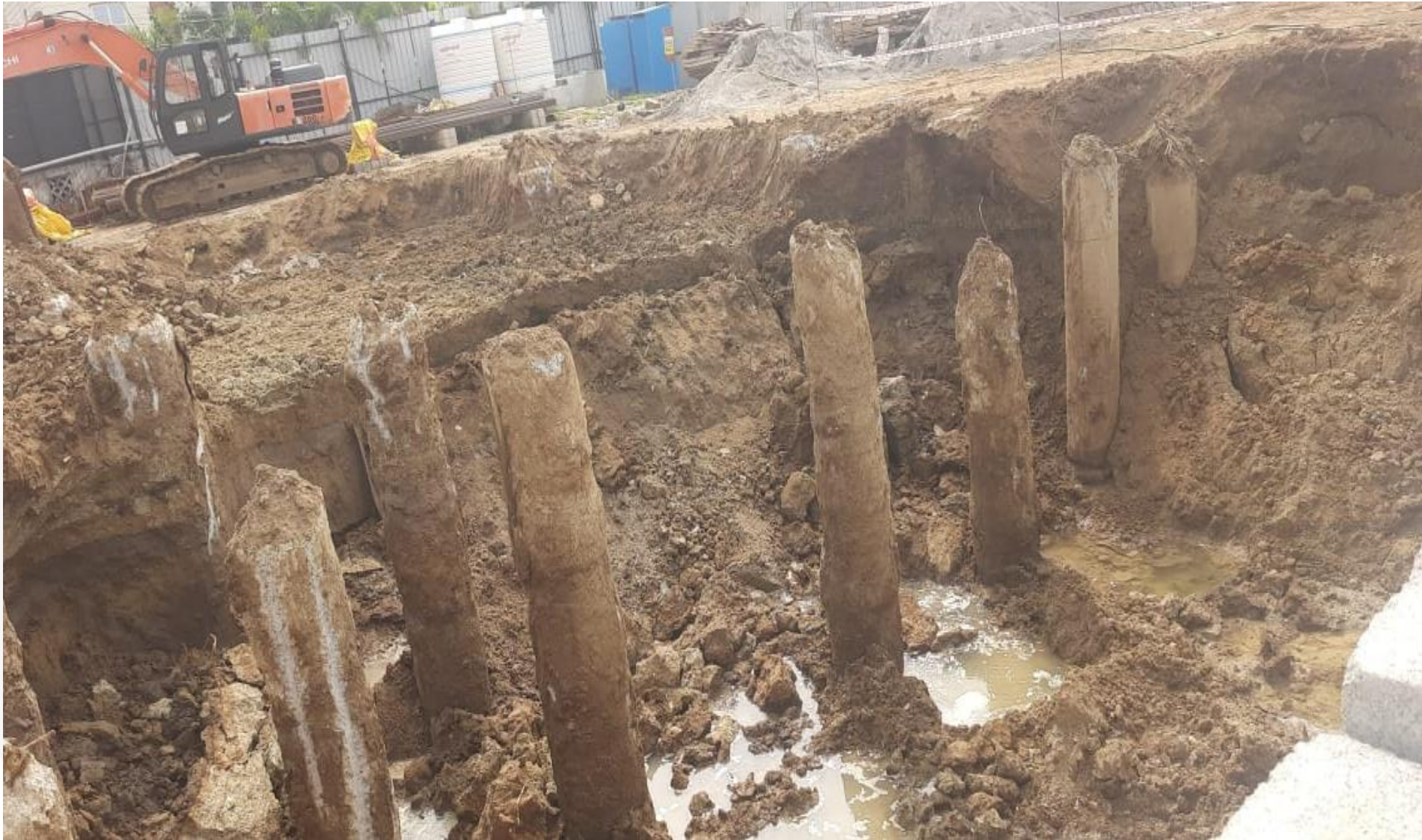
UG Sump Earth Work Excavation Work in Progress.
