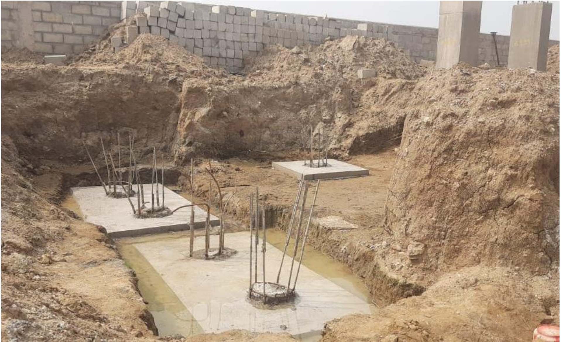
Main Building Pile Cap PCC work in progress.
