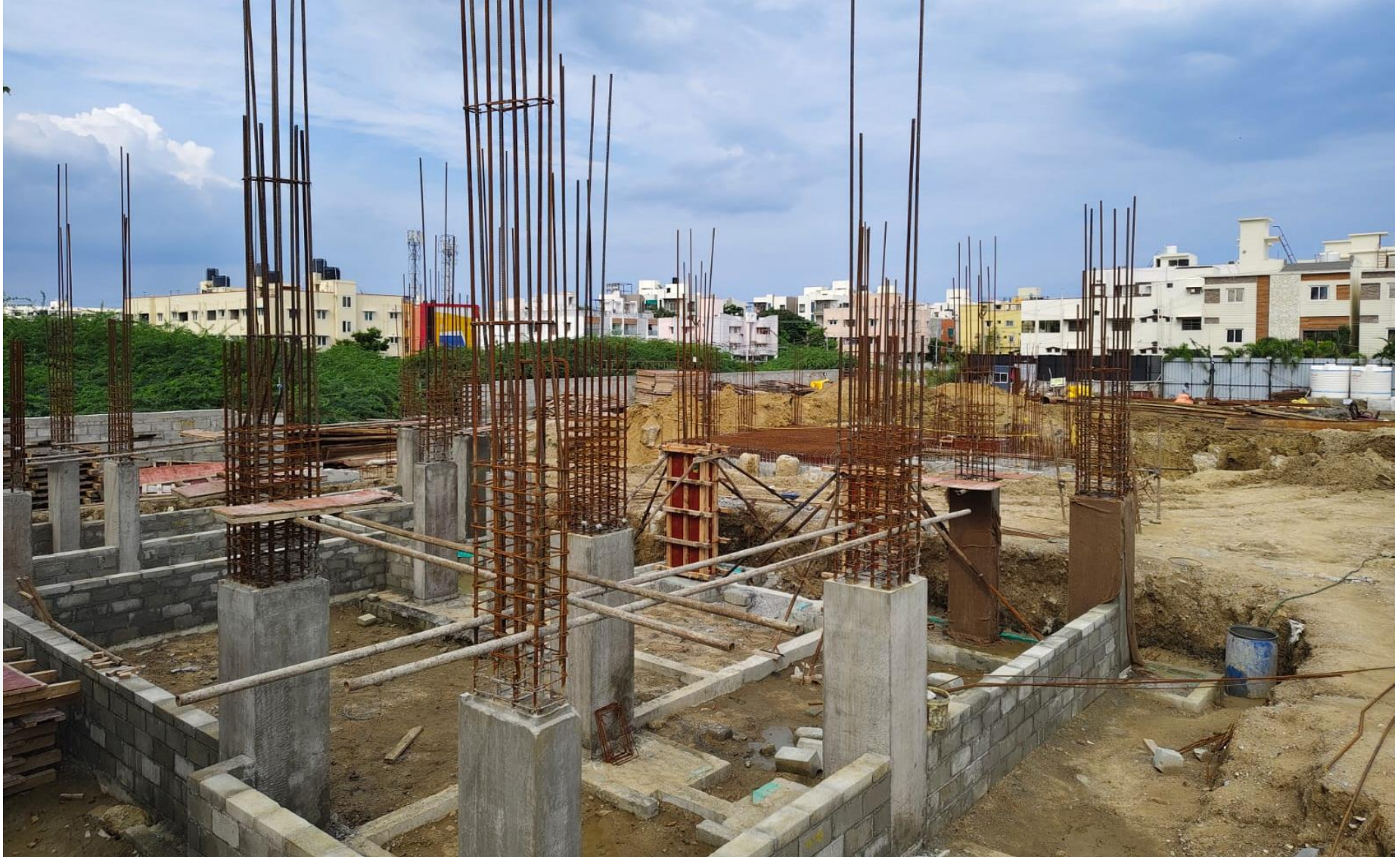
Main Building west side column concrete work in progress.
