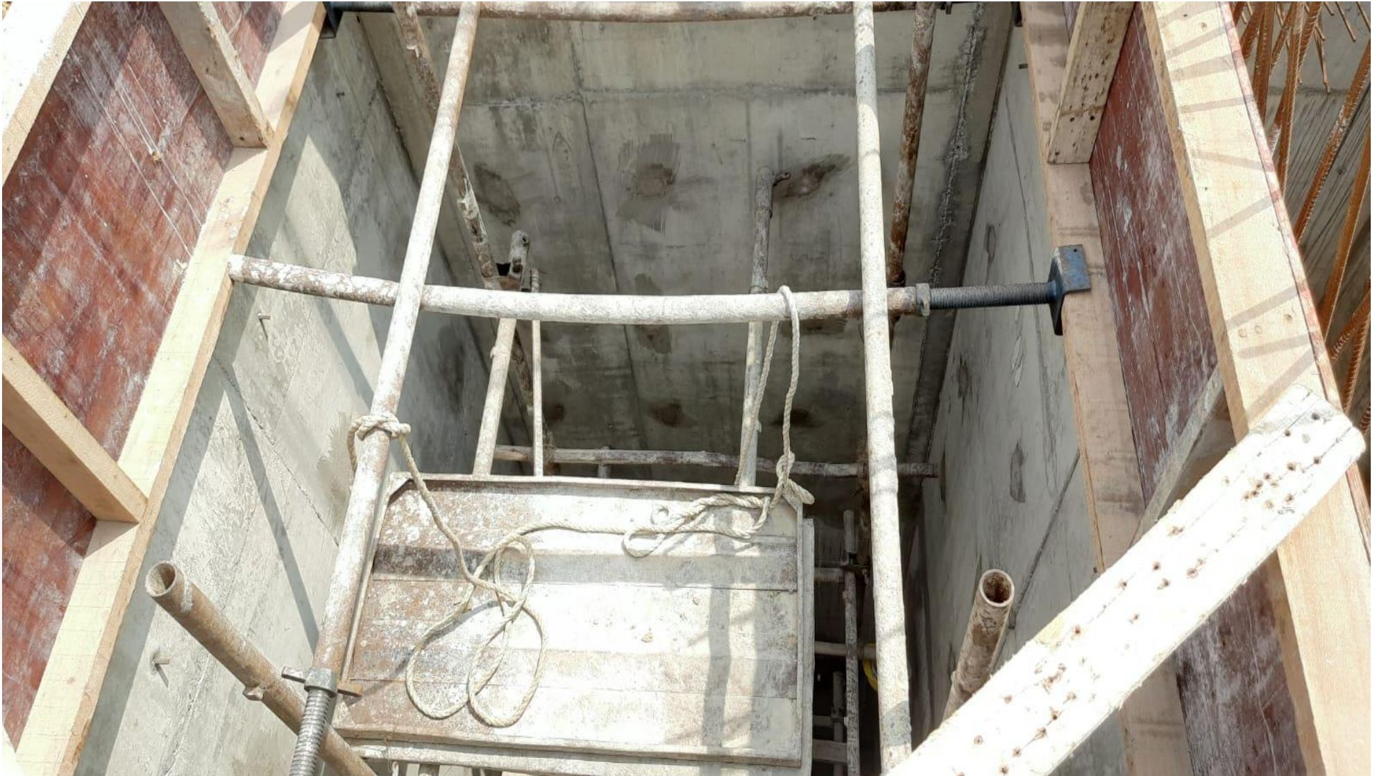
STP Internal Waterproofing Work in progress.
