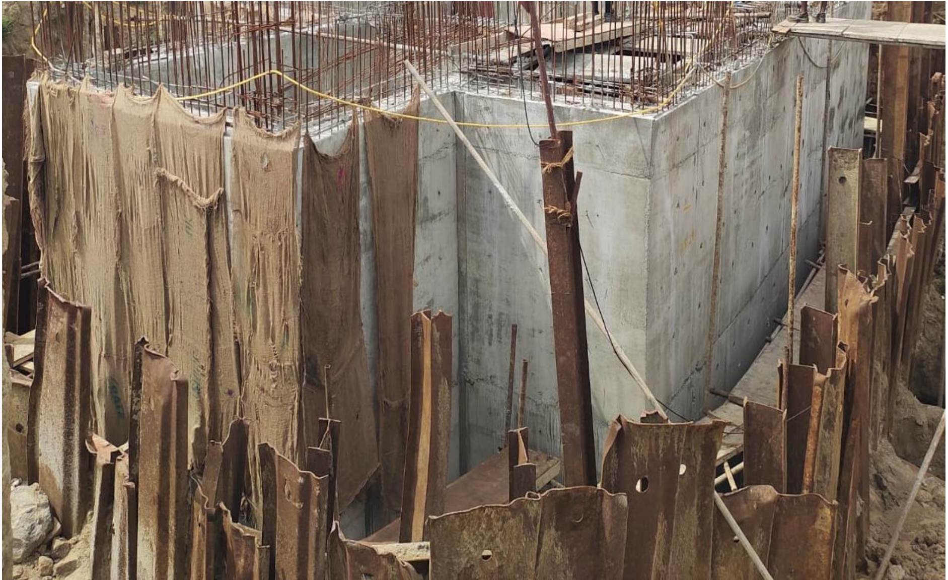
STP 2nd Lift RCC Wall Concrete Work Completed.
