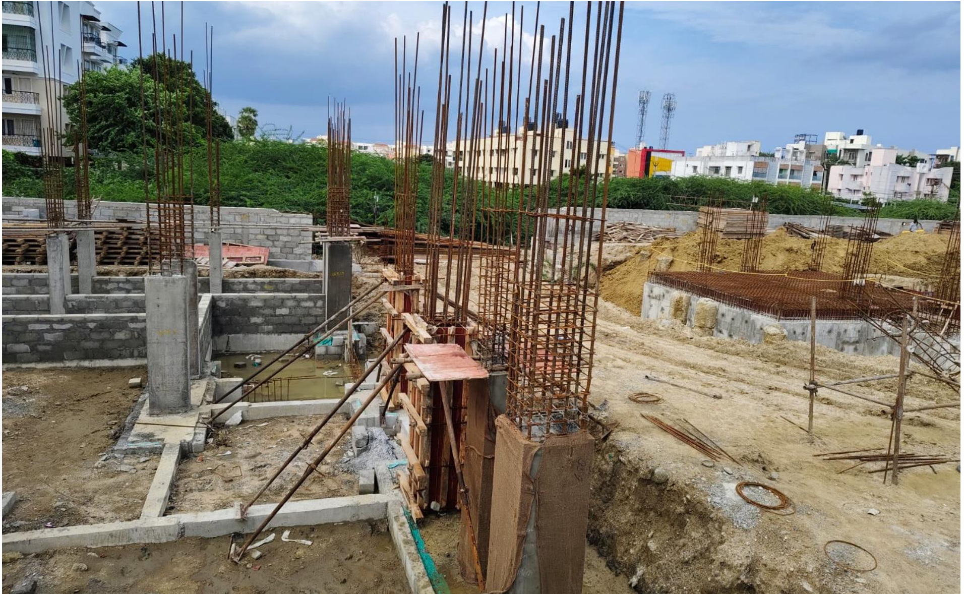
Main Building column reinforcement work in progress.
