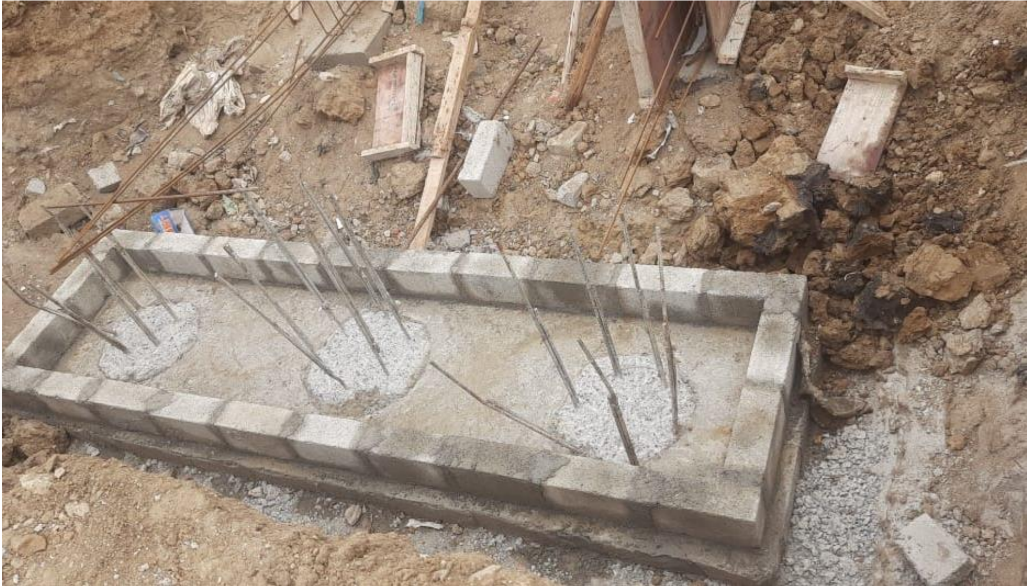
Main Building Pile Cap 2 nd pour PCC work Completed.
