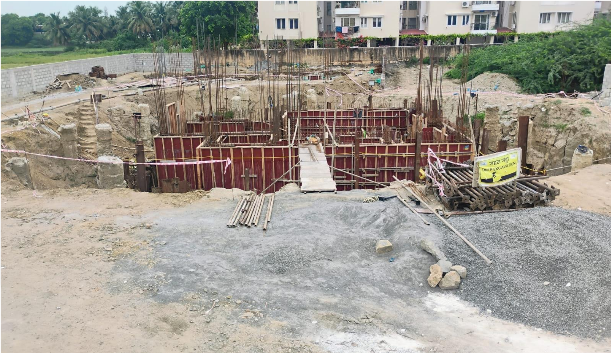
Overall Site view.
