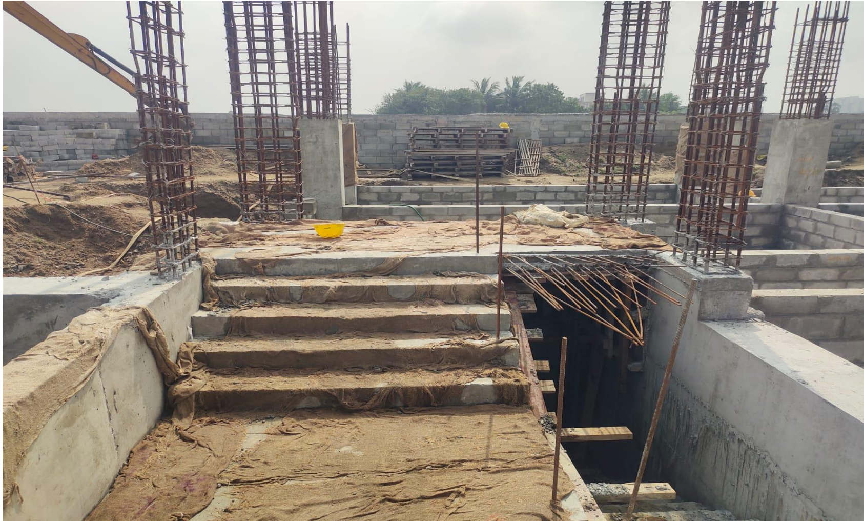
STP – Staircase Concrete Work Completed.
