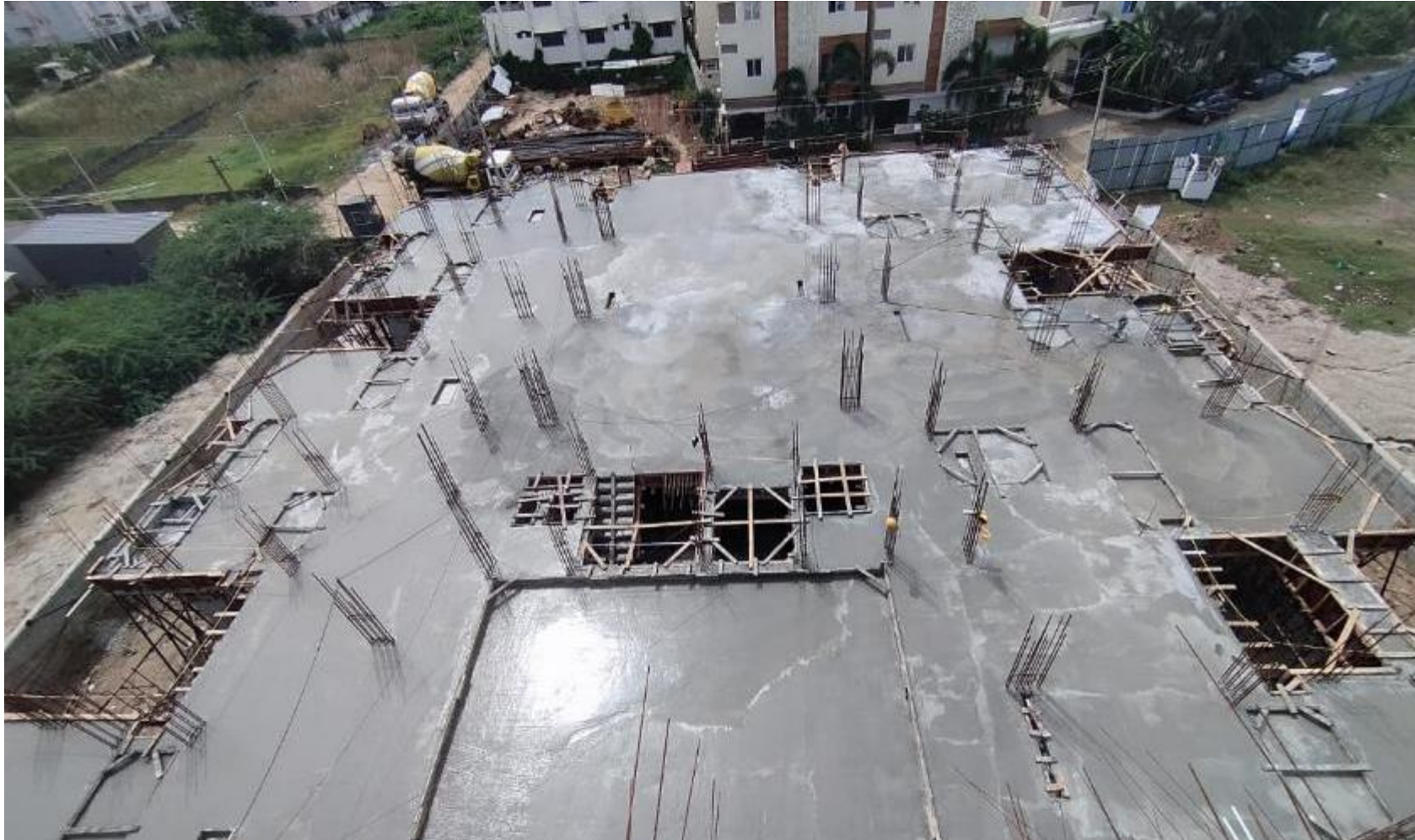
Main Building Pour-2 Stilt Floor Roof Slab Concrete Work Completed.
