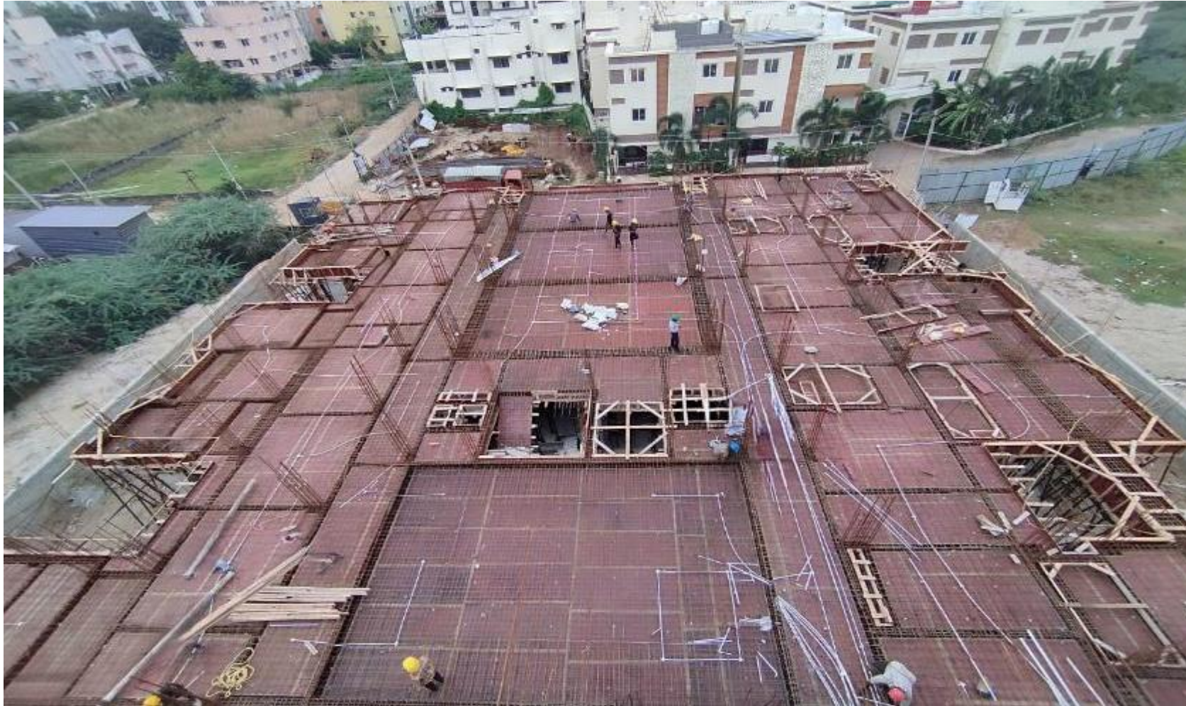
Main Building Pour-2 Stilt Floor Roof Slab Reinforcement Work Completed.
