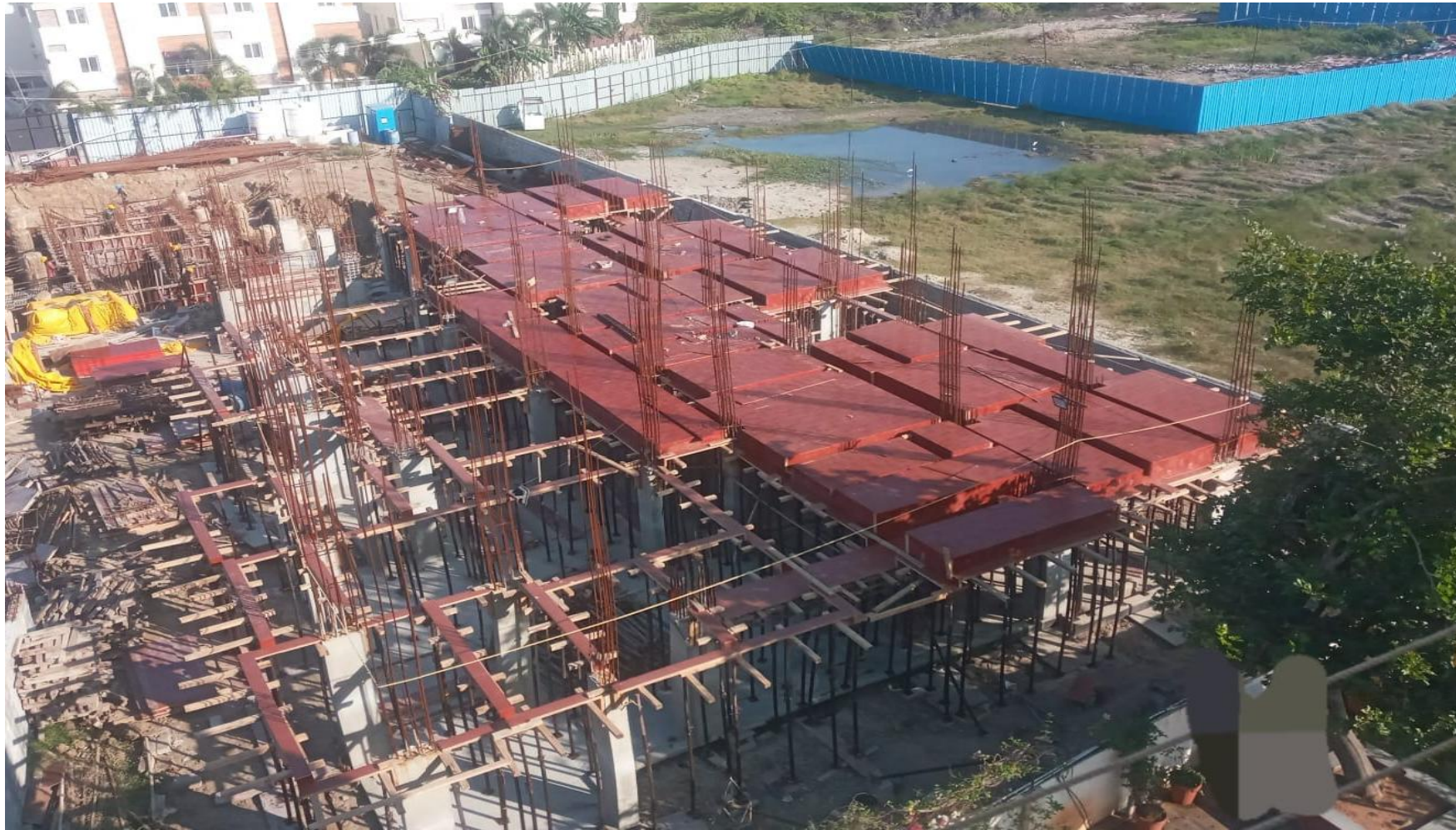
Main Building Stilt Floor Pour-1 Roof Slab Shuttering Work Nearing Completion.
