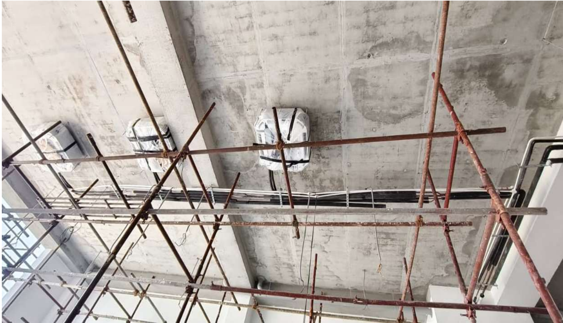
Multipurpose Hall AC Fixing Work Completed.
