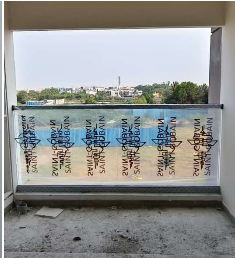
Main Building Balcony Handrail Fixing Work Nearing Completion.
