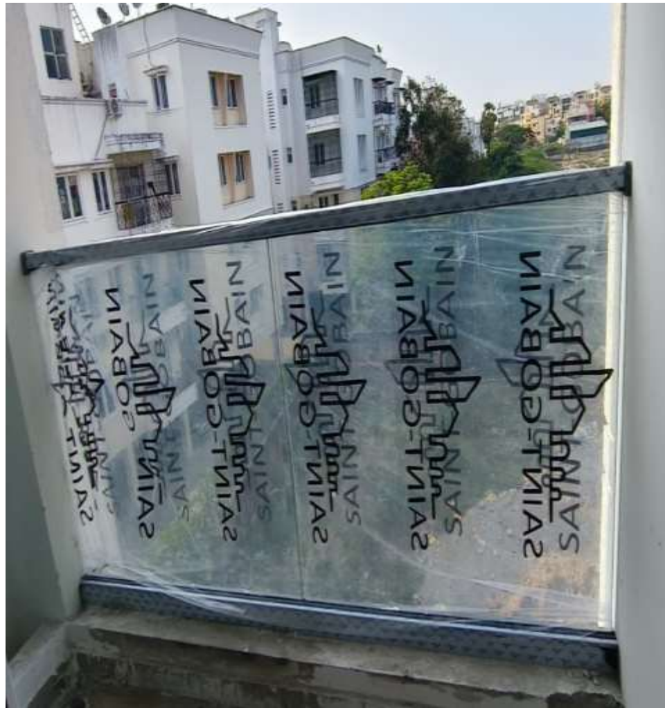
Main Building Balcony Handrail Fixing Work Nearing Completion.
