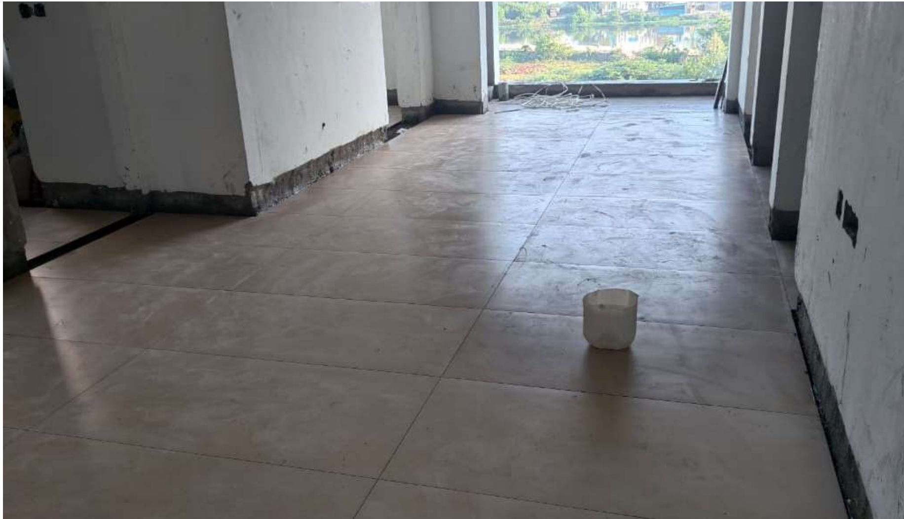
Main Building Pour-2 5 th floor Tiles Work Completed.
