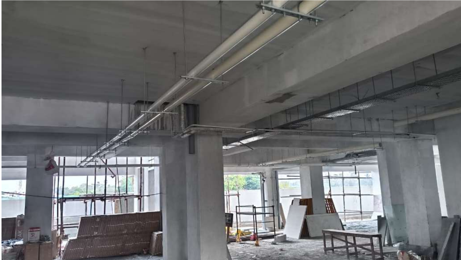
Main Building Pour-2 Stilt Floor Plumbing Work Nearing Completion.
