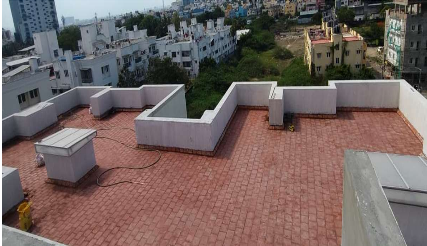
Main Building Terrace Press Tiles Work Nearing Completion.
