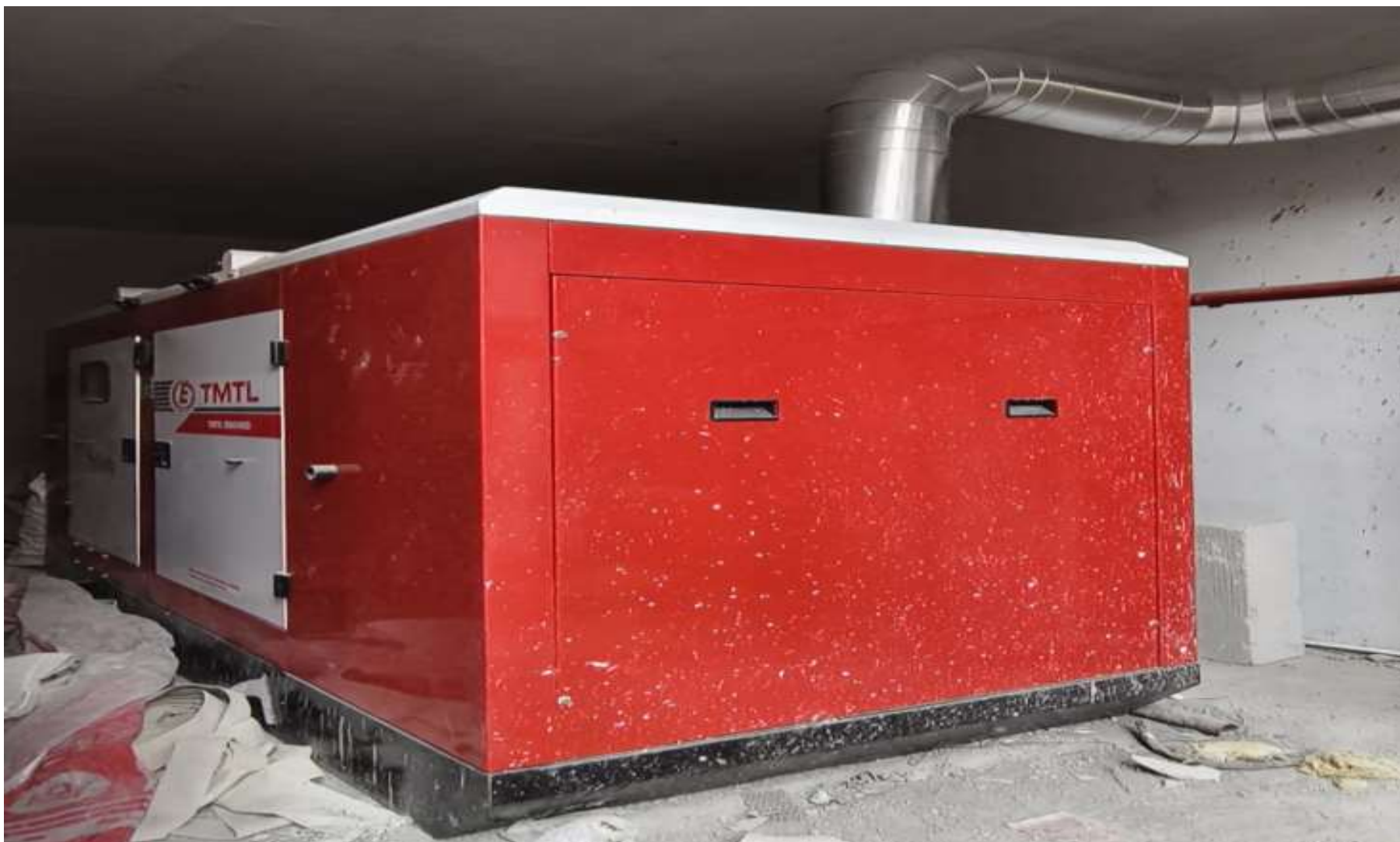
DG Exhaust Pipe Fixing Work Completed.
