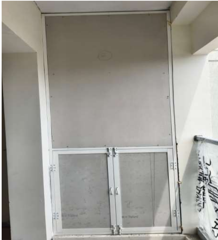
Main Building Balcony Plumbing Shaft Shera Door Fixing Work In Progress.
