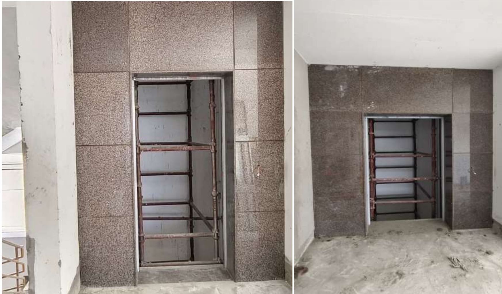
Main Building Pour-1 Lift Granite Wall Glazing Work Nearing Completion.
