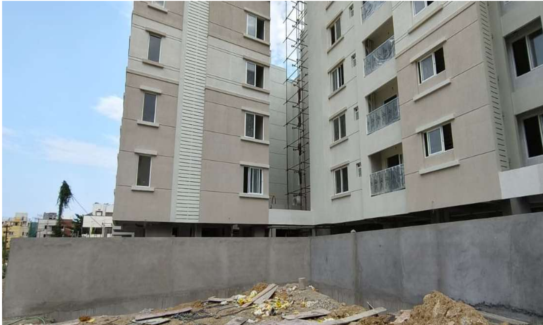
Compound Wall External Plastering Work Nearing Completion.
