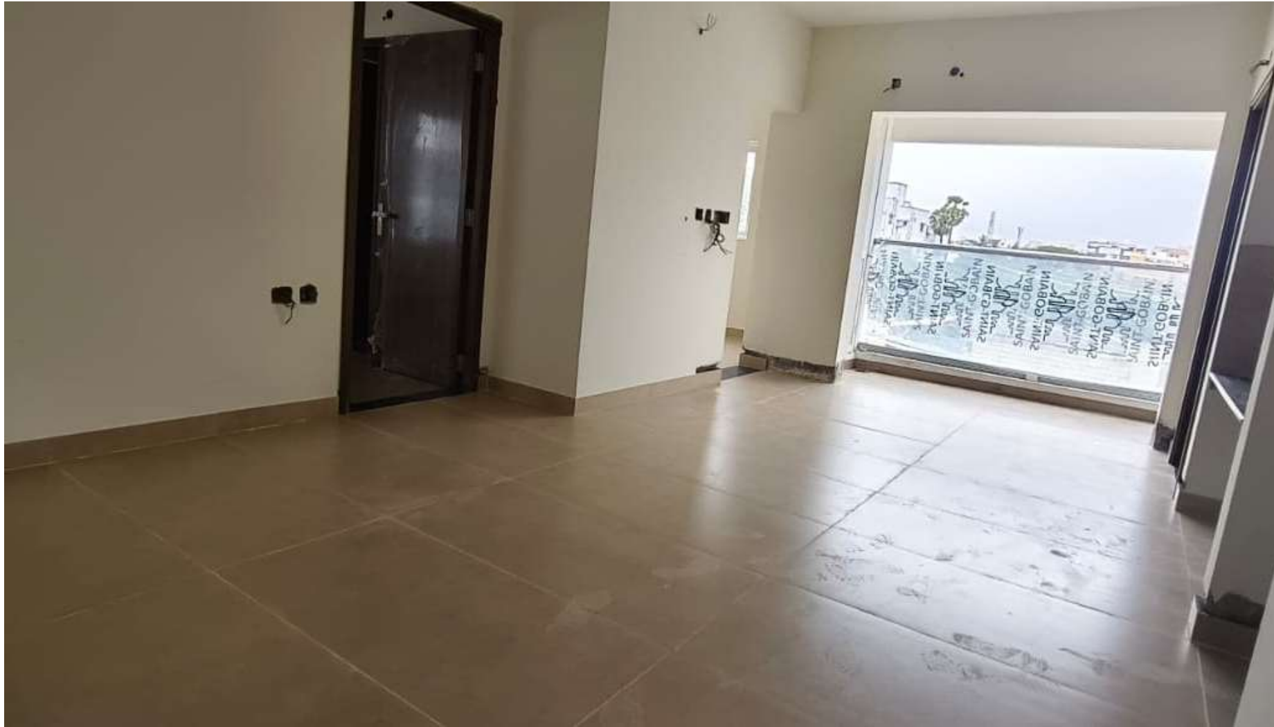
Main Building Pour-2 1 st floor Tiles Acid Wash Work In Progress.
