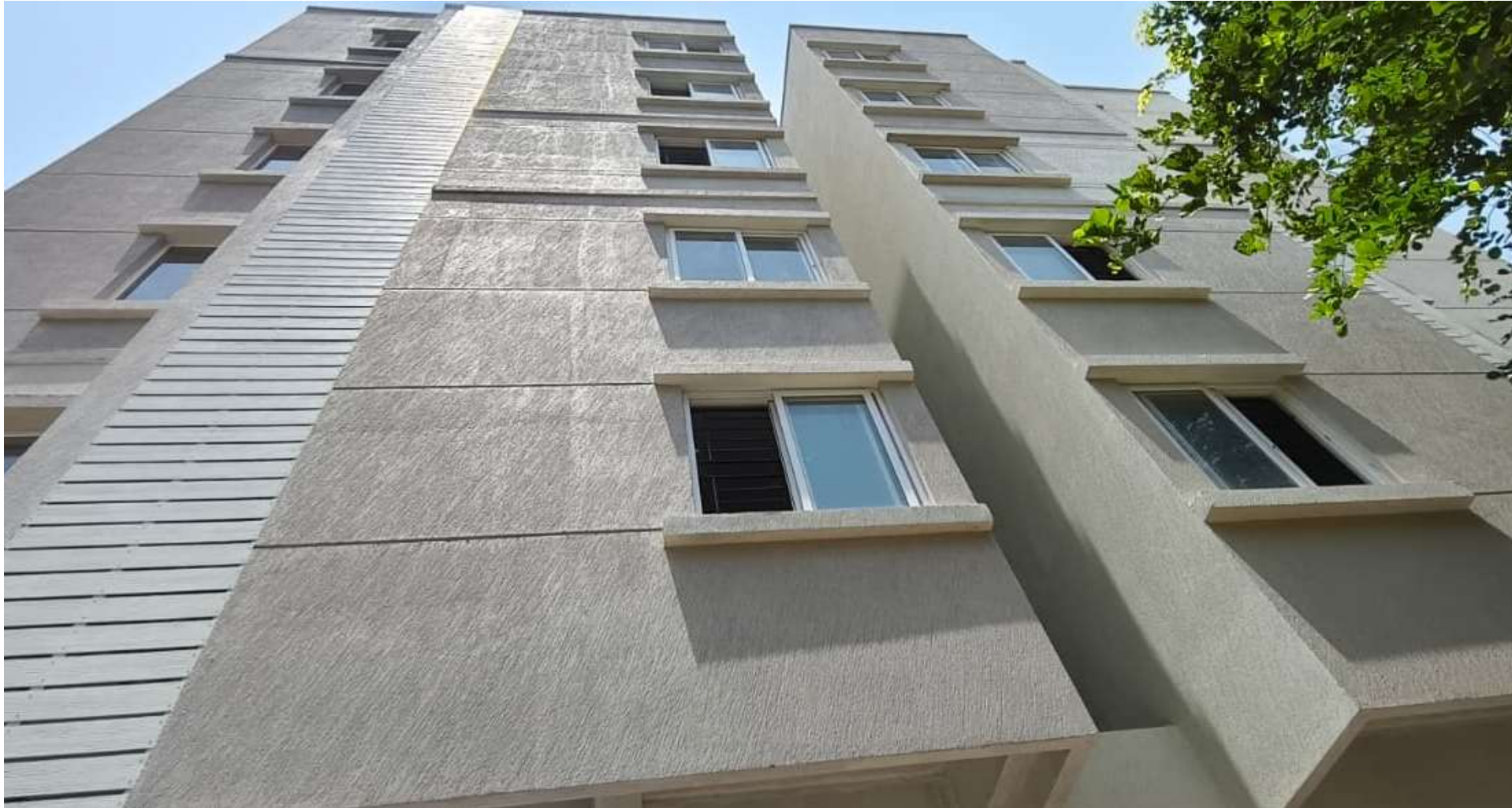
Main Building West Side External Texture Painting 1 st Coat Work Completed.
