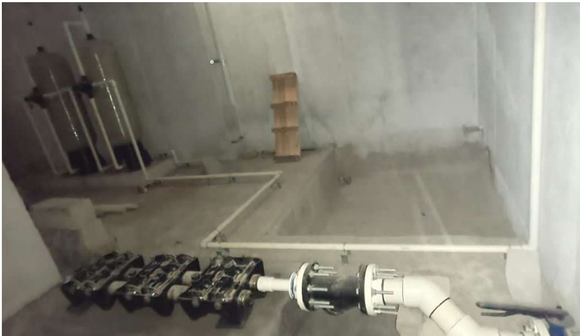
UG Sump Pump and Filter Fixing Work In Progress.
