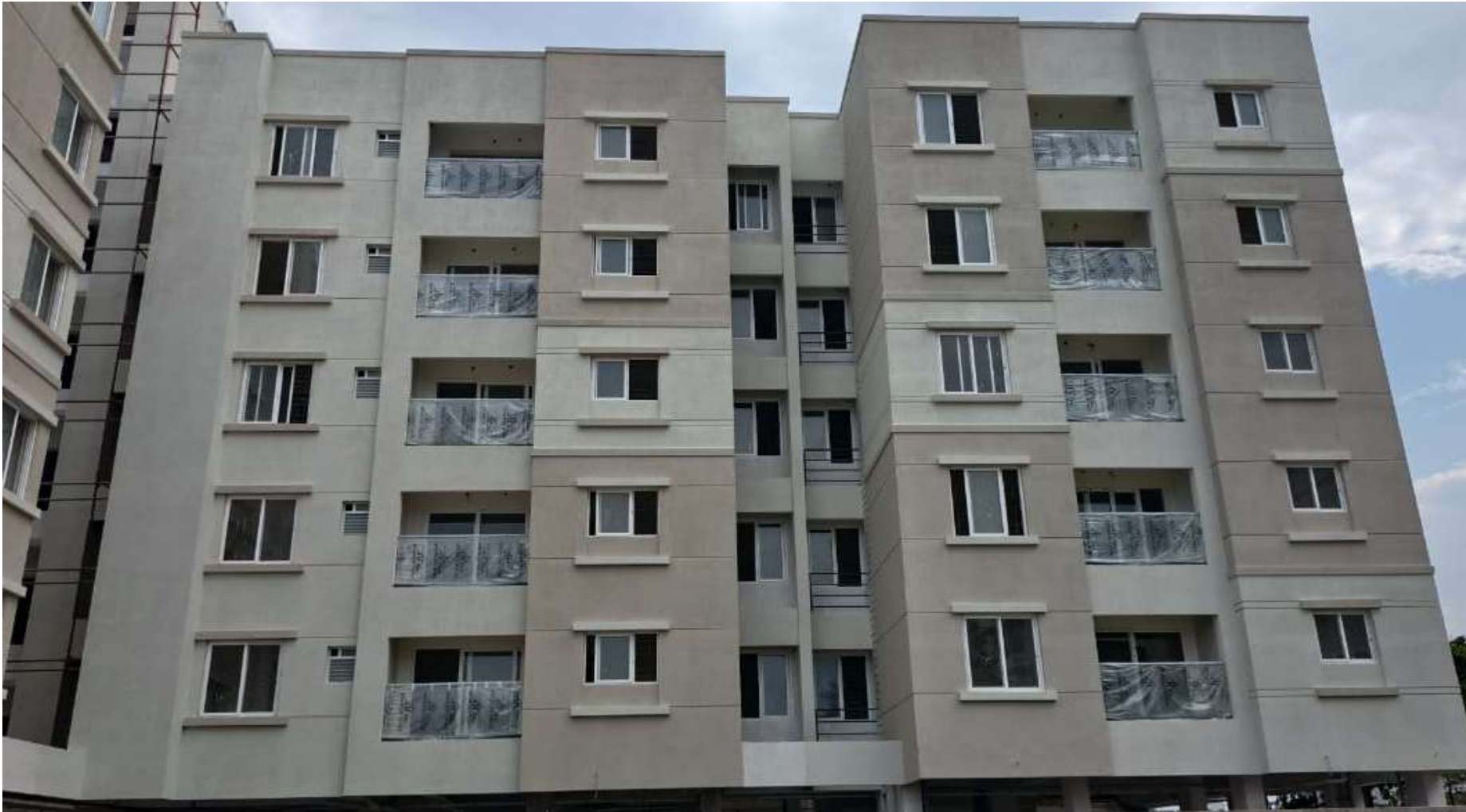
Main Building North Side External Texture Painting 1 st Coat Work Completed.
