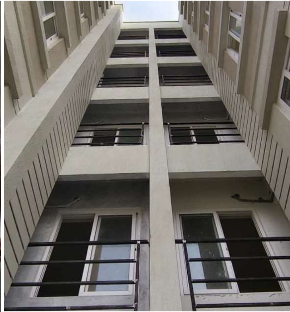
Main Building Plumbing Shaft Shera Plank Covering Work Nearing Completion.
