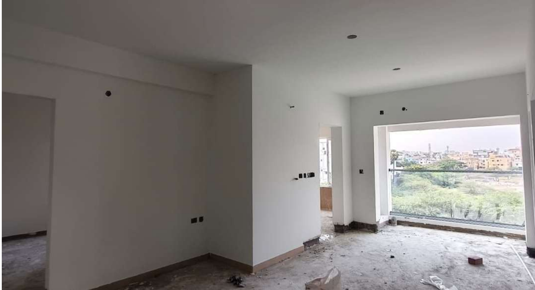
Main Building Pour-2 4 th Floor Putty Work Completed.
