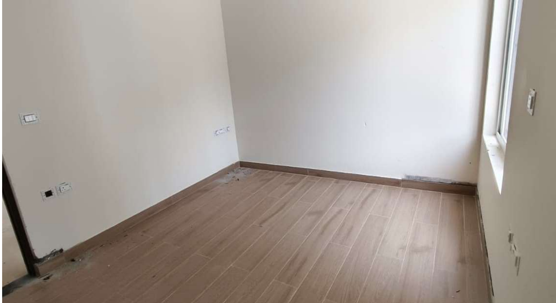
Main Building 1 st Floor Electrical Switch Plate Fixing Work In Progress.
