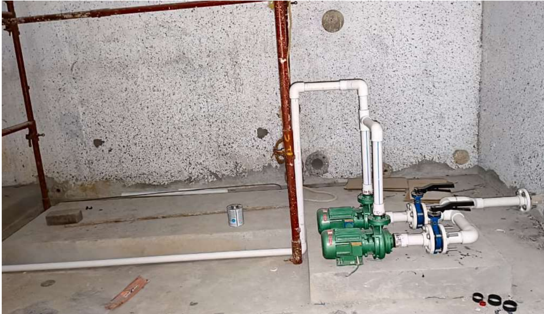
STP Pump and Filter Fixing Work In Progress.
