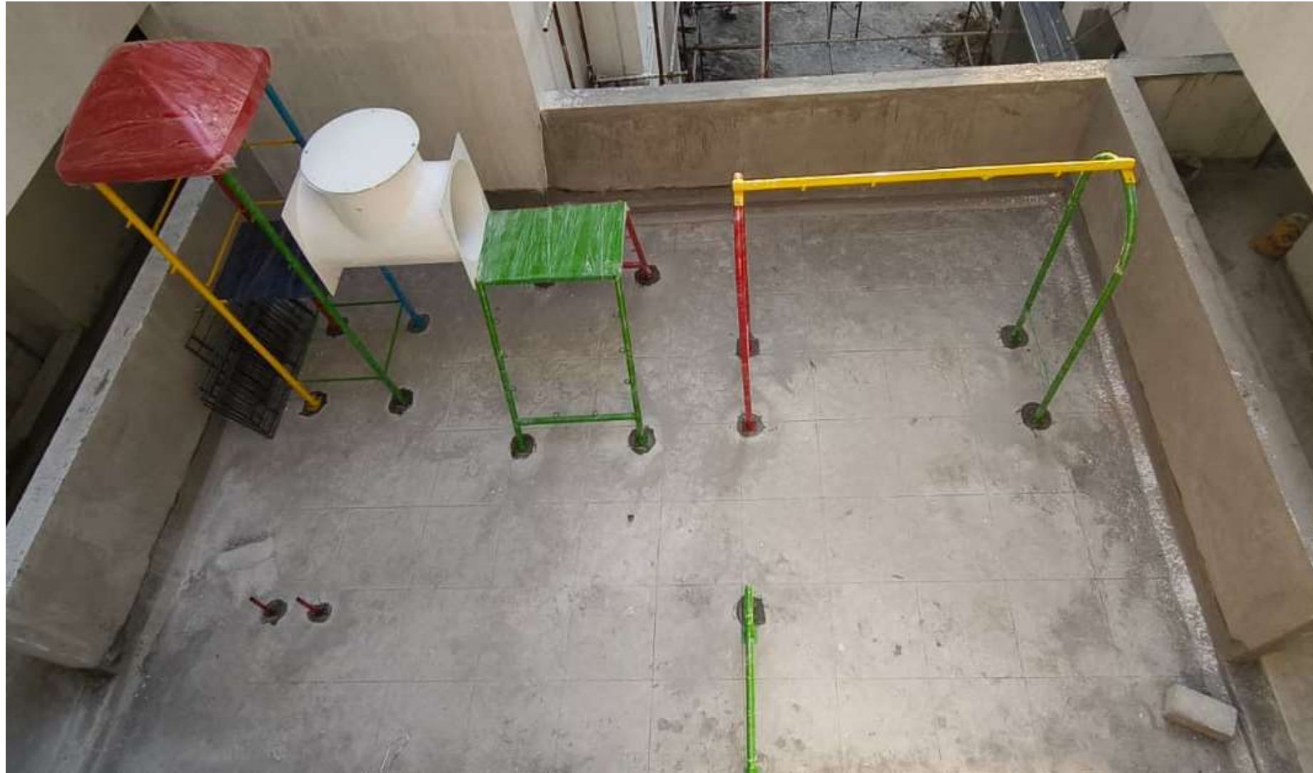
Kids Play Equipment's Fixing Work In Progress.
