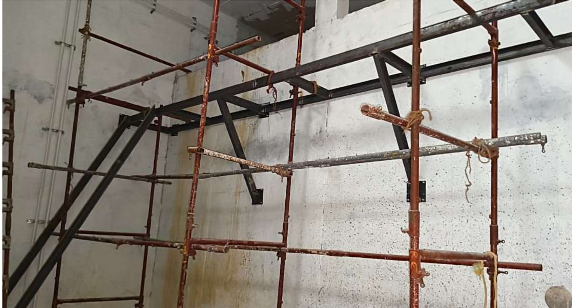
STP Pump Room Walkway Platform Channel Fixing Work In Progress.
