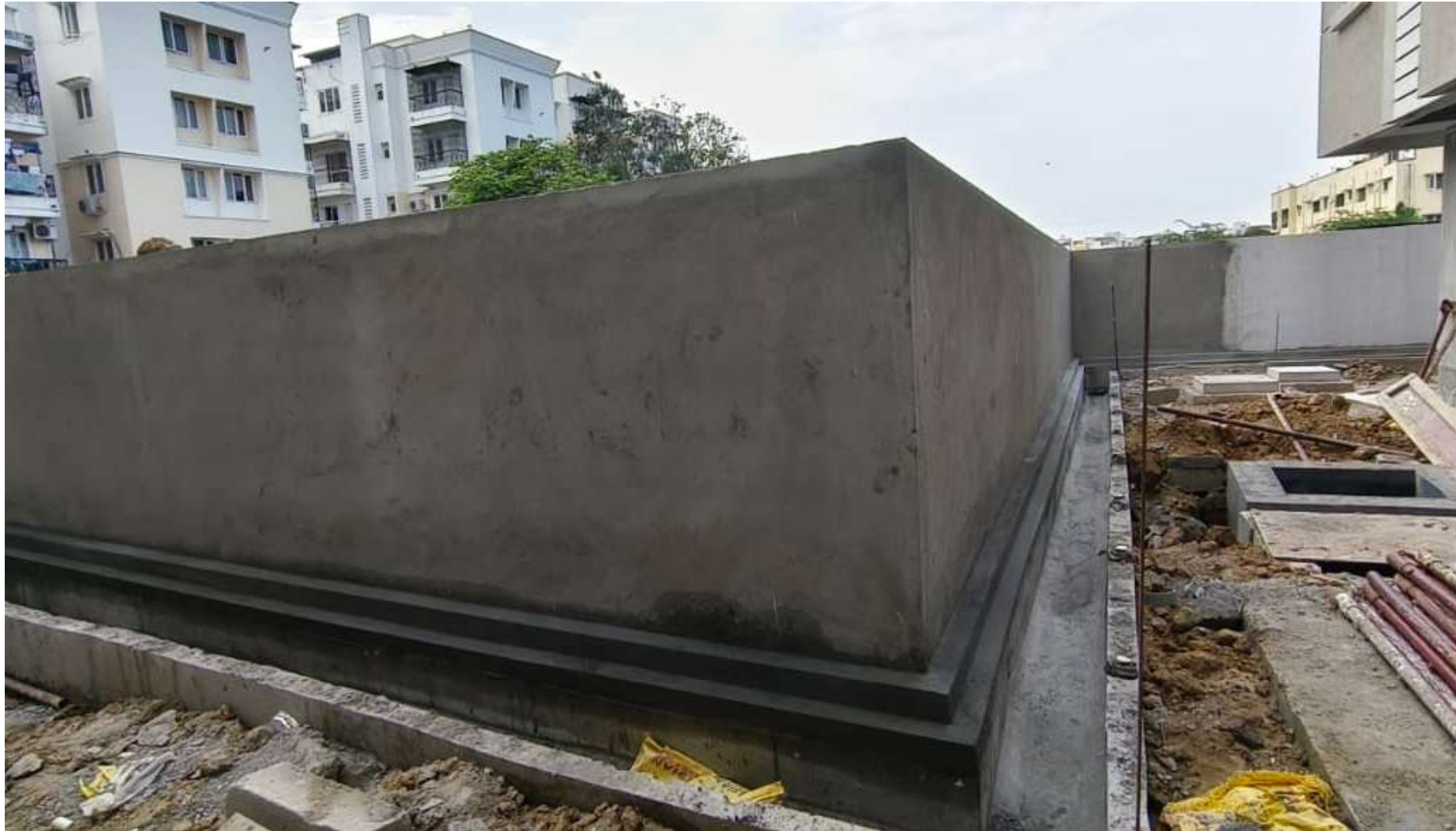
Storm Water Drain Top Finishing Work Nearing Completion.
