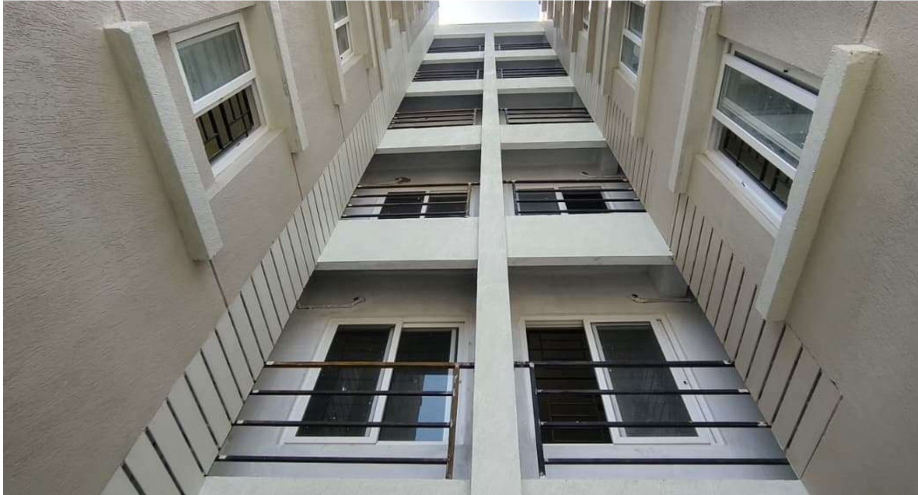
Main Building AC Outdoor Handrail Fixing Work Nearing Completion.
