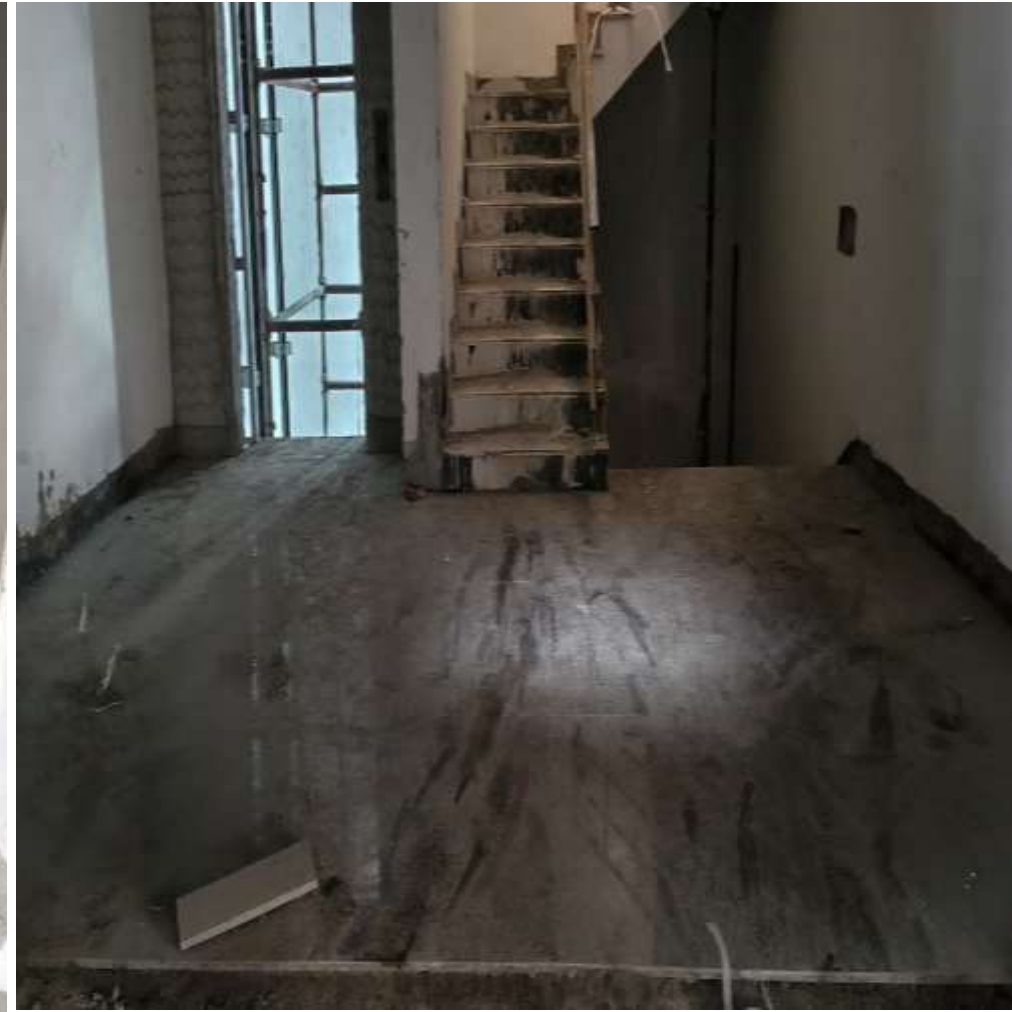
Main Building Stilt Floor Granite Lobby Flooring Work Nearing Completion.
