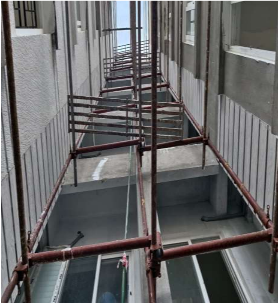
Main Building Plumbing Shaft Shera Plank Covering Work Nearing Completion.
