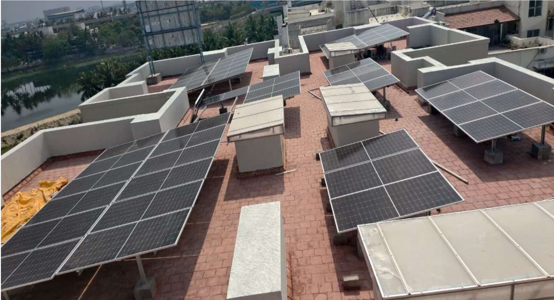
Main Building Terrace Solar Pannel Fixing Work Nearing Completion.
