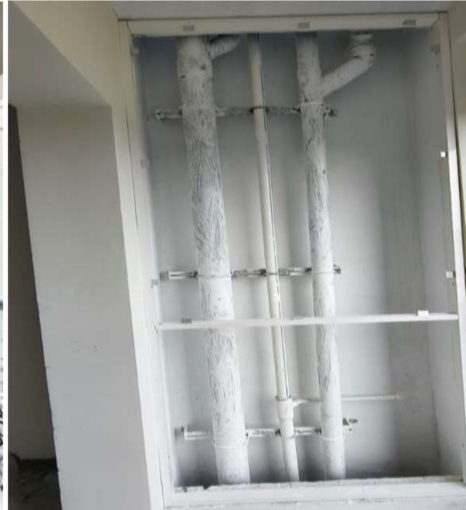
Main Building Balcony Plumbing Shaft Shera Door Fixing Work In Progress.
