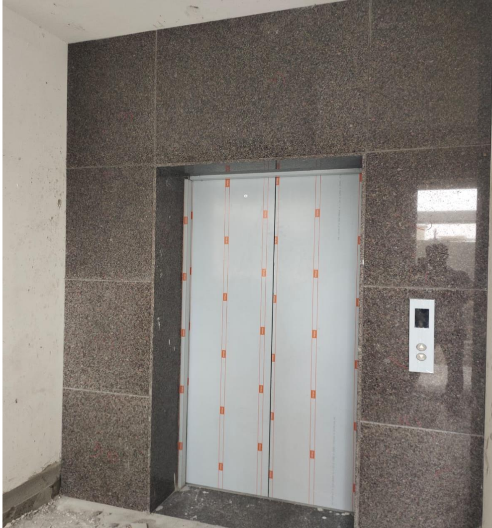
Main Building Lift Granite Wall Cladding Work Completed.
