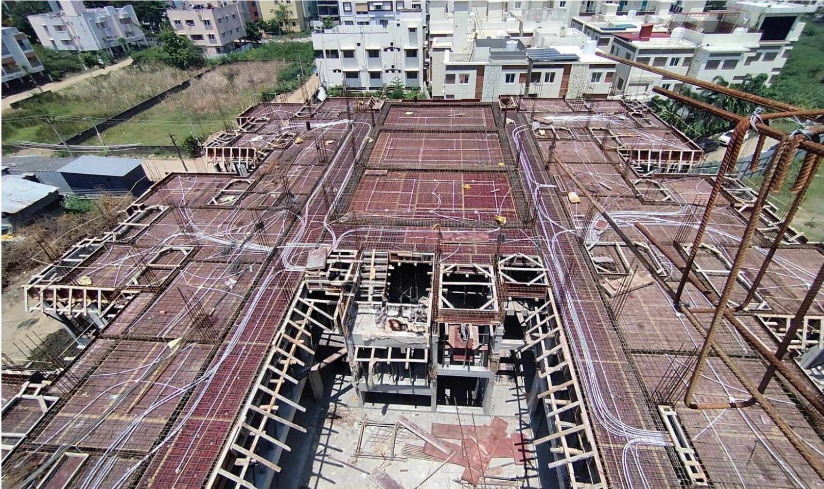
Main Building Pour-2 2 nd Floor Roof Slab Shuttering Work Completed.
