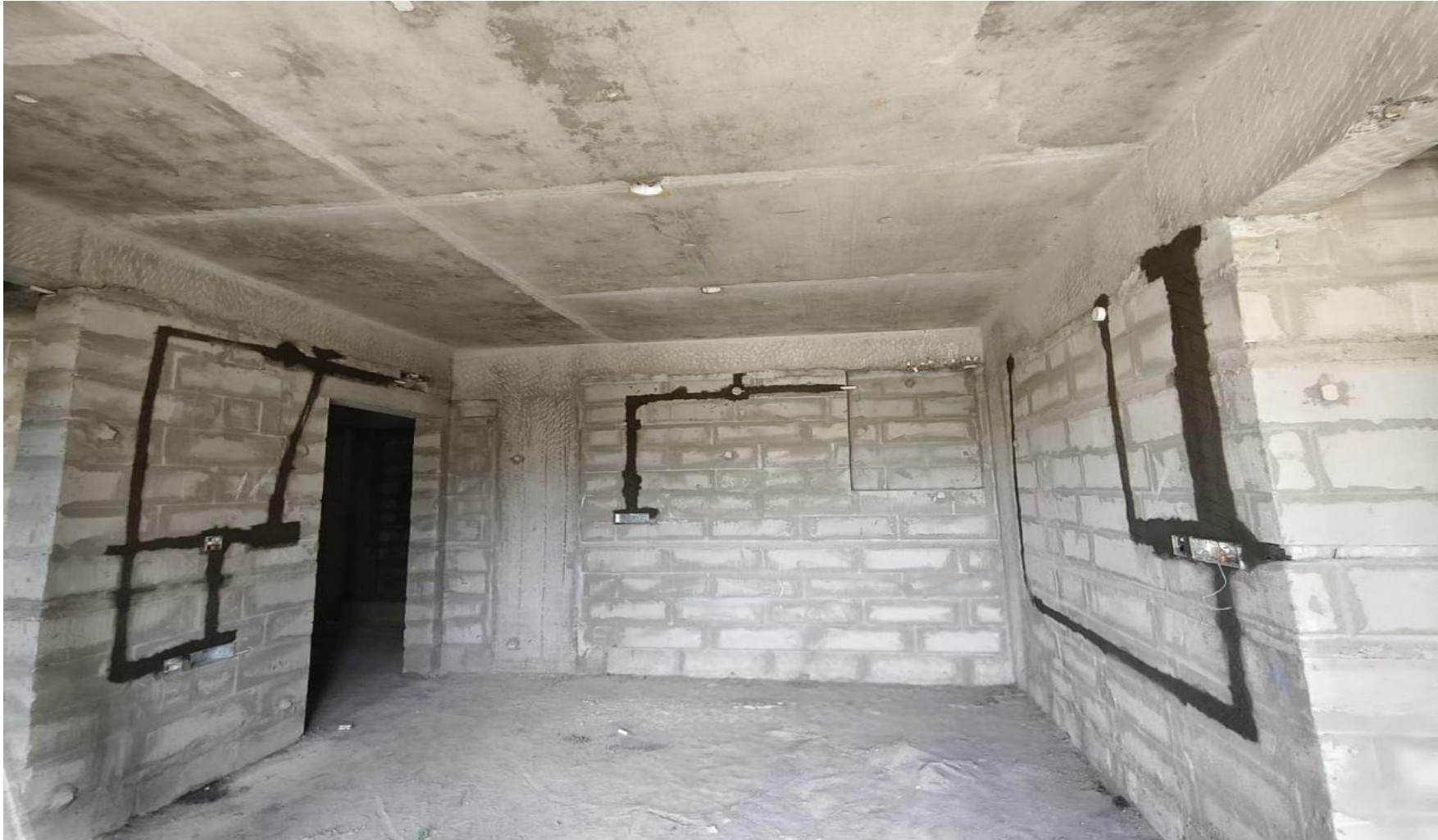
Main Building Pour-1 2 nd Floor Electrical Box Fixing and Pipe Laying Work Completed.
