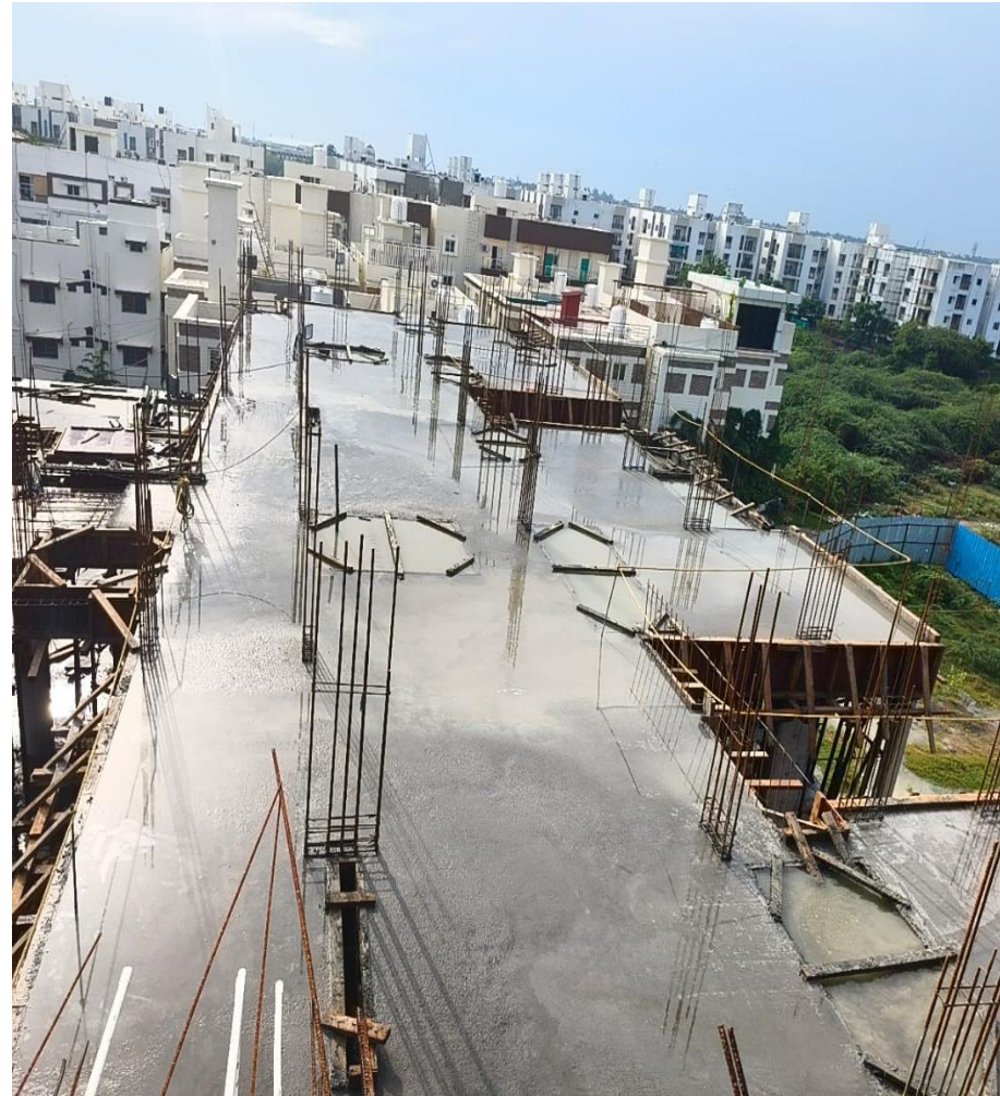
Main Building Pour-2 3 rd Floor Roof Slab Concrete Work Completed.
