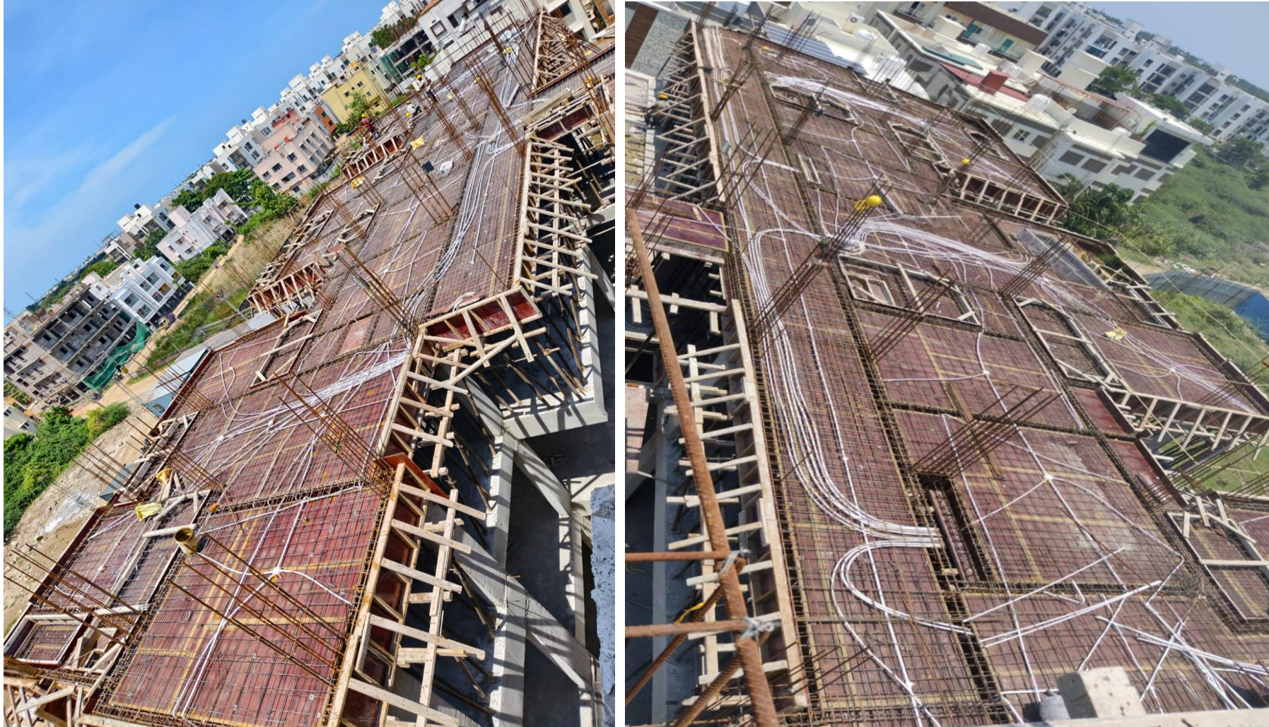
Main Building Pour-2 3 rd Floor Roof Slab Shuttering Work Completed.
