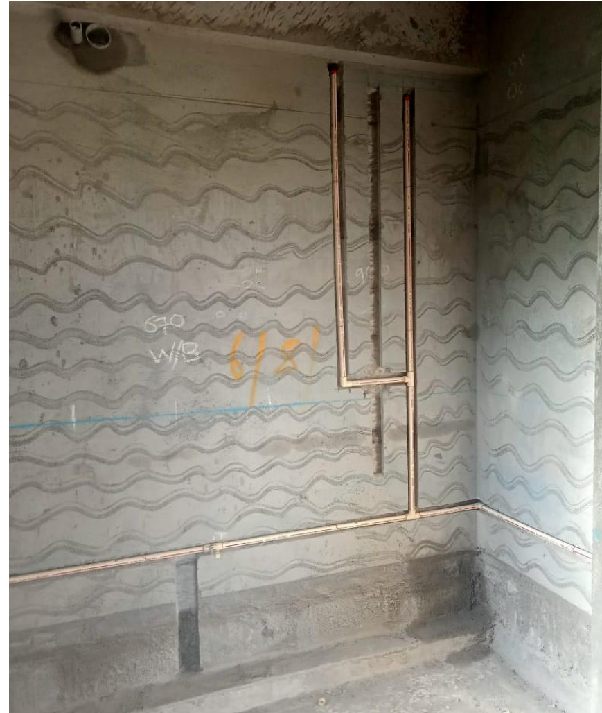
Main Building Pour-1 1 st Floor Plumbing Toilet Concealed pipe Line Work In Progress.
