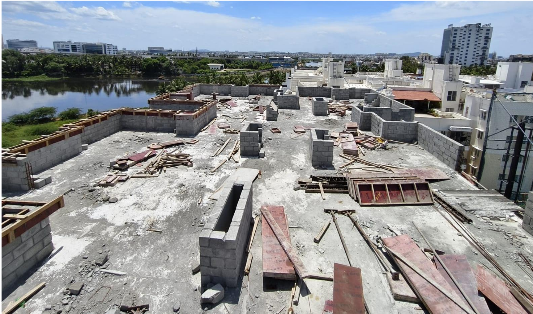
Main Building Pour-1 Terrace Floor Parapet Wall Blockwork Work Completed.
