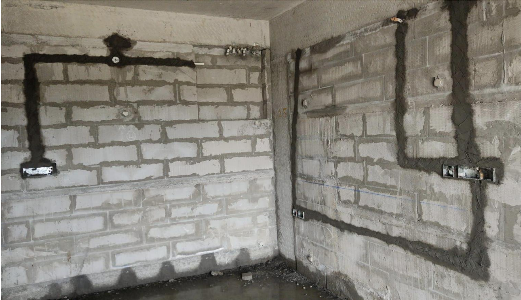
Main Building Pour-1 1 st Floor Electrical Box Fixing and Pipe Laying Work Completed.
