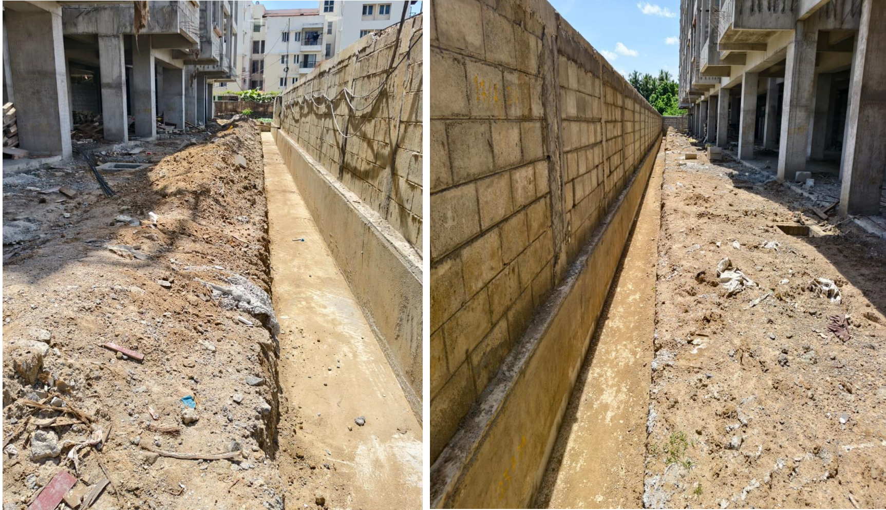
Main Building External Storm Water Drain PCC Work Nearing completion.
