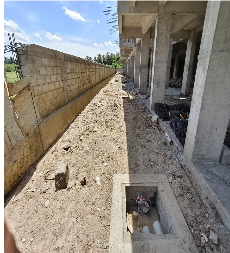
Main Building Stilt Floor Manhole Blockwork and plastering Work Nearing completion.
