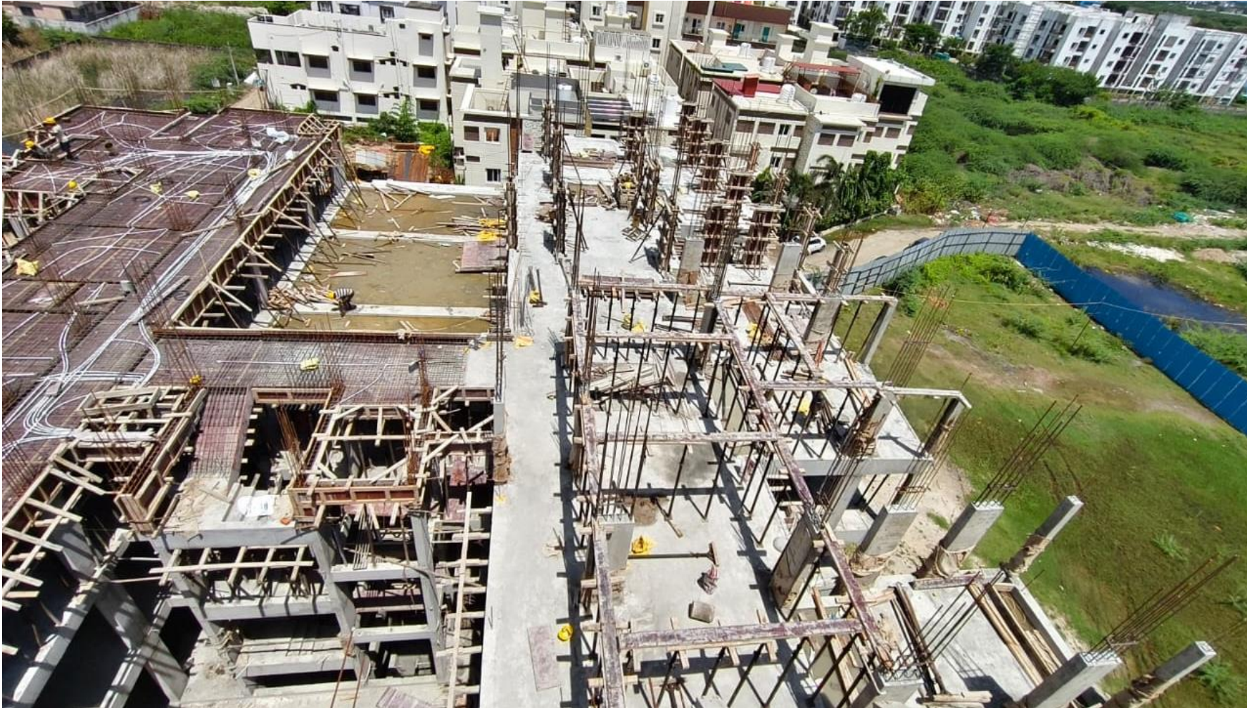
Main Building Pour-2 4 th Floor Roof Slab Shuttering Work Commenced.
