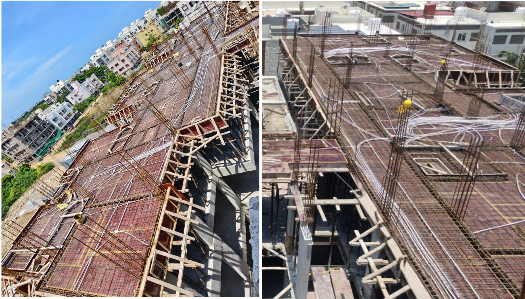
Main Building Pour-2 3 rd Floor Roof Slab Reinforcement Work Completed.
