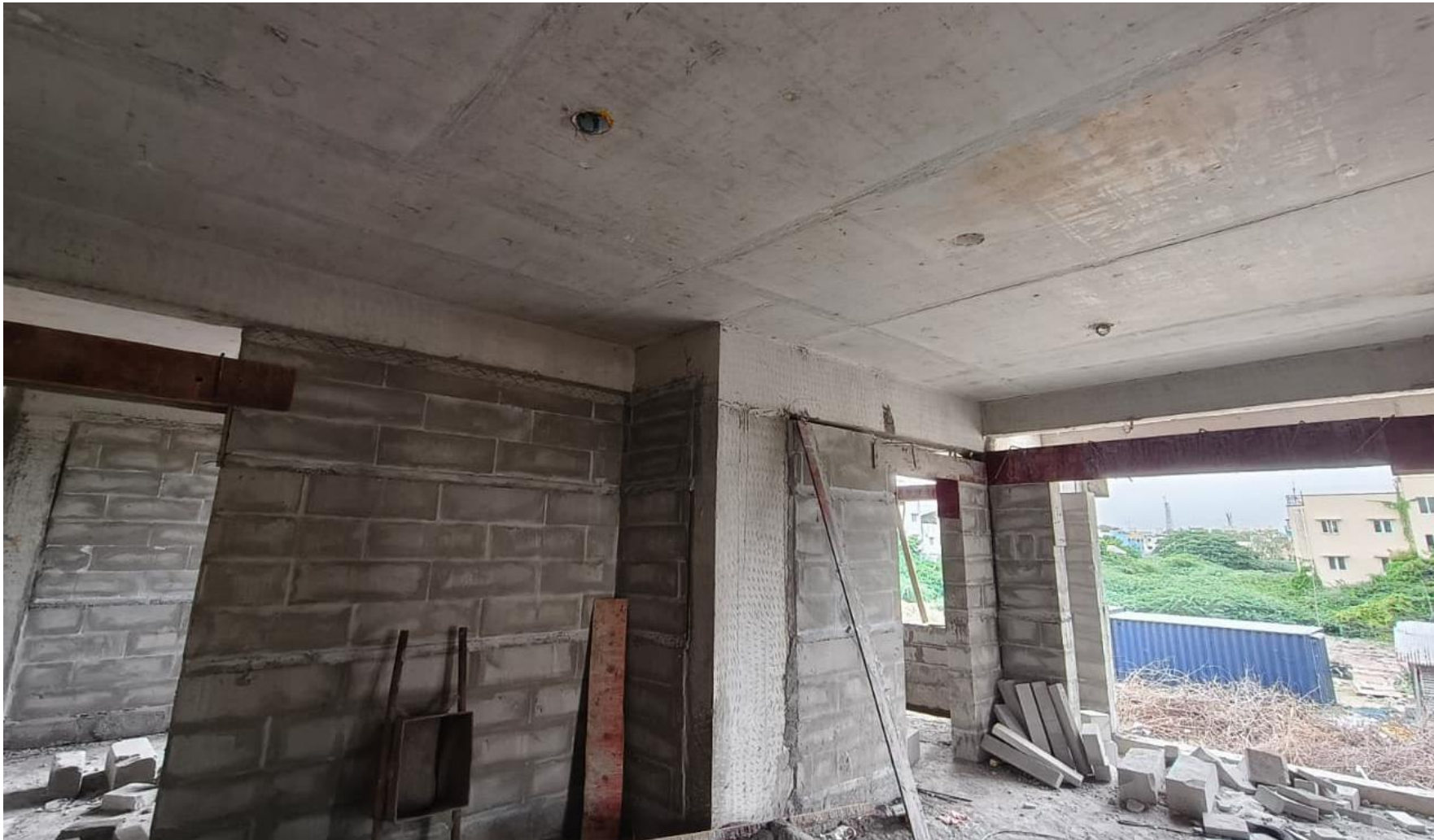
Main Building Pour-2 1 st Floor Blockwork Work In Progress.
