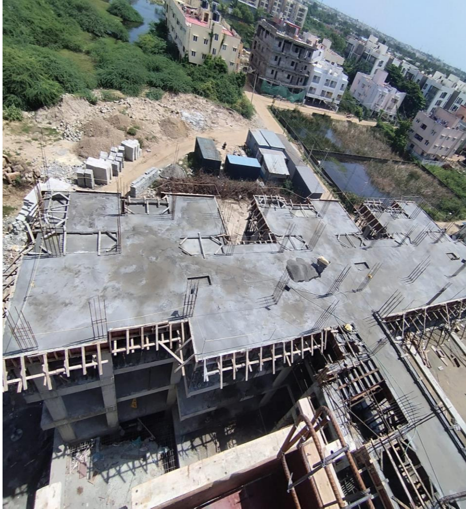
Main Building Pour-2 3 rd Floor Roof Slab Concrete Work Completed.
