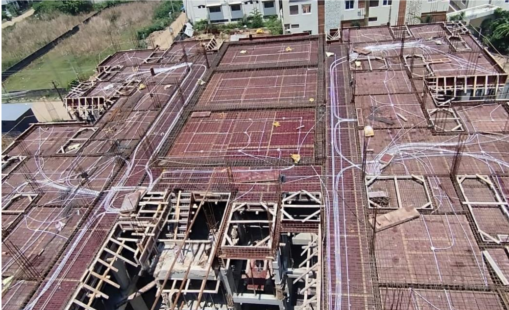
Main Building Pour-2 2 nd Floor Roof Slab Reinforcement Work Completed.
