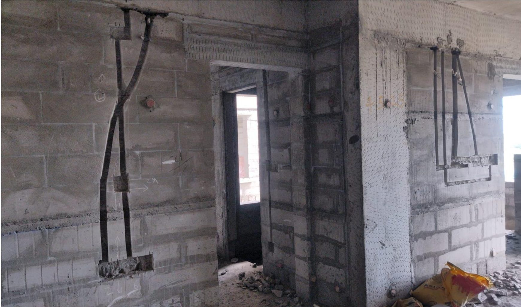
Main Building Pour-1 3 rd Floor Electrical Box Fixing and Pipe Laying Work In Progress.
