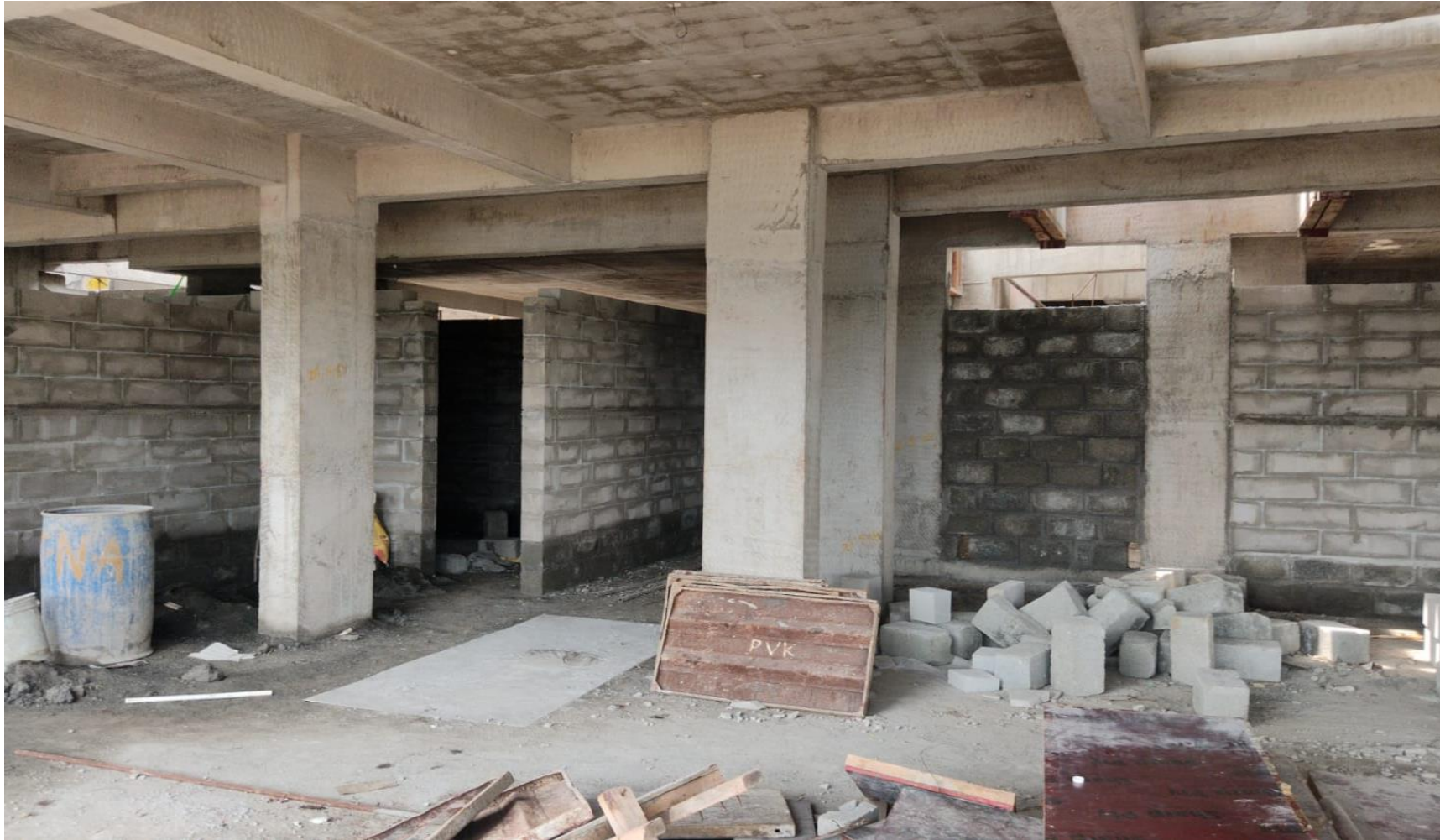
Main Building Stilt Floor Blockwork Up to Lintel Level Work Completed.
