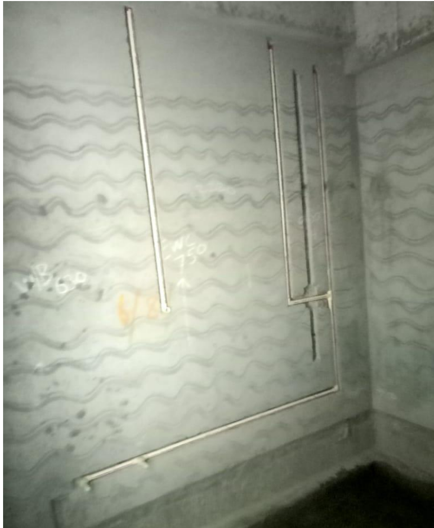
Main Building Pour-1 1 st Floor Plumbing Toilet Concealed pipe Line Work In Progress.
