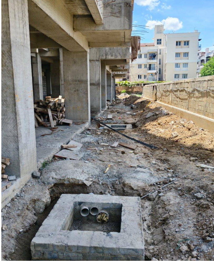
Main Building Stilt Floor Manhole Blockwork and plastering Work Nearing completion.
