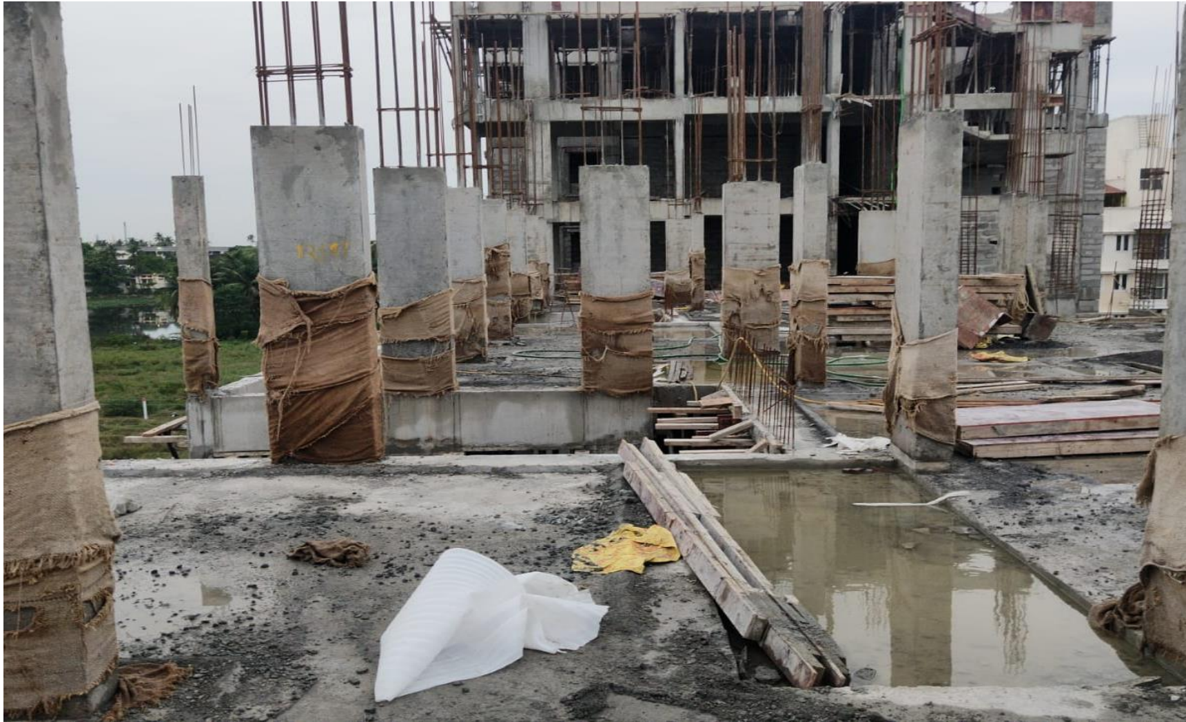
Main Building Pour-2 3 rd Floor Column Concrete Work Completed.
