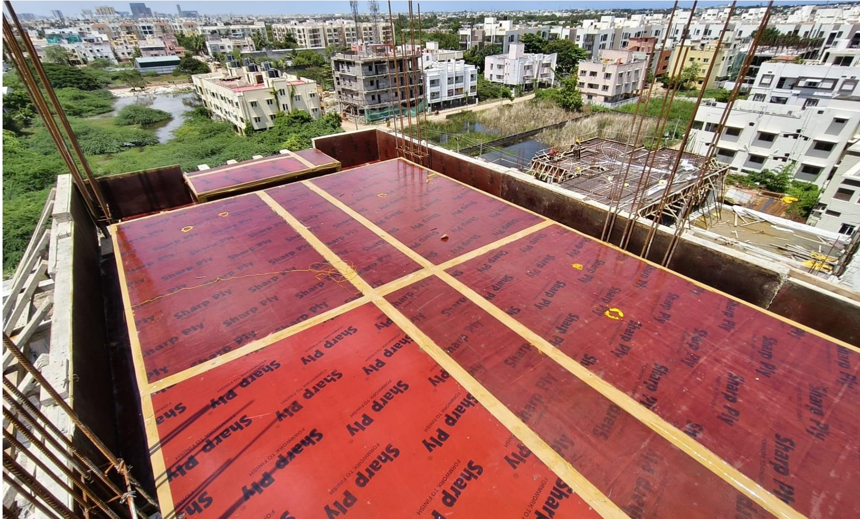
Main Building Pour-1 Staircase Head Room Shuttering Work Completed.
