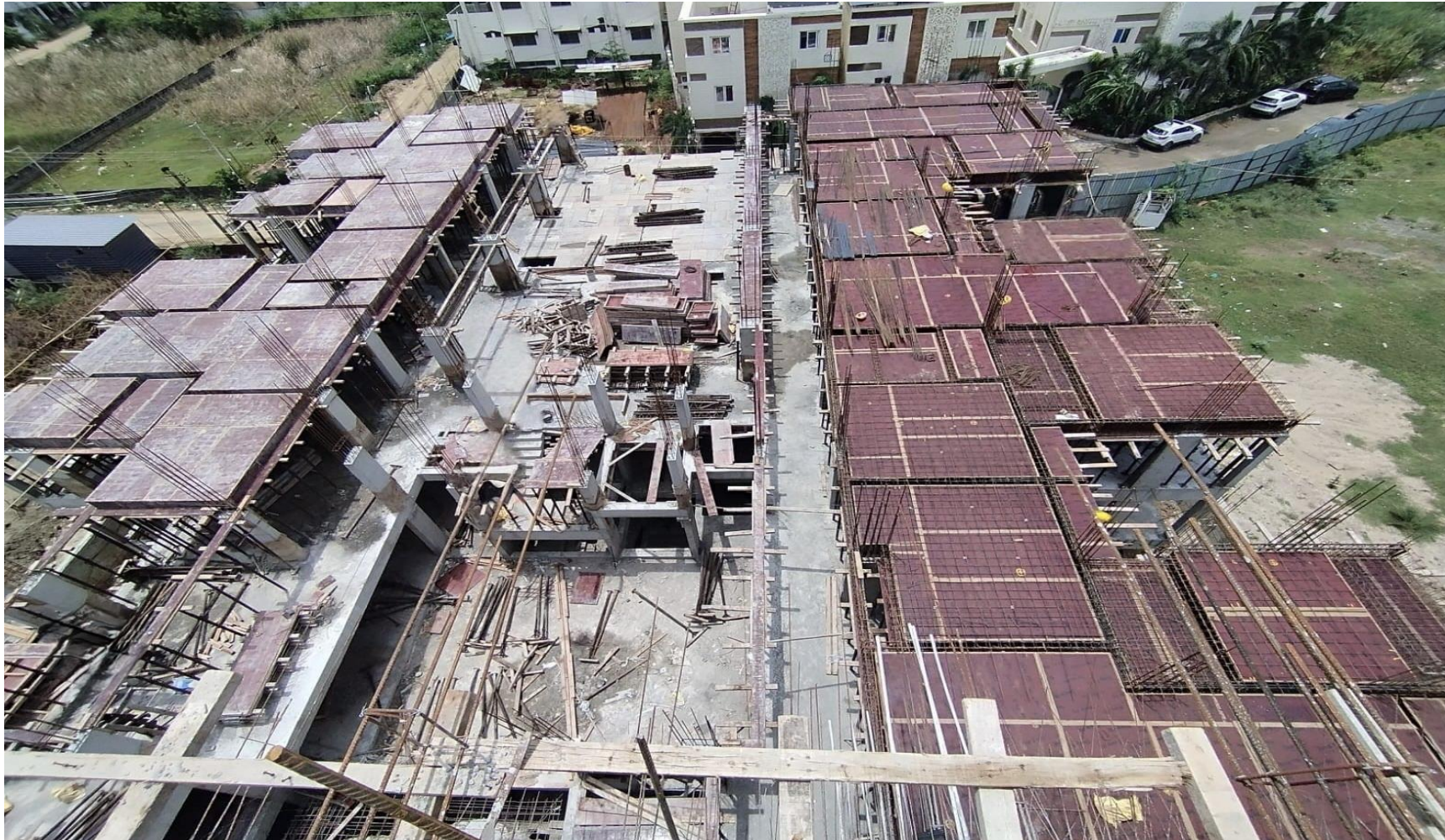
Main Building Pour-2 2 nd Floor Roof Slab Shuttering Work In Progress.
