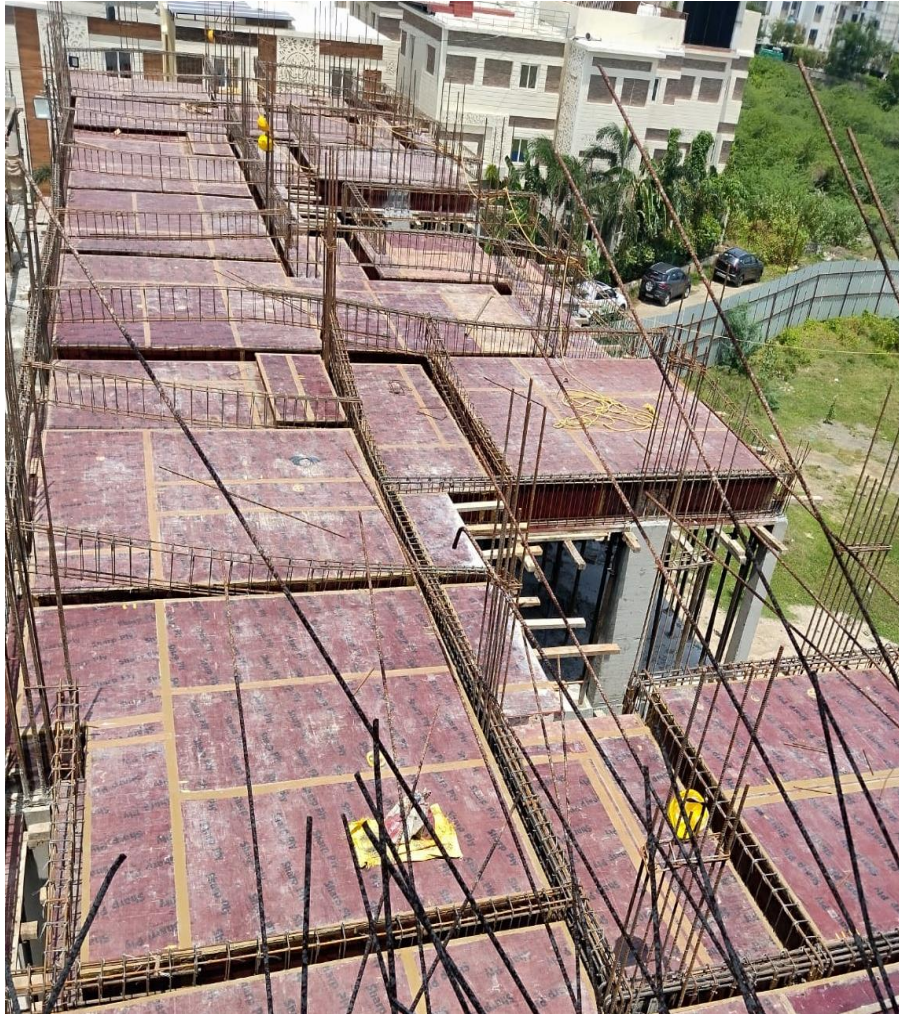
Main Building Pour-2 2 nd Floor Roof Slab Reinforcement Work In Progress.
