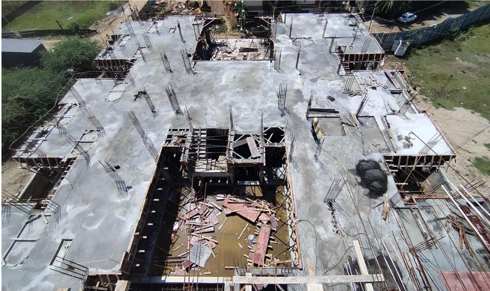
Main Building Pour-2 1 st Floor Roof Slab Concrete Work Completed.
