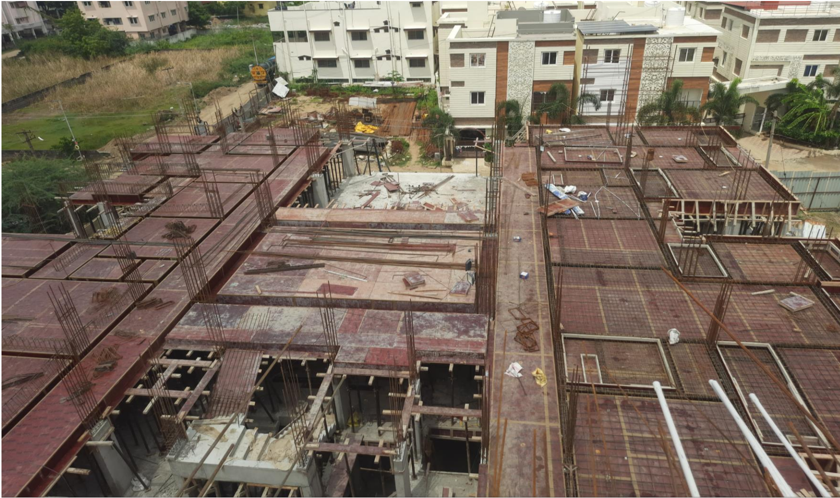
Main Building Pour-2 1 st Floor Roof Slab Shuttering Work Completed.
