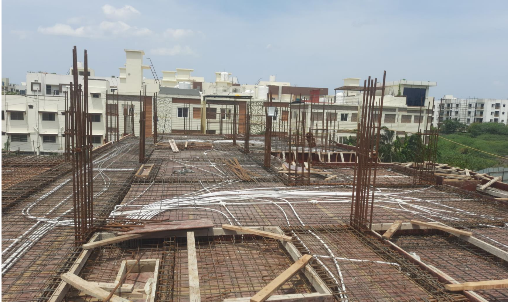
Main Building Pour-2 1 st Floor Roof Slab Reinforcement Work Completed.
