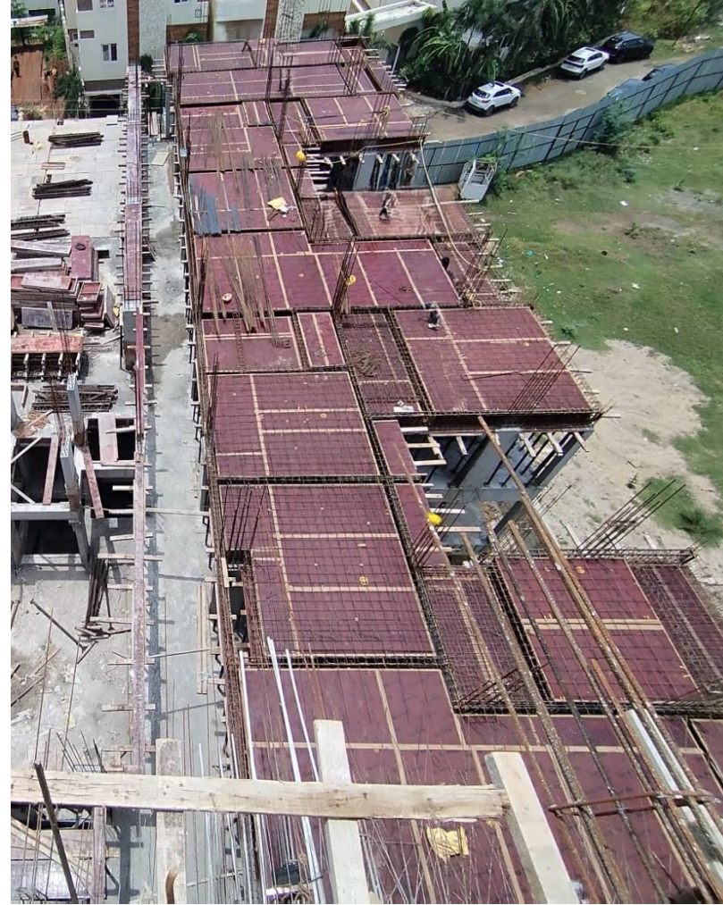
Main Building Pour-2 2 nd Floor Roof Slab Reinforcement Work In Progress.
