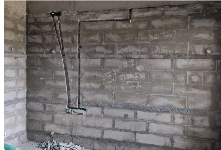
Main Building Pour-1 1 st Floor Electrical Wall Chasing Work In Progress.
