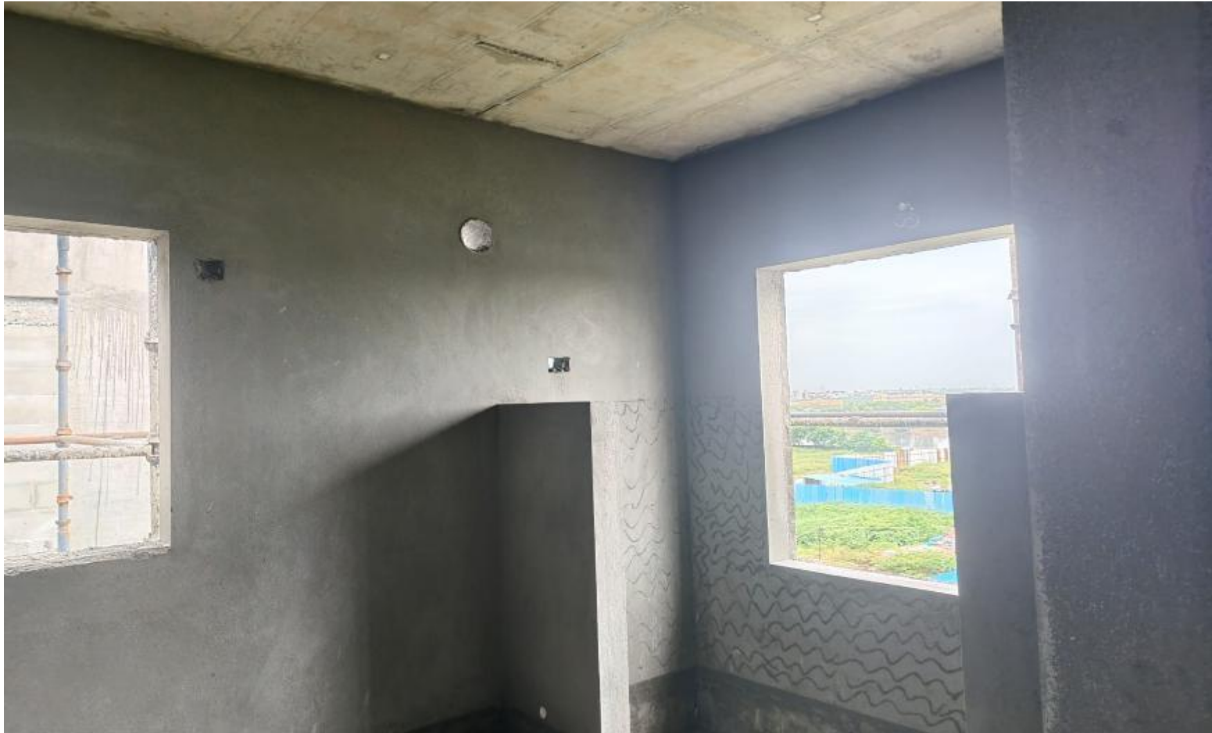
Main Building 5 th Floor Pour-1 Plastering Work In Progress.
