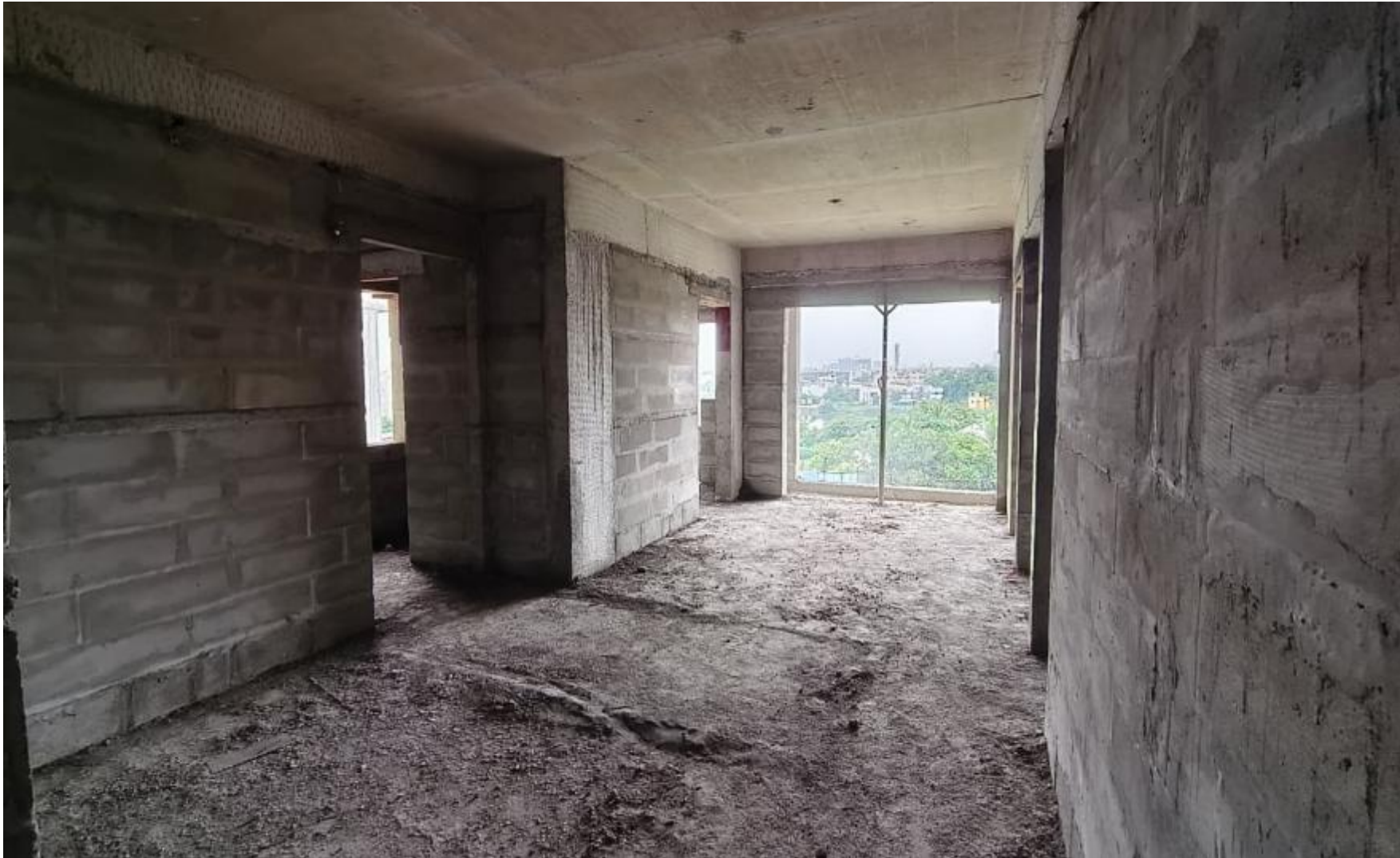
Main Building Pour-2 1 st Floor Blockwork Work Completed.
