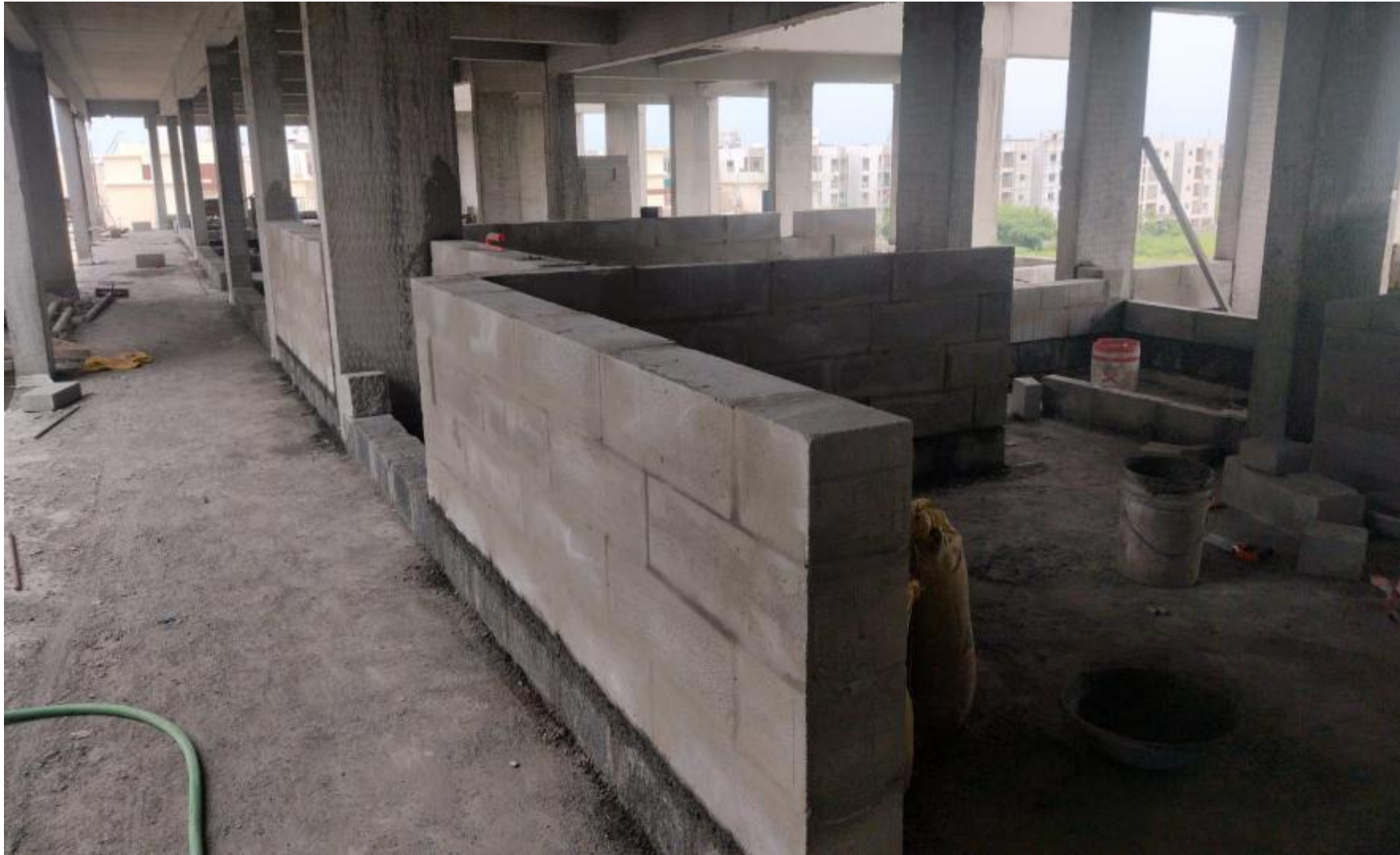
Main Building Pour-2 4 th Floor Blockwork Work In Progress.
