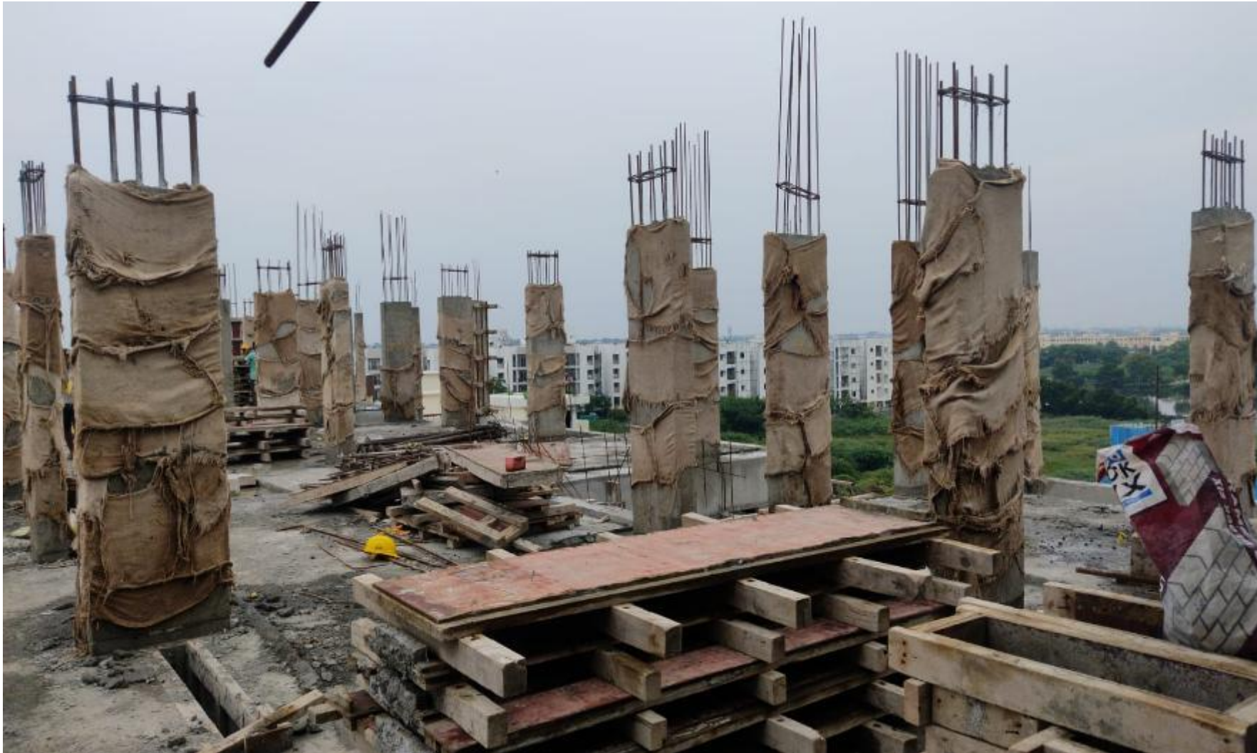
Main Building Pour-2 5 th Floor Column Concrete Work Completed.
