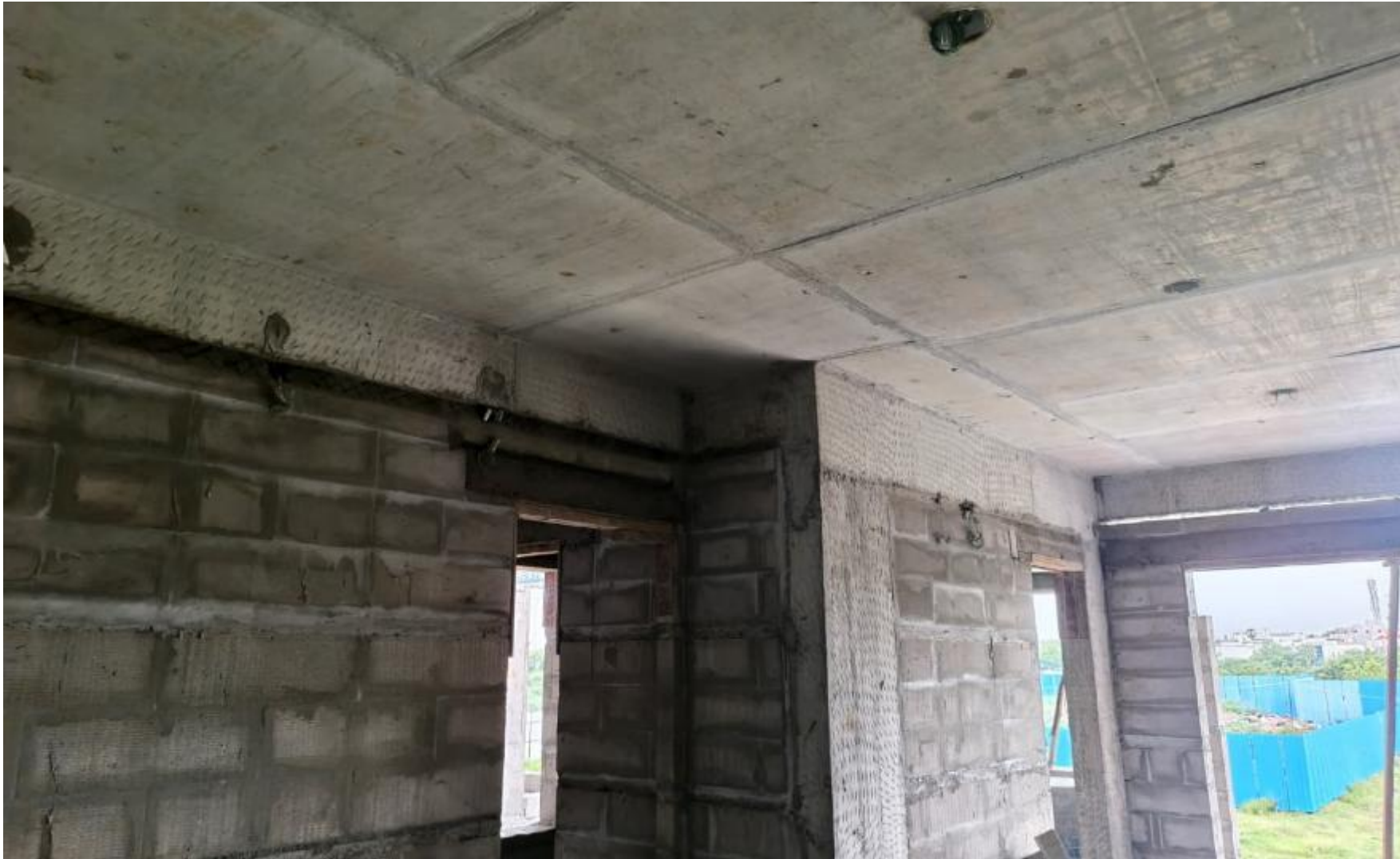
Main Building Pour-2 2 nd Floor Blockwork Work Nearing Completion.
