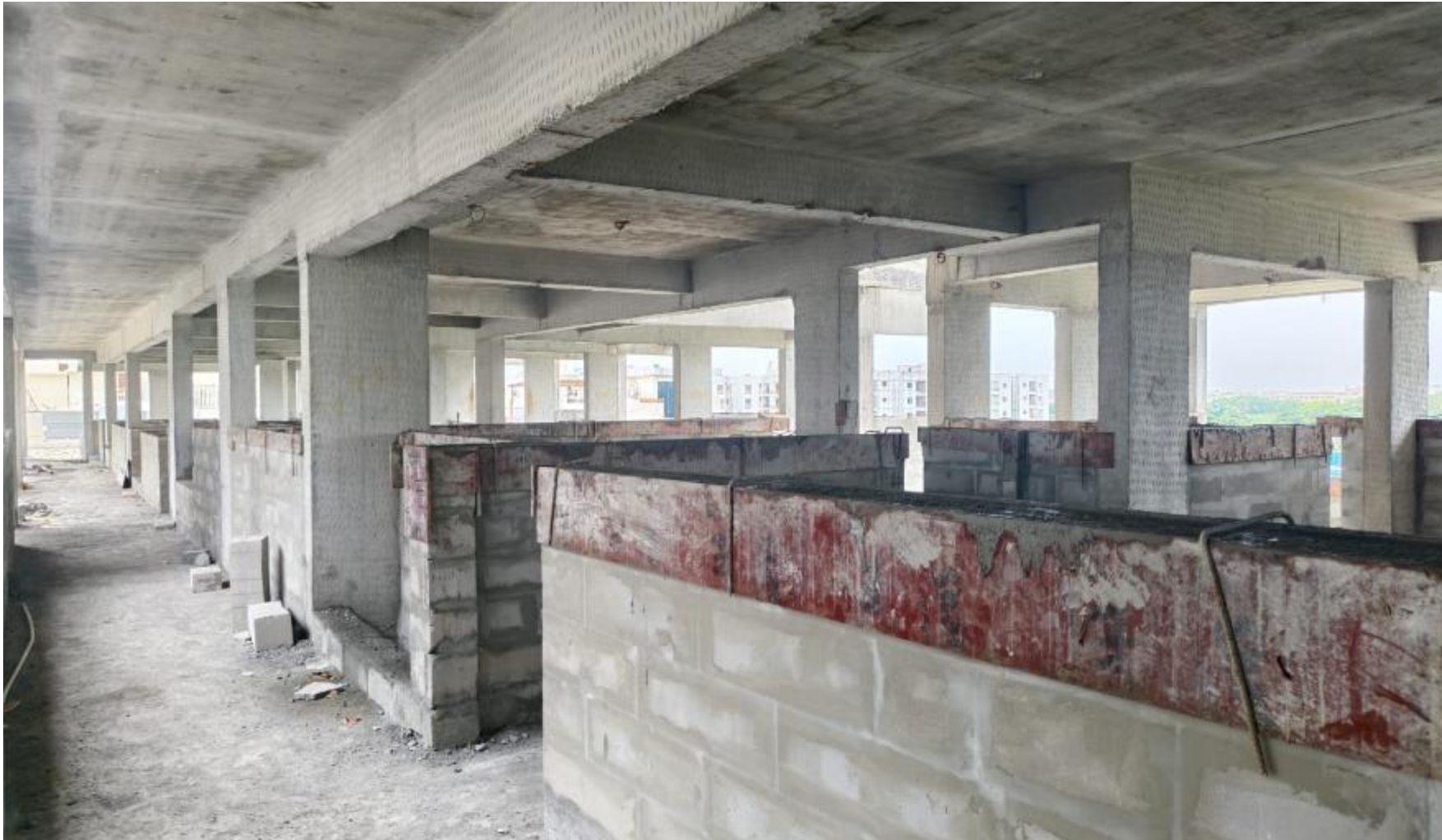
Main Building Pour-2 3 rd Floor Blockwork Up to Sill Level Work Completed.
