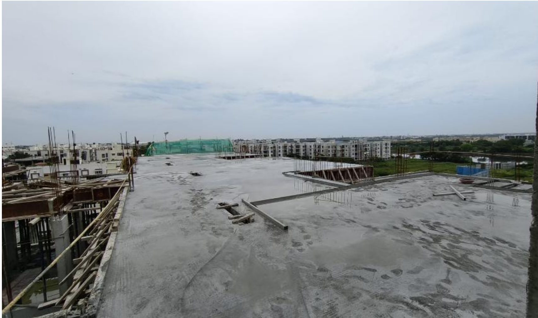
Main Building Pour-2 Terrace Floor Slab South Side Concrete Work Completed.
