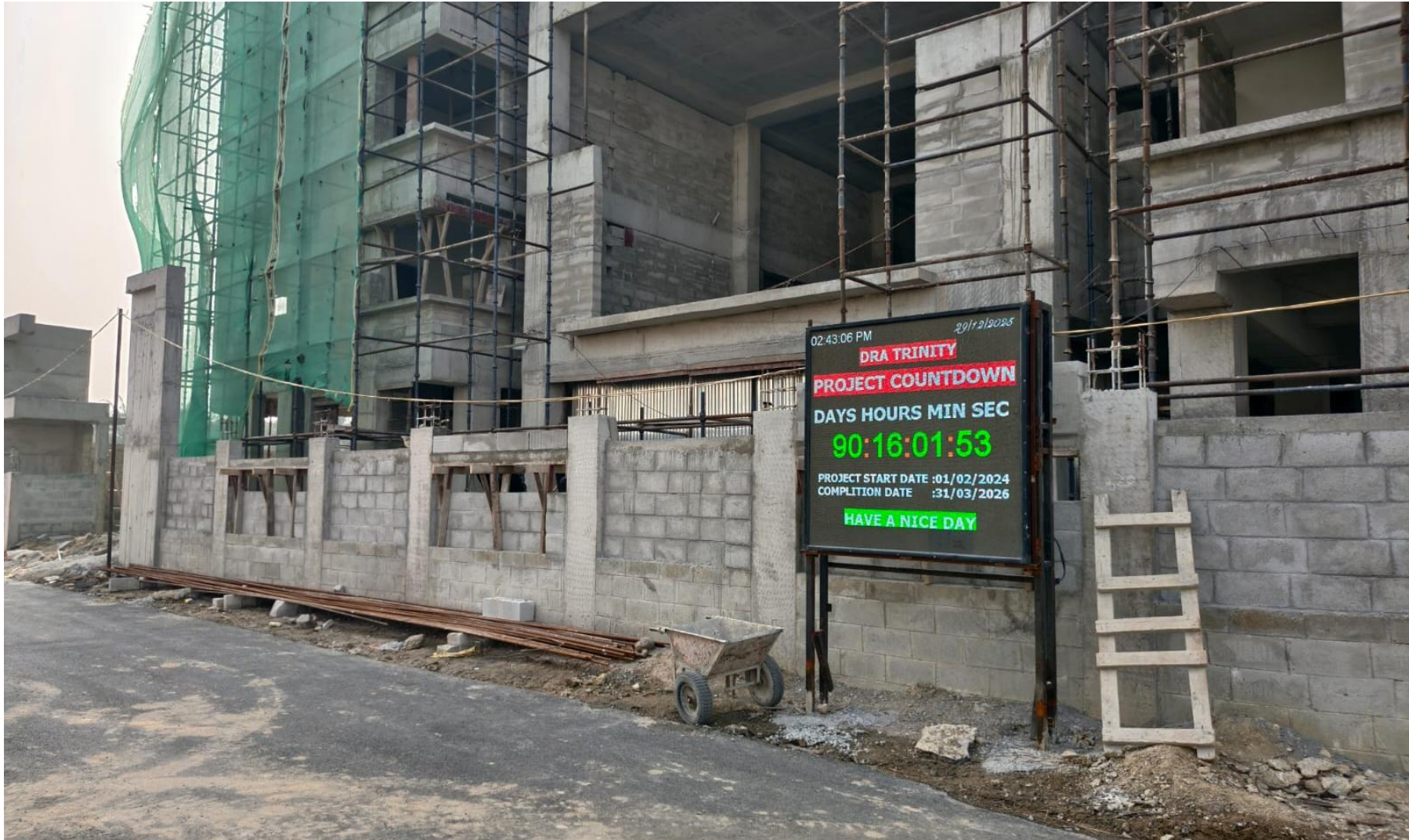
Compound Wall Entrance Blockwork Work Nearing Completion.
