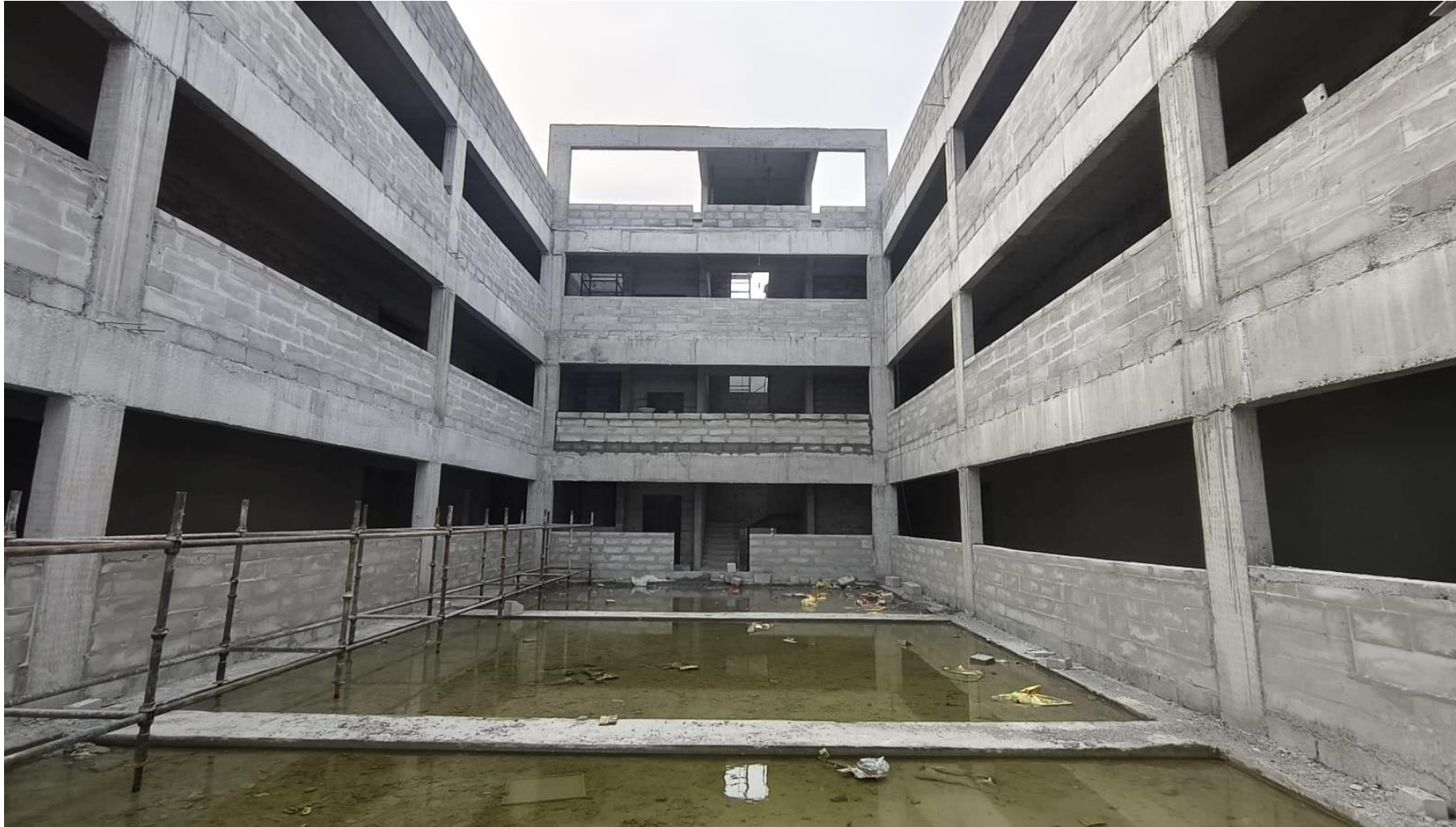
Main Building Pour-2 Podium Area Blockwork Work Nearing Completion.
