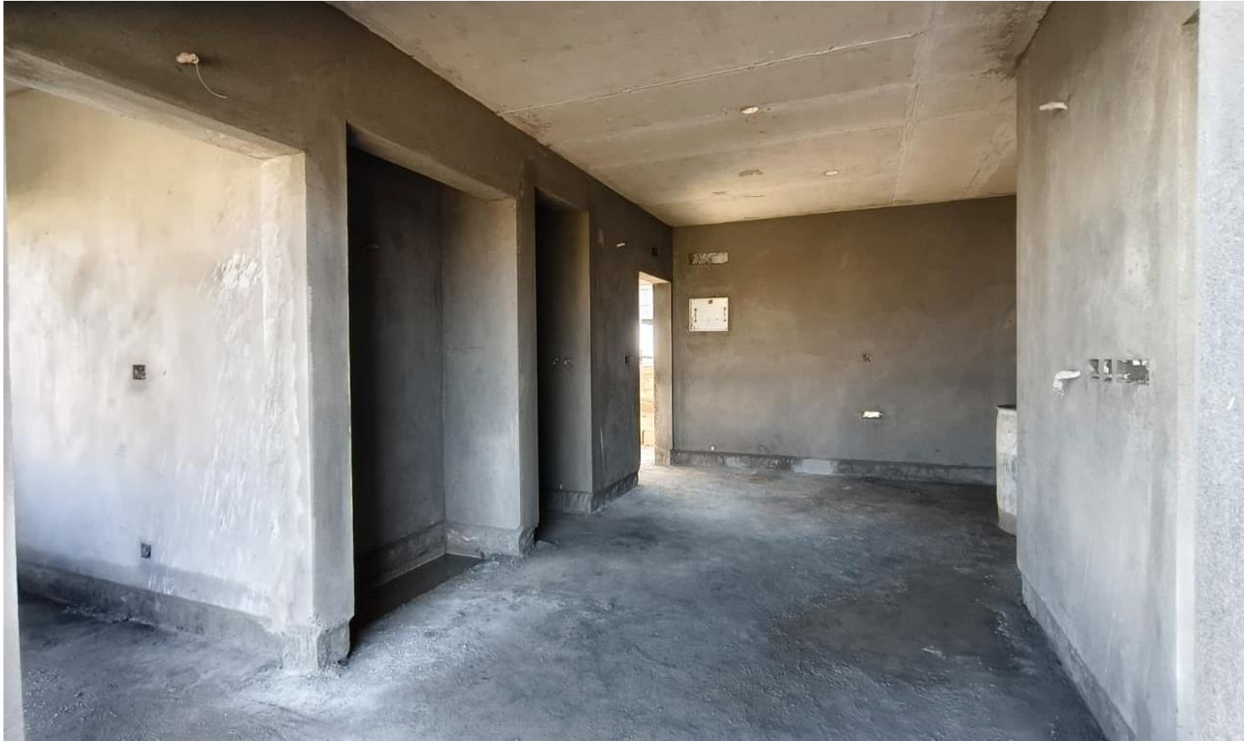
Main Building Pour-2 5 th Floor Plastering Work In Progress.
