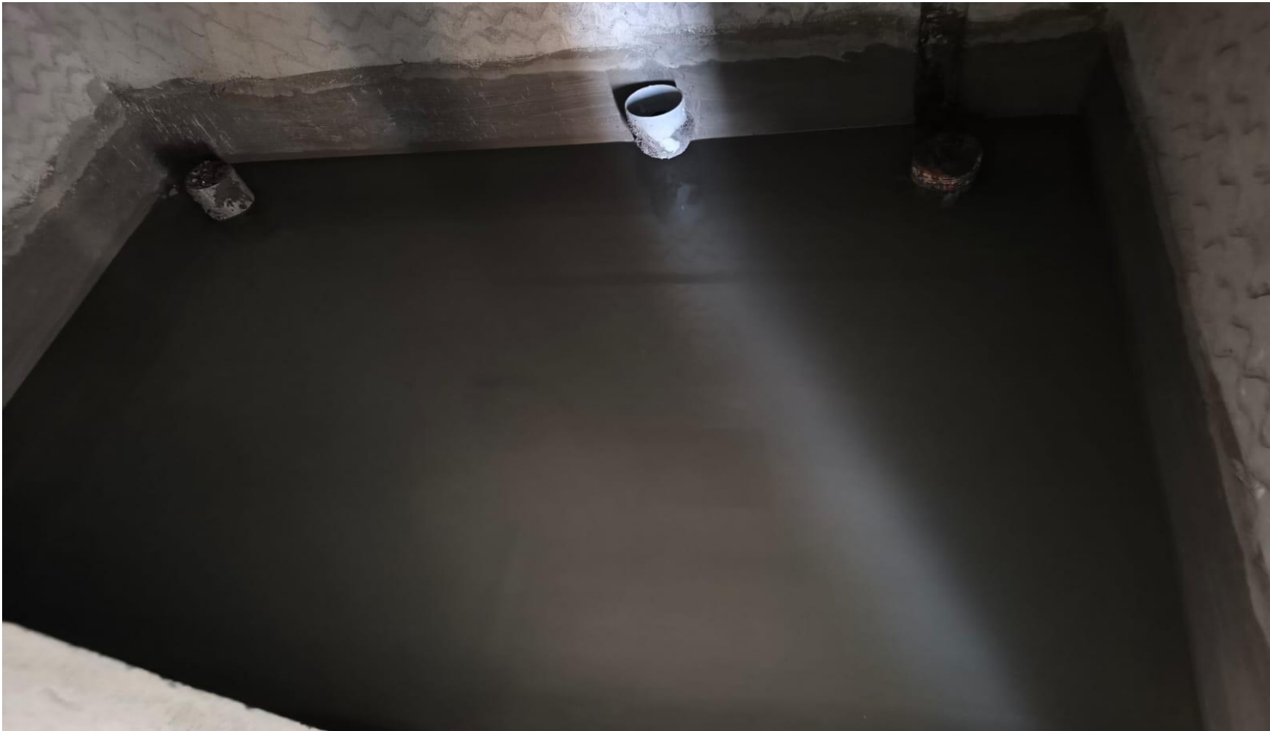
Main Building Pour-2 2 nd Floor Sunken Waterproofing Work Completed.
