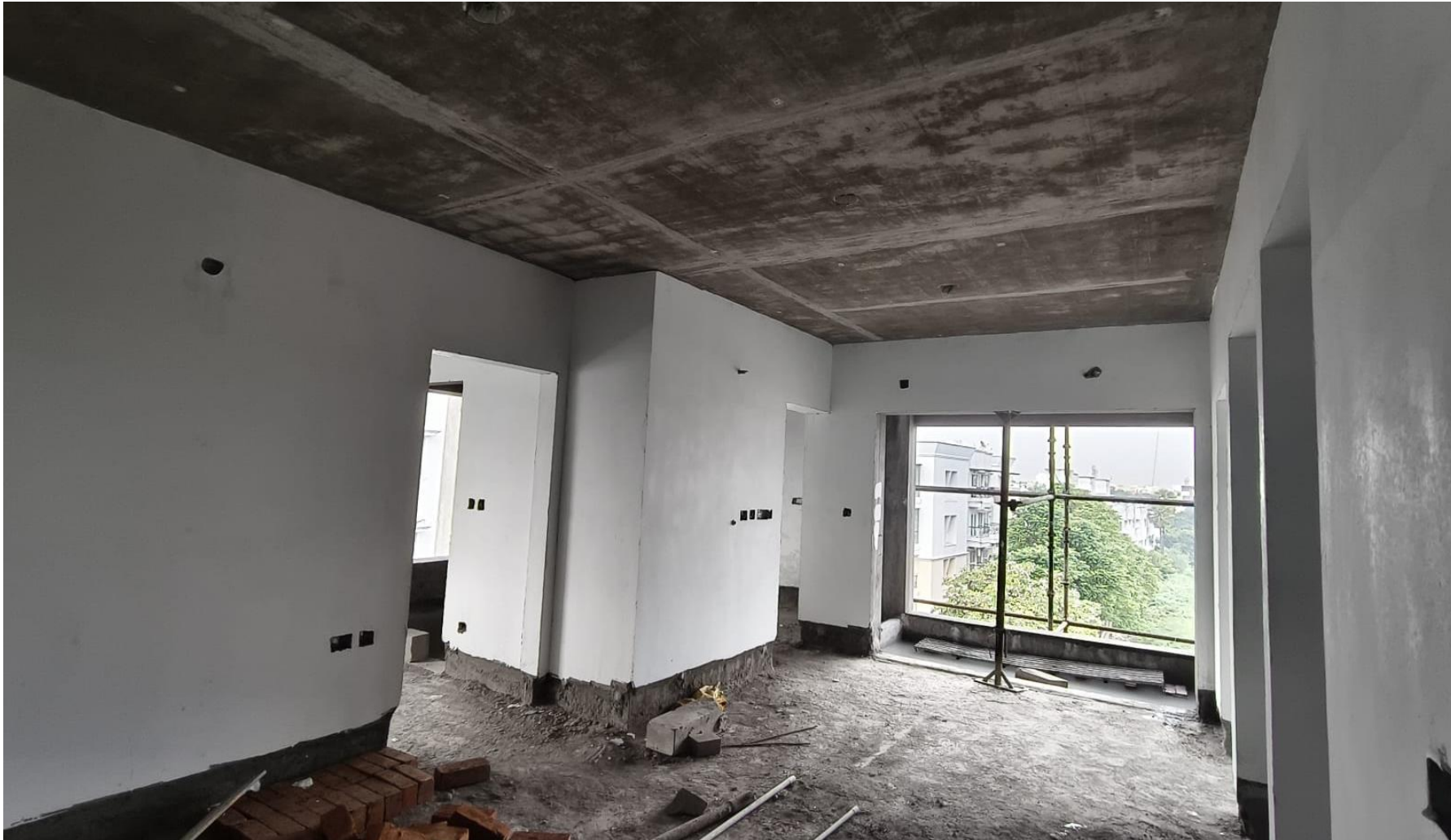
Main Building Pour-1 Up to 5 th Floor Wall Putty 1 Coat Work Completed.
