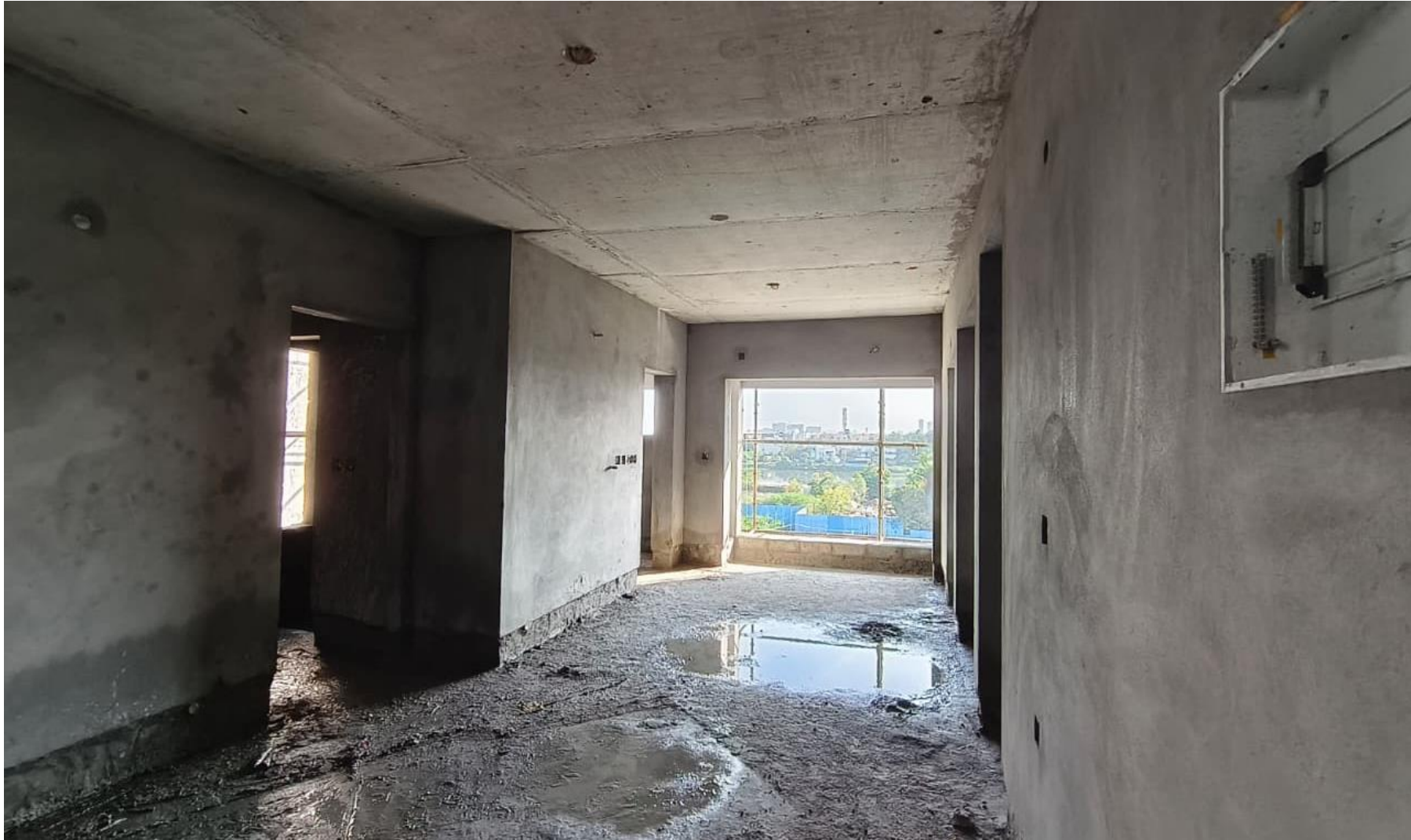
Main Building Pour-2 4 th Floor Plastering Work Completed.
