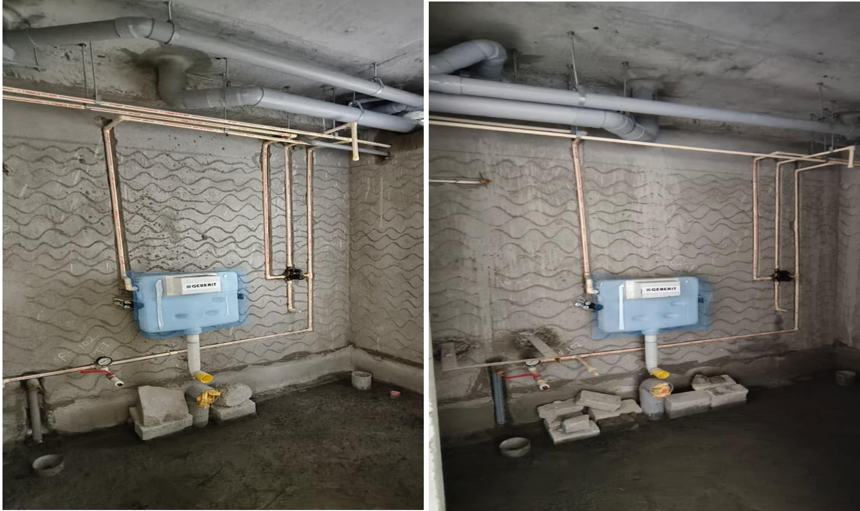
Main Building Pour-2 1 st Floor Plumbing Work Nearing Completion.
