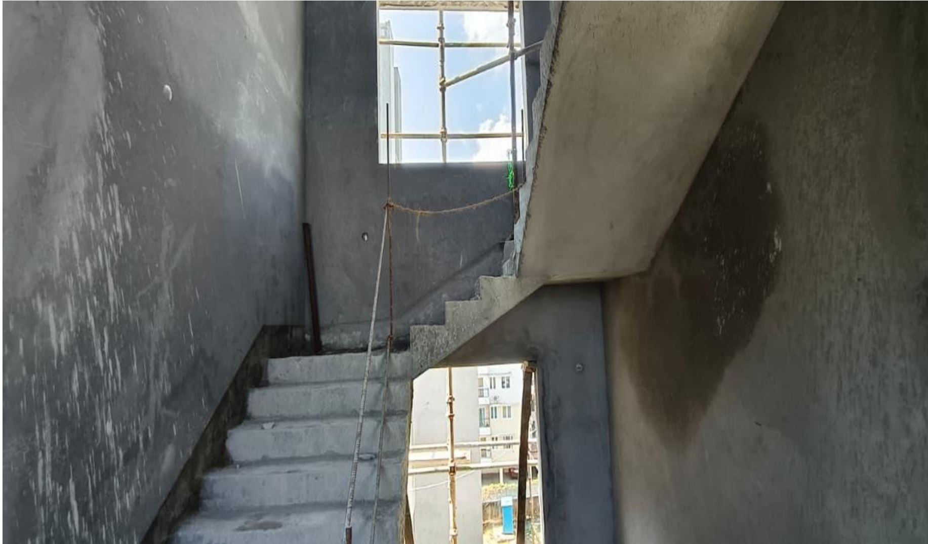
Main Building Pour-2 Staircase Plastering Work Completed.
