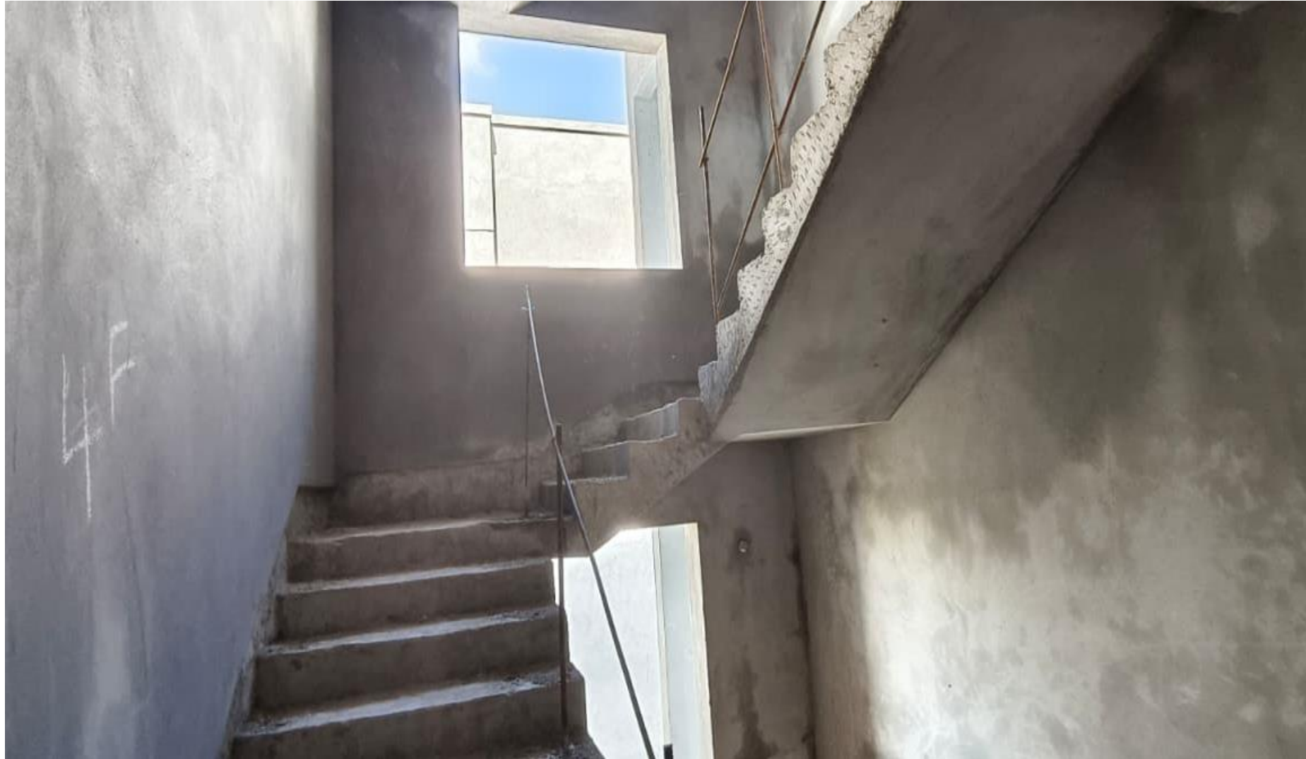
Main Building Pour-1 Staircase Plastering Work Completed.
