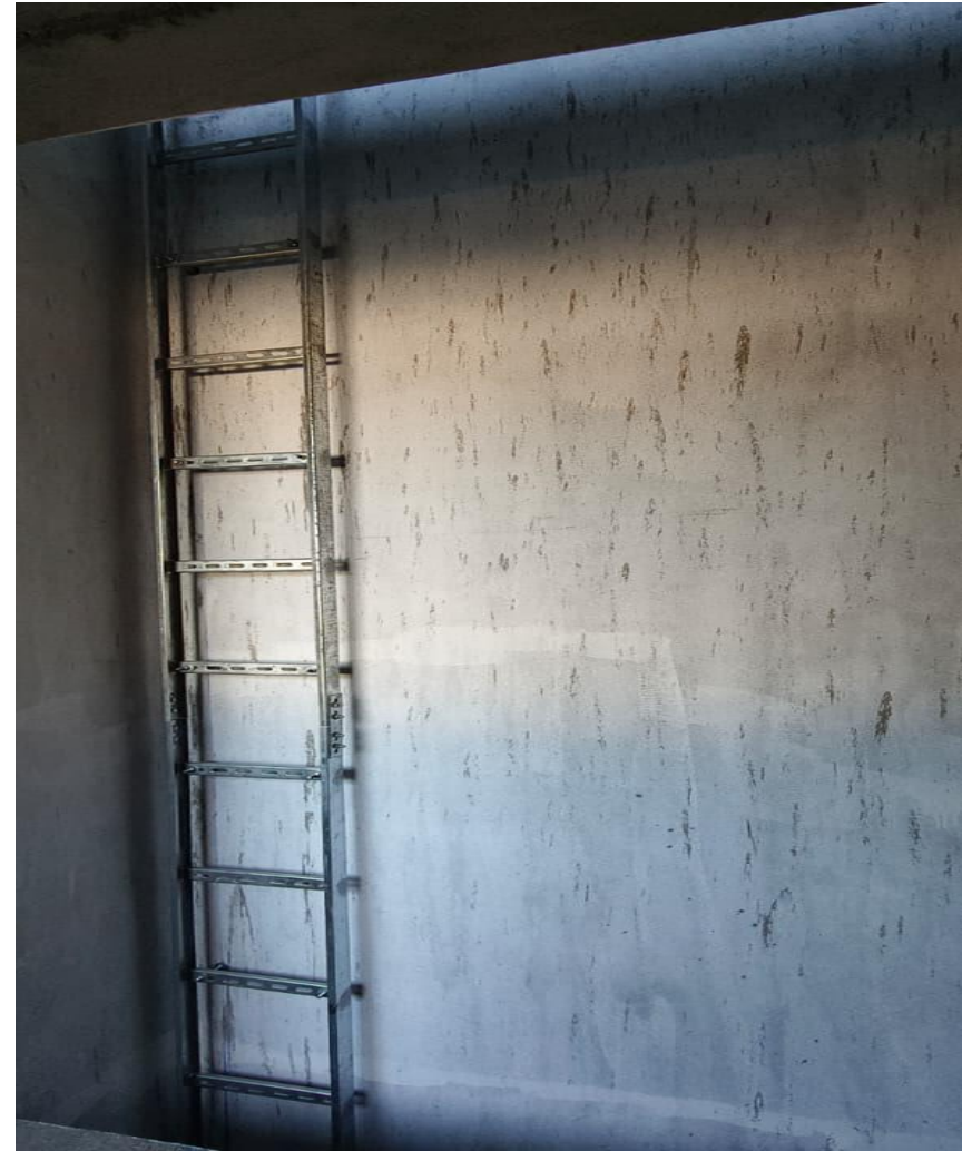
Main Building Electrical Shaft Tray Work In Progress.
