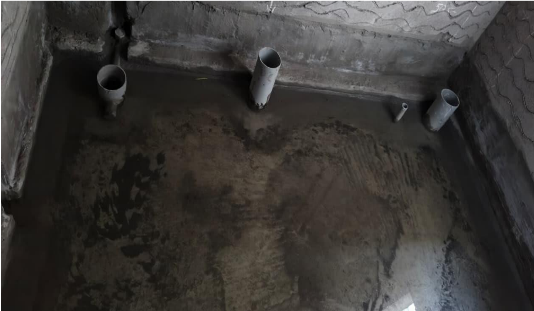
Main Building Pour-2 4 th Floor Sunken Waterproofing Work In Progress.
