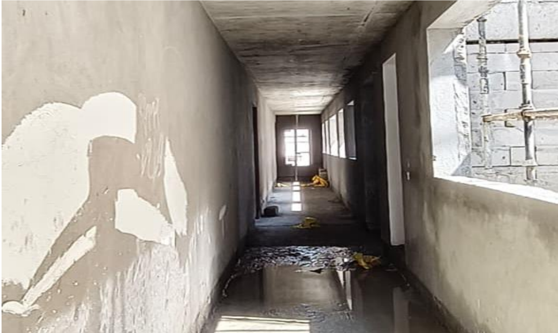
Main Building Pour-2 3 rd Floor Corridor Plastering Work Completed.
