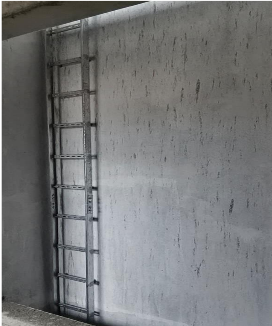
Main Building Electrical Shaft Tray Work In Progress.
