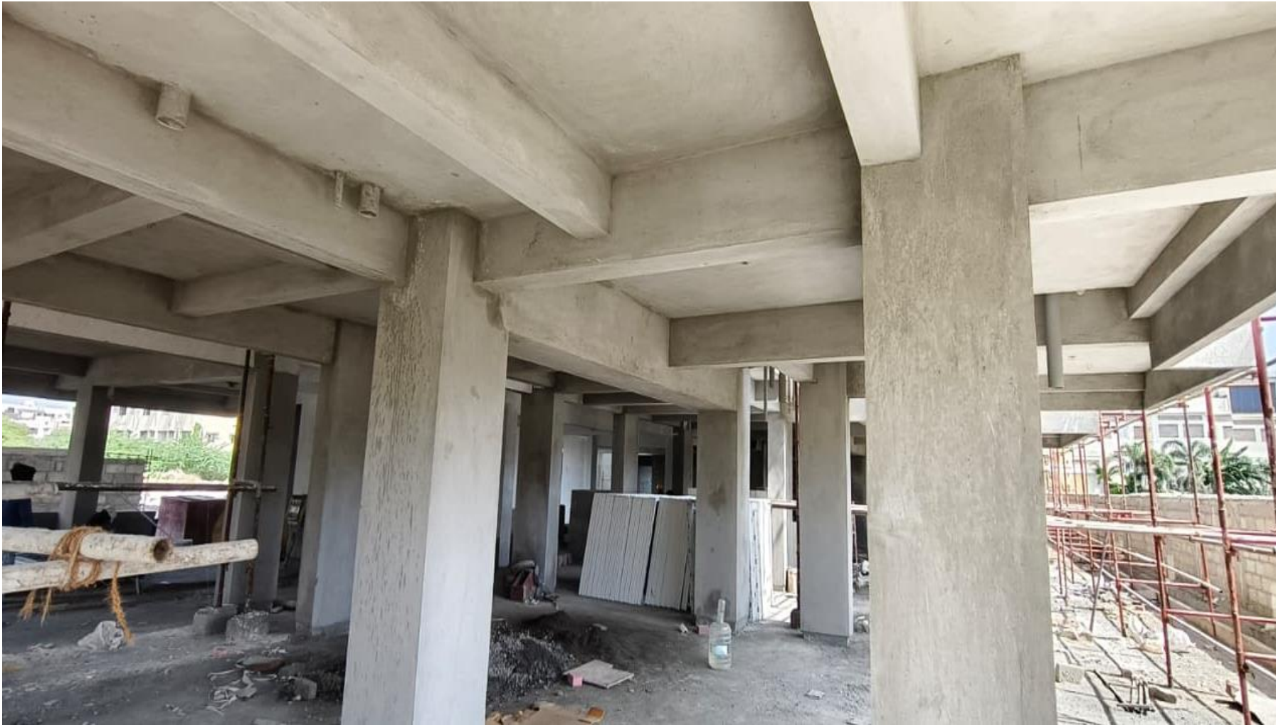
Main Building Pour-1 Stilt Floor Ceiling and Column Plastering Work Completed.
