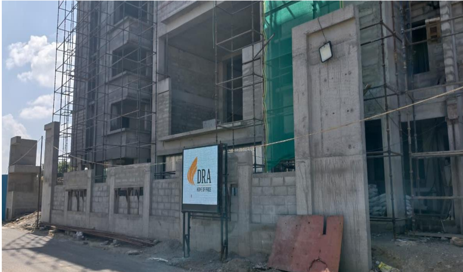
Compound Wall Entrance Blockwork Work Completed.
