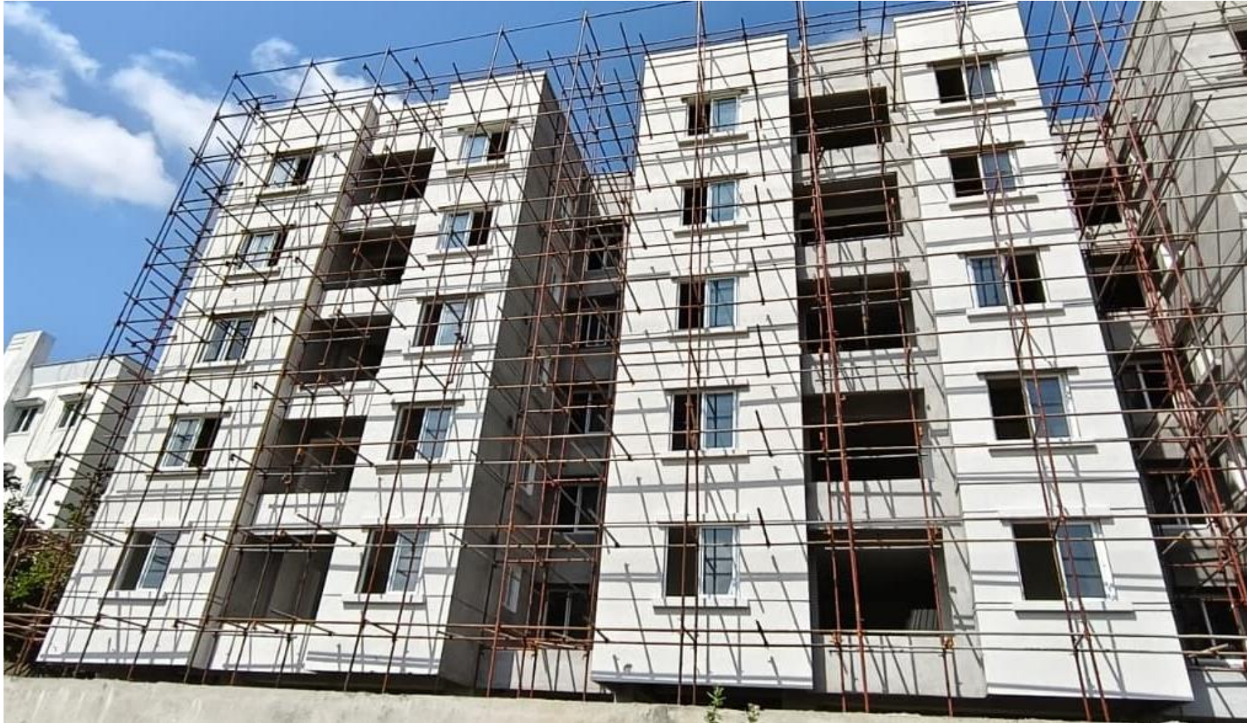
Main Building Pour-1 South Side External Texture Painting Work In Progress.
