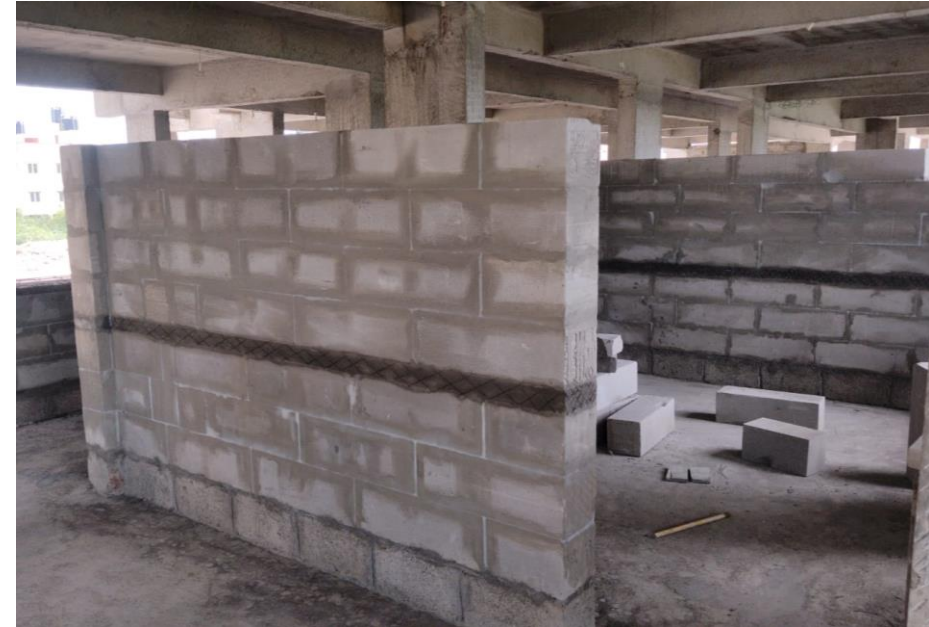
Main Building 1 st Floor Pour-1 Blockwork Work In Progress.
