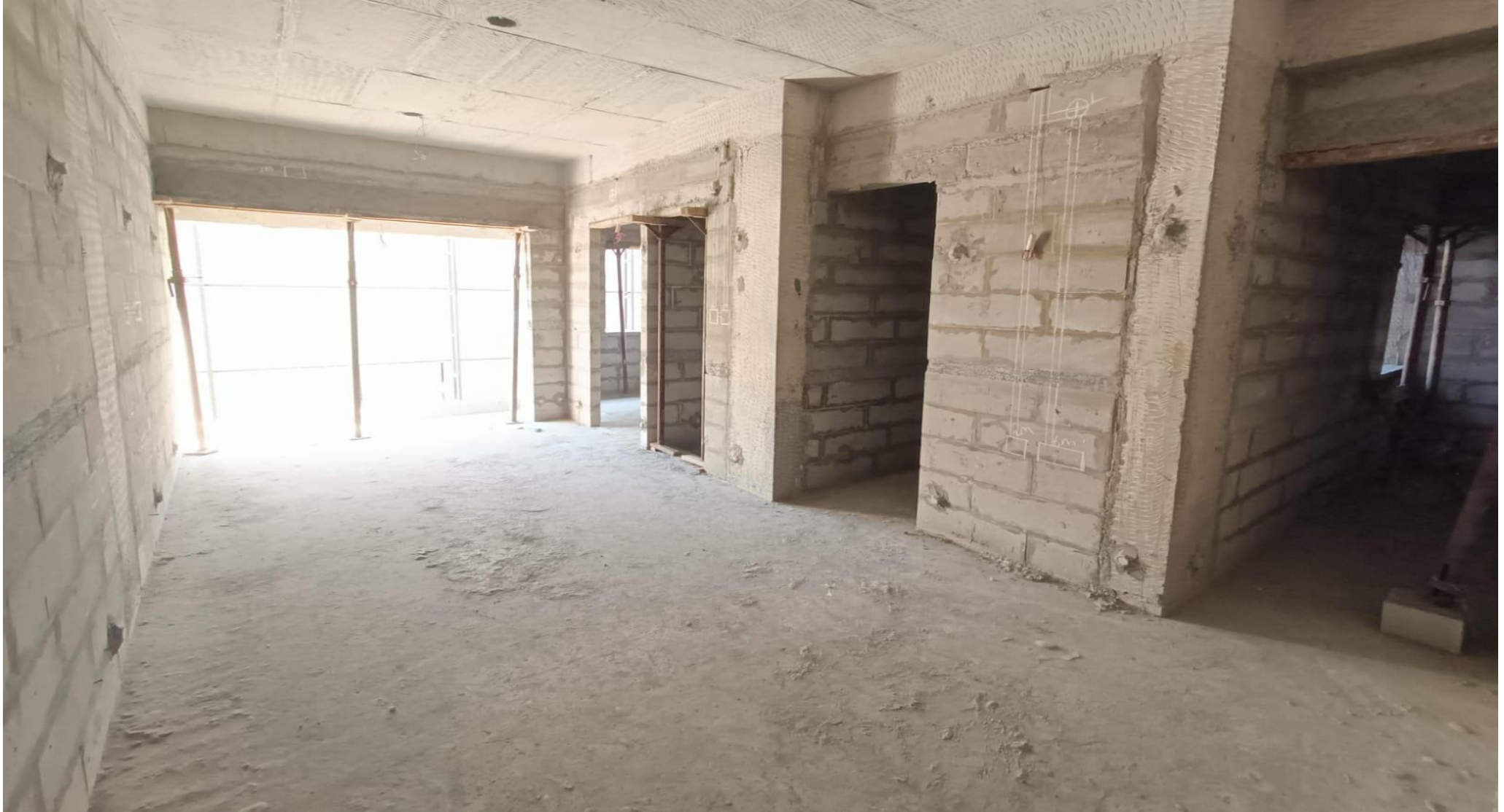
1 st Floor Masonry Work Completed- Wing 3D & 3E
