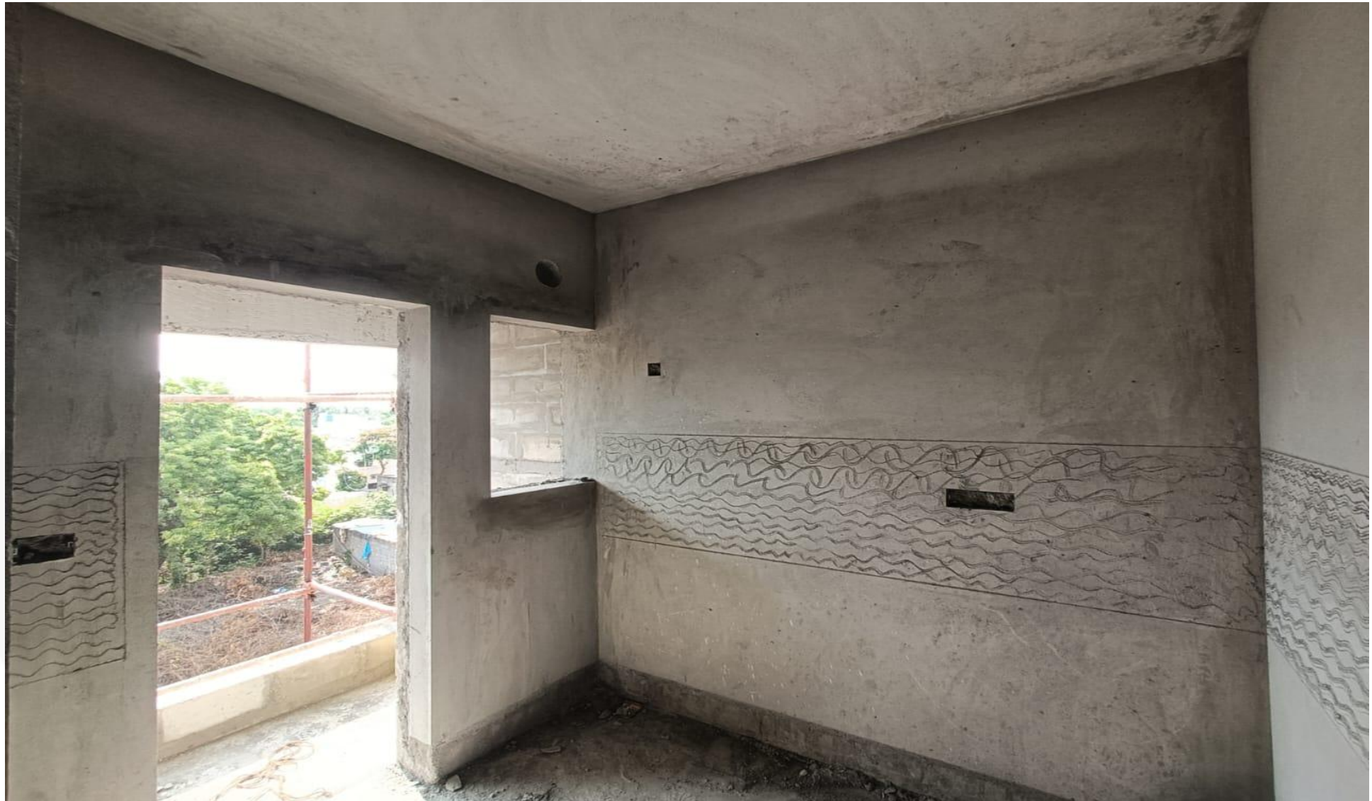
Wing 3E – 3 rd Floor Internal Plastering Work has been completed
