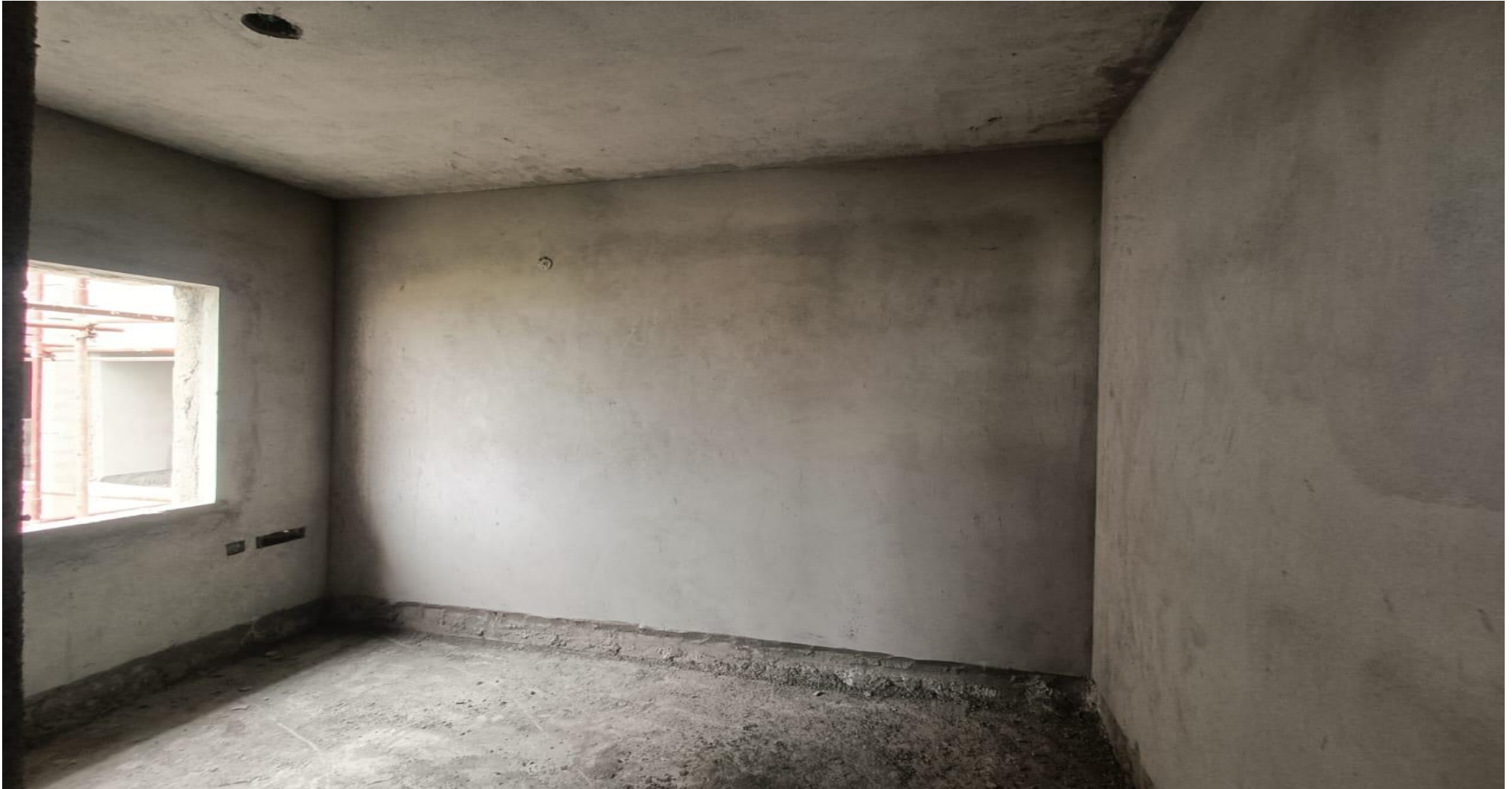
Wing 3D – 4 th Floor Plastering work in Progress
