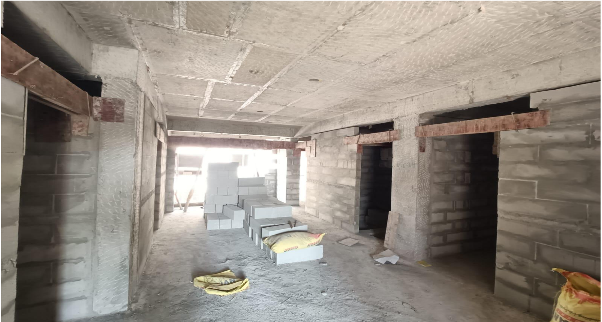
Wing 4A & 4B – 2 nd Floor Block work in Progress
