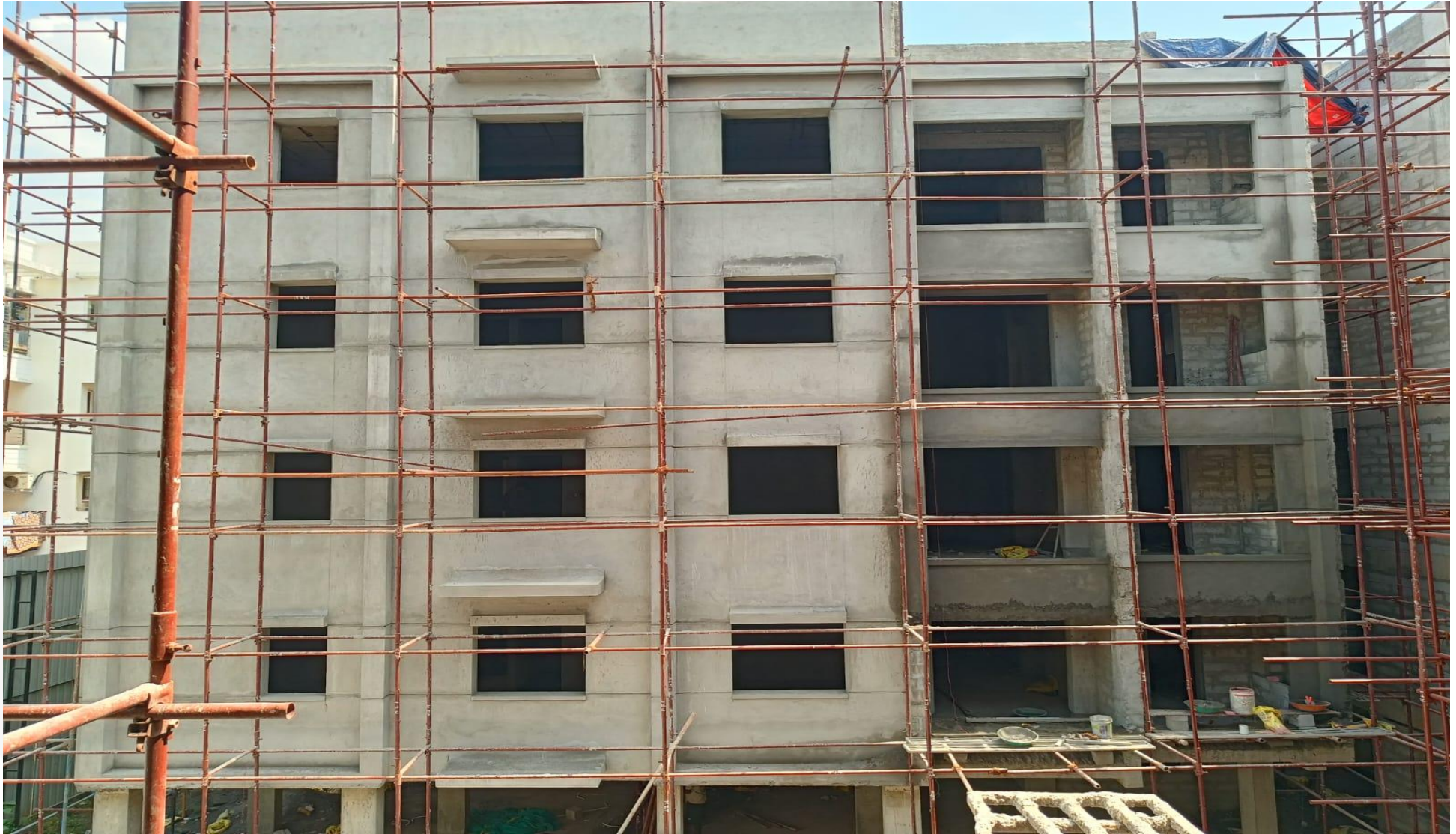
Wing 3C – North Elevation View
