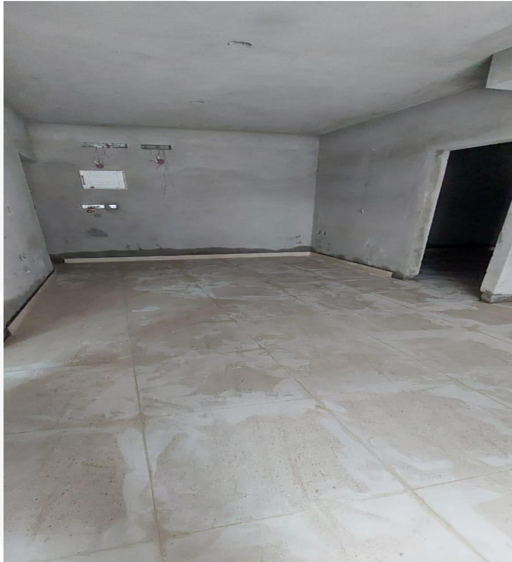
Wing 3D – 2 nd Floor Tile Work in Progress
