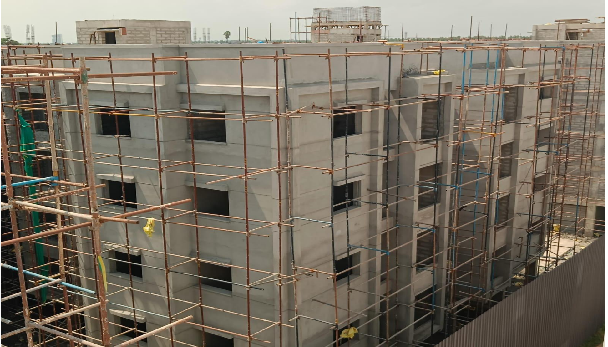
Wing 3C – East & South Elevation View
