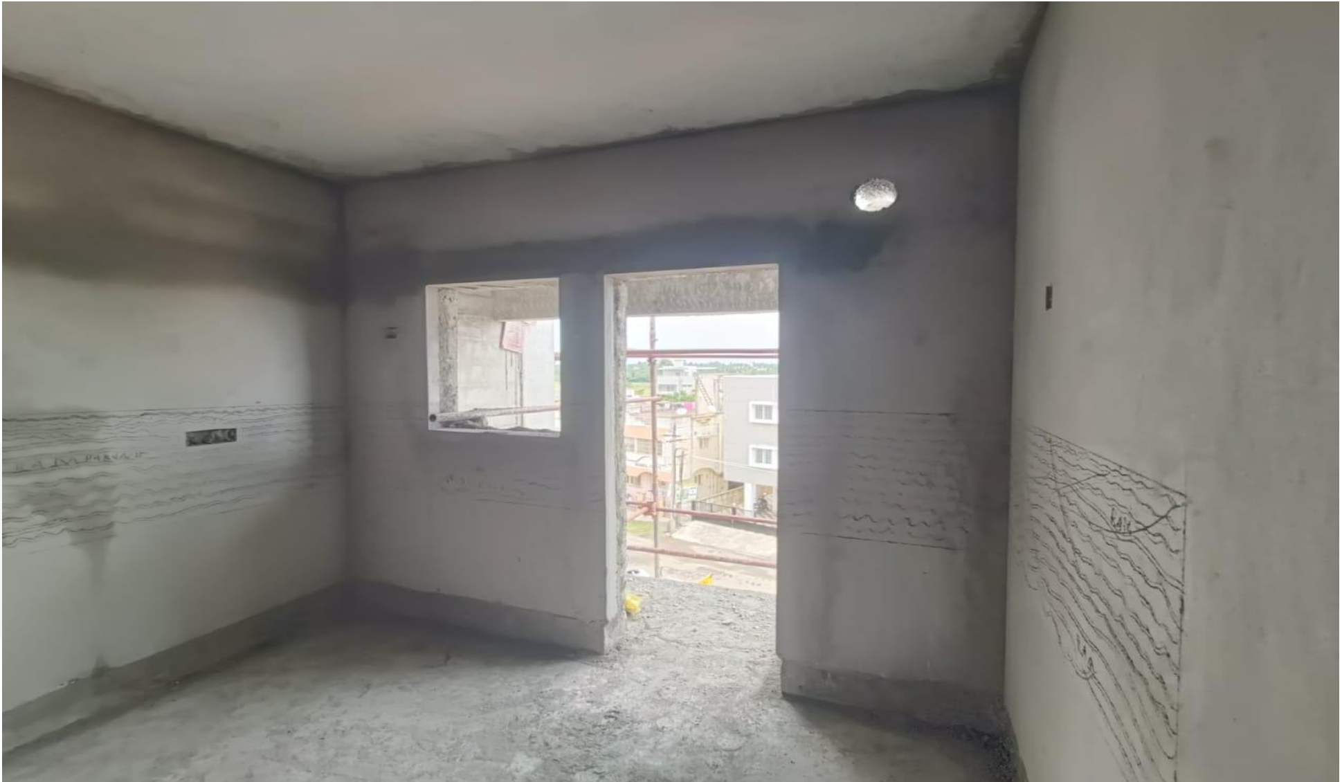
Wing 3A – 3 rd Floor Internal Plastering Work has been completed
