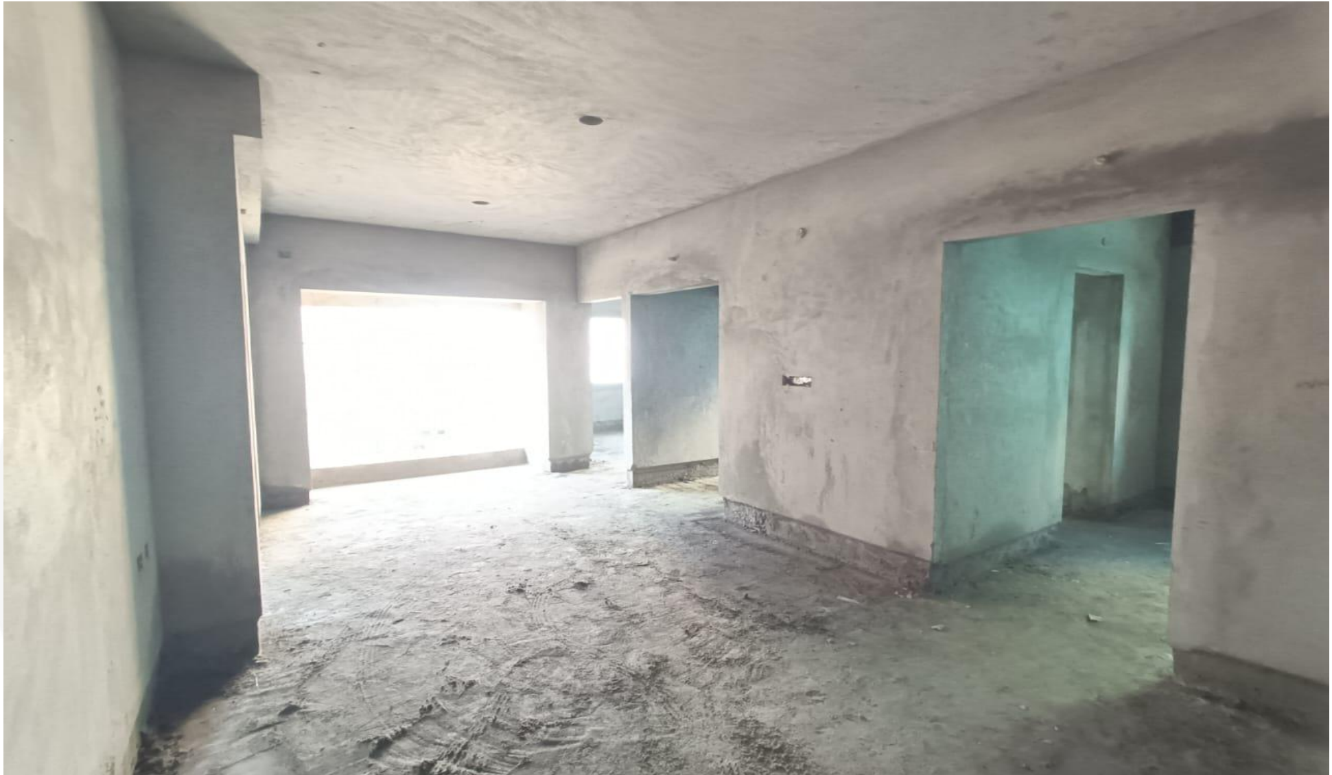
Wing 3D – 3 rd Floor Internal Plastering Work has been completed
