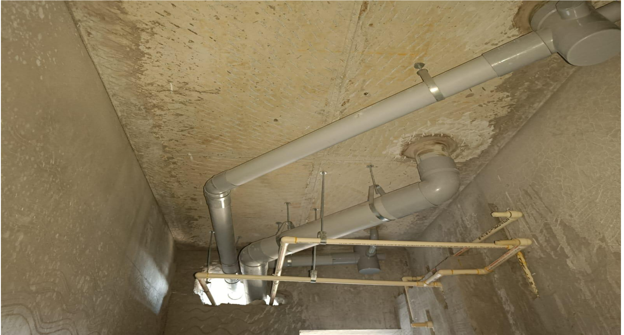
Wing 3D – 2 nd Floor Ceiling Suspended Line work in Progress
