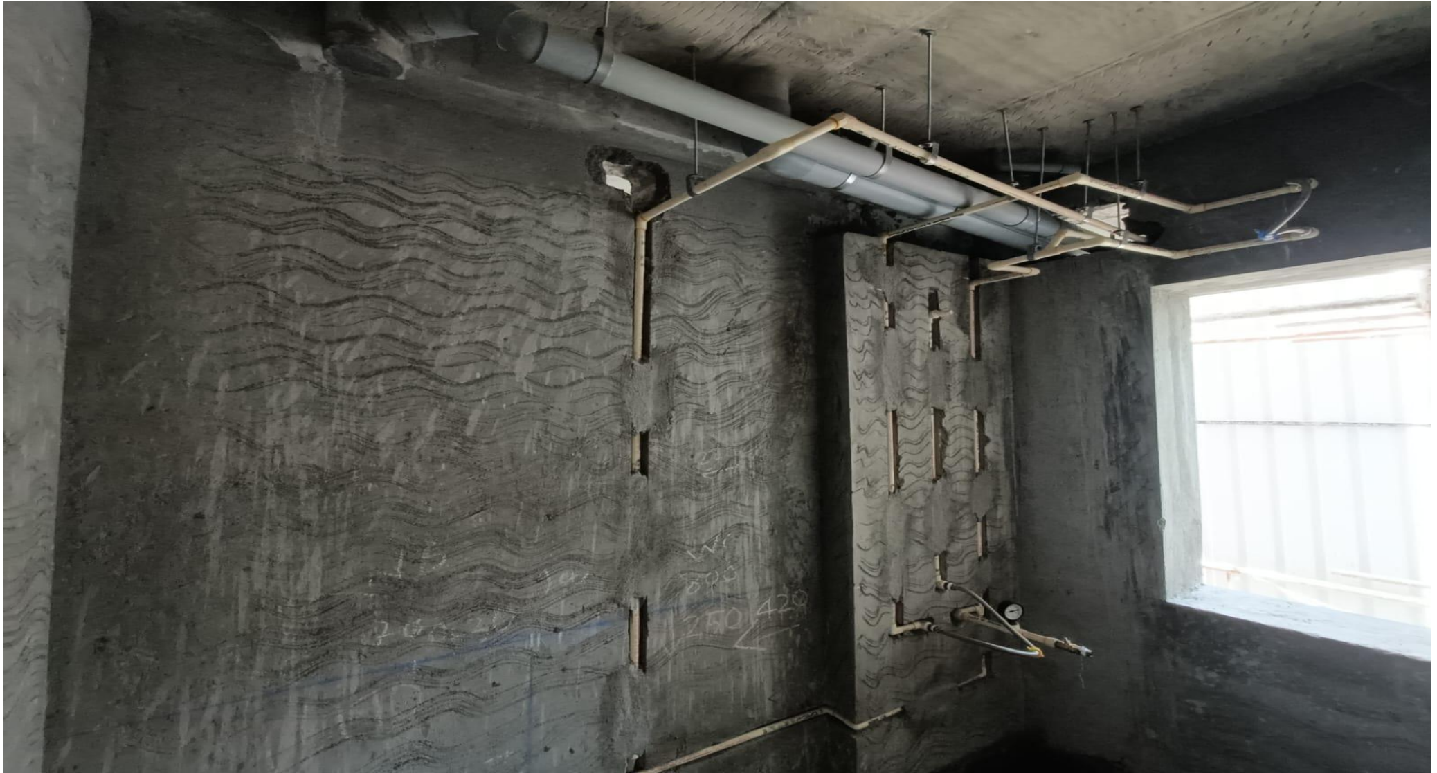
Wing 3E – 1 st Floor Toilet Ceiling Suspended Line Work in Progress
