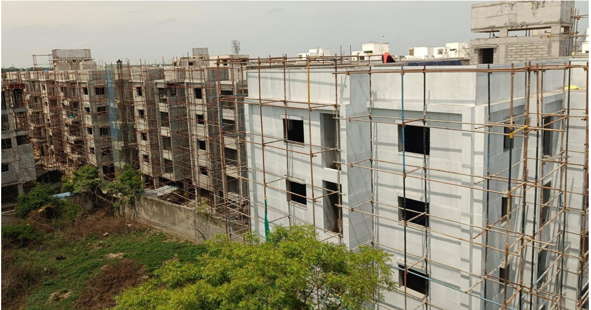
Wing 3E, 3C & 3A – West Elevation View
