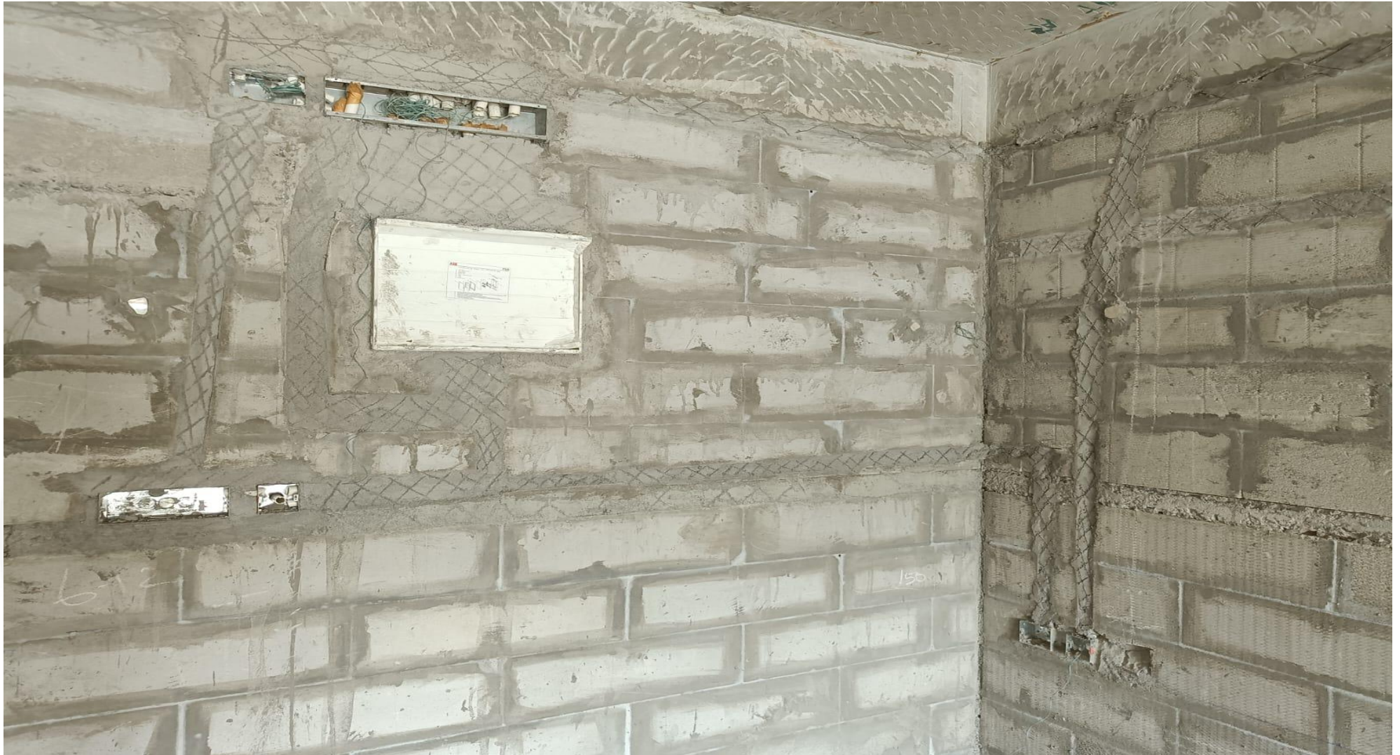
Wing 4A & 4B – 1st Floor Electrical conduit Work in Progress
