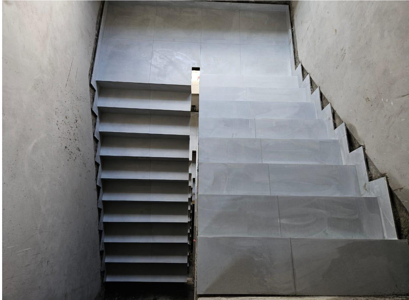
Wing 3A, 4 th Floor – Staircase Tile Works in Progress
