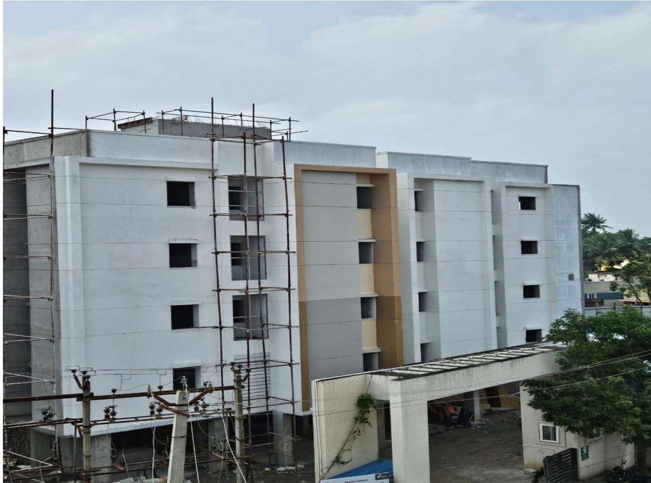
Wing 4A – North Elevation View
