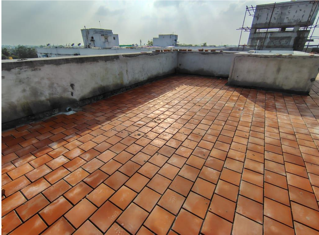
Wing 3D – Terrace Pressed Tile Works in Progress
