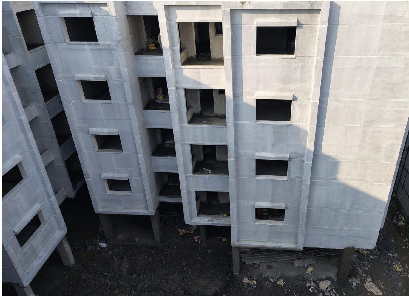
Wing 3A & 3B – Exterior Damp proof works in Progress
