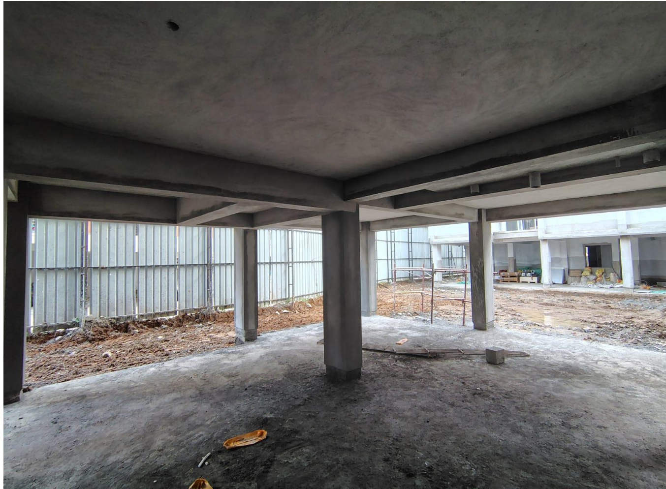
Wing 3A, 3B & 3C – Stilt Floor Plastering Works in Progress
