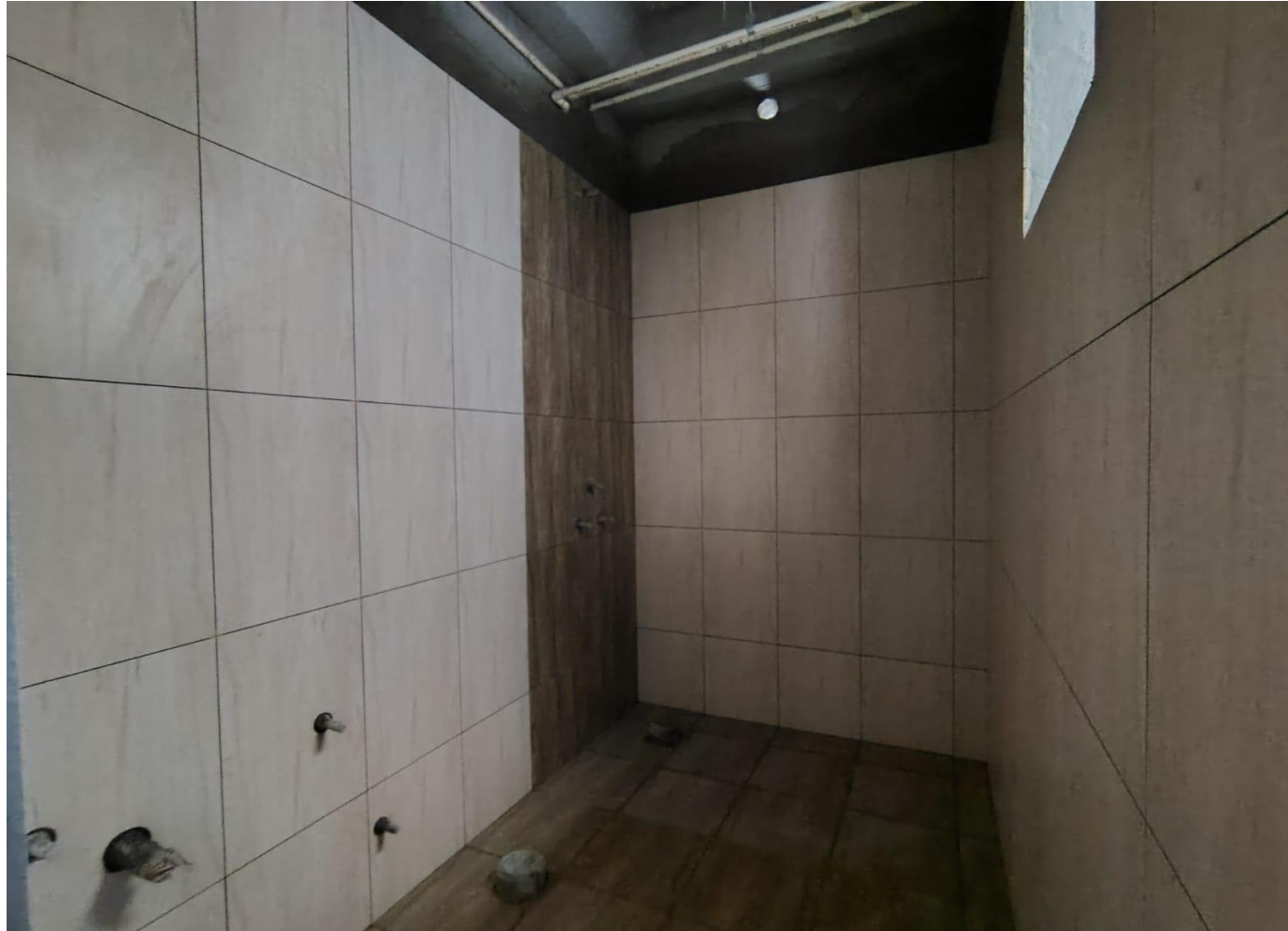
Wing 3A, 4 th Floor – Master Toilet Tile Works in Progress
