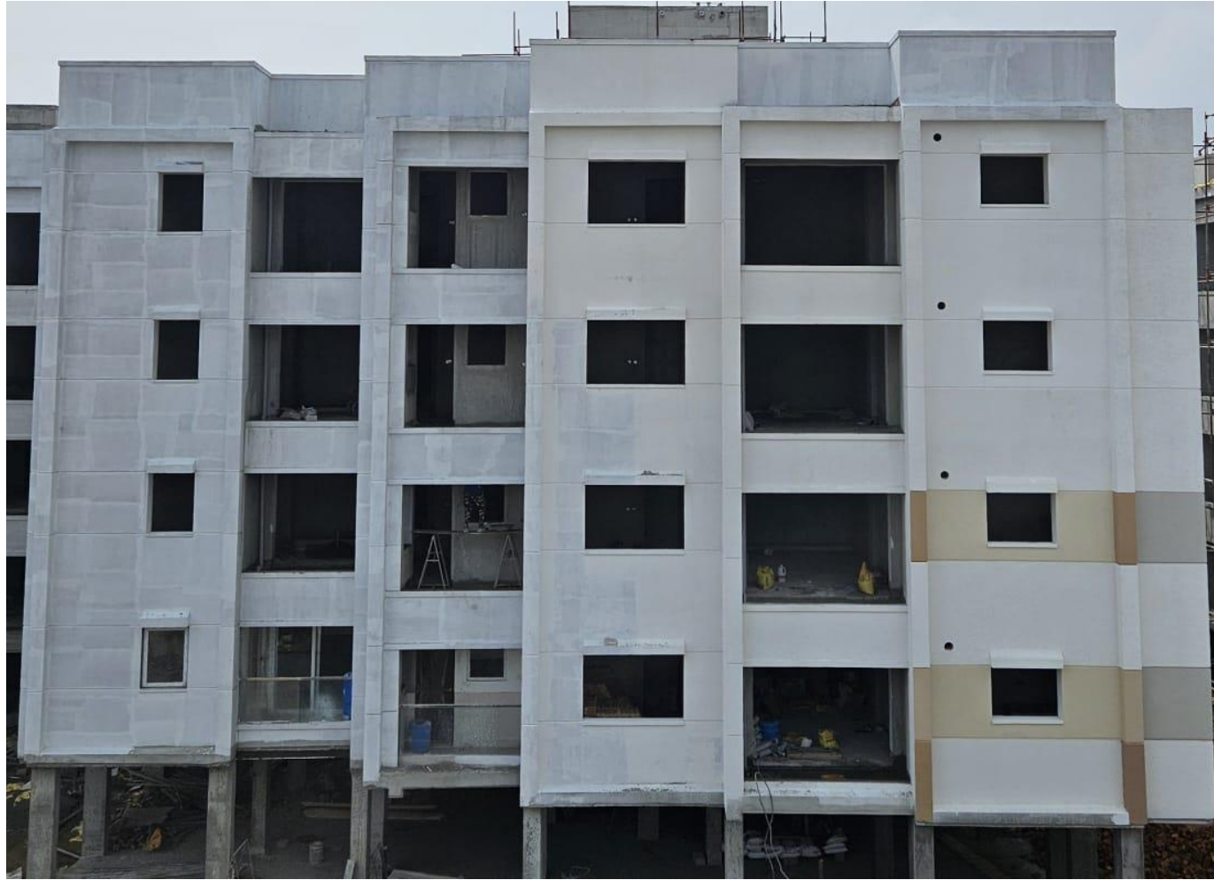
Wing 3A – North Elevation View
