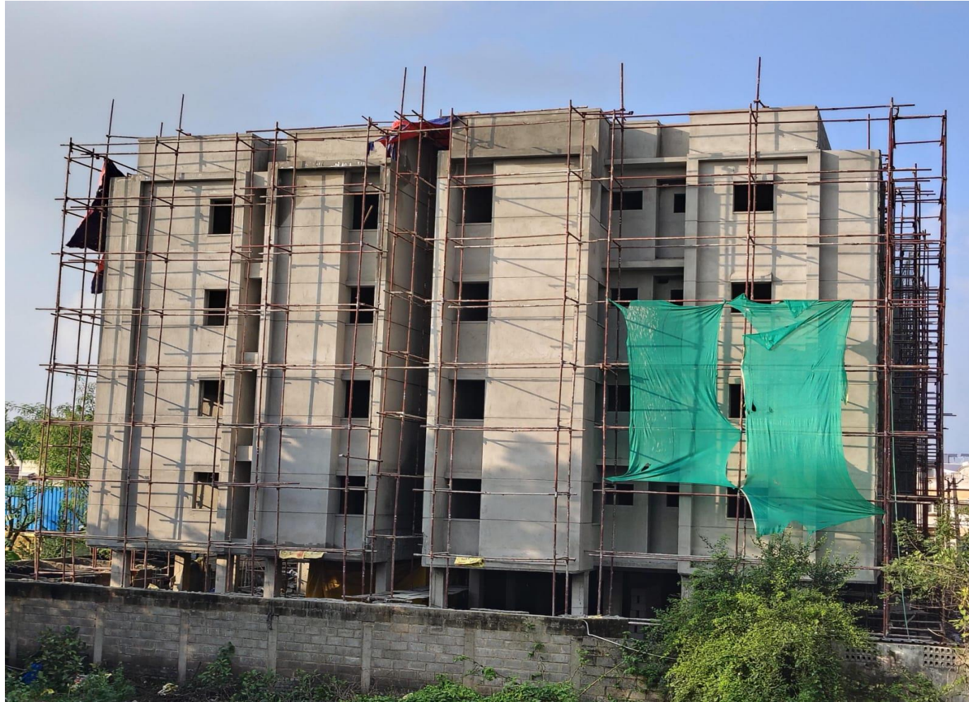
Wing 4B – South Elevation View
