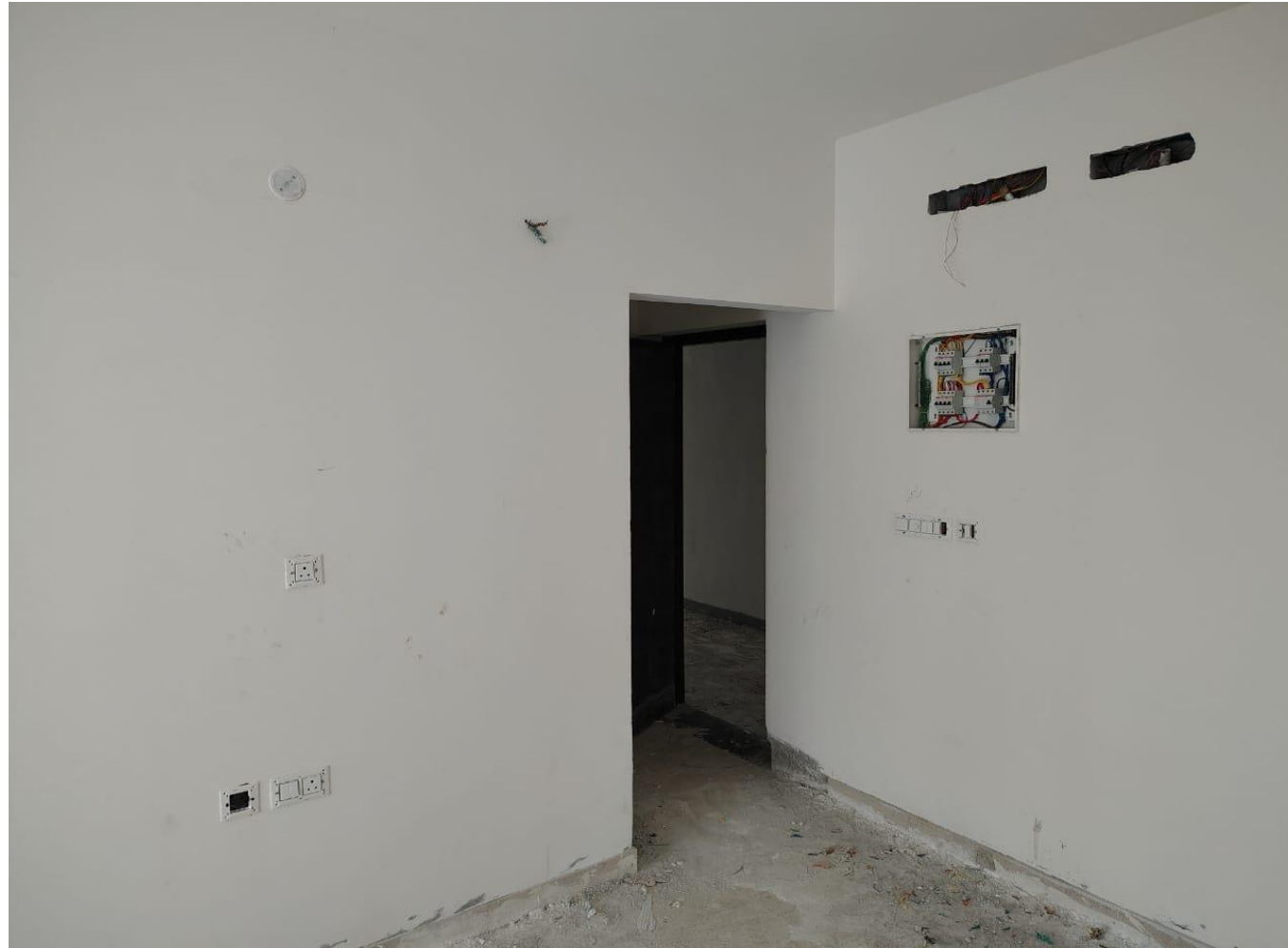
Wing 3D, 2 nd Floor – Wiring Works in Progress
