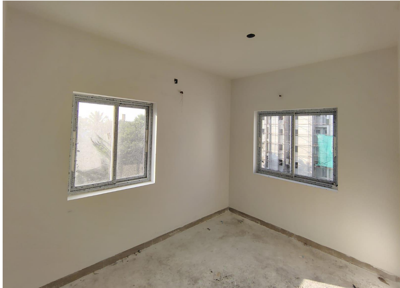
Wing 3E, 2 nd Floor – Primer Works in Progress
