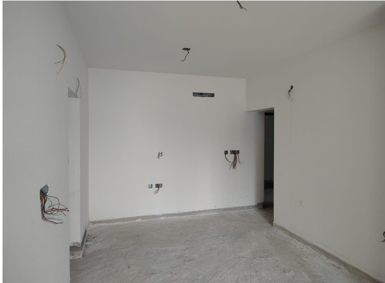
Wing 3D, 3 rd Floor– Flat Wiring Works in Progress
