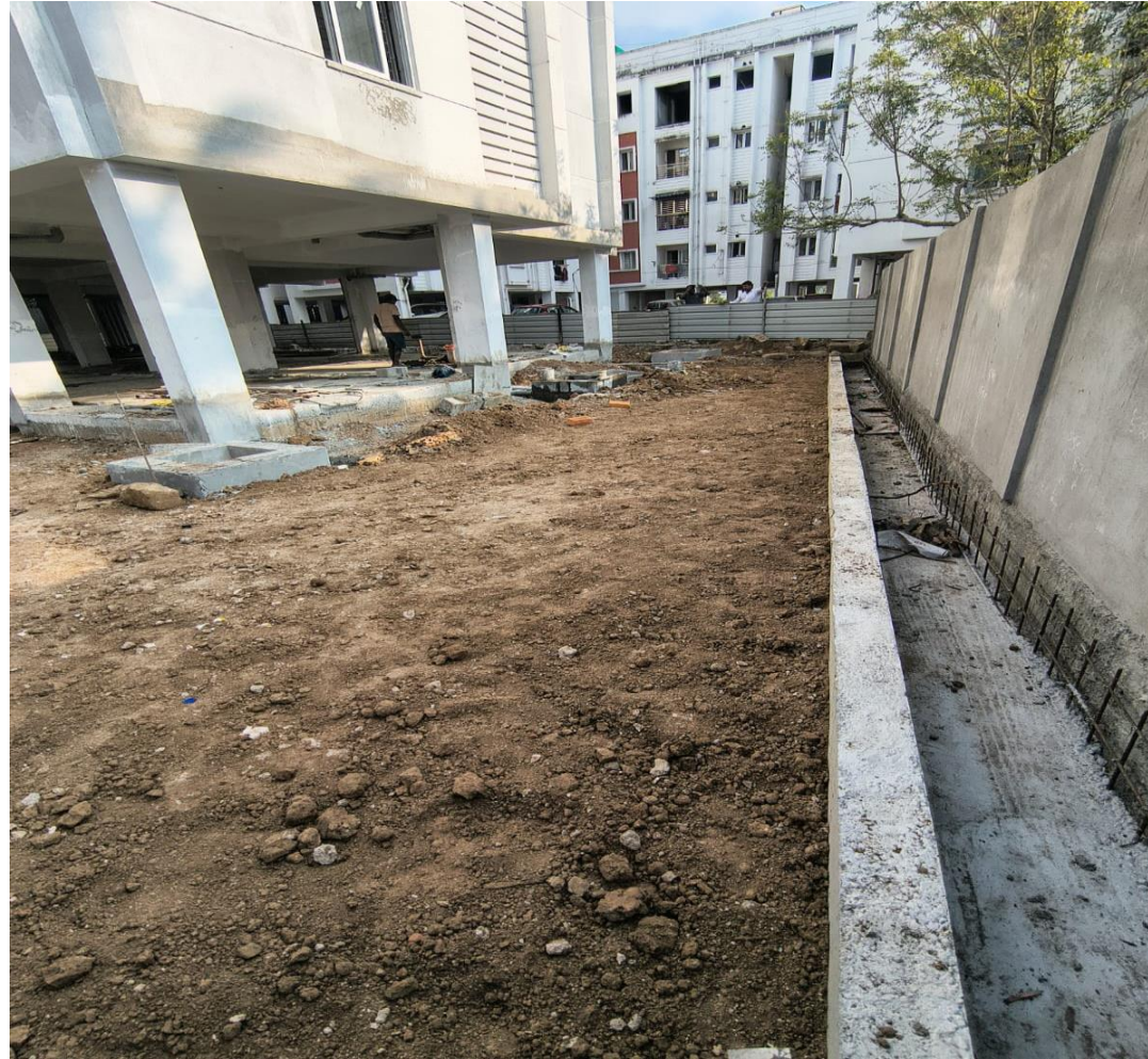
Wing 3E, External – Sub Grade Preparation Works in Progress
