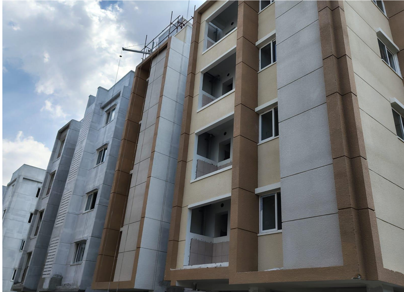
Wing 3B – East Elevation View
