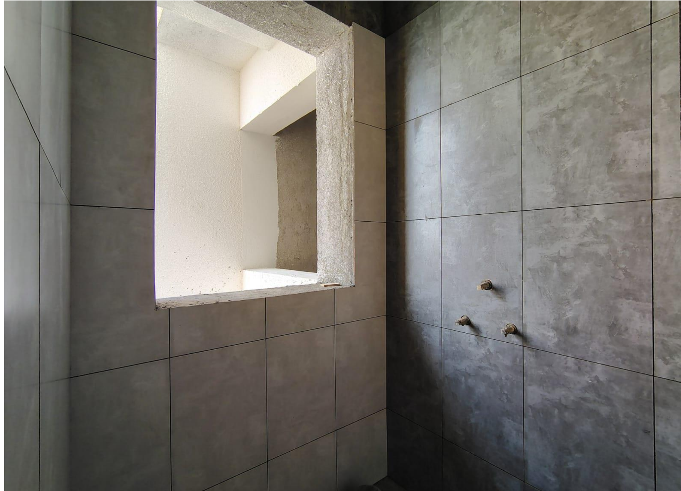
Wing 4A & 4B – Toilet Tile Work in Progress
