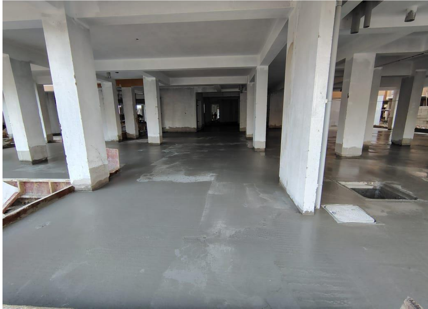
Wing 3A – Stilt Floor Screed Works in Progress
