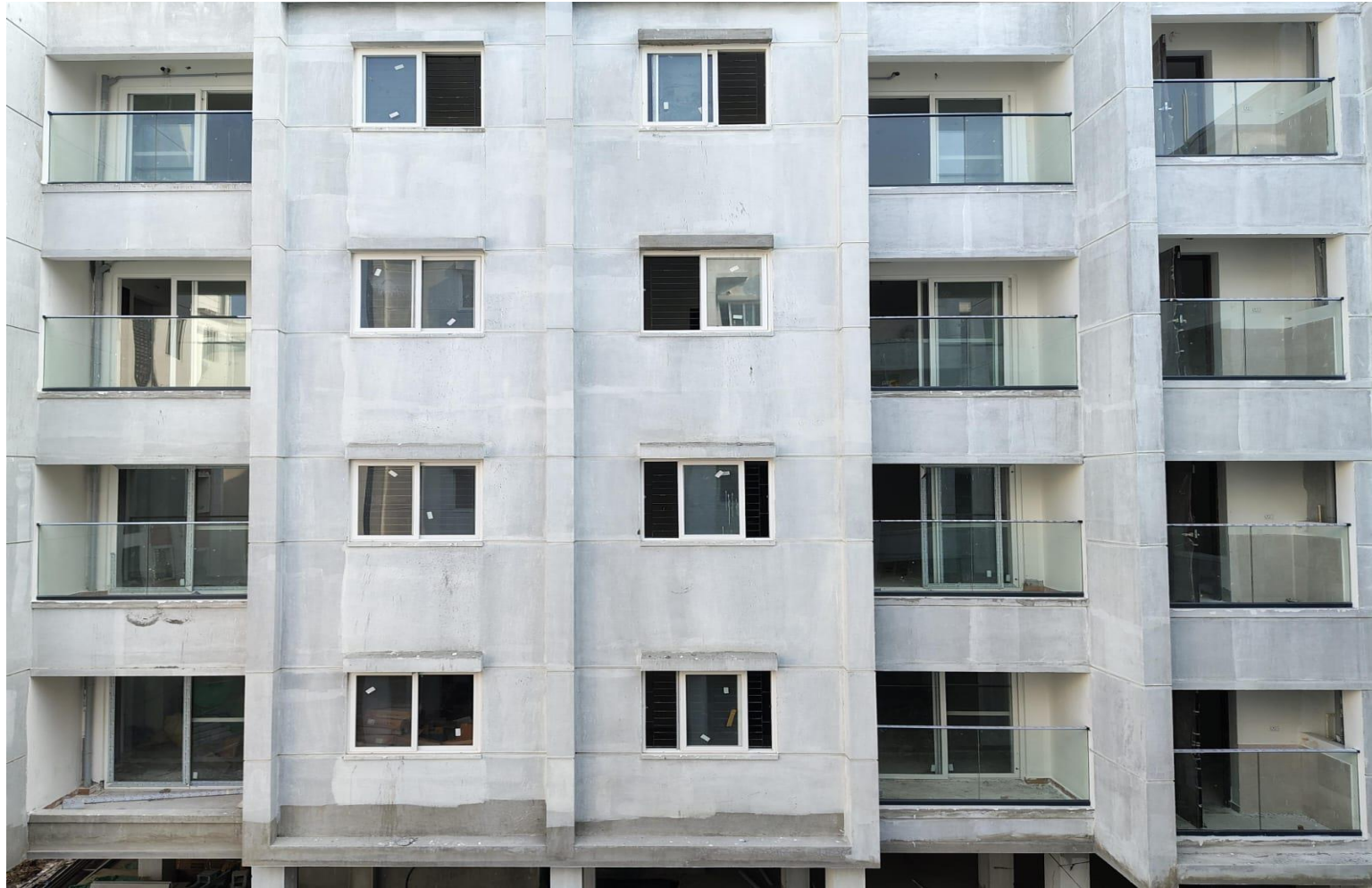
Wing 3D & 3E – Balcony & Utility Handrail Works in Progress
