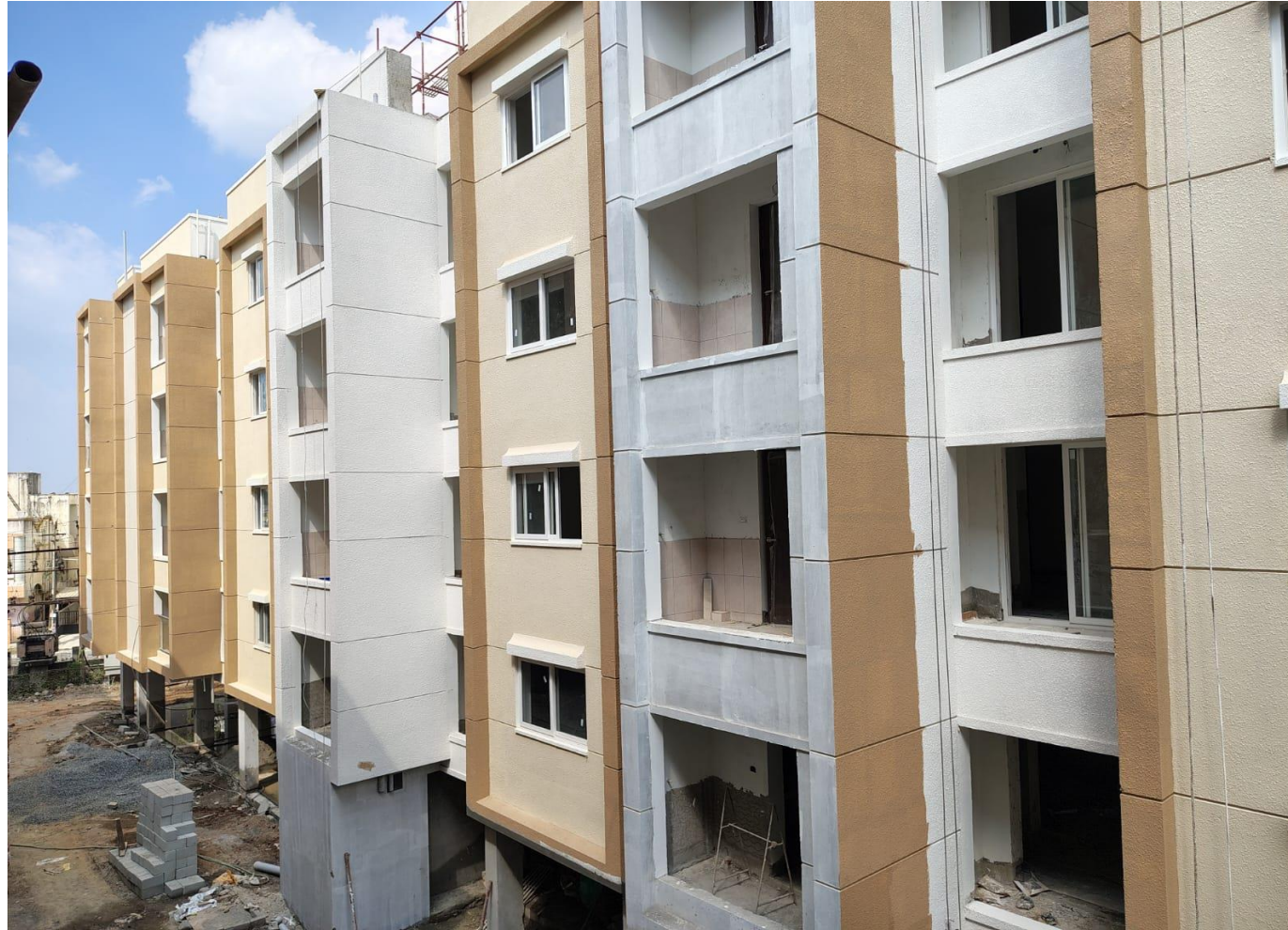
Wing 3A – West Elevation View
