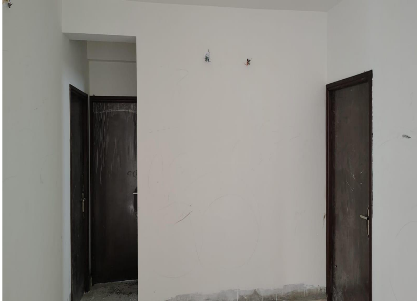
Wing 3A, 4 th Floor – Door Fixing Works in Progress
