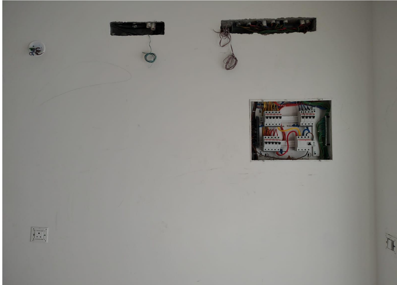
Wing 3A, 3 rd & 4 th Floor – Wiring Works in Progress
