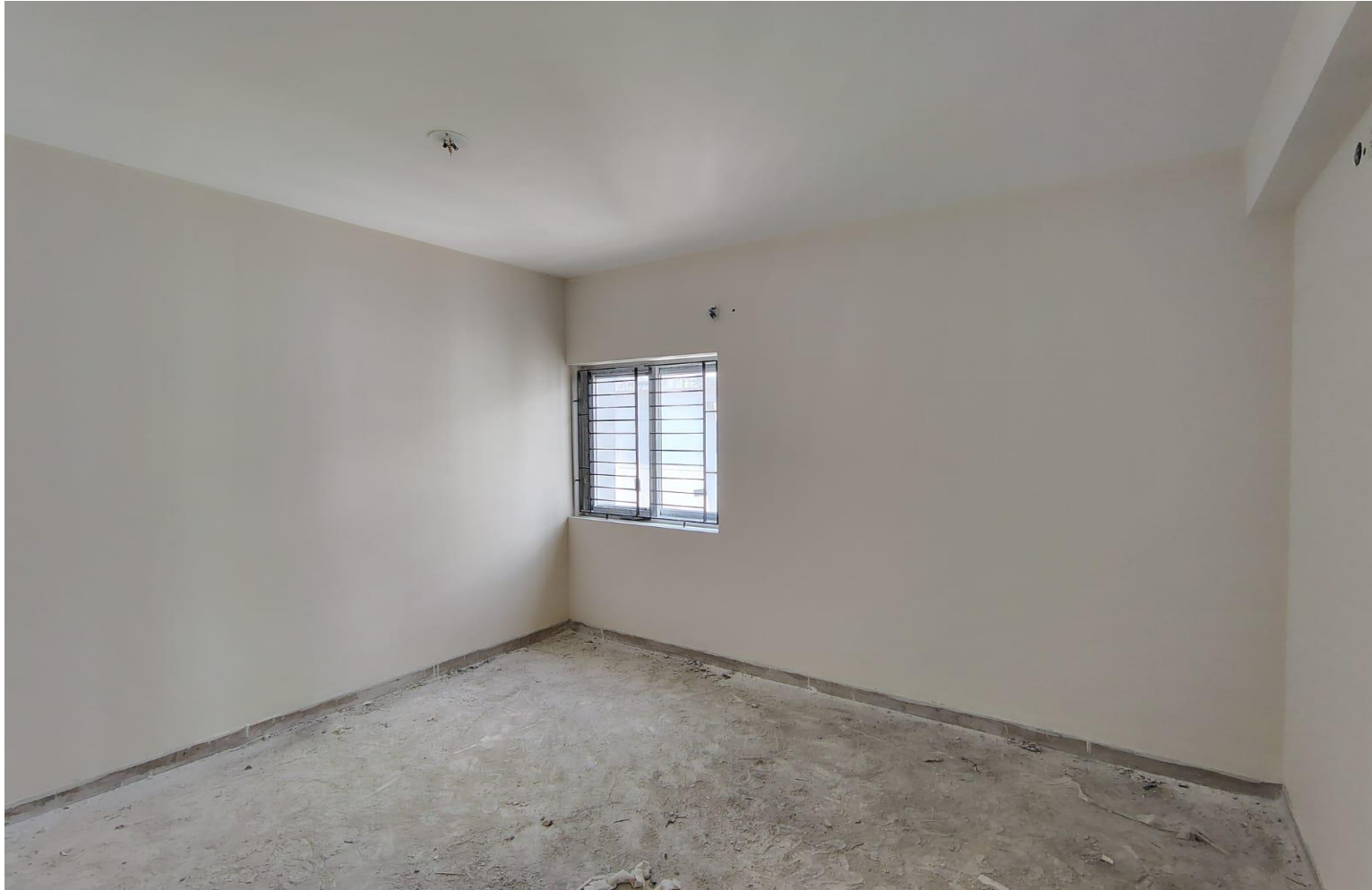
Wing 3D – 1 st Coat Paint Work in Progress
