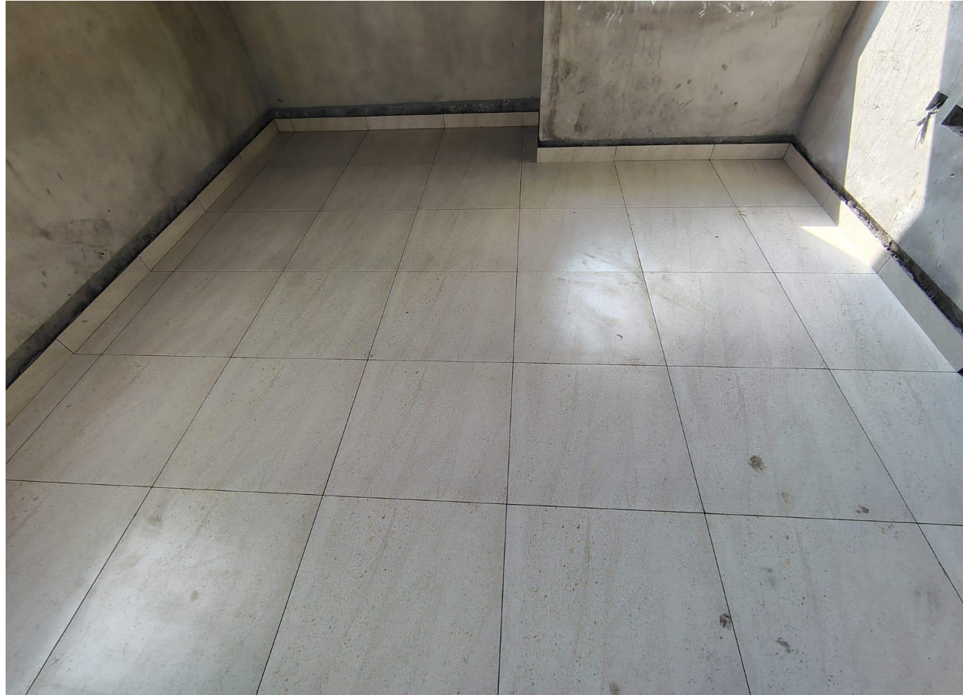
Wing 4A & 4B, 3 rd & 4 th Floor –Tile Work in Progress
