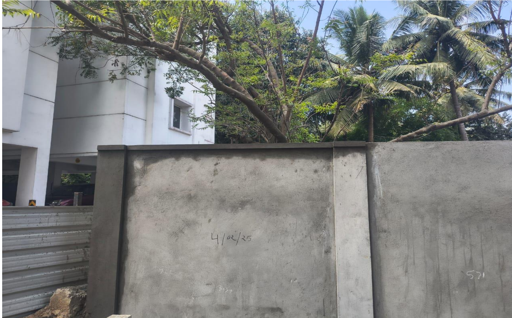
Compound Wall – Band Work in Progress
