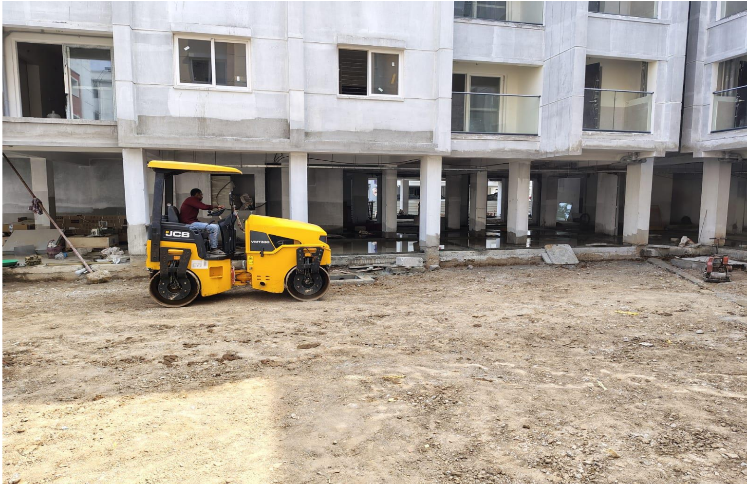
Wing 3D, External – Sub Grade Preparation Works in Progress
