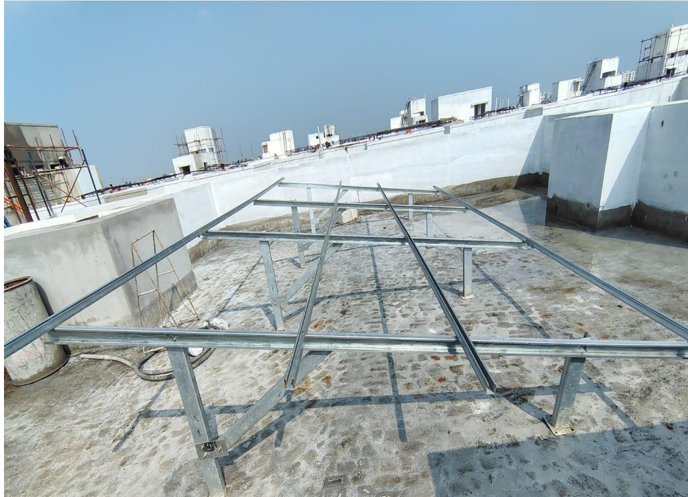
Wing 4A & 4B – Terrace Solar Panel's Framing Works in Progress
