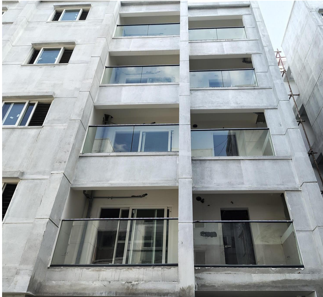
Wing 3C, Balcony & Utility – Handrail Work in Progress
