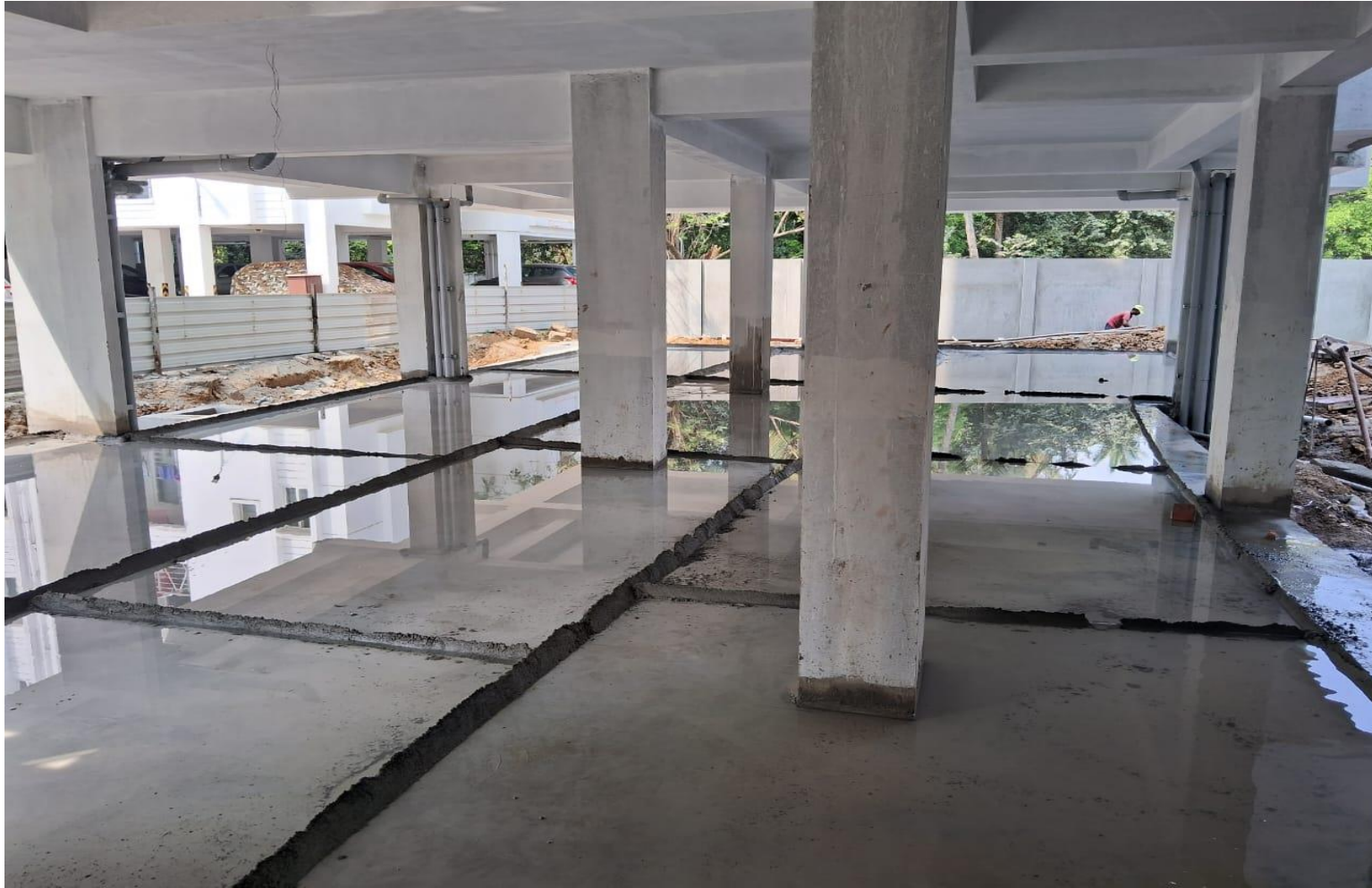
Wing 3D & 3E – Screed Works in Progress
