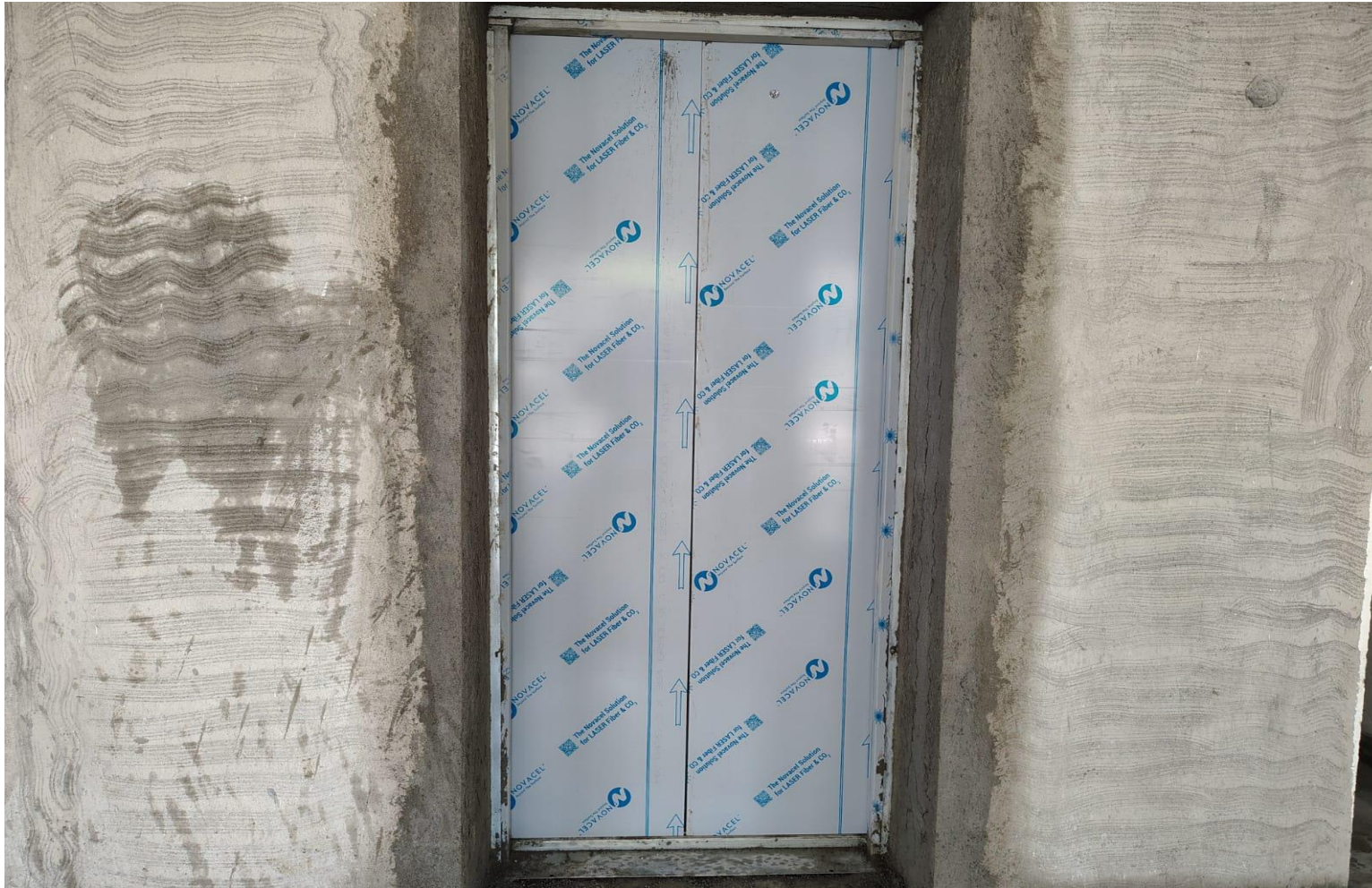
Wing 3D – Lift Installation Works in Progress
