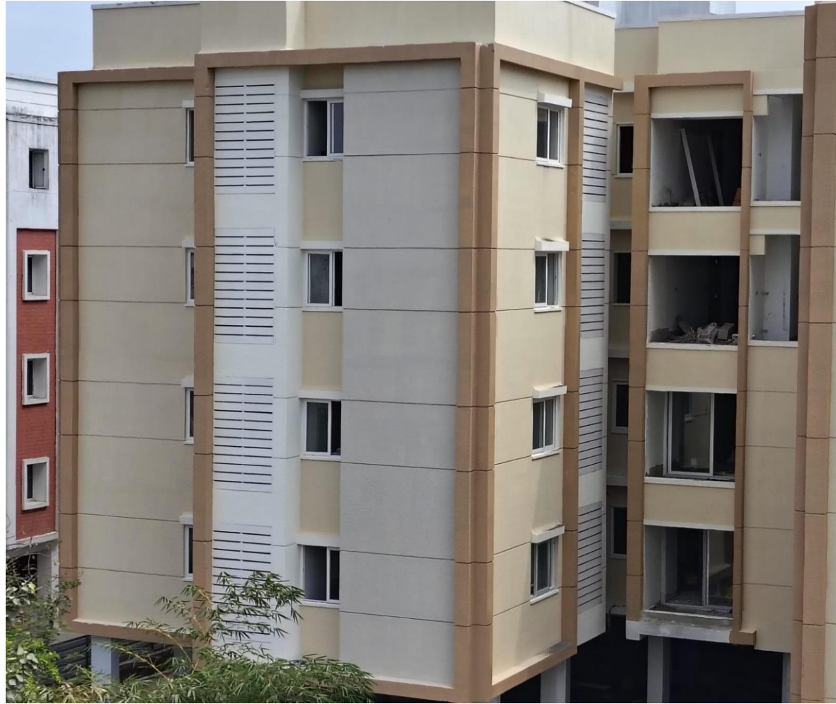
Wing 3B – North Elevation View
