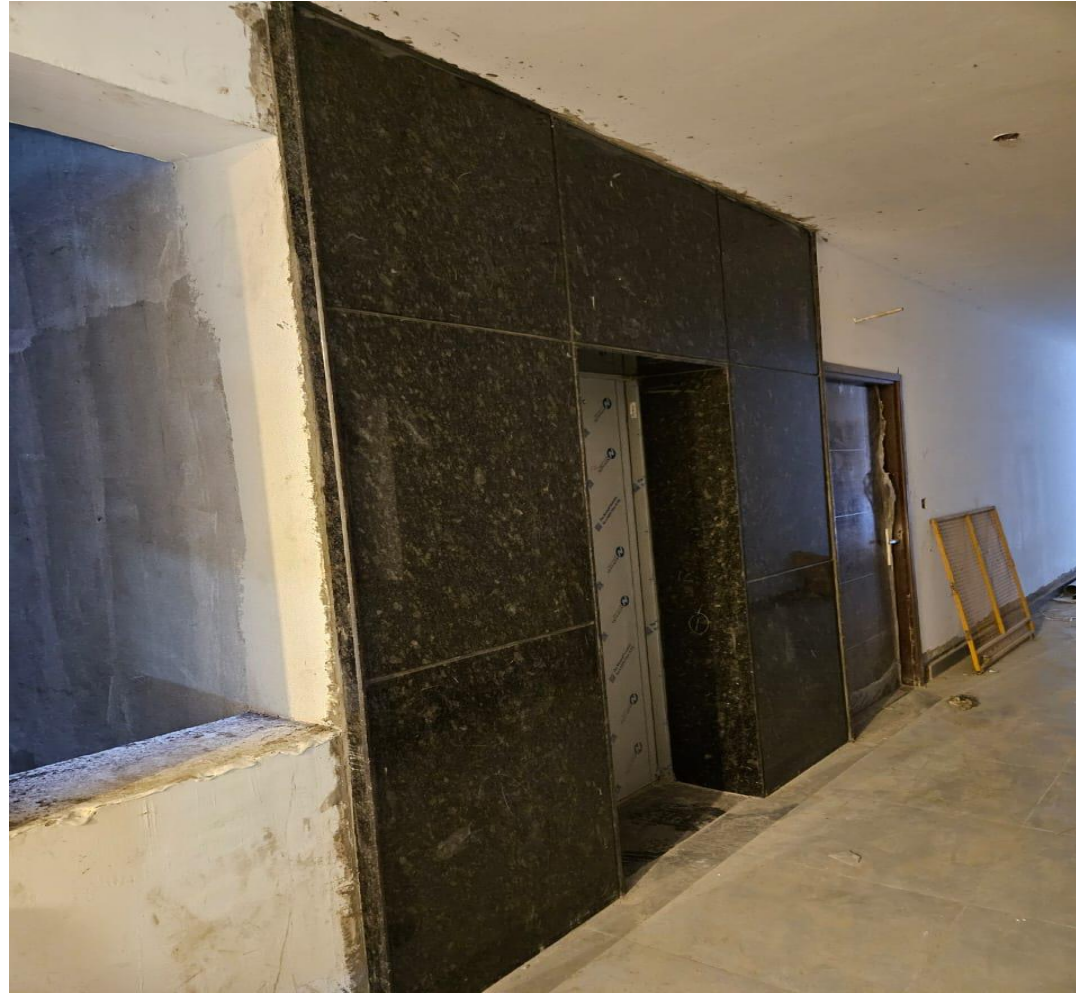
Wing 3A – Lift Granite Cladding Works in Progress
