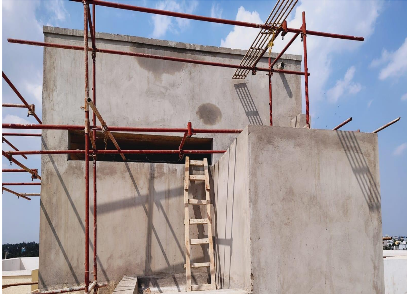
Wing 4A & 4B –OHT Plastering Works in Progress
