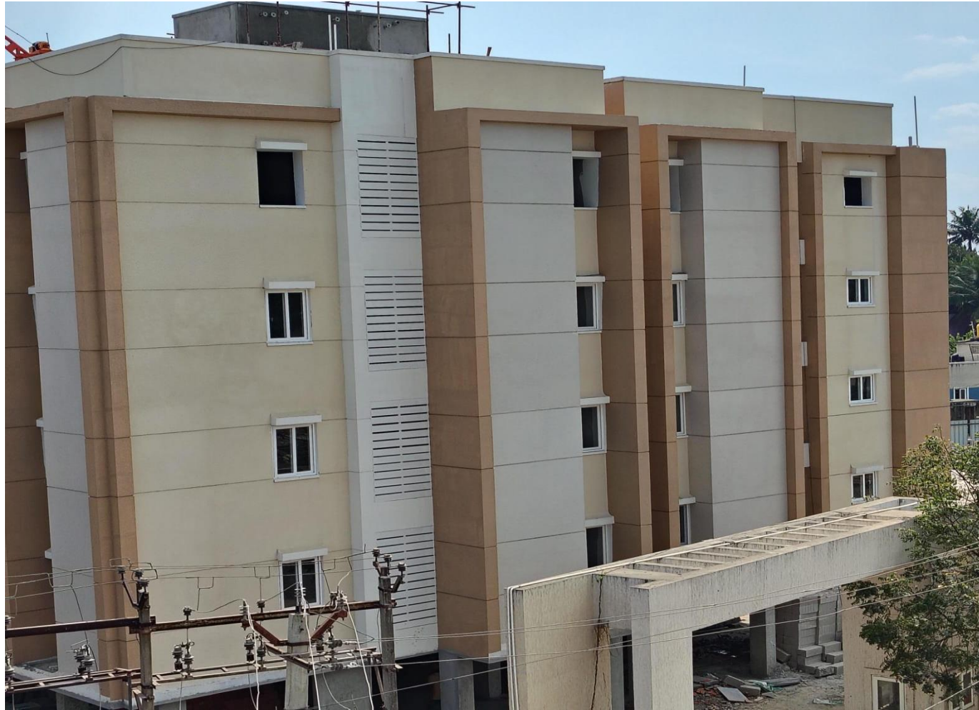
Wing 4A – North Elevation View
