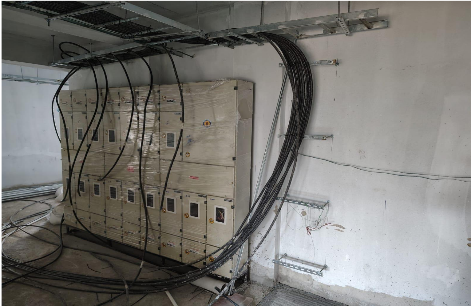
Wing 3C – Meter Panel Work in Progress
