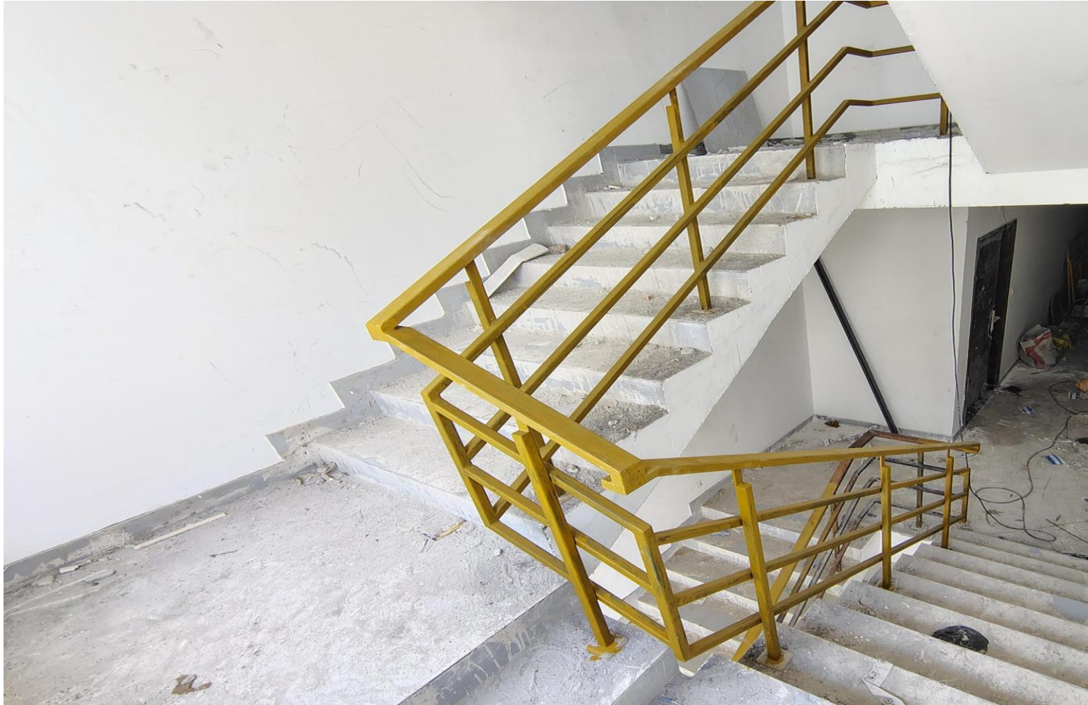
Wing 3D – Staircase Handrail Works in Progress
