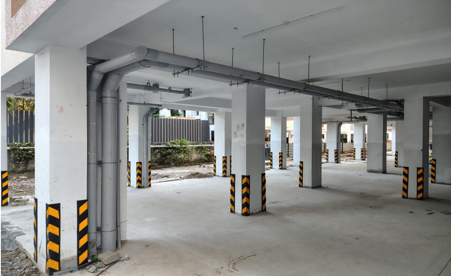
Block -3D & 3E Stilt Floor Column Guard Fixing Work In Progress
