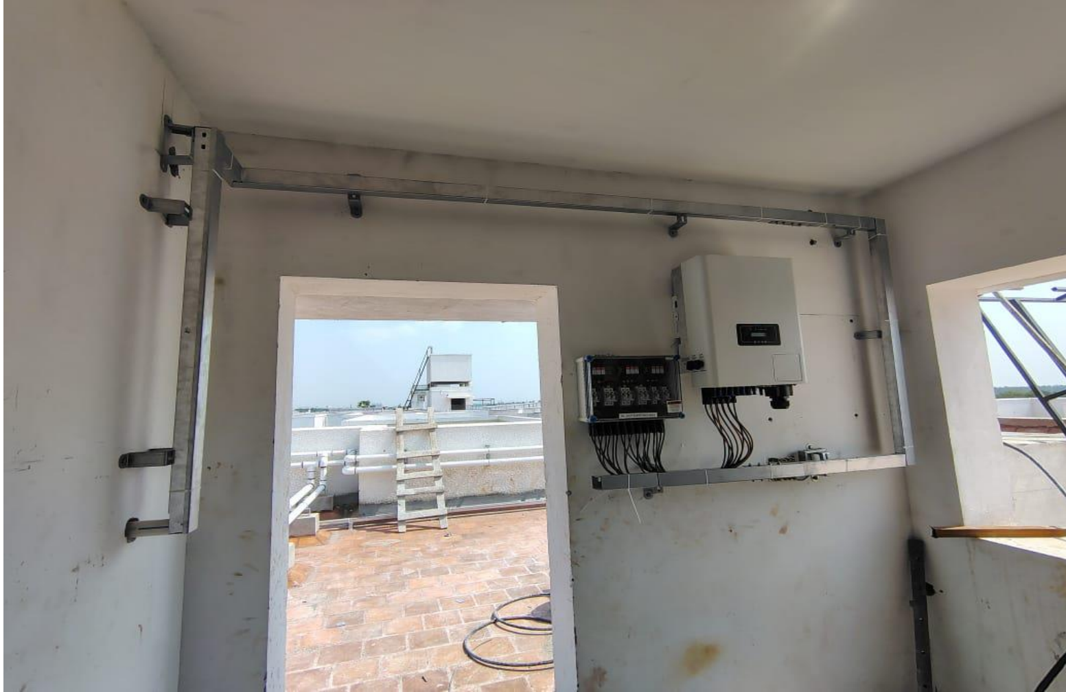
Block 3 & 4 Solar Inverter & Wiring Work In progress
