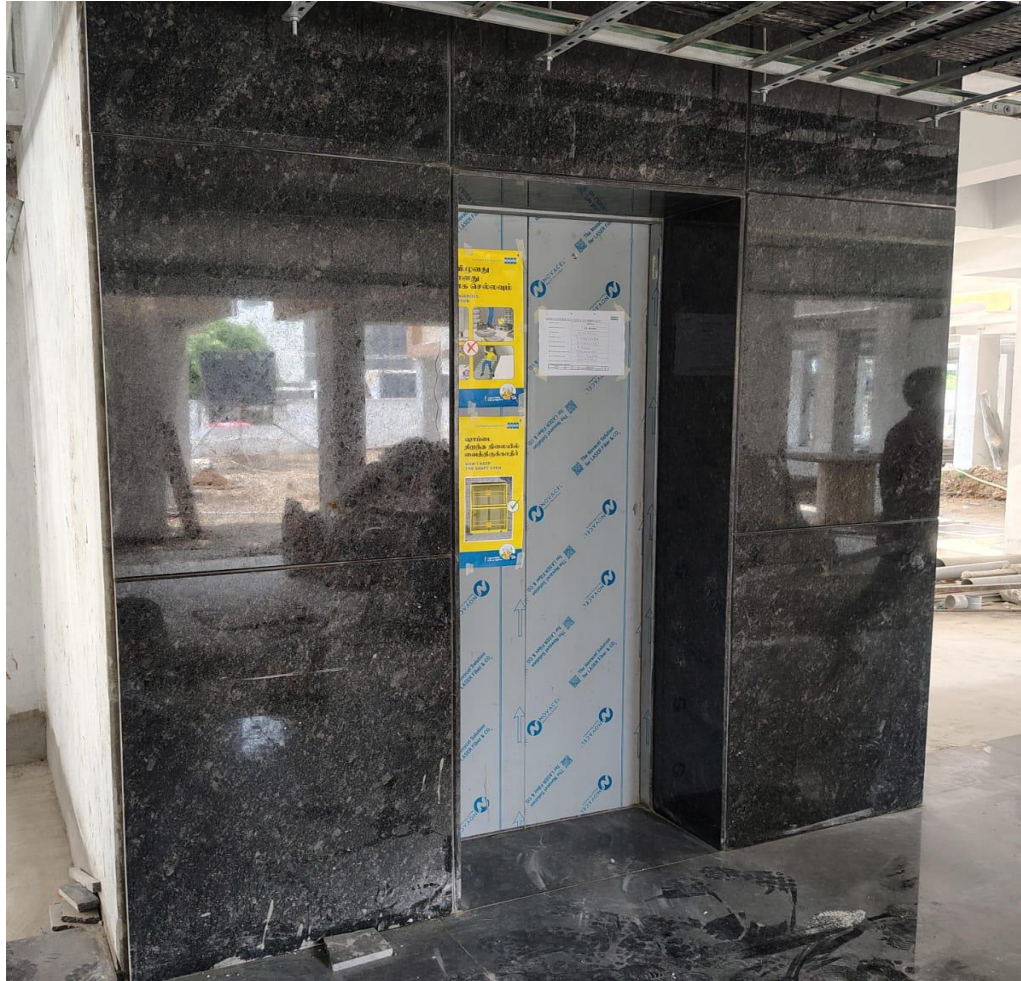
Wing 3B, 3C & 3D Stilt Floor – Lobby Granite Works in Progress
