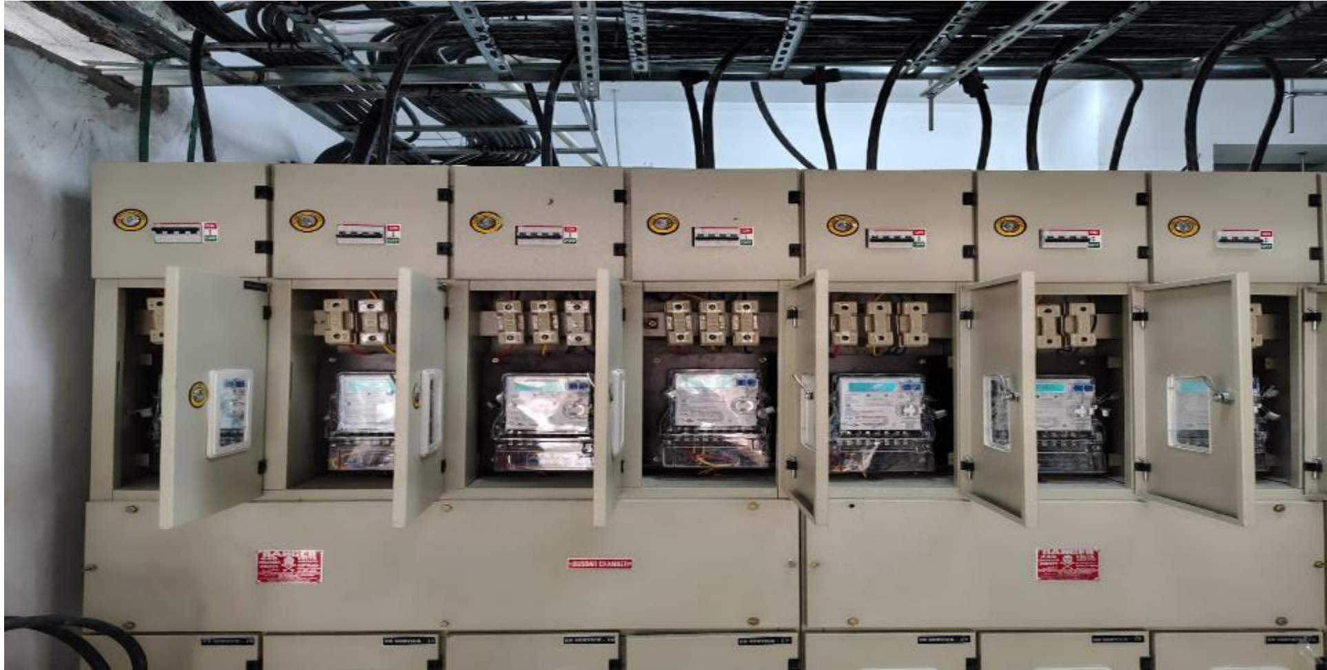
Block -3 & 4 EB Meter Installation & Termination Work Completed
