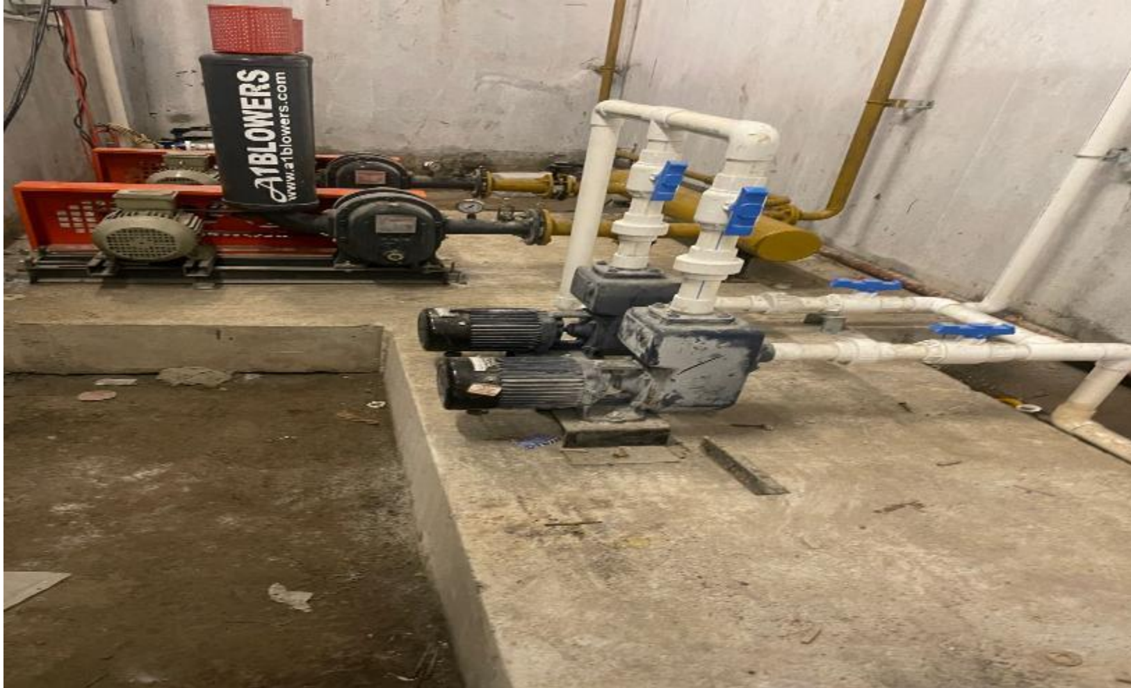
STP Pump Erection Work In progress
