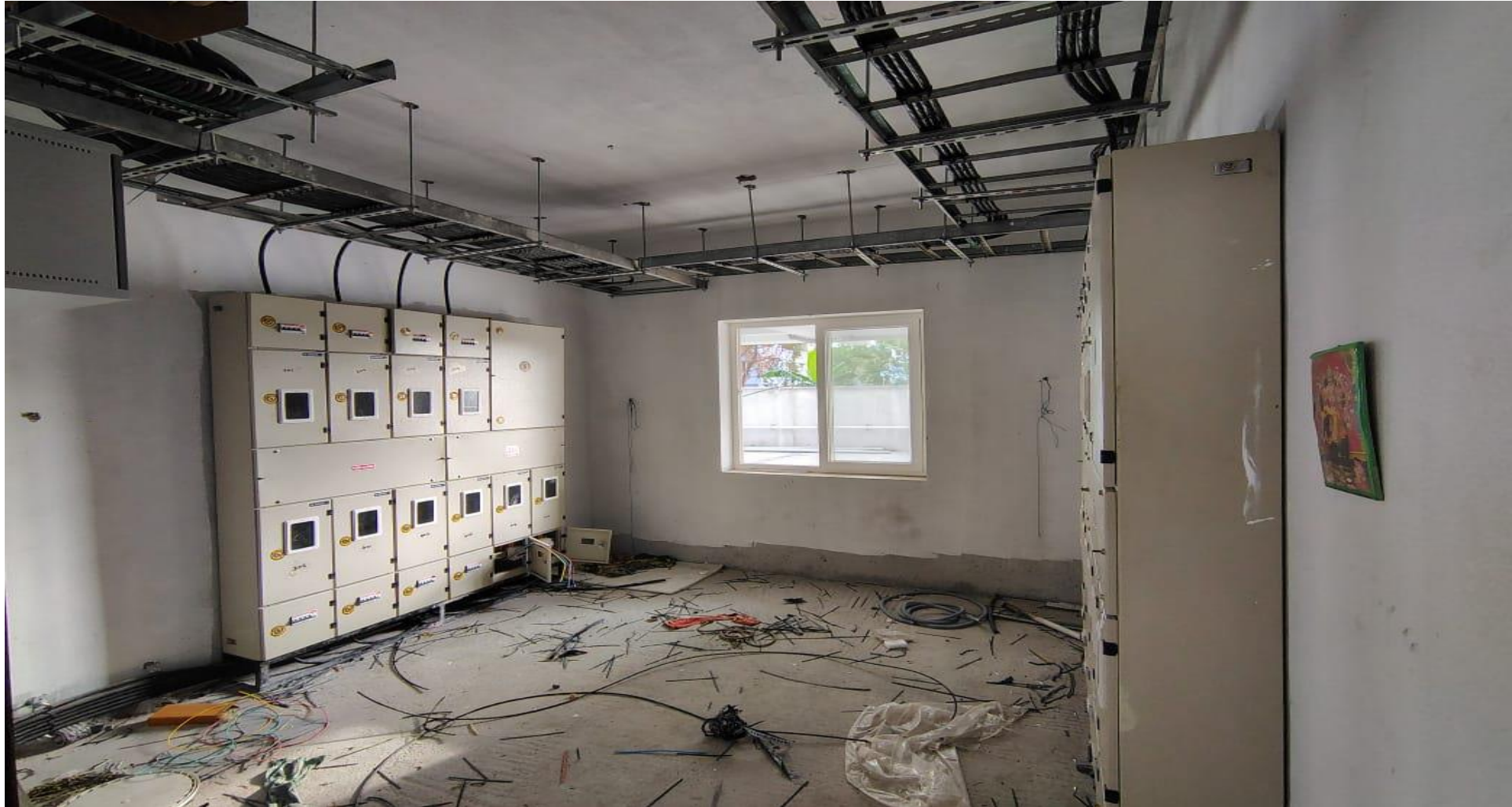
Wing 4A & 4B – Meter Panel Board Installation & Wiring Work In progress
