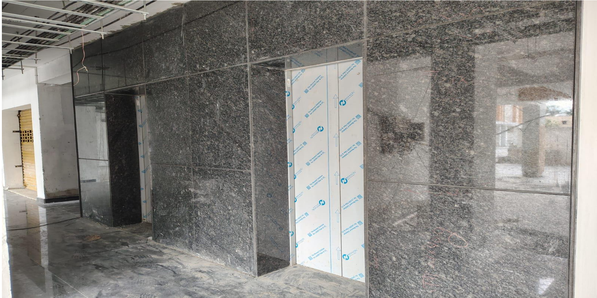
Wing 3A & 3C Stilt Floor – Lobby Granite & Lift Cladding Works in Progress
