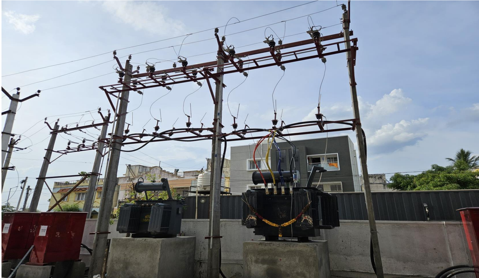
Transformer & Pillar Box Erection Work In Progress
