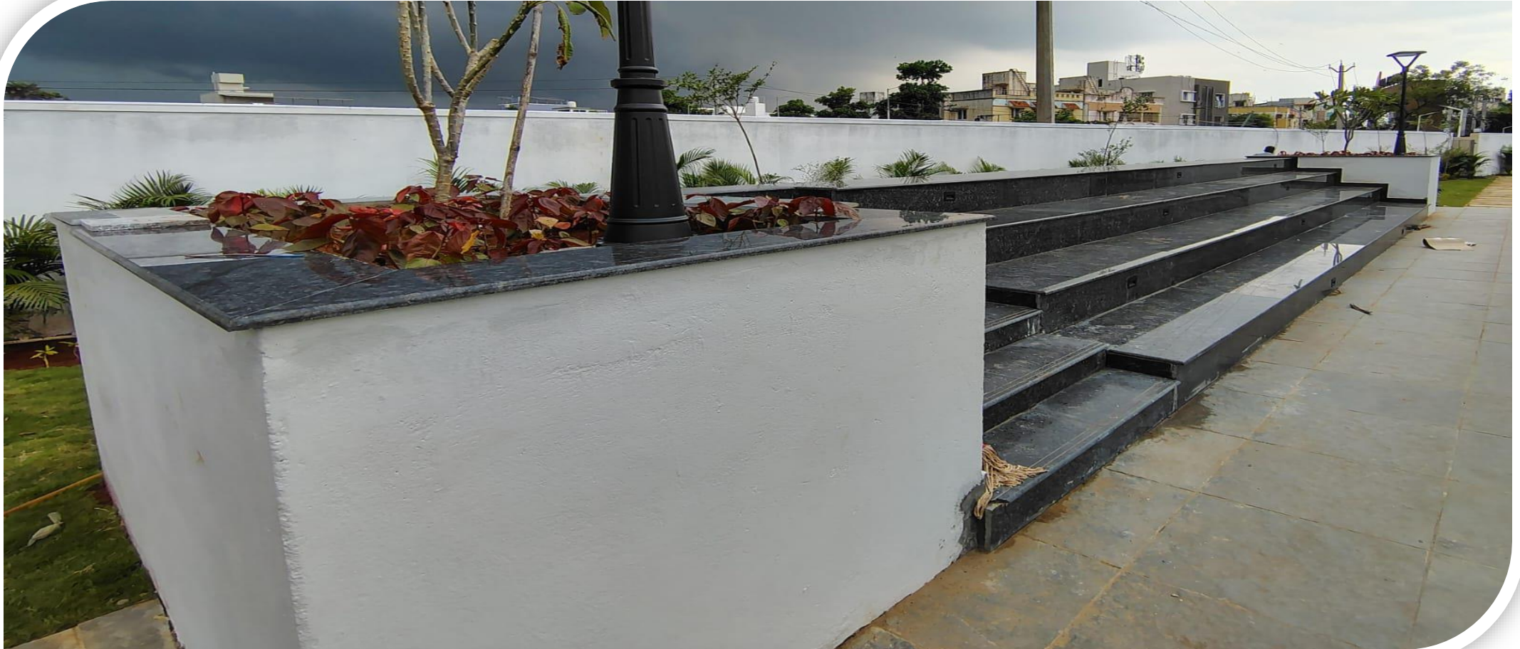
OSR – Amphitheatre Work Completed
