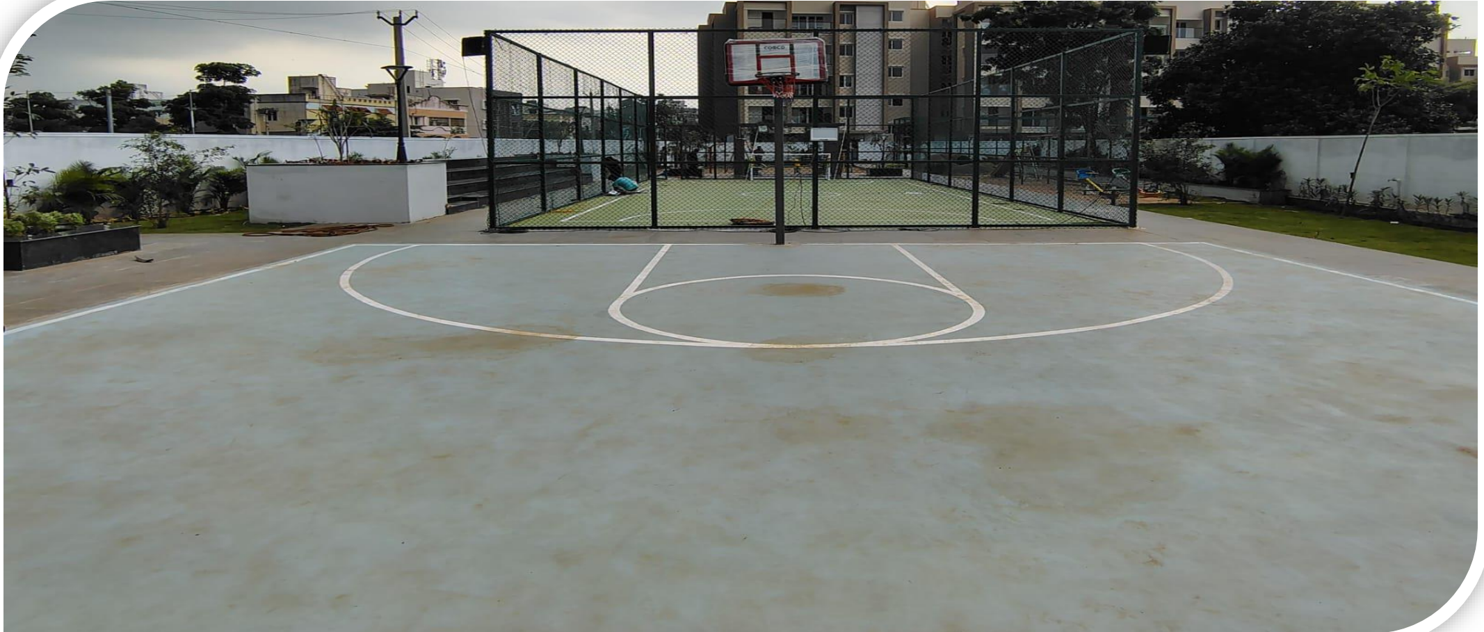
OSR – Basketball Court Completed
