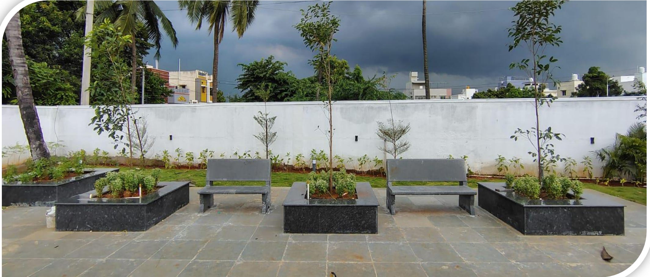
OSR – Seater & Planter Box Work Completed
