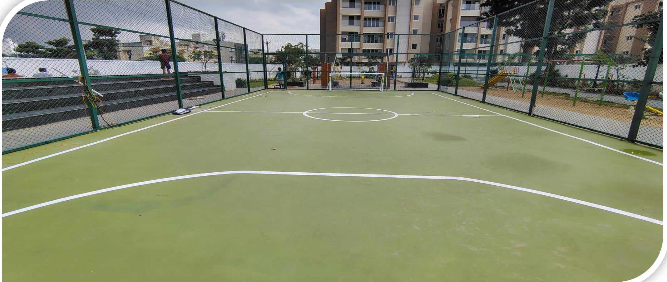
OSR – Football Court Completed
