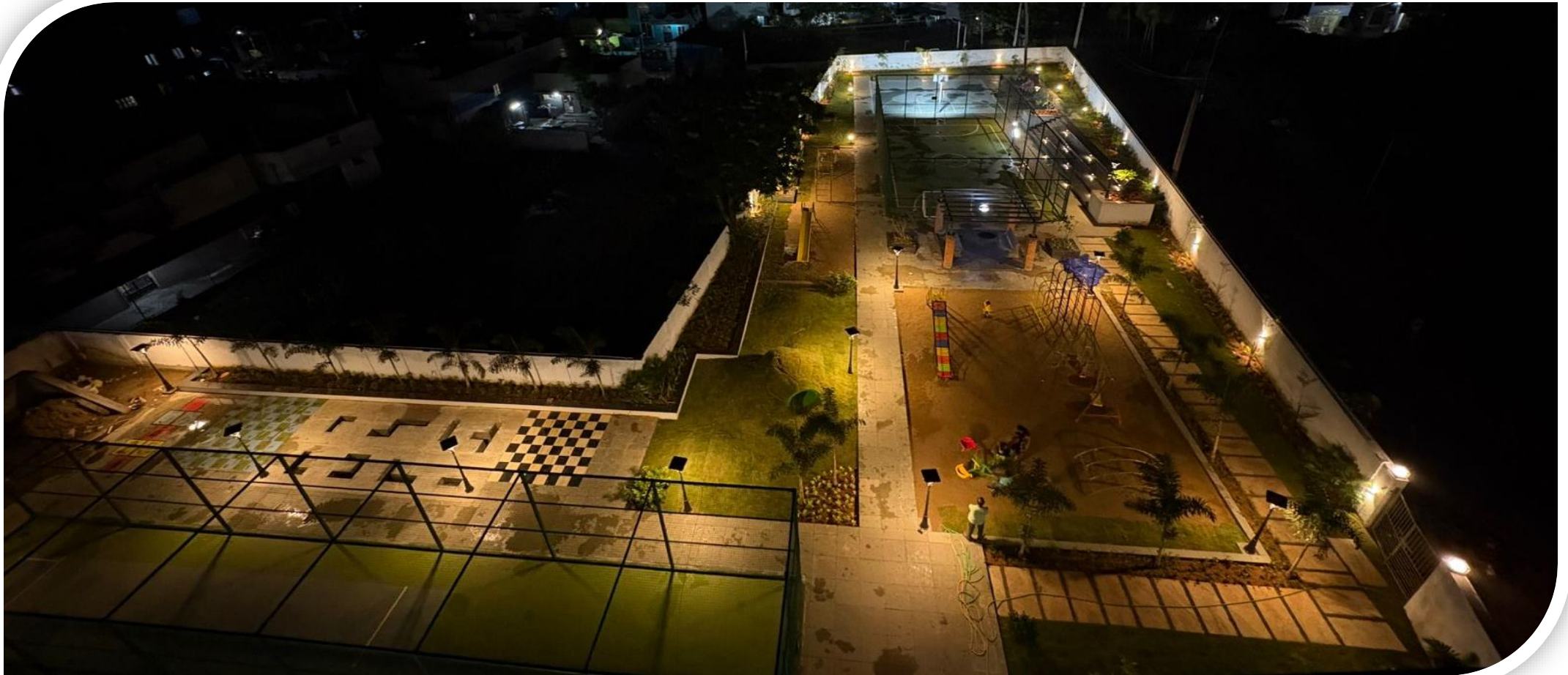
OSR – Lighting Work Completed
