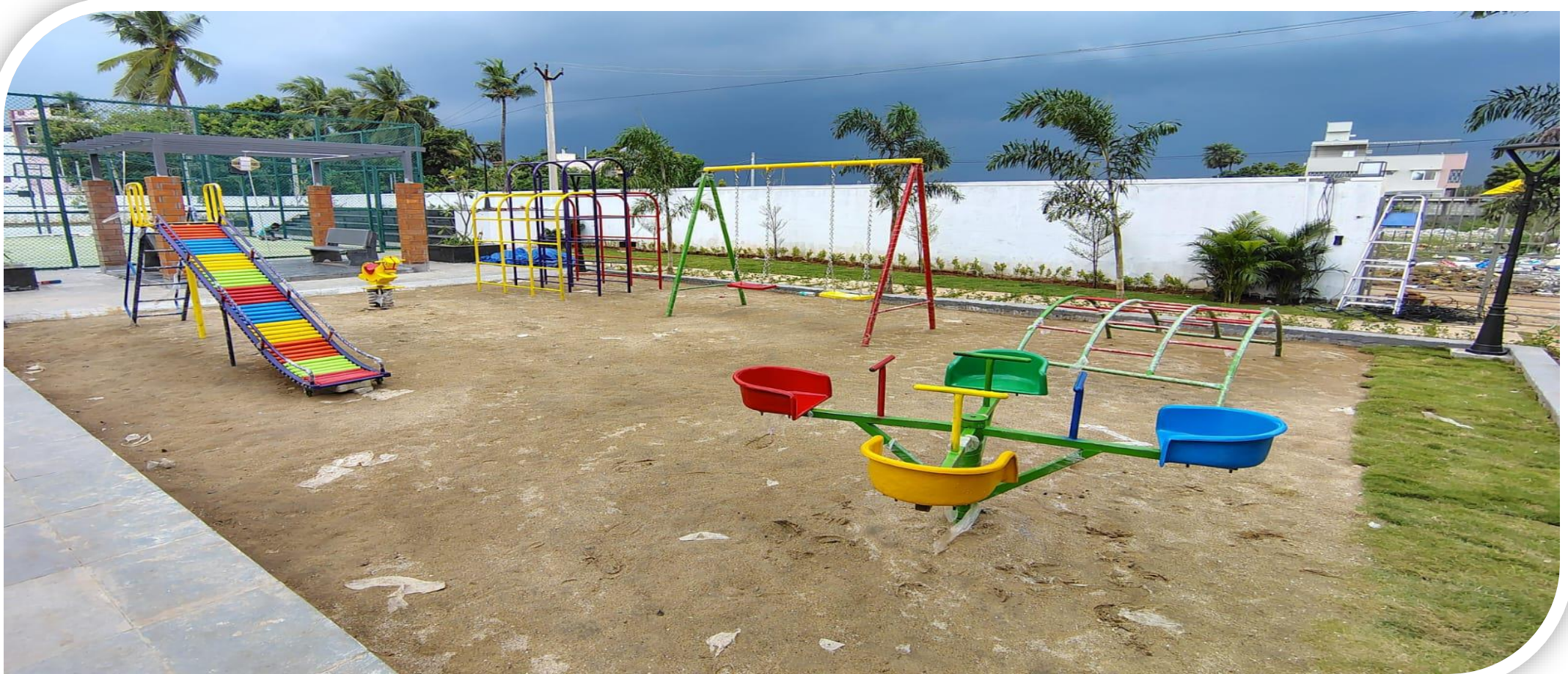
OSR – Kids Play Equipment Installation Work Completed
