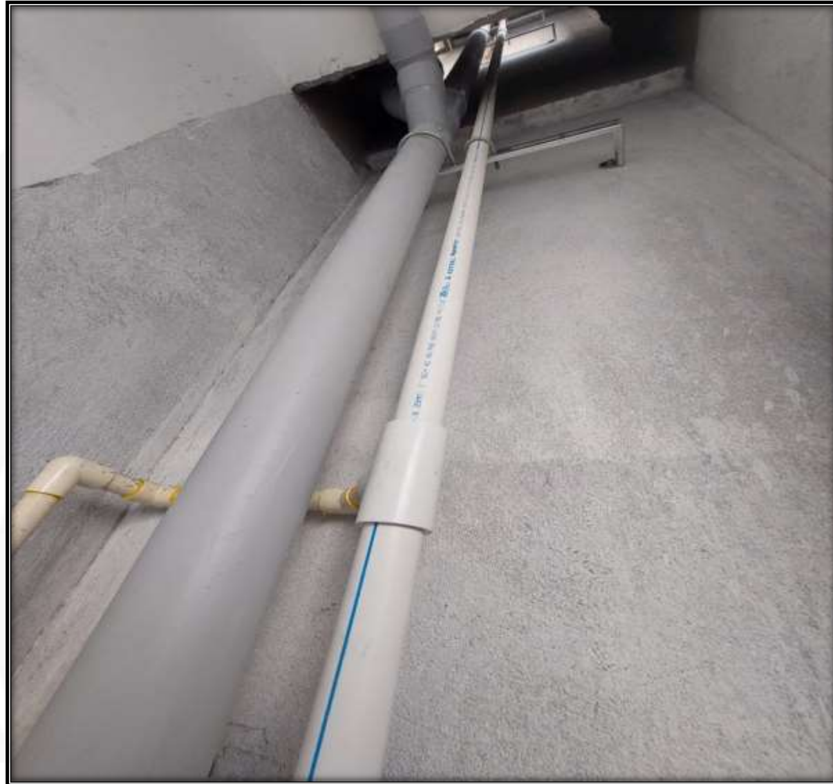
Wing 3D – Utility Shaft Plumbing Works in Progress
