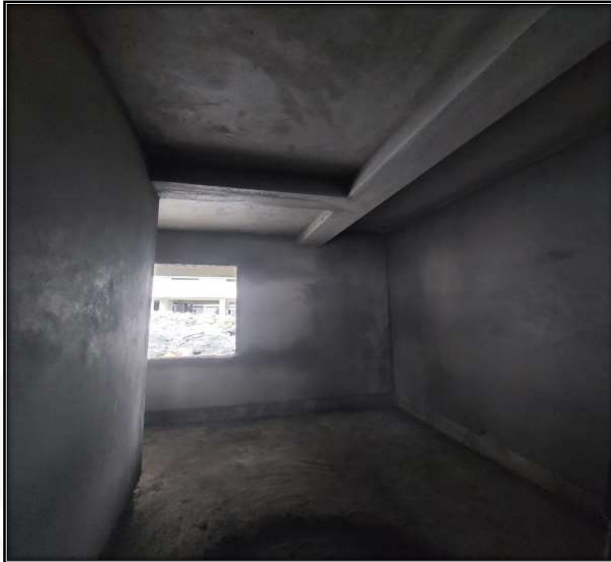
Wing 3D – EB Room Plastering Work in Progress
