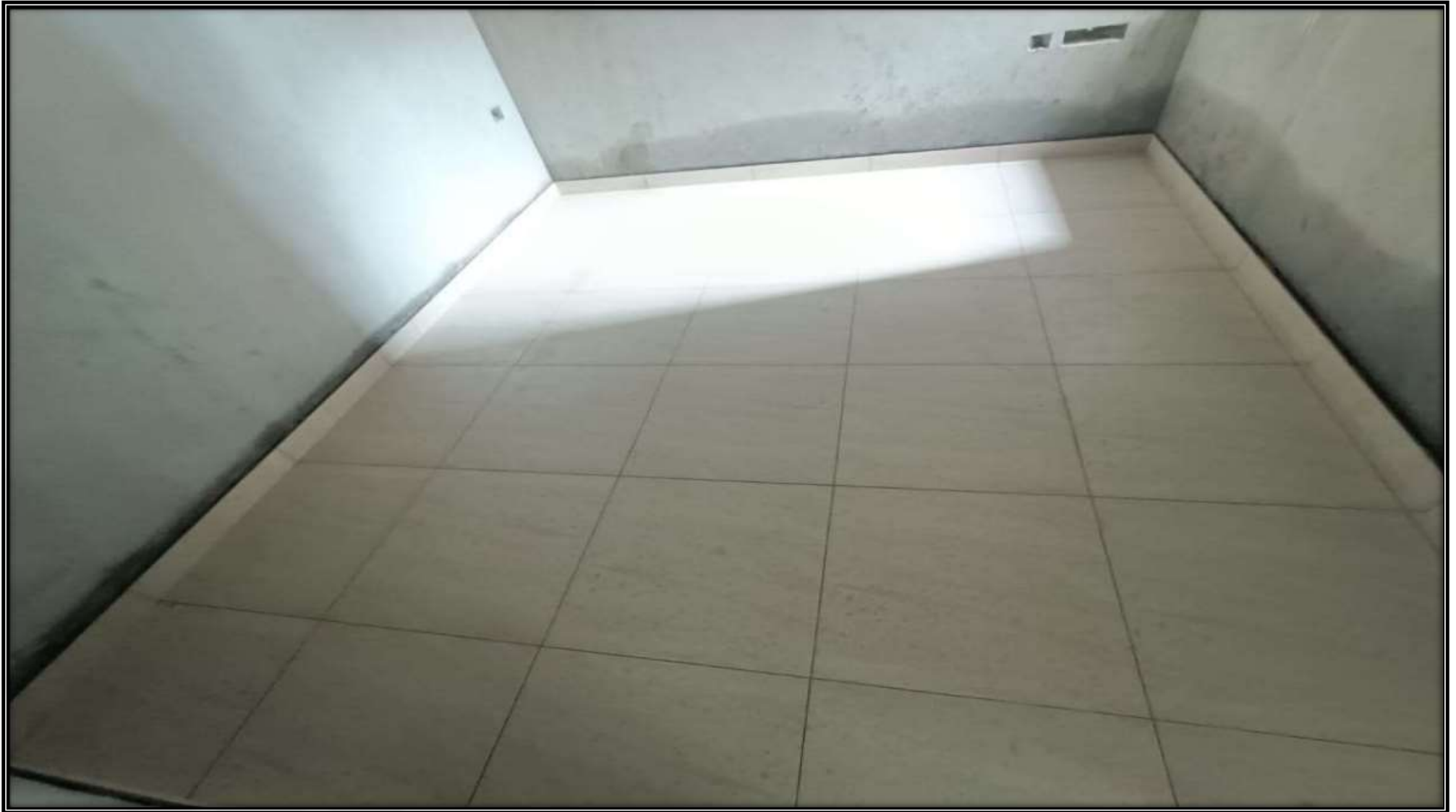
Wing 3C, 4 th Floor – Floor Tile Works in Progress
