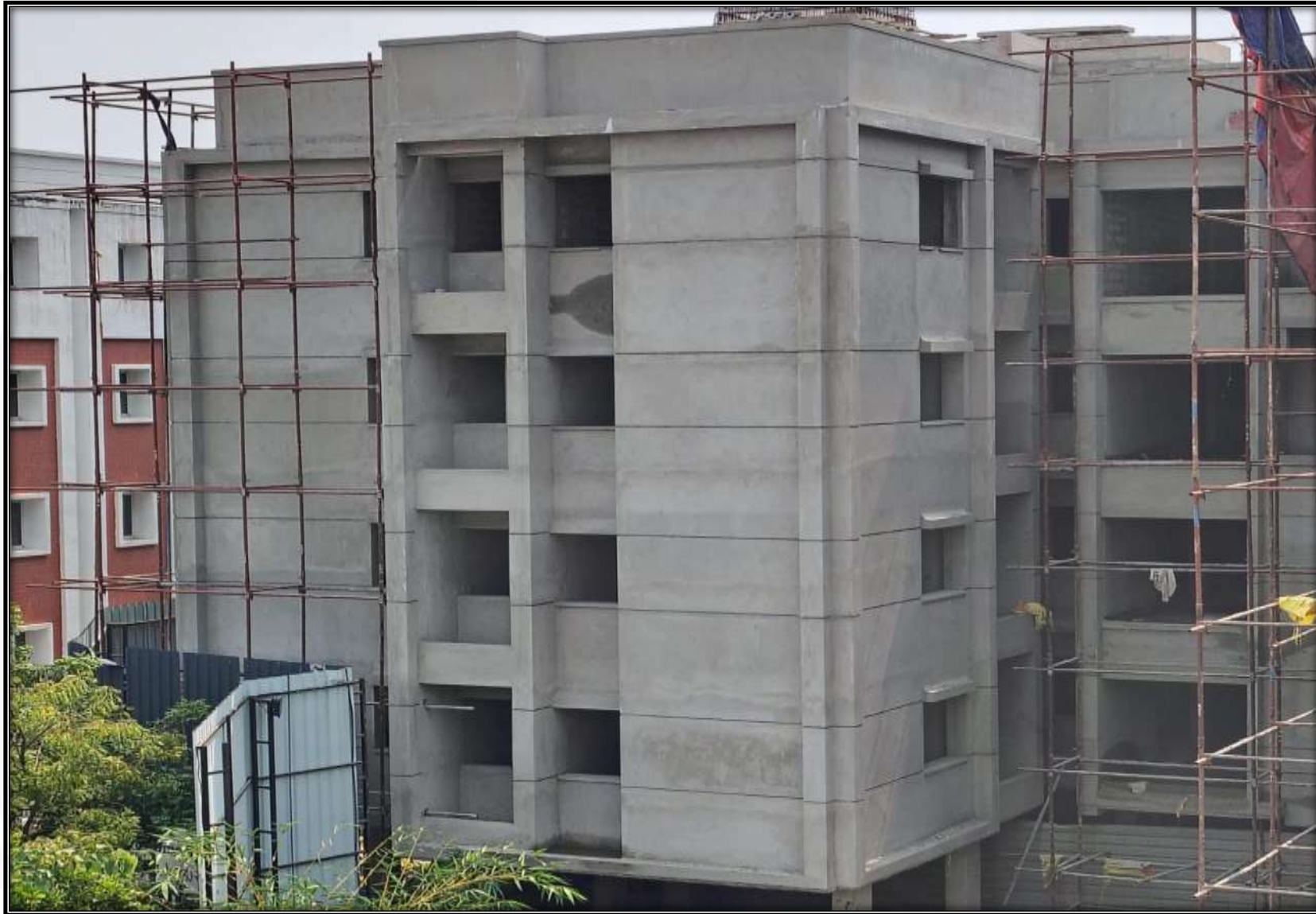
Wing 3B – North Elevation View
