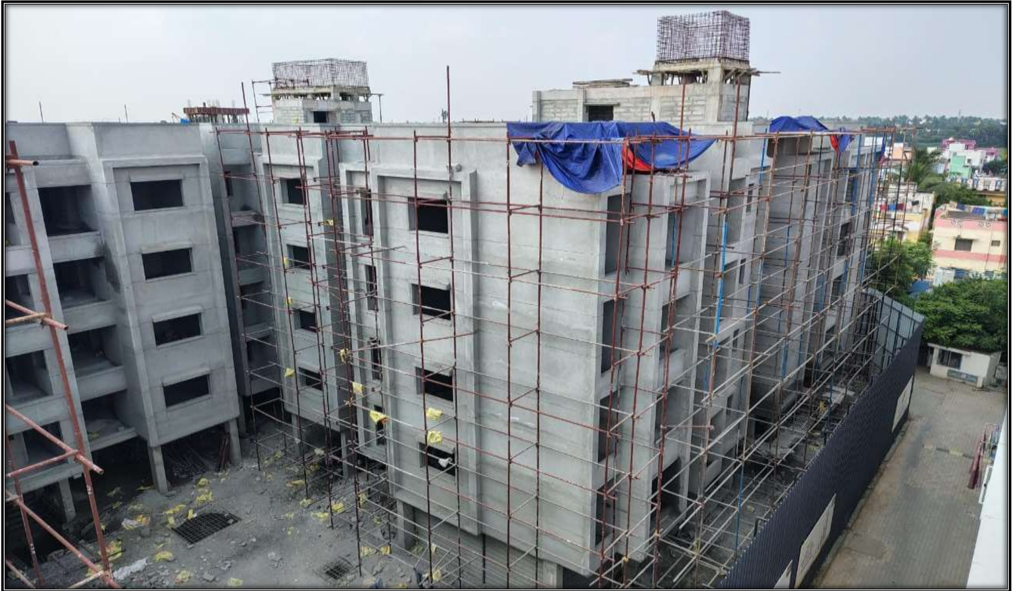
Wing 3B – South & East Elevation View
