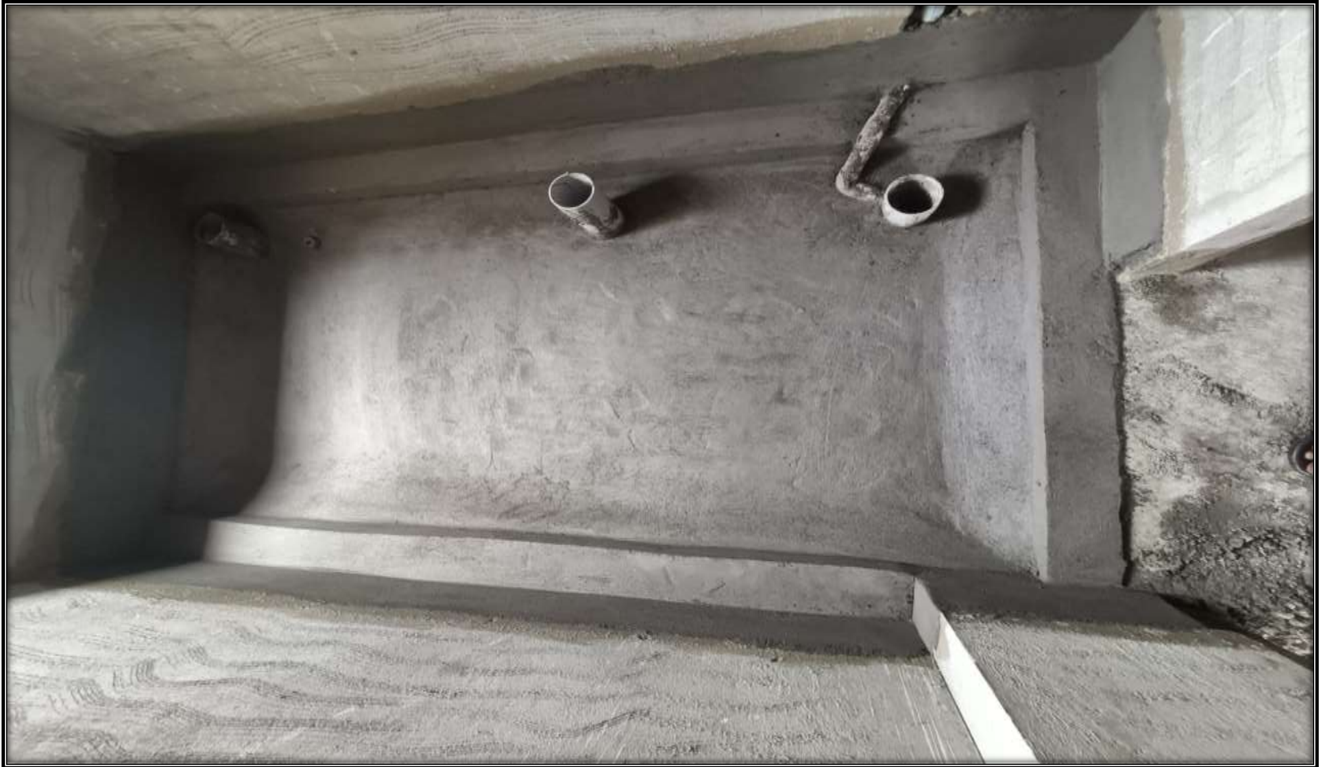
Wing 3A, 3 rd Floor – Sunken Water Proofing Works in Progress
