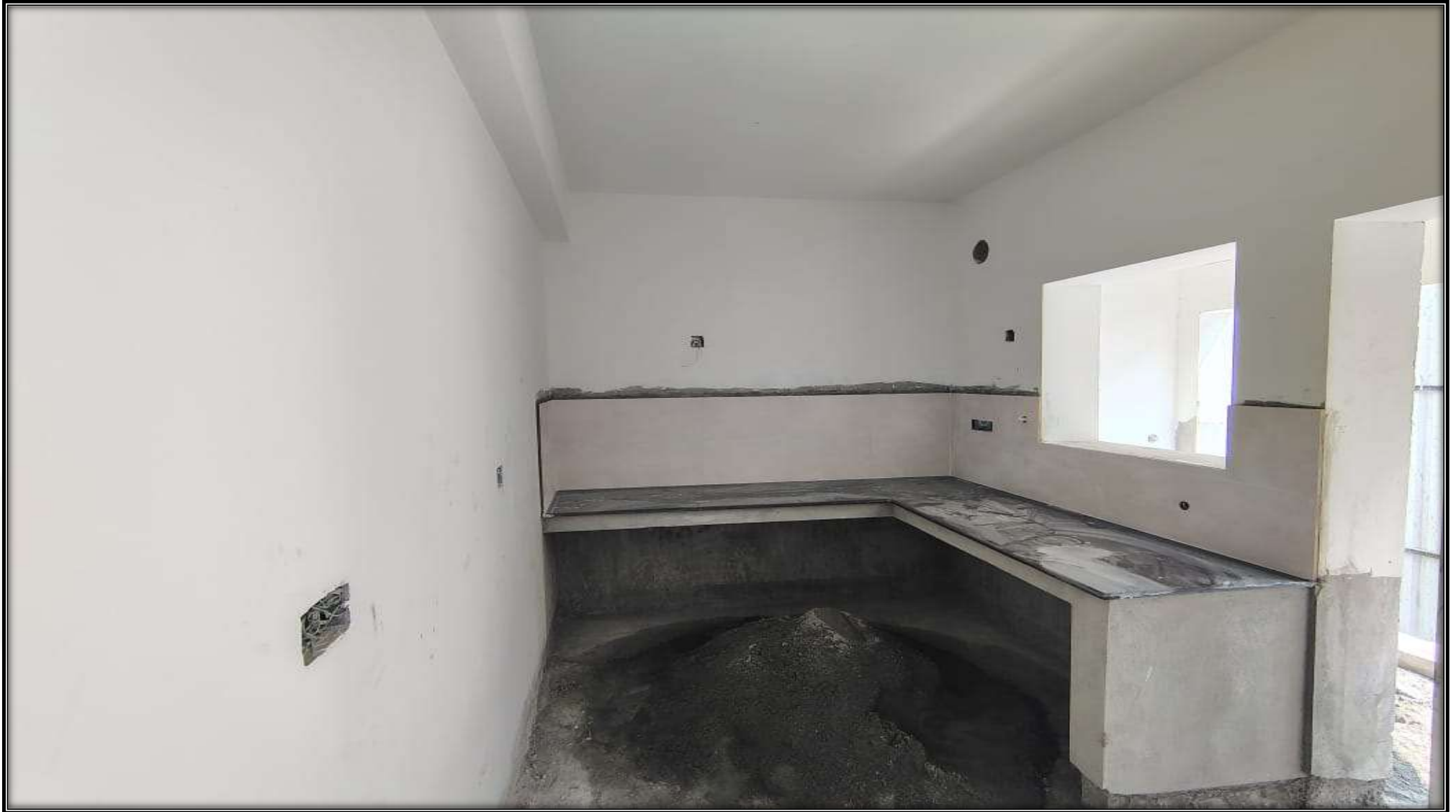
Wing 3D, 2 nd Floor – Kitchen Dado Works in Progress
