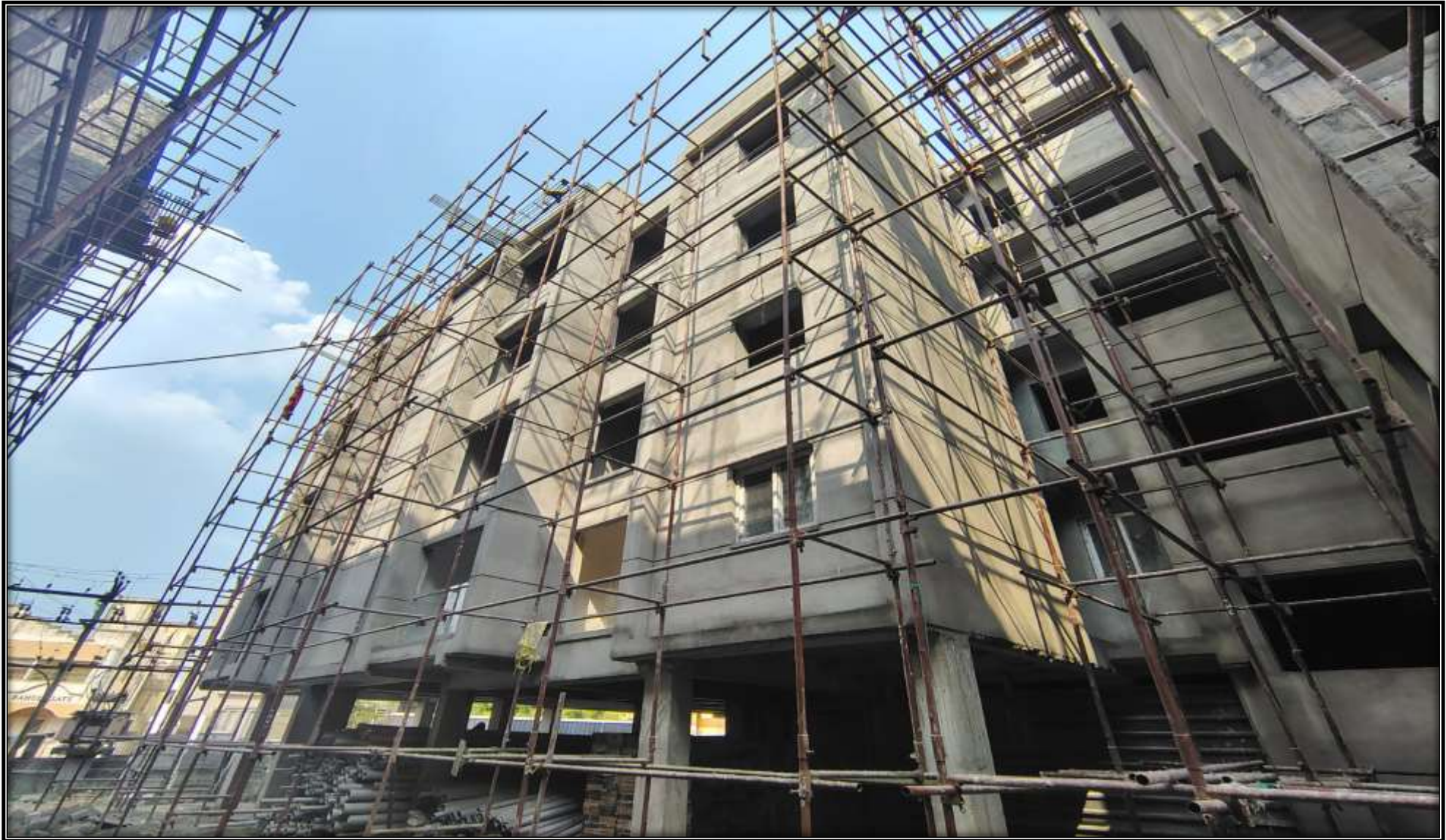
Wing 3A – West Elevation View
