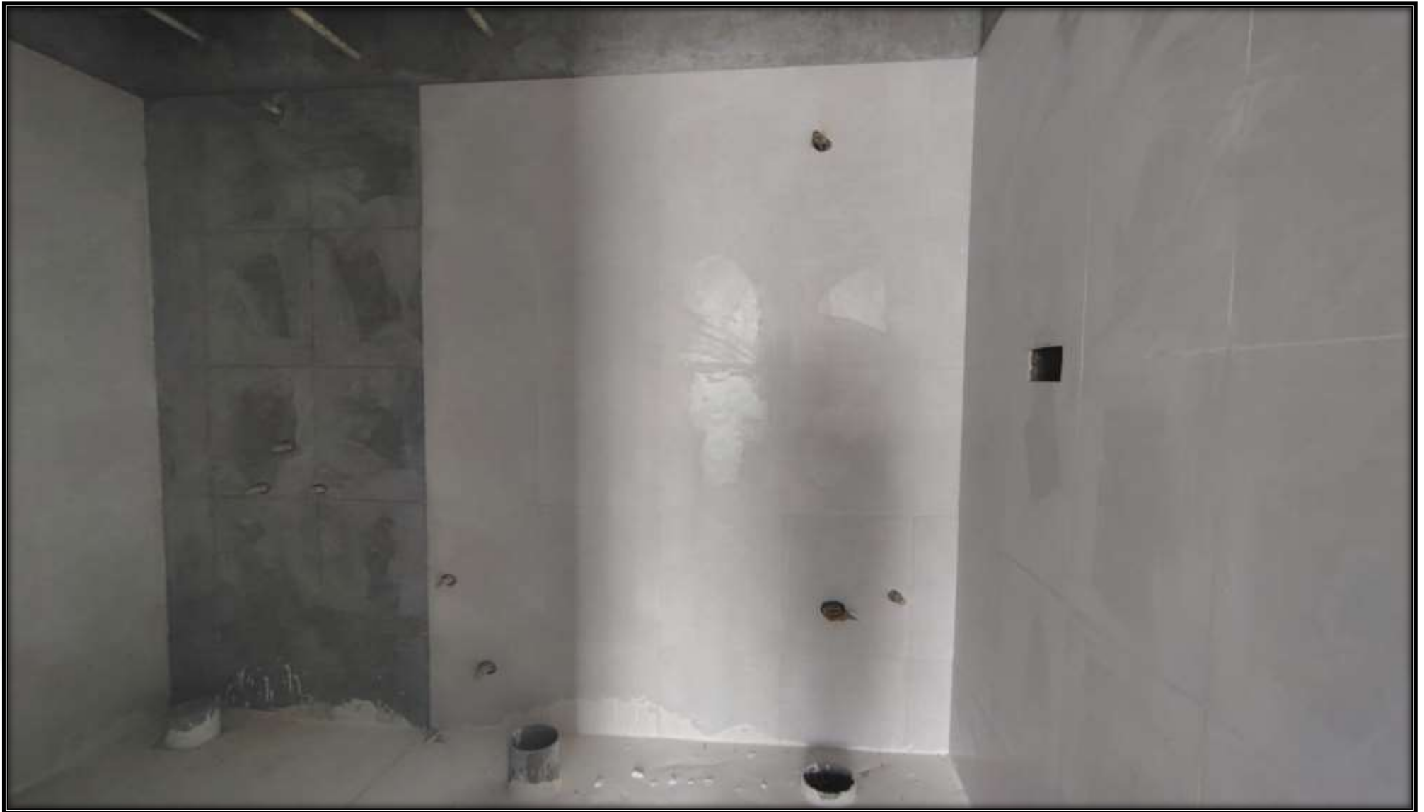
Wing 3C, 2 nd Floor – Toilet Tile works in Progress
