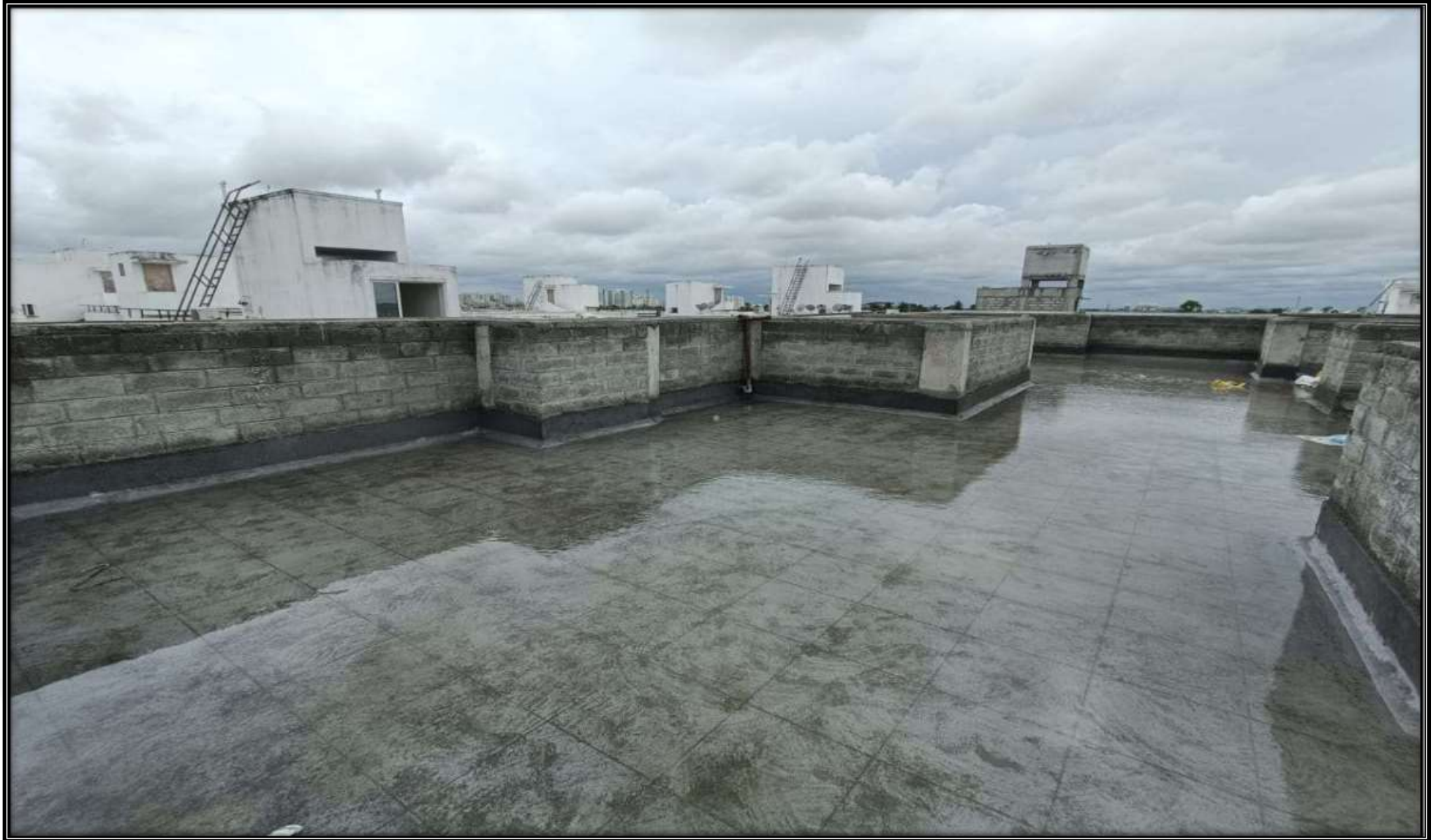
Wing 3C, 3D & 3E – Terrace Water Proofing Works Completed
