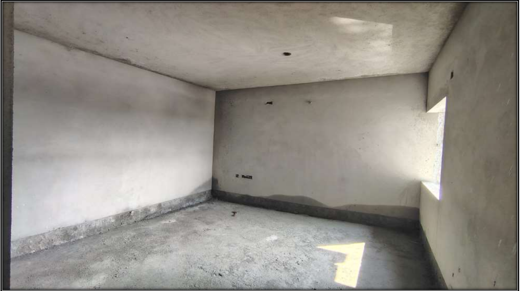
Wing 4A & 4B, 3 rd Floor - Plastering Works in Progress
