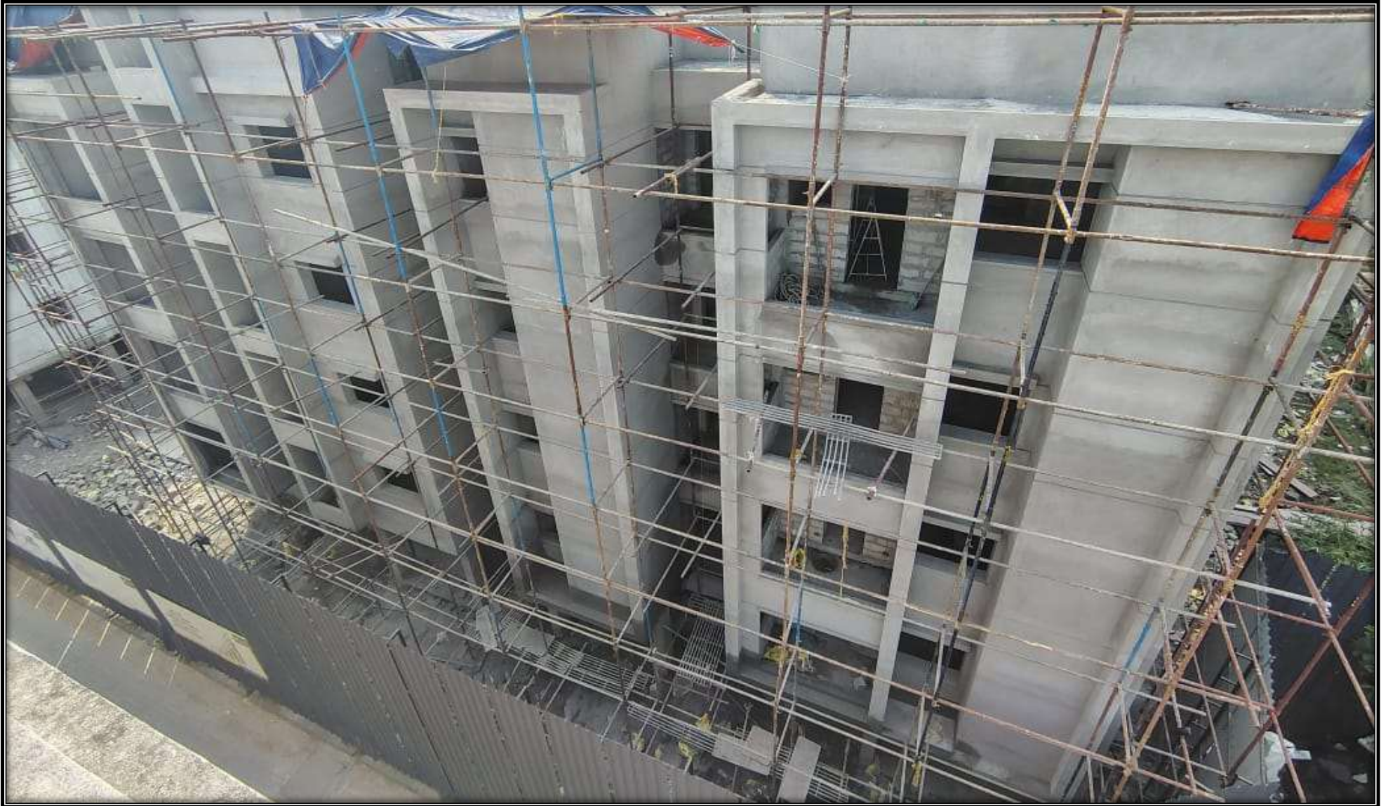
Wing 3B – East Elevation View
