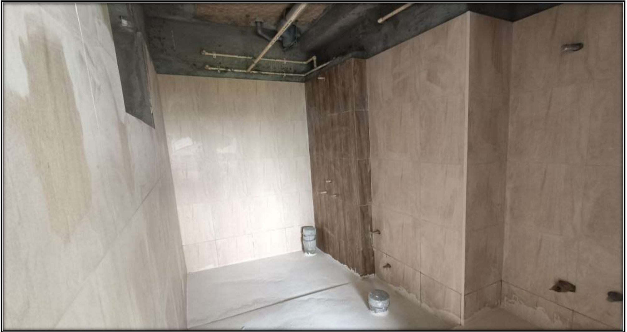
Wing 3D, 4 th Floor – Toilet Tile Works in Progress
