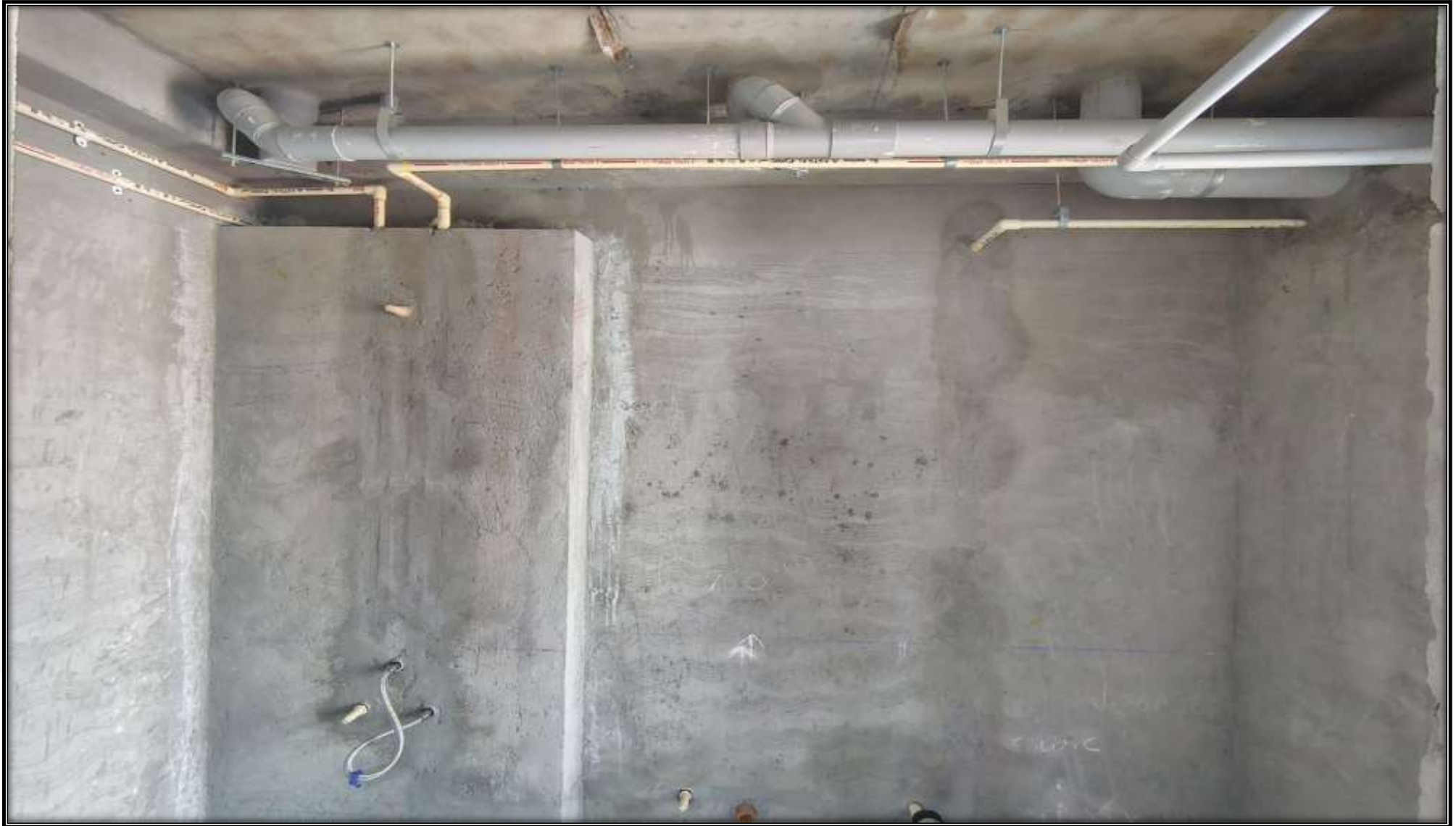
Wing 3C, 3 rd Floor – Toilet Ceiling Suspended Line works in Progress
