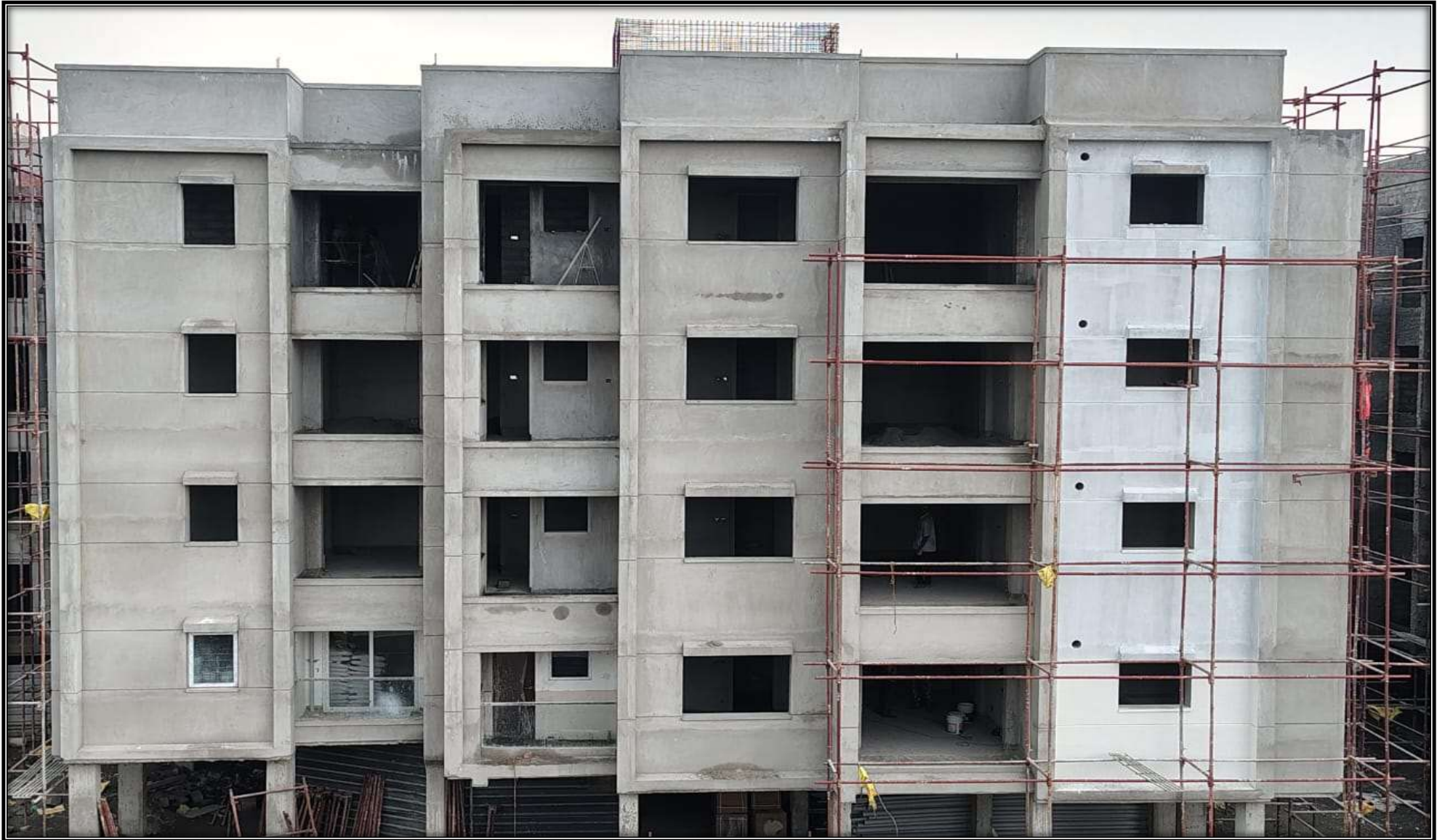
Wing 3A – North Elevation View
