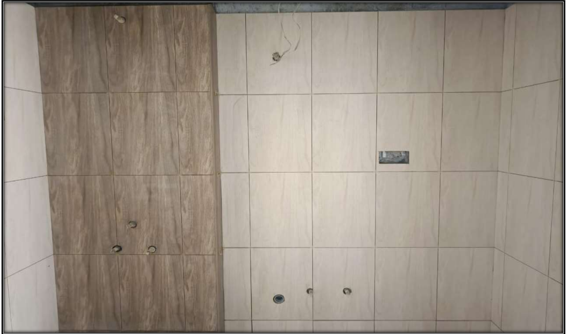
Wing 3E, 3 rd Floor – Toilet Tile Work in Progress
