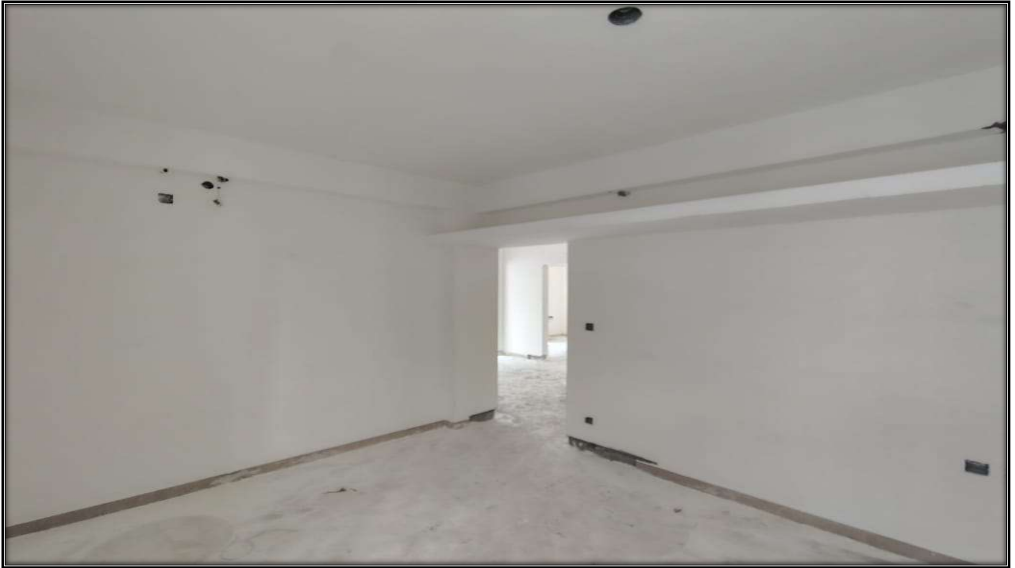
Wing 3D, 2 nd Floor – Wall & Ceiling Sanding Works in Progress
