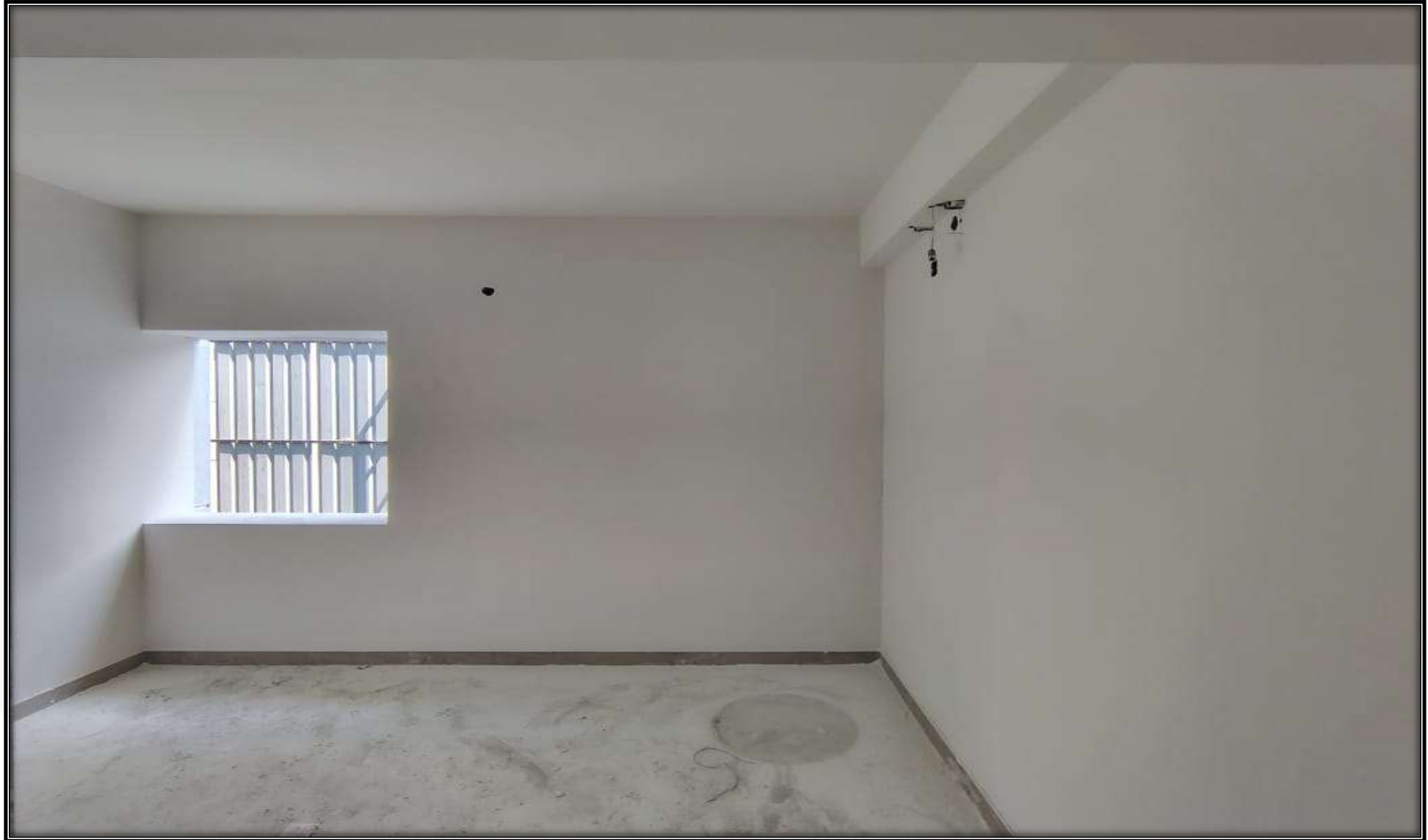
Wing 3E, 2 nd Floor – Ceiling & Wall Sanding Work in Progress
