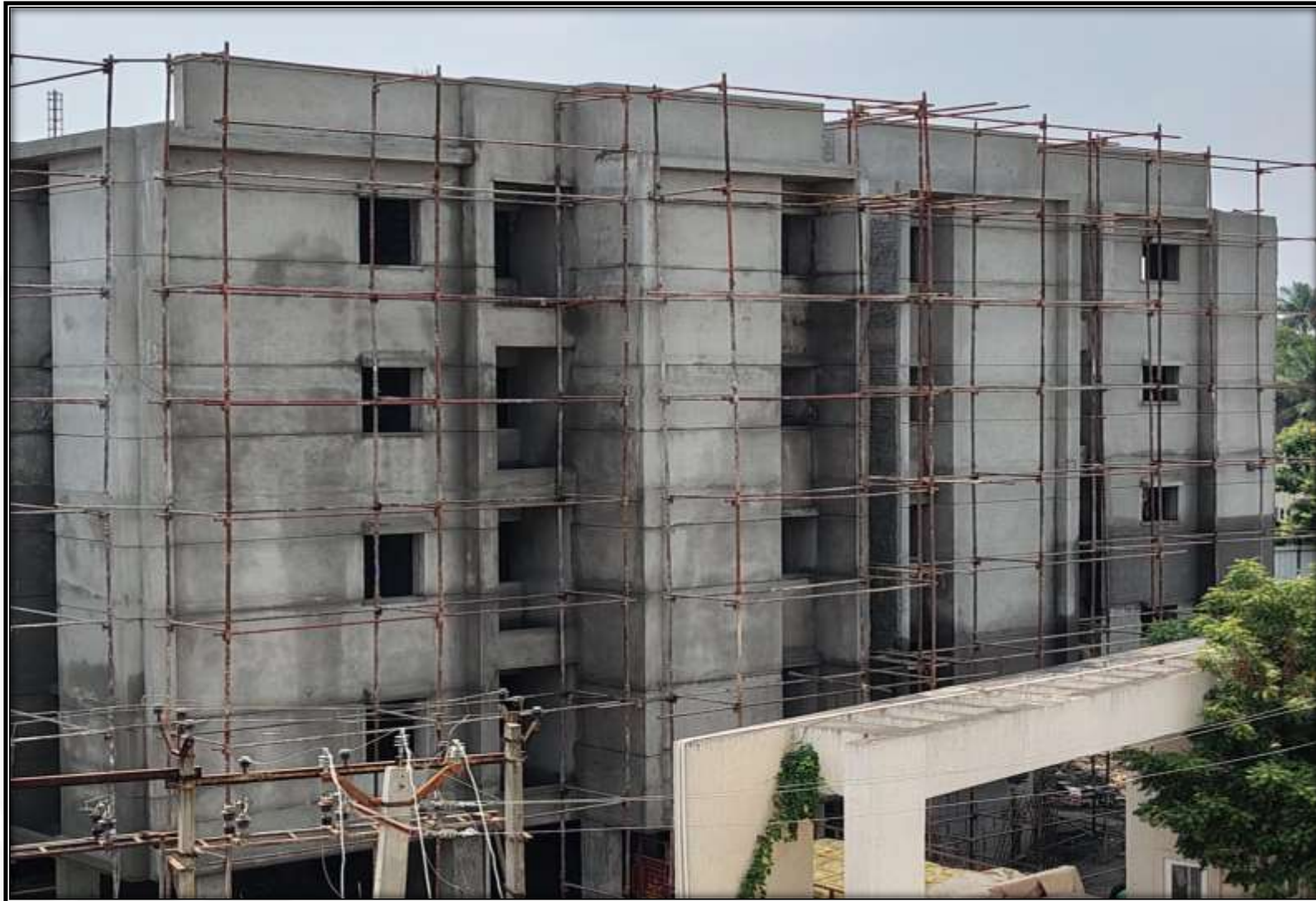
Wing 4A – North Elevation View
