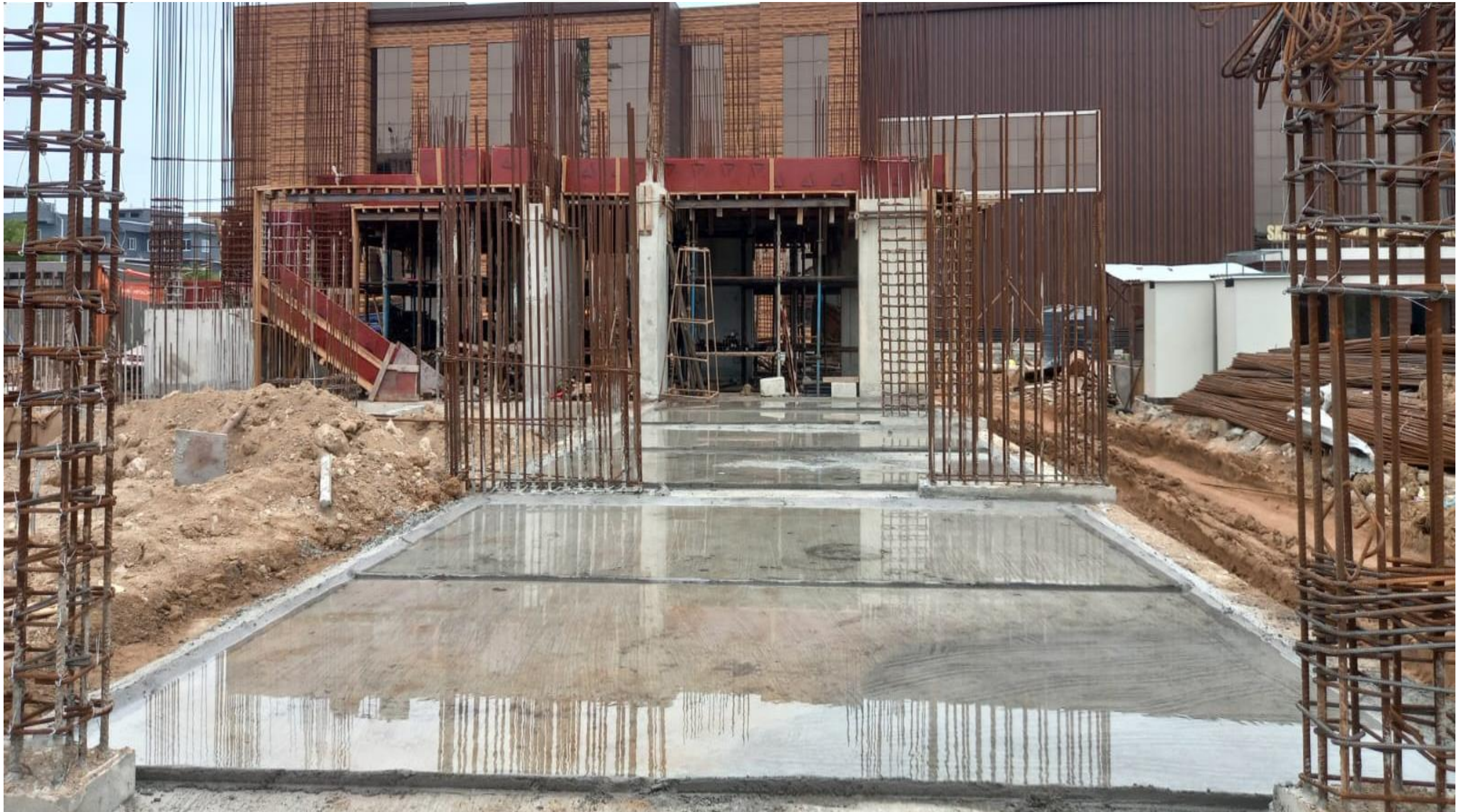
BLOCK 2 – STILT FLOOR PCC (POUR 1) IN PROGRESS.
